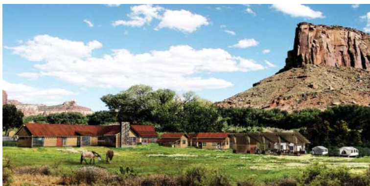
Figure 1. Scenes of the new Canyonlands Research Center environment and facilities as rendered by the designer for the completed center, and under construction. Photos: B. Baker, Drawing, CRSA Architecture.
