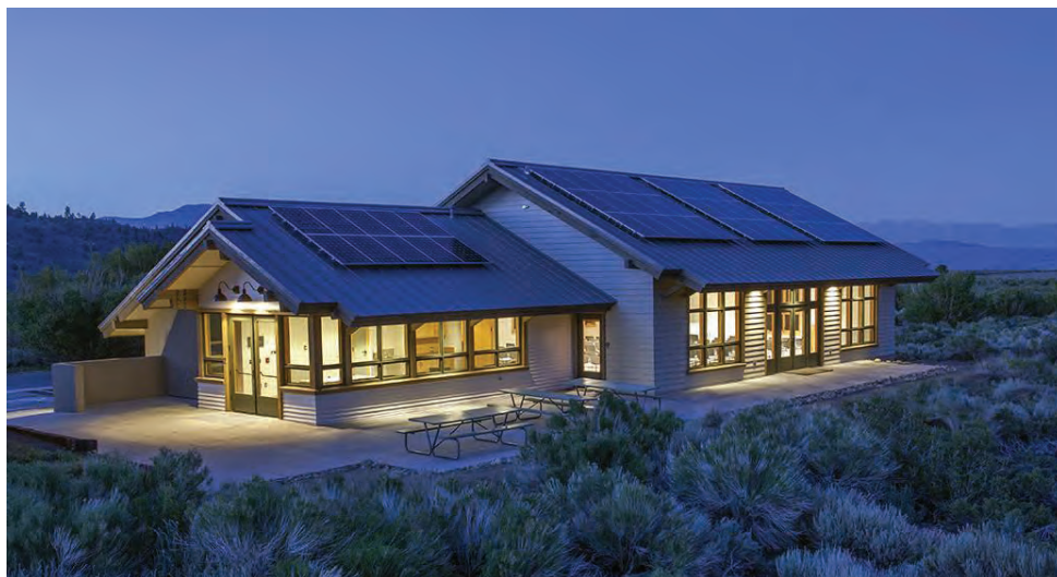
Figure 6. The new Page Center
