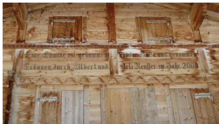
Figure 14 Inscription on chalet: “An avalanche came and took our hut [chalet] from us. Rebuilt by Albert and Heli Keuffer in the year 2000.
