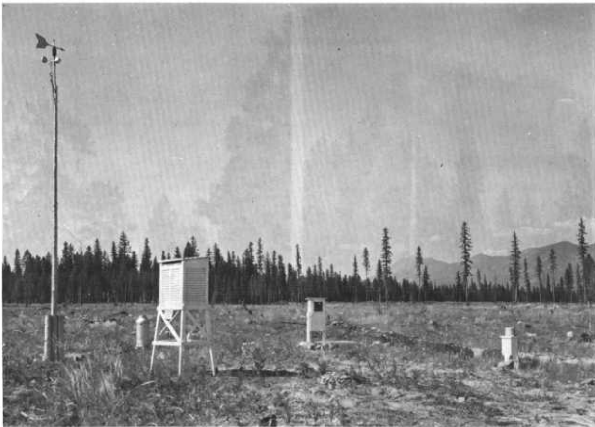
Figure 8.4. — A standard anemometer installation 20 feet above open, level ground.
