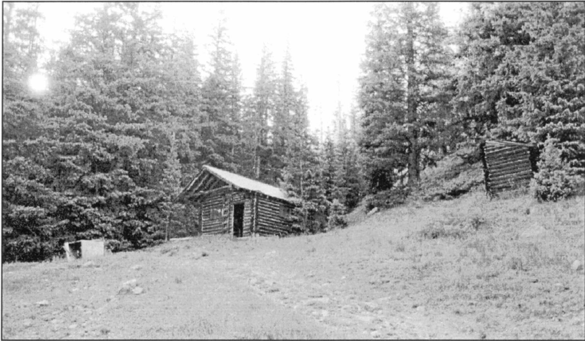
Figure 145 McCormick Cabin View to the Northwest. Outhouse to the right.
