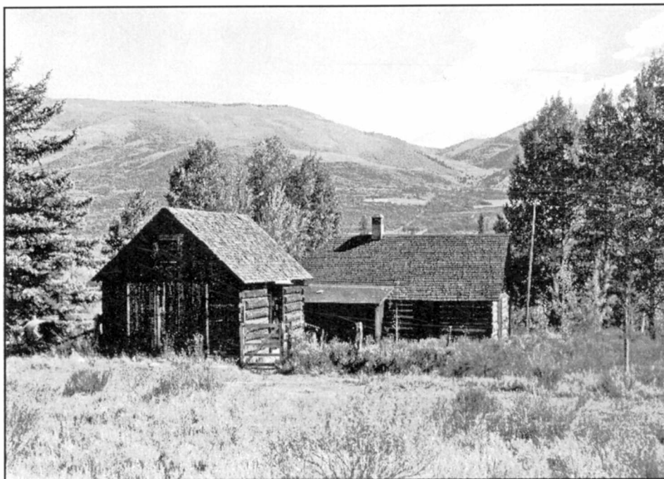
Figure 163 Cayton Guard Station Dwelling in background
