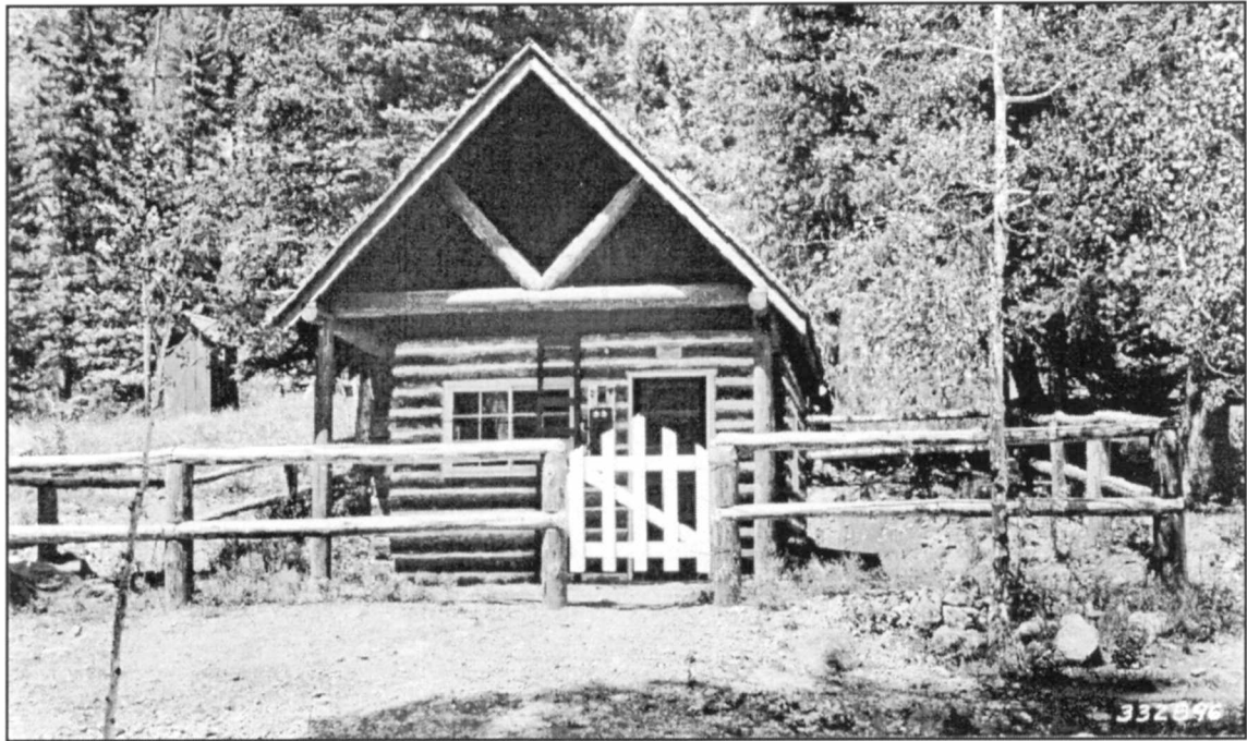
Figure 150 Front View of Silver Falls Ranger Station
