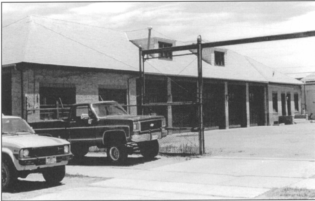
Figure 73 Gunnison Garage View to the Northeast
