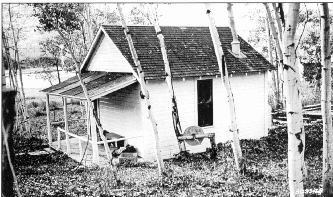
Figure 167 Lily Lake Ranger Station Dwelling, Side View
