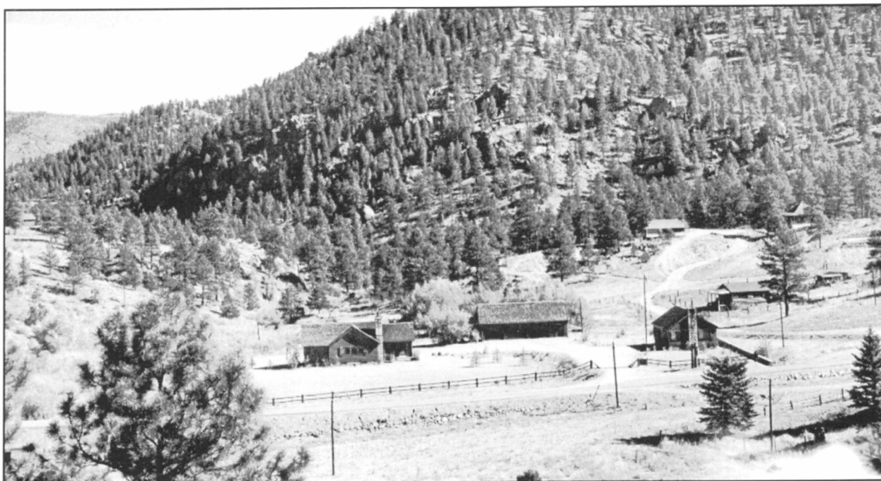
Figure 81 Buffalo Creek Ranger Station from the west
