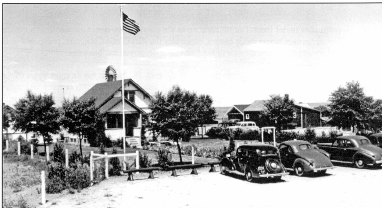
Figure 56 Briggsdale Work Center View to the Northwest
