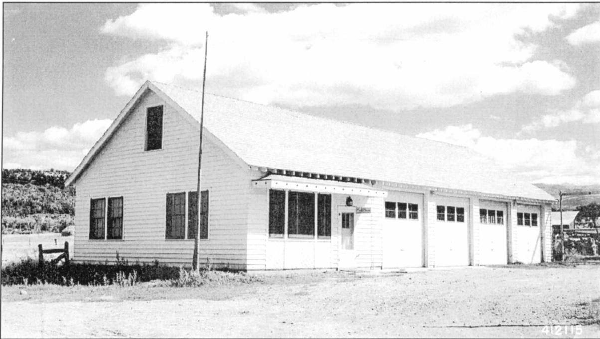
Figure 143 Ranger's Office and Garage Building Located in Mancos, Colorado.
