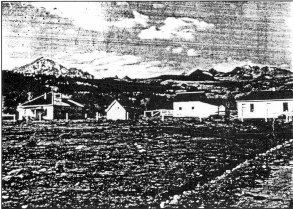
Figure 178 Slate Creek Ranger Station Barn and shed in background
