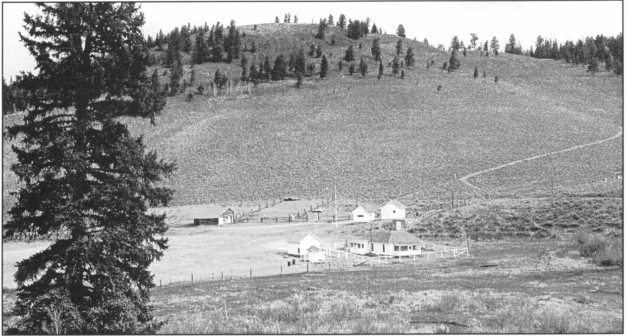
Figure 74 The Long Branch Ranger Station Building Group Located Near Sargents, Colo.
