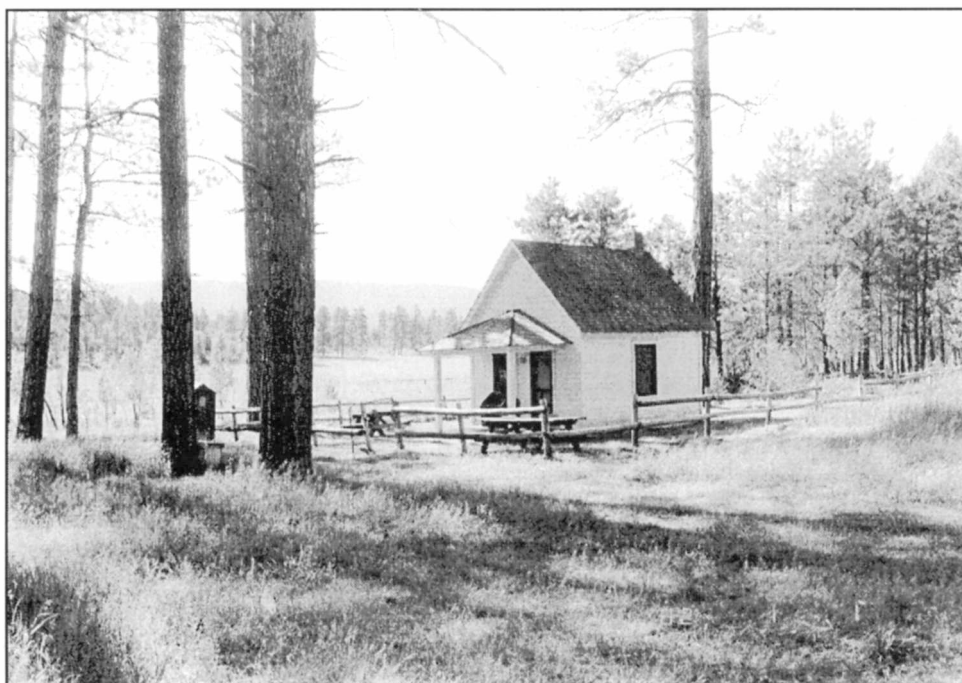
Figure 154 Turkey Springs Guard Station View to the Northwest
