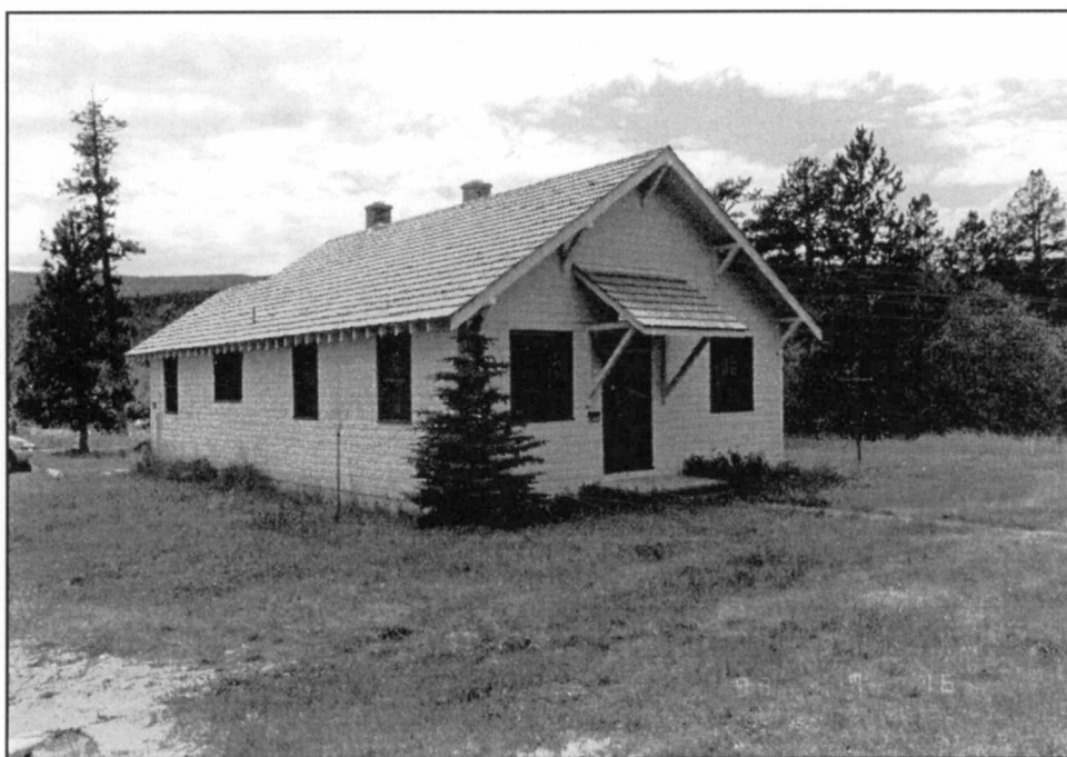
Figure 51 Buckhorn Work Center View to the Southwest
