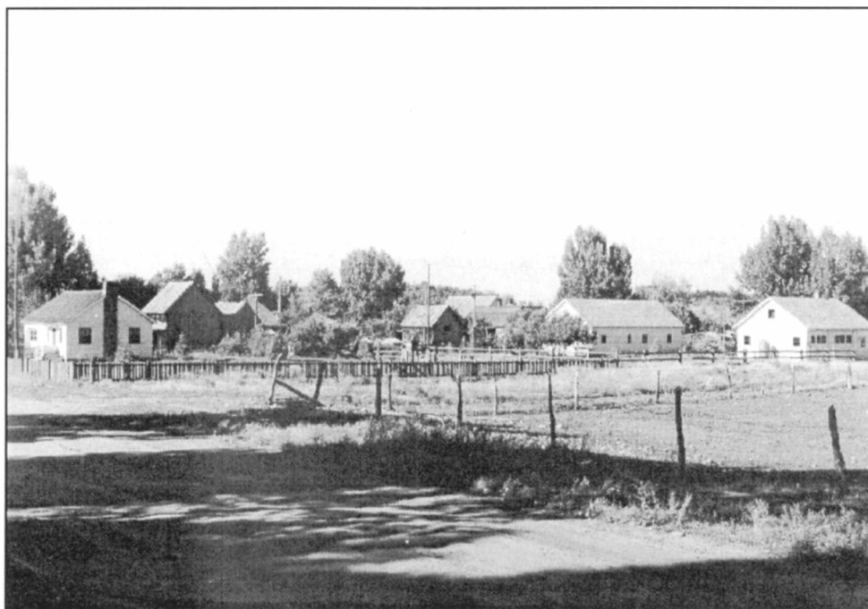
Figure 132 Bayfield Ranger Station Site in Bayfield
