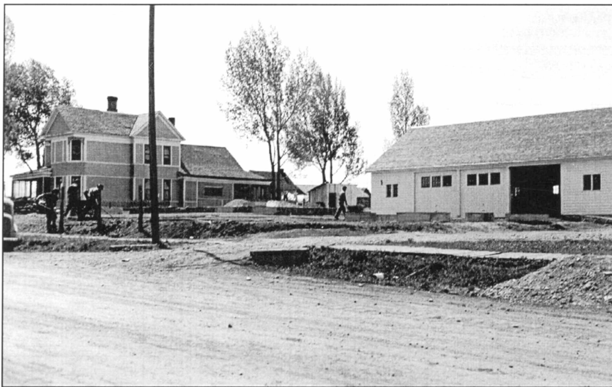
Figure 29. Norwood Ranger Station under construction. USFS Rocky Mountain Region Office. Garage to right.
