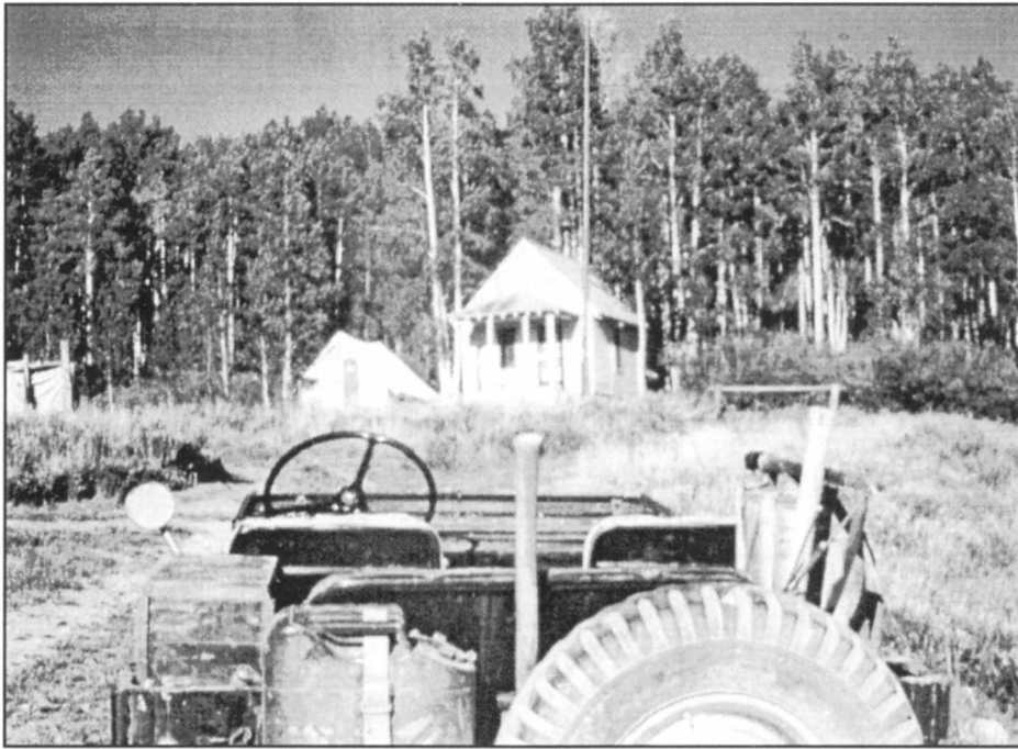
Figure 115 California Park G.S. with Prefab Sections Under Tarps for Remodeling
