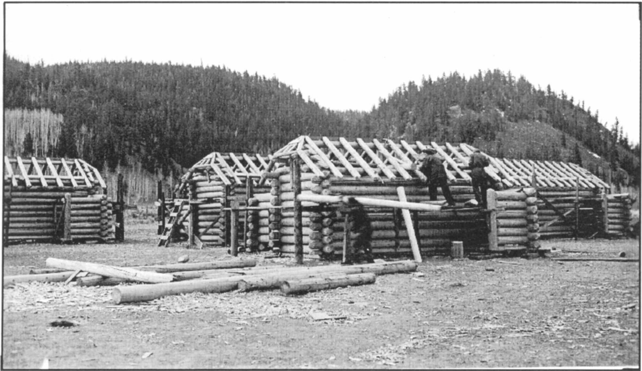
Figure 7. CCC Enrollees at Camp F-49-C Constructing Latrines. Photo taken April 1940 by J.C. Higgins. Rio Grande National Forest Supervisor's Office.
