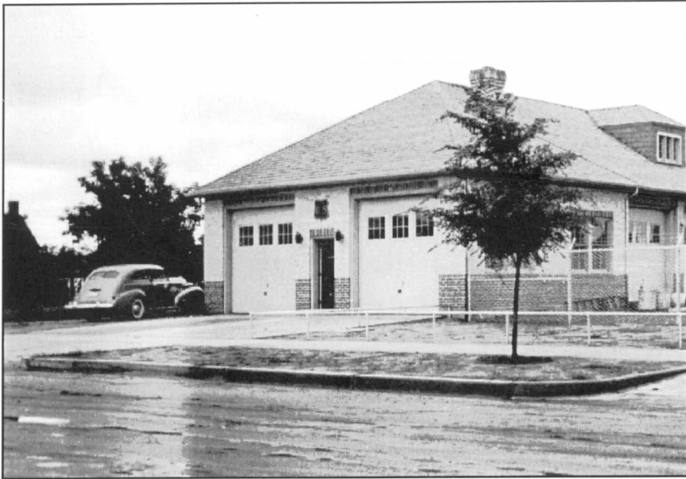
Figure 85 Colorado Springs Garage Pike National Forest
