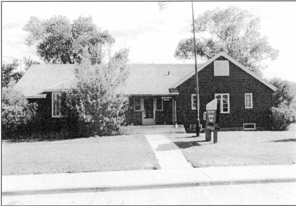
Figure 161 Carbondale Ranger Station Dwelling View to the South
