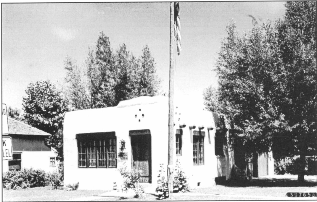
Figure 84 Office, District Ranger San Isabel National Forest
