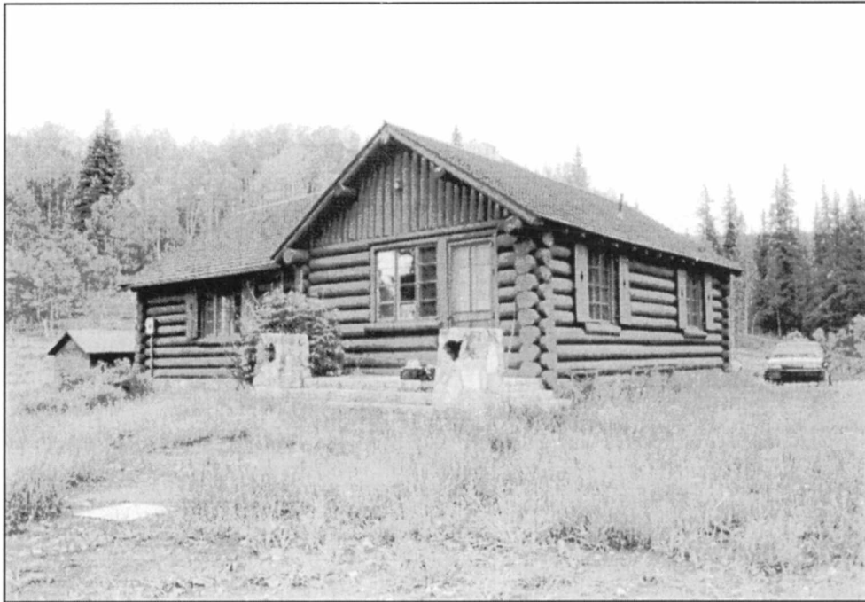
Figure 136 Dunton Guard Station View to the Northwest
