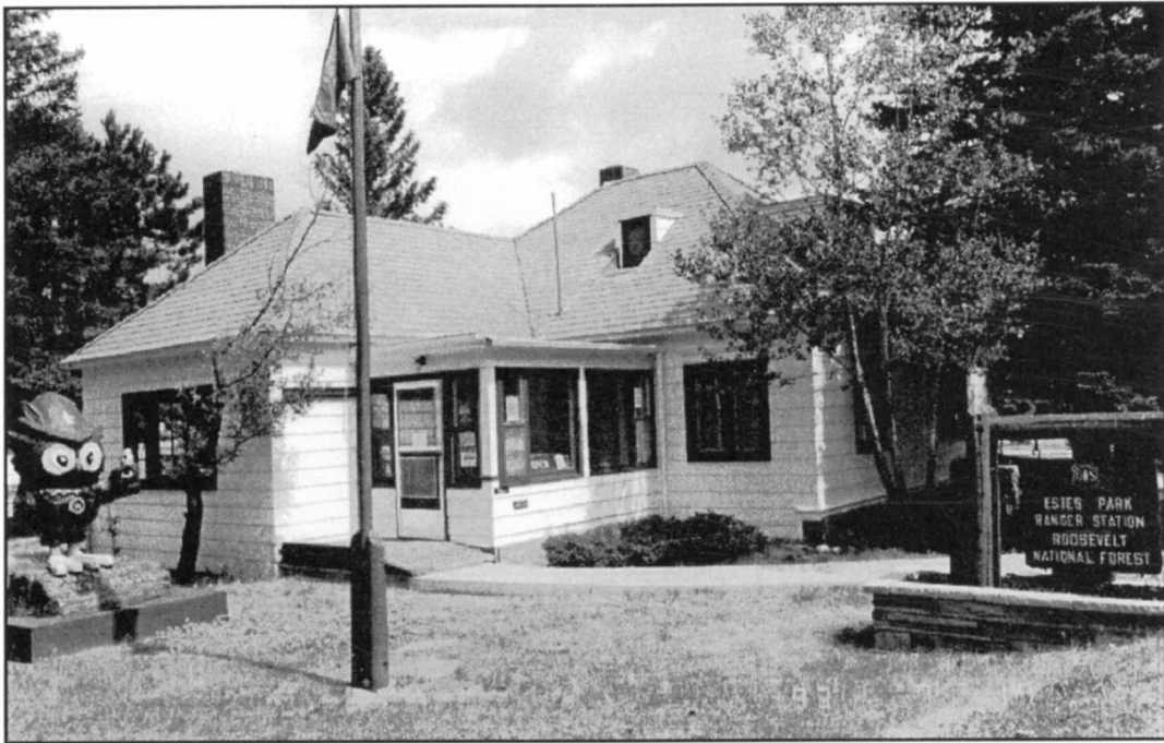
Figure 52 Office/Former Dwelling View to the North
