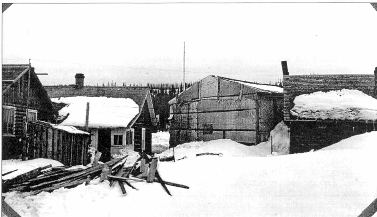
Figure 5. Construction at Mesa Lakes with Emergency Relief Administration (ERA) Camp. Photo # 398193 taken February 1940 by H.P. Gaylor. GMUG National Forests Supervisor's Office. Note garage enclosed by tent.
