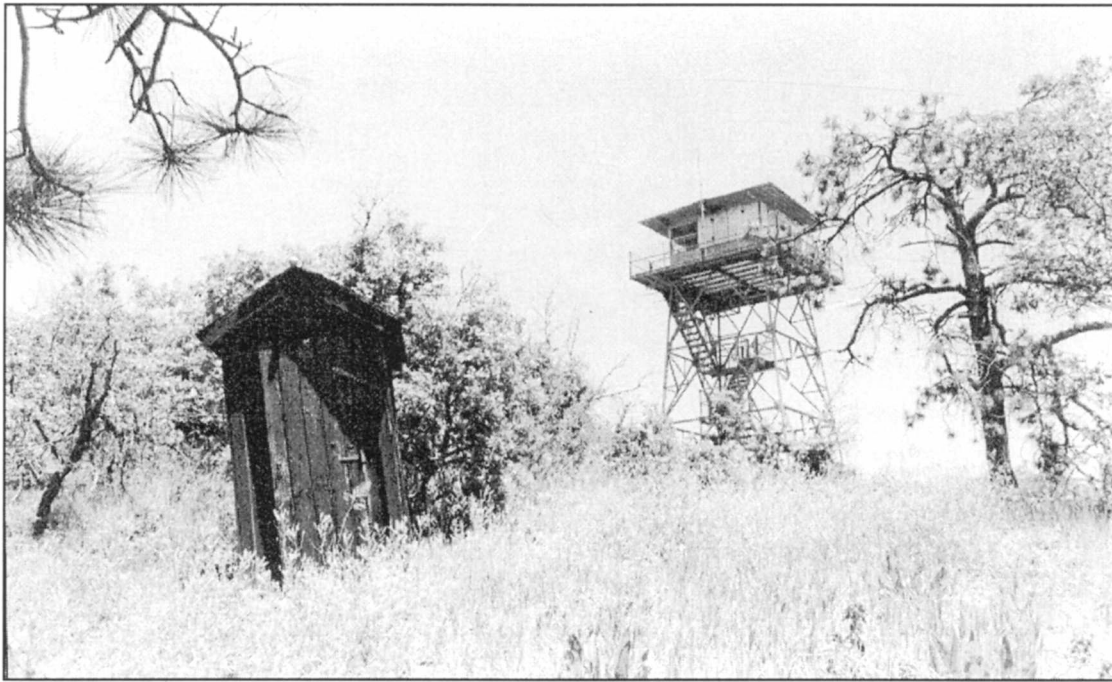
Figure 139 Eight Mile Lookout Tower View to the North
