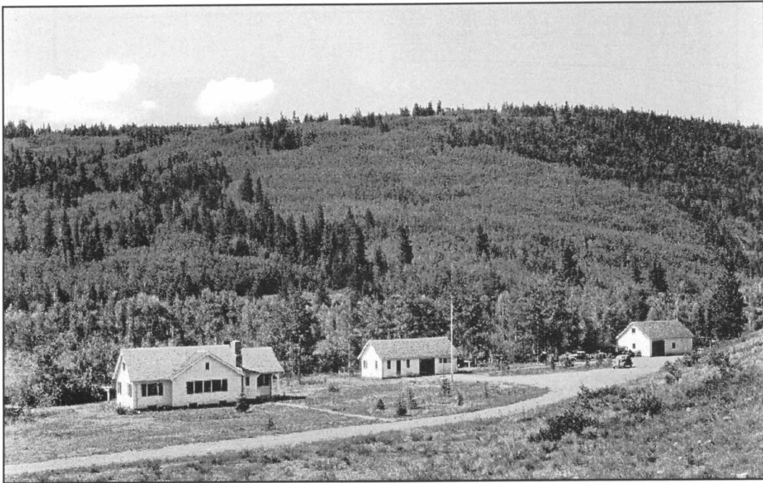
Figure 108 River Springs Ranger Station View to the Southwest
