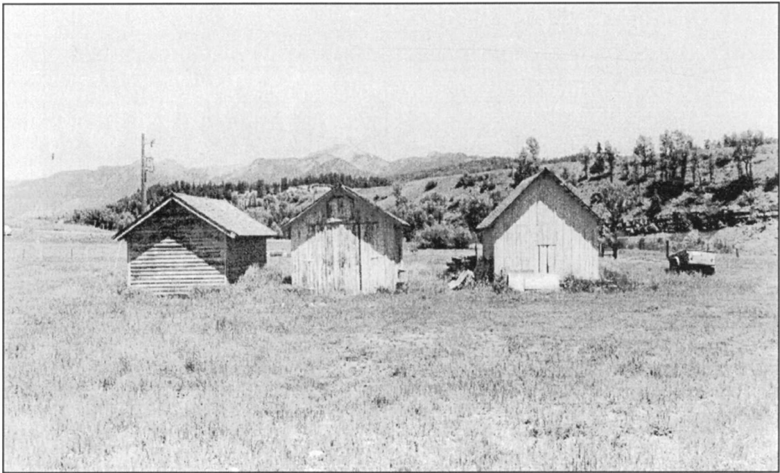
Figure 148 Piedra Guard Station View to the Southwest
