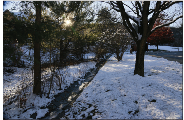
Figure 2.27. View looking southwest at the stone gutter on the east side of the parking lot.. (OCLP 2022, IMG_1901)
