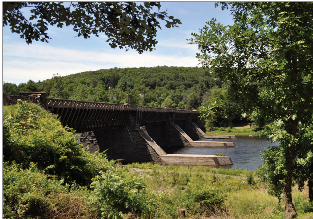
Figure 0.3. View looking southwest at Roebling's Delaware Aqueduct. (OCLP 2016, DSC_0392)
