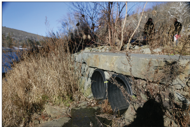
Figure 2.12. A two-pipe culvert is located under the aqueduct/bridge and empties stormwater from the original canal. (OCLP 2022, IMG_1847)
