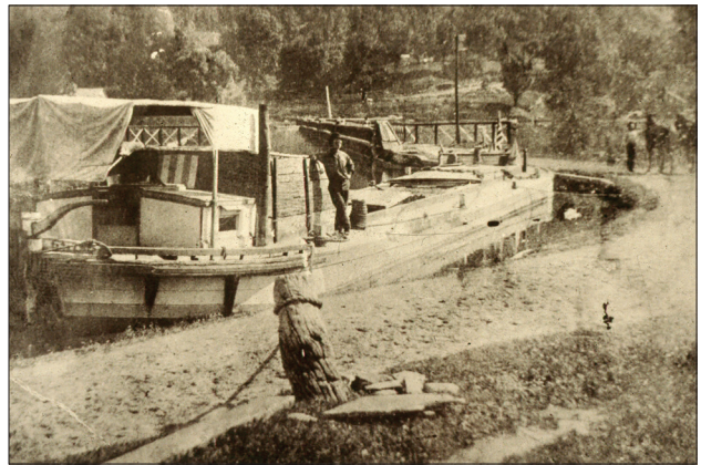
Figure 3.4b. View looking east at the turning basin on the Pennsylvania side, 1849-1898. Note the earthen tow path and the wood bollard to tie up boats. (UPDE Archives, PA_Scan4)
