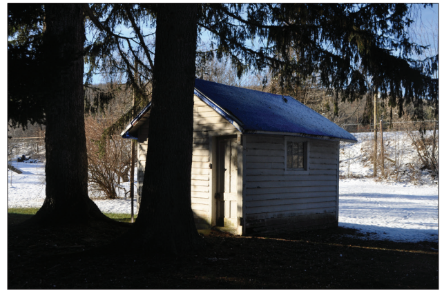
Figure 2.50. View looking southwest at the coal shed. (OCLP 2022, DSC_7367)
