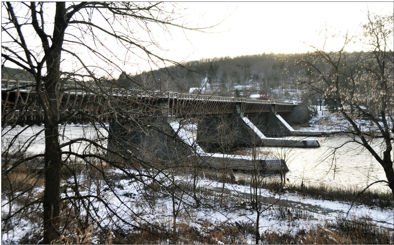
Figure 2.1. View looking south from the New York side parking lot to the upstream side of Roebling's Delaware Aqueduct. (OCLP 2022, DSC_7492)
