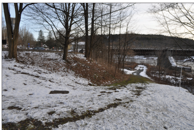
Figure 3.2e. View looking south at the Maintenance Access Road as it descends to the Towpath Trail under the aqueduct/bridge. (OCLP 2022, DSC_7498)
