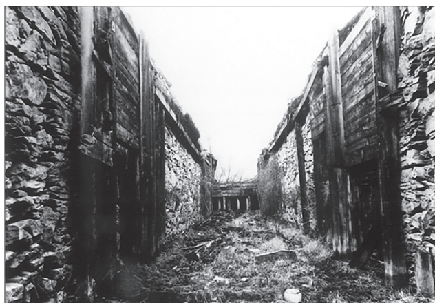
Figure 1.33. View looking northwest at Lock 71 in 1923. (Minisink Valley Historical Society, #P-82-8-6)
