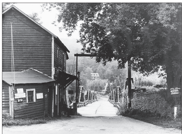
Figure 1.52. View looking west at the toll house and the aqueduct/bridge, c.1968. The toll gate is a simple hinged horizontal crossbar (shown here in a raised position). (Historic American Engineering Record, HAER PA-1, 1968, #140680pv)
