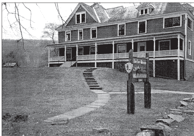
Figure 1.67. Zane Grey House and Museum and its sign, 1999. Note also the bluestone walkway and brick and bluestone steps. (O'Donnell et.al., Cultural Landscape Treatment Plan [CLPT] for the Zane Grey Property, Lackawaxen, Pennsylvania. Prepared for the National Park Service, Upper Delaware Scenic and Recreational River, Lackawaxen, Pennsylvania, 1999: 47)
