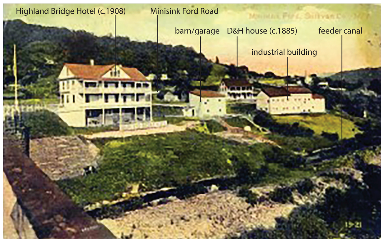
Figure 1.31. View looking southeast at lands on the New York side, south of the aqueduct, 1921. The hotel, barn/garage, and likely an industrial building crowd the hill above the old feeder canal and towpath. (UPDE Archives, 1921_minisinkford-300x184)
