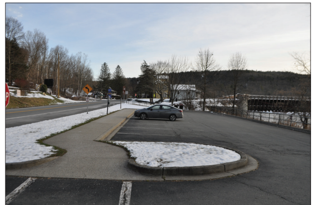
Figure 2.16. View looking southeast at the parking lot and sidewalks on the New York side of the bridge/aqueduct. (OCLP 2022, DSC_7500)
