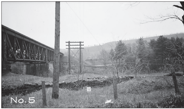
Figure 1.5. View looking south at stone walls associated with the original canal on the north side of the Lackawaxen River, 1933. (Historic American Engineering Record, HAER PA-24, 2001, #140643pv)
