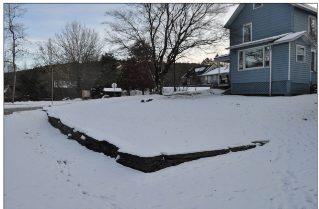
Figure 2.25. View looking south at a stone retaining wall at the Margold house. (OCLP 2022, DSC_7447)
