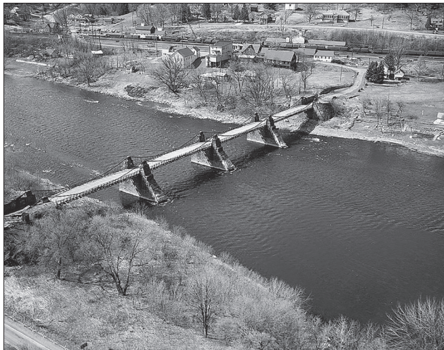
Figure 1.54. View looking southwest, c.1969. By this time the area north of the aqueduct/bridge on the New York side was filled with successional vegetation. On the Pennsylvania side, the partially wooded and partially graded vacant lot still stood between the aqueduct/bridge and development to the south. (Historic American Engineering Record, HAER PA-1, 1969, #140673pv)
