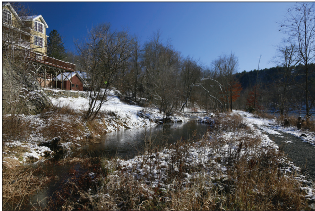
Figure 2.3. View looking southeast at the original canal prism and towpath. The river is at image right. (OCLP 2022, IMG_1848)
