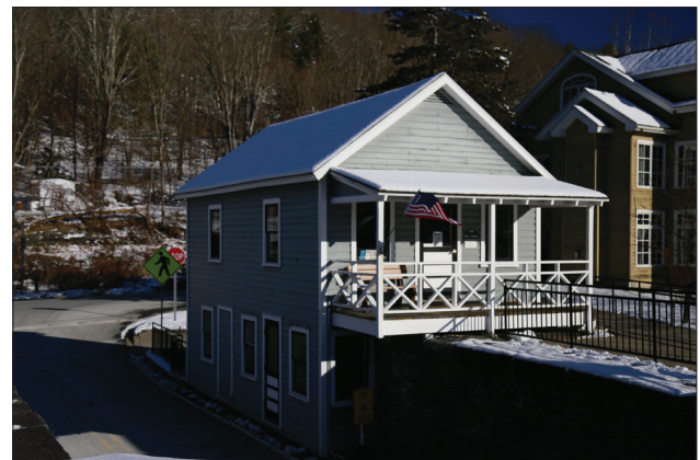
Figure 2.9. View looking west at the two-story toll house, constructed in 1908 next to the aqueduct/bridge's east abutment. (OCLP 2022, IMG_1885)
