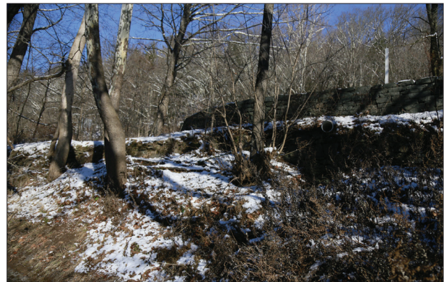
Figure 2.5. View looking west at the original towpath stone wall and a curved contemporary stone wall above it, which supports the Maintenance Access Road. (OCLP 2022, IMG_1839)
