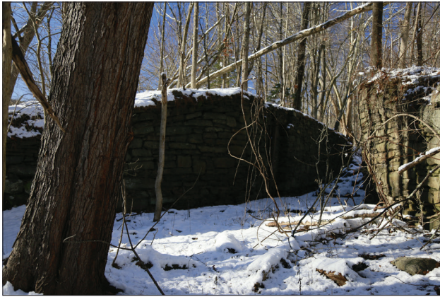
Figure 3.3c. View looking west at the new canal prism and south end of Lock 71. (OCLP 2022, IMG_1874)
