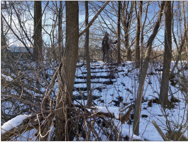
Figure 3.6o. View looking southwest at Option C, at the steps on park property that access the riverbank. (OCLP 2022, IMG_0472)
