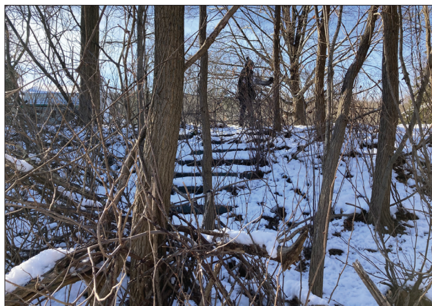
Figure 2.32. View looking southwest at remnant stone steps leading to the riverbank. (OCLP 2022, IMG_0742)
