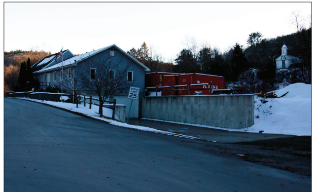
Figure 2.24. View looking south at the park's maintenance facility. (OCLP 2022, IMG_1911)
