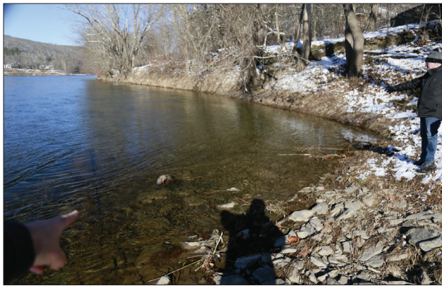
Figure 2.2a. View of parallel lengths of submerged timbers associated with a guardlock at the former entrance of the original canal. (OCLP 2022, IMG_1877)
