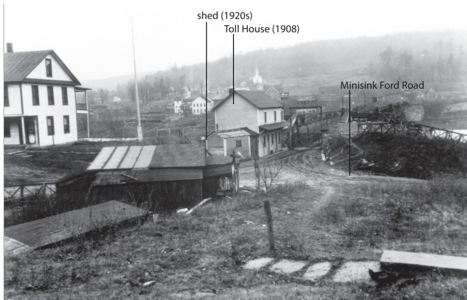
Figure 1.26. View looking southwest at the turning basin (far image left) and toll house on the New York side, 1923. The toll house was built in 1908 and a shed was added to it in the early 1920s. Note the reuse of the towpath fences at image right and left. (Delaware and Hudson Railway Company, New York State Library)
