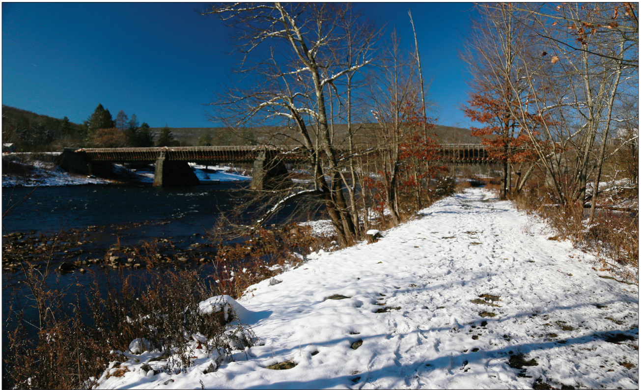
Figure 2.18a. View looking northwest from the original canal towpath to Roebling's Delaware Aqueduct. (OCLP 2022, IMG_1851)
