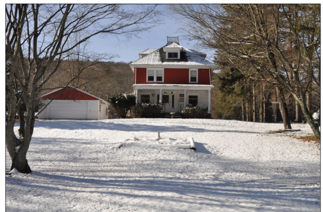
Figure 2.29. View looking southwest at the Cortright house. (OCLP 2022, DSC_7443)
