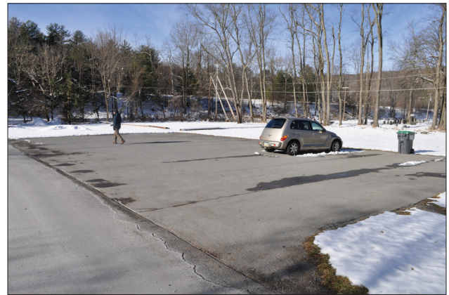
Figure 2.41. View looking west at the Roebling Inn parking lot. (OCLP 2022, DSC_7435)
