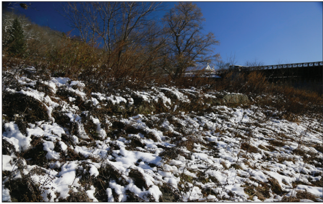
Figure 2.6. The top of a partially hidden section of stone wall associated with the original canal prism or towpath. (OCLP 2022, IMG 1841)
