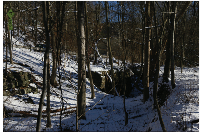
Figure 3.3f. View looking east at the new canal prism and north end of Lock 71. (OCLP 2022, IMG_1880)
