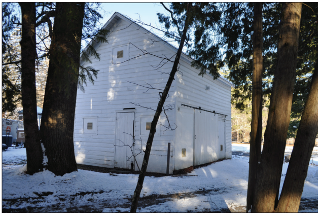
Figure 2.49. View looking northwest at the barn. (OCLP 2022, DSC_7368)
