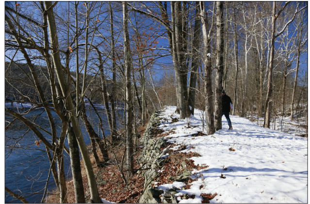
Figure 2.7. View northwest at a stone wall supporting the original canal towpath. (OCLP 2022, IMG_1867)
