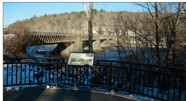
Figure 3.5a. View looking north at Roebling's Delaware Aqueduct from the overlook. (OCLP 2022, IMG_1899)
