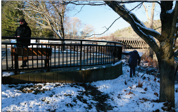
Figure 2.30. View looking north at the paved overlook on the Pennsylvania side of the bridge/aqueduct. (OCLP 2022, IMG_1900)
