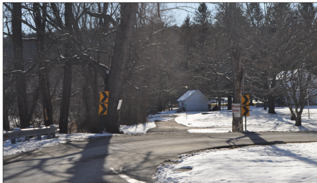
Figure 2.31. View looking southeast at the road providing access to the Brown Keller house. (OCLP 2022, DSC_7427)
