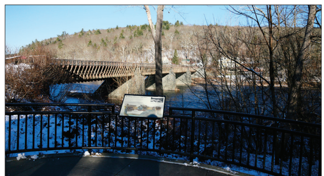
Figure 2.34. View looking north at Roebling's Delaware Aqueduct from the overlook. (OCLP 2022, IMG_1899)
