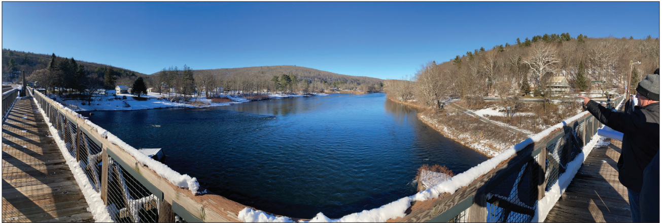
Figure 2.2. Panoramic view from the aqueduct/bridge's upstream towpath, traces of the slackwater dam are still visible in normal river level conditions (ripples, image left). (OCLP 2022, IMG_0740)
