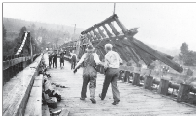
Figure 1.47. View looking west at the removal of the aqueduct/bridge trunk walls, c.1931. (UPDE Archives, Scan168)
