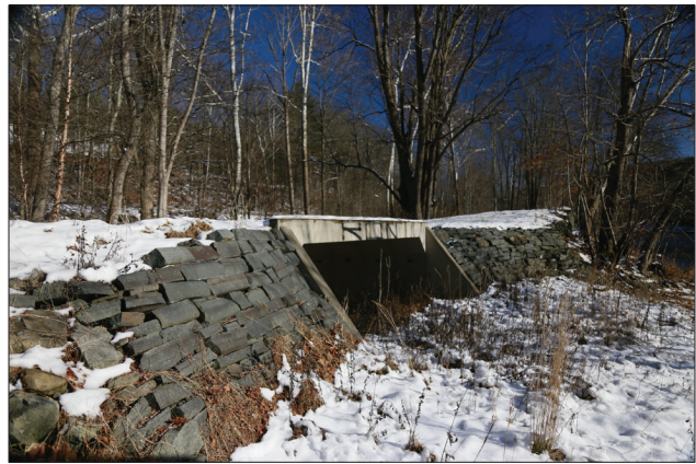
Figure 2.13. A concrete box culvert on the Towpath Trail spans the breach in the original canal and also serves as a footbridge. (OCLP 2022, IMG_1858)
