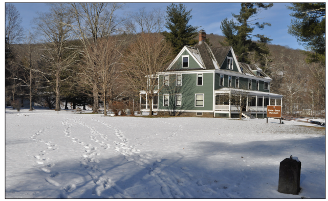
Figure 3.11b. View looking northwest at the former garden plot area. (OCLP 2022, DSC_7457)
