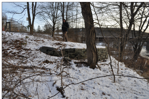
Figure 3.2d. View looking southeast at the contemporary retaining wall that supports the Maintenance Access Road. (OCLP 2022, DSC_7495)
