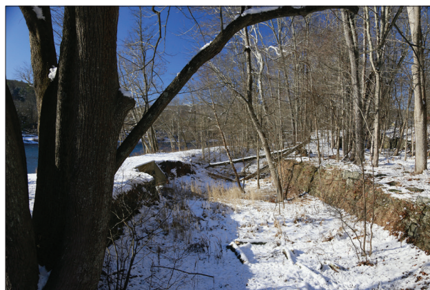
Figure 3.1e. View looking west at woody vegetation in the canal prism and on the new canal towpath (image right). (OCLP 2022, IMG_1868)
