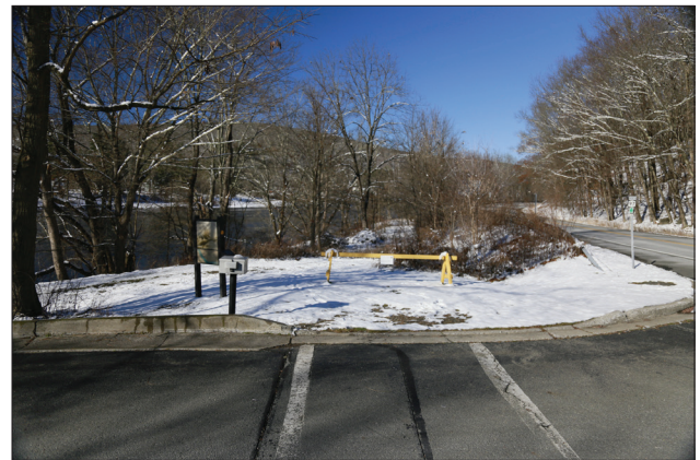
Figure 3.2a. View looking northwest at the upper end of the Maintenance Access Road, where it meets the parking lot on the New York side of Roebling's Delaware Aqueduct. (OCLP 2022, IMG_1824)
