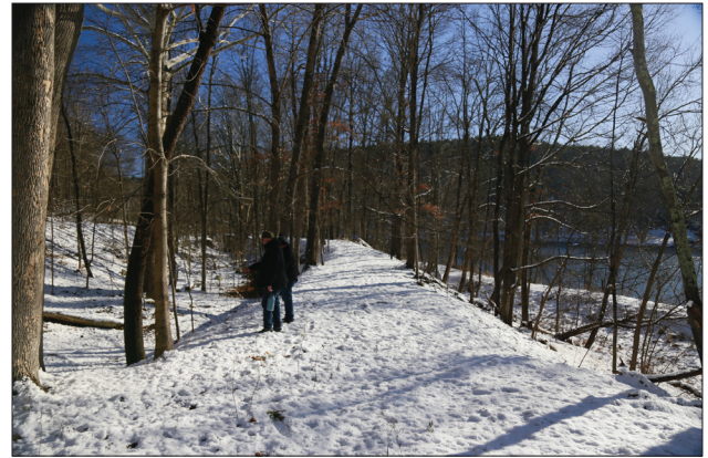
Figure 2.15. View looking south at the new canal towpath, located north of Lock 71. The new canal is at image left and the original canal and towpath are down the hill at image right. (OCLP 2022, IMG_1881)
