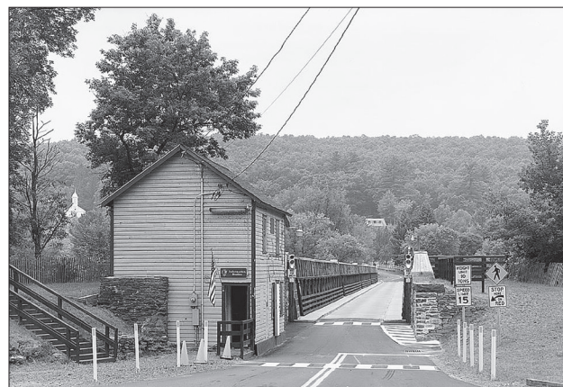
Figure 1.65. View looking west at the tollhouse and former aqueduct after it reopened to vehicular traffic, c.1988, before the towpaths were reconstructed in 1994. (Historic American Engineering Record, HAER Addendum PA-1, 1988, #123818pv)
