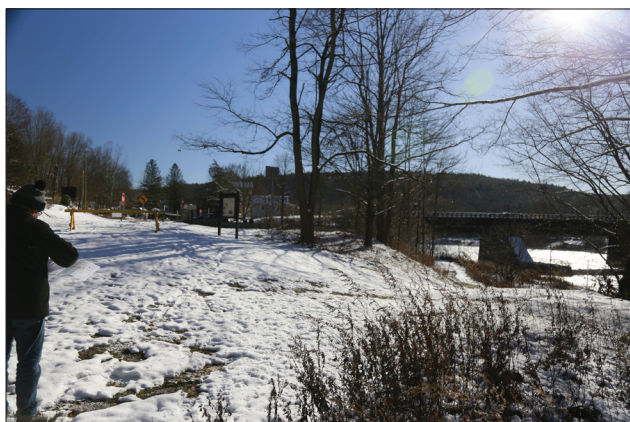
Figure 3.2c. View looking southeast at the sharp turn of Maintenance Access Road, from the former Emergency Access Road. (OCLP 2022, IMG_1826)
