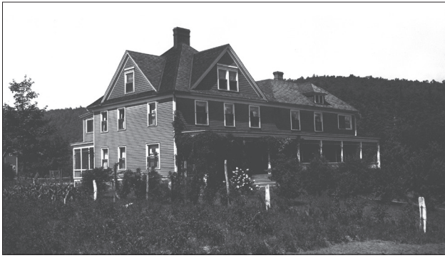
Figure 1.41. View looking northwest at the “Big House,” c.1916-18, after north additions were built. Note the vegetable garden plot in foreground, front walk shrubs, and vines on the porch. (Courtesy Ohio Historical Society, from CLPT 1999: 21; Hawley Public Library, #1604)
