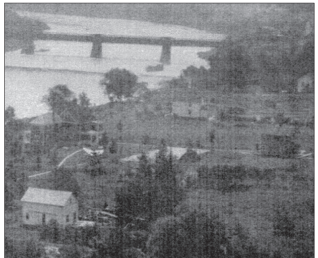
Figure 3.12a. Portion of photograph looking from Prospect Rock, c.1918. The light colored rectangular area (image center) west of the Zane Grey house may be the tennis court. ( Historic Structures Report, Alice Josephine Grey House, Barn & Accessory Buildings, Zane Grey Family Compound , 2012: 8)
