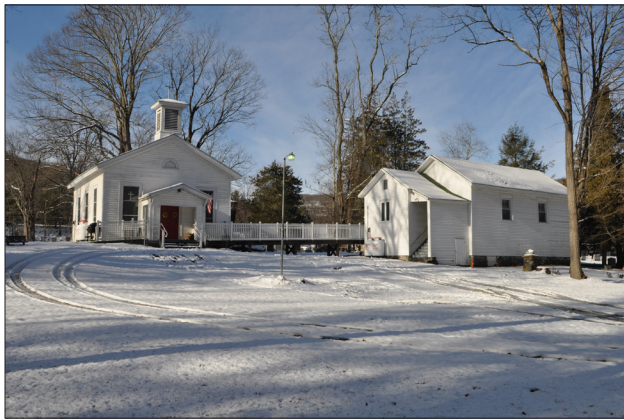
Figure 2.36. View looking west at the former St. Mark's Church (left) and social hall (right). (OCLP 2022, DSC_7423)
