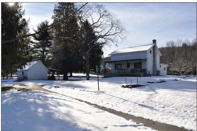
Figure 2.28. View looking south at the Brown Keller house and garage, located just north of the former canal (which was just beyond the spruce trees). (OCLP 2022, DSC_7450)
