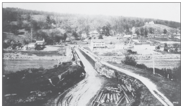
Figure 3.4c. View looking east at the former turning basin on the Pennsylvania side, after 1908. (Minisink Valley Historical Society, P-82-8-28/Delaware and Hudson Railway Company, New York State Library/Canal Society of New York State negative 10339C)
