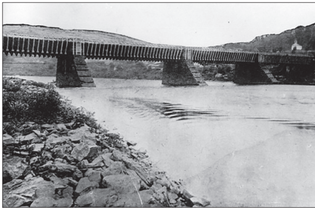
Figure 1.8. View looking southwest at the Delaware Aqueduct, 1849-1898. The west wall of the original canal on the New York side is in the foreground. (UPDE Archives, NY_Image 4-11B)
