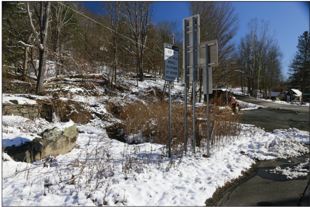
Figure 2.14. View looking west at the former turning basin site and remnant canal and towpath stone walls. (OCLP 2022, IMG_1813)
