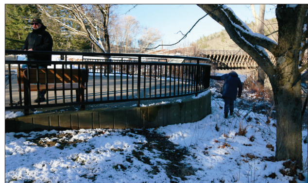
Figure 3.5b. View looking northwest at the overlook. Note the tilt of the overlook. (OCLP 2022, IMG_1900)
