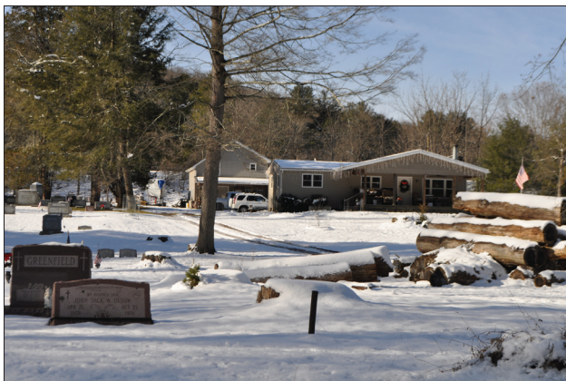
Figure 2.37. View looking west at the buildings on the George property. (OCLP 2022, DSC_7402)
