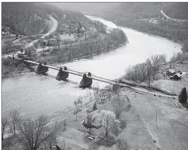
Figure 1.55. View looking southeast, c.1968. Note the dense vegetation on the New York side south of the aqueduct/bridge. On the Pennsylvania side north of the aqueduct/bridge, the former canal bed and towpaths (image lower right) have been leveled to the surrounding grades. A row of young trees marks the property line, which generally coincides with the outer edge of the former towpath. (Historic American Engineering Record, HAER PA-1, 1969, #140671pv)
