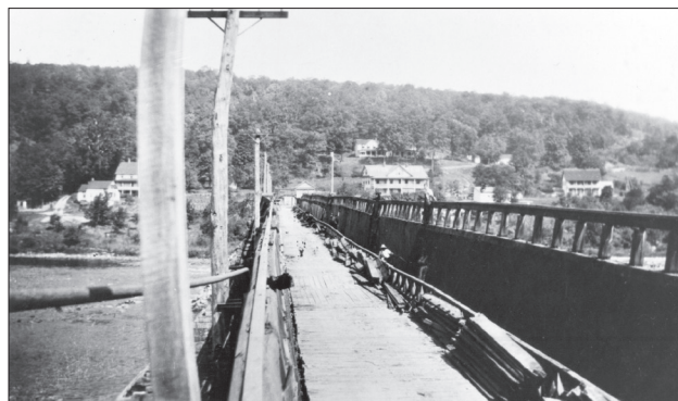
Figure 1.46. View looking east at the beginning of the project to replace the bridge deck and remove the aqueduct/bridge trunk walls, c.1931. (UPDE Archives, Scan 165)
