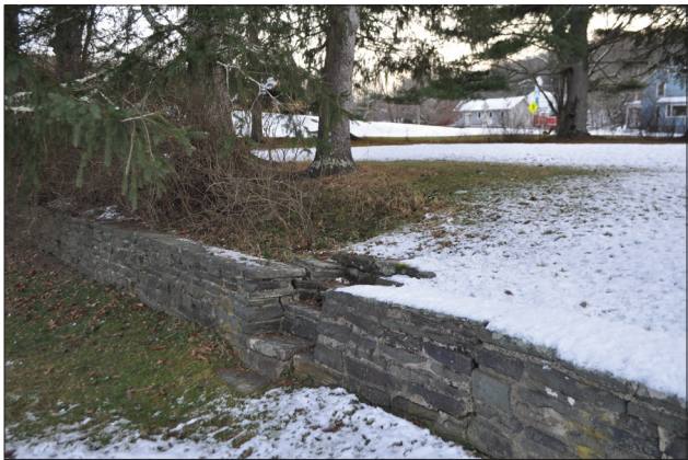
Figure 2.26. View looking south at a stone wall and steps east of the Brown Kelley garage. (OCLP 2022, IMG_1911)
