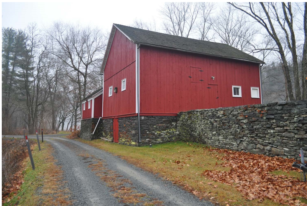
Figure 31. View looking south at the Corwin Shed (left) and Corwin Barn (right). (OCLP 2013, DSC_0695)
