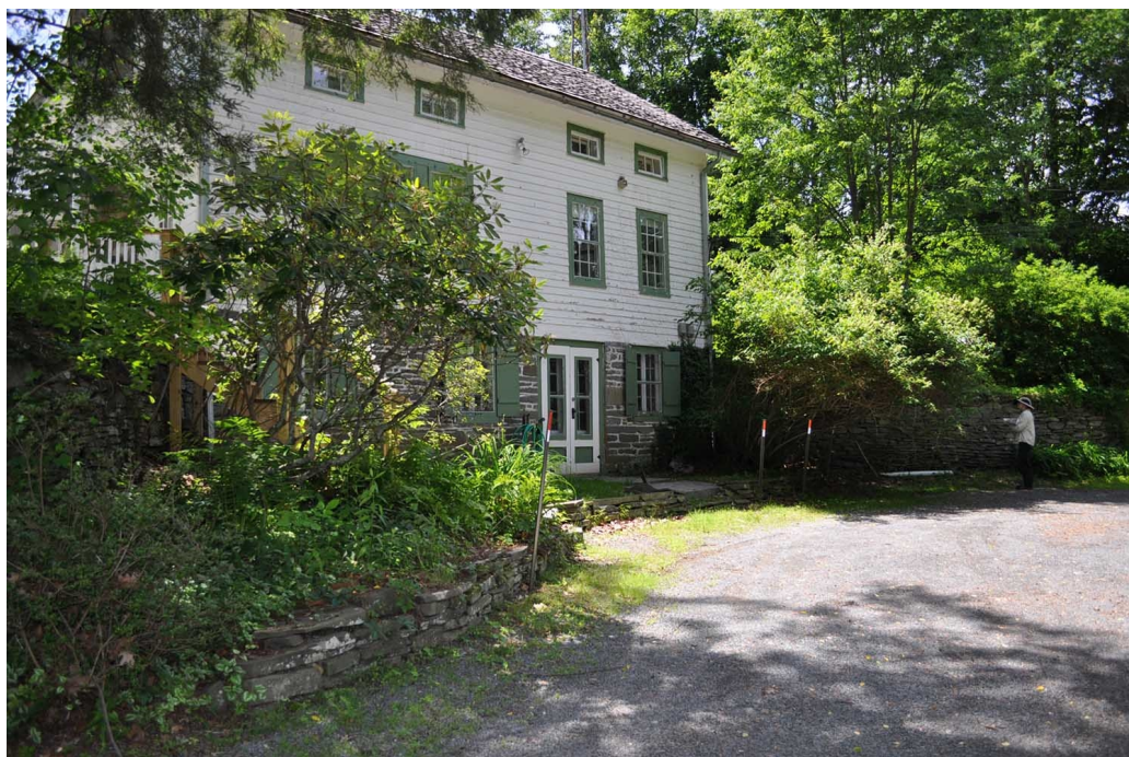
Figure 32. View looking northwest at the retaining walls on the east side of the Corwin House. (OCLP 2014, DSC_0600)
