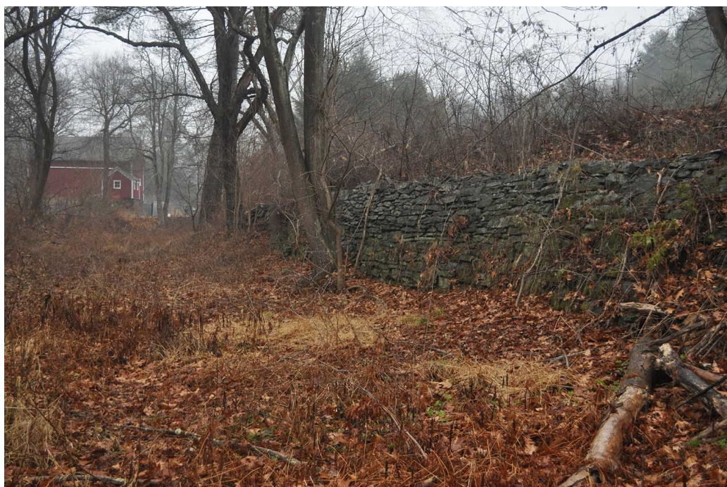
Figure 26. View looking north from at some of the retaining walls, from the canal prism. (OCLP 2013, DSC_0724)
