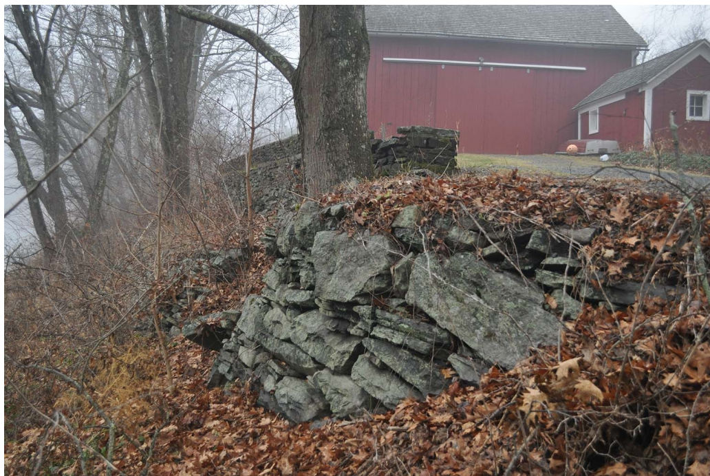
Figure 23. View looking northwest at successional vegetation and stone retaining walls along the bluff. (OCLP 2013, DSC_0704)
