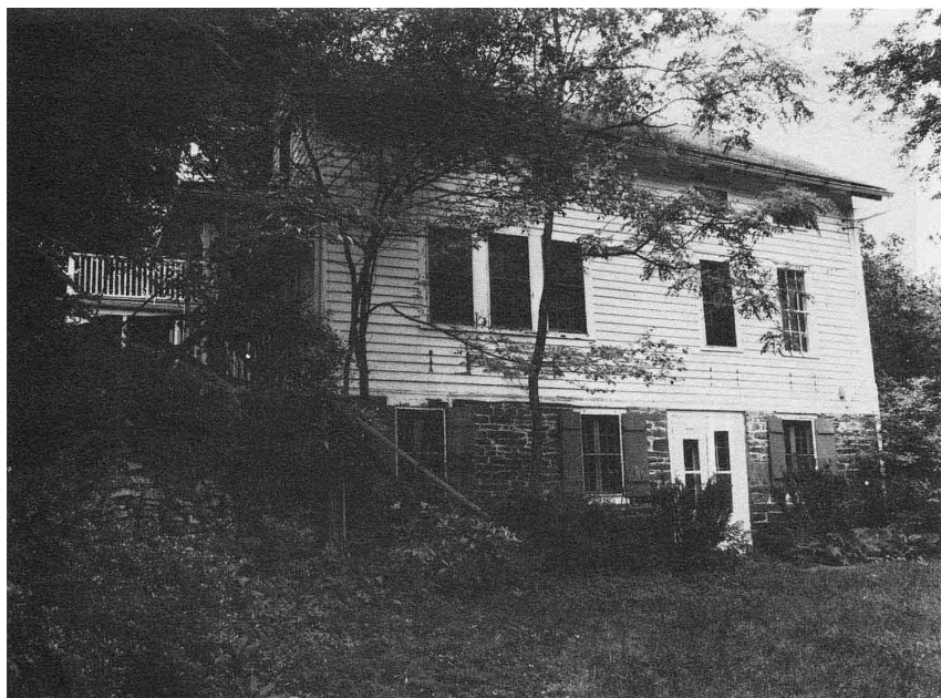
Figure 9. View of the east side of the Corwin House in c.1980. (Dekin, Cultural Resources Survey 1983: 6-201)
