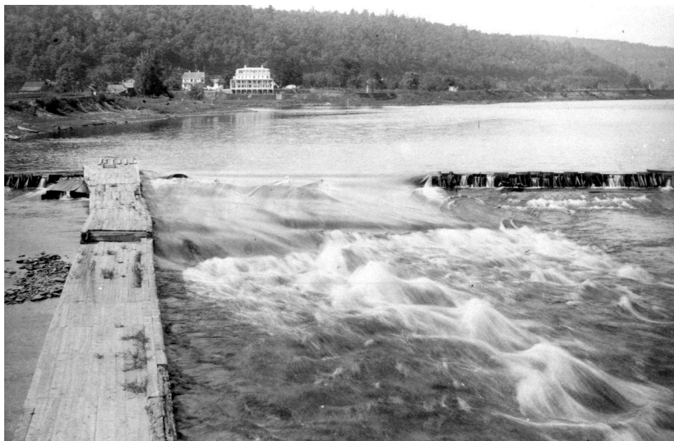
Figure 8. View of the opening in the slackwater dam upstream from the Delaware Aqueduct. Note the two men at the right side of the breach. (UPDE, I8_Scan211-MVHS-P98-8-18)
