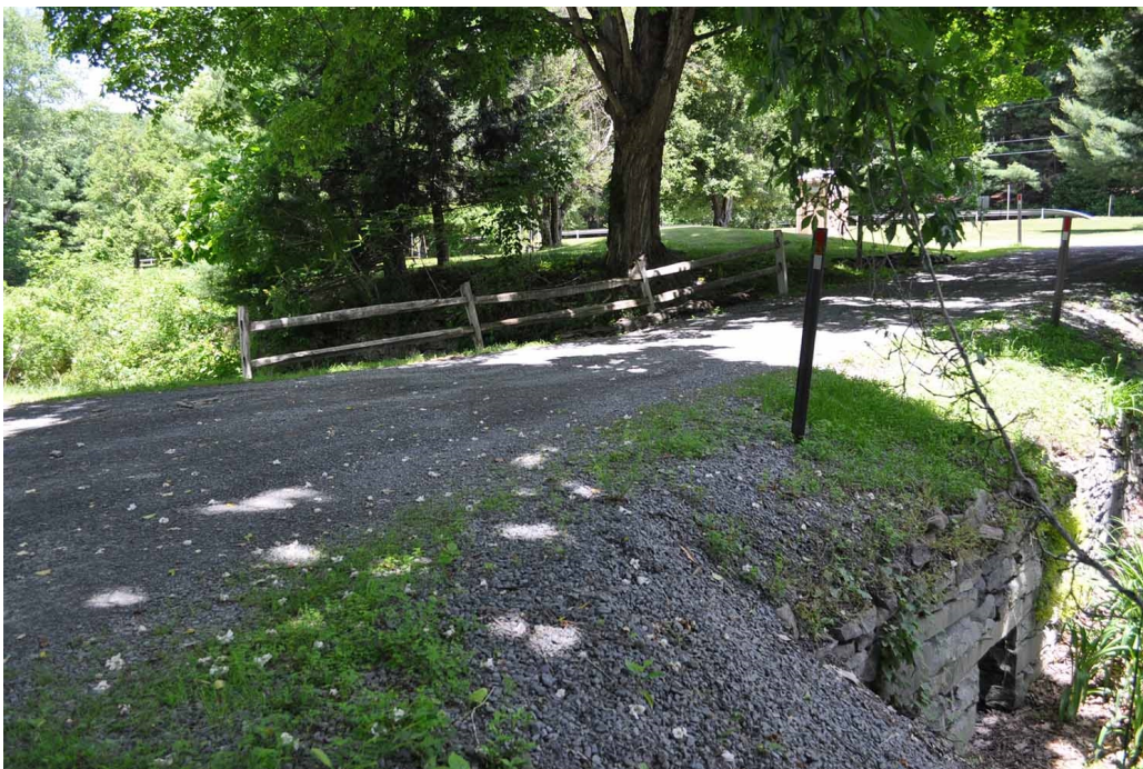
Figure 28. View looking north from within the canal prism at some of the retaining walls. (OCLP 2014, DSC_0489)
