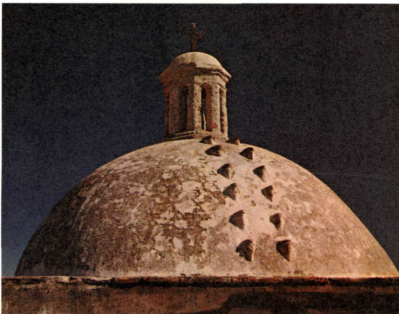
This is a close-up of the dome of the mission building. Note the built-in steps to allow easy access to the lantern.
