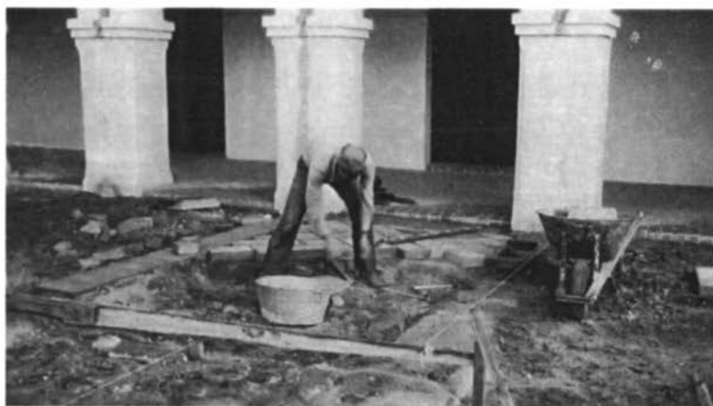
CCC worker installing visitor center courtyard garden walkway, 1940
