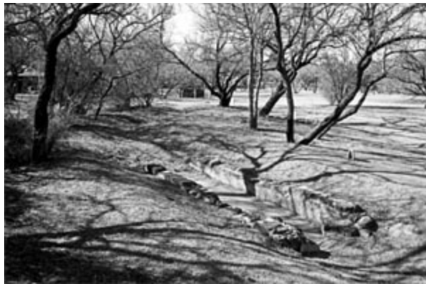
The compuerta or lavandaria just inside the south garden wall.
