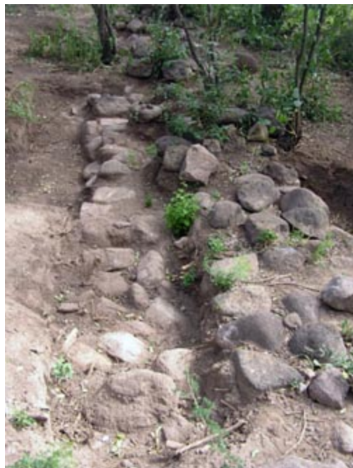
Photo of the foundation for the south garden wall showing lower ledge or footing along the interior. Adobes were probably stacked on the portion of the foundation showing at the surface in the right.
