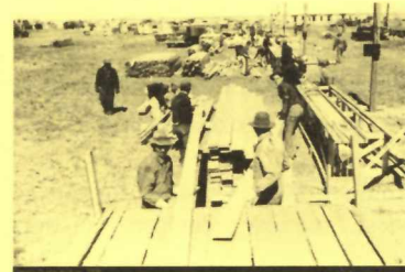
Construction of Barracks
