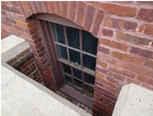
FIGURE 68. View looking down at a typical basement window.
