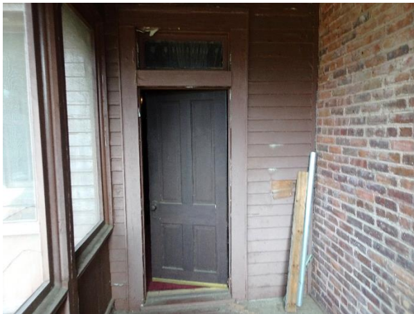
FIGURE 73. Typical door found on the second floor of the double deck porch.
