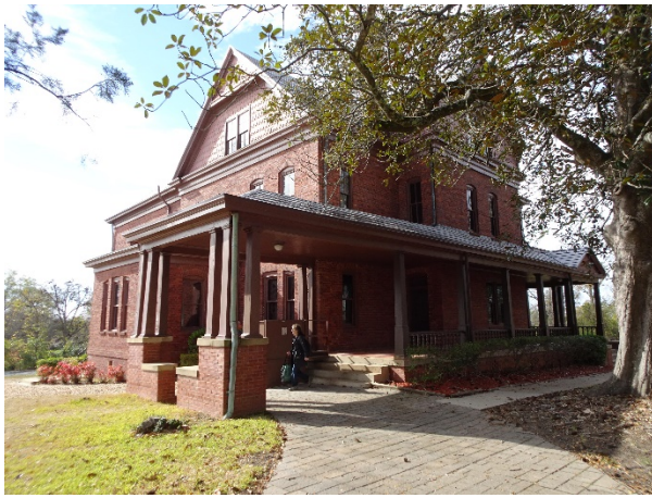
FIGURE 30. The Oaks, north elevation, looking southwest.
