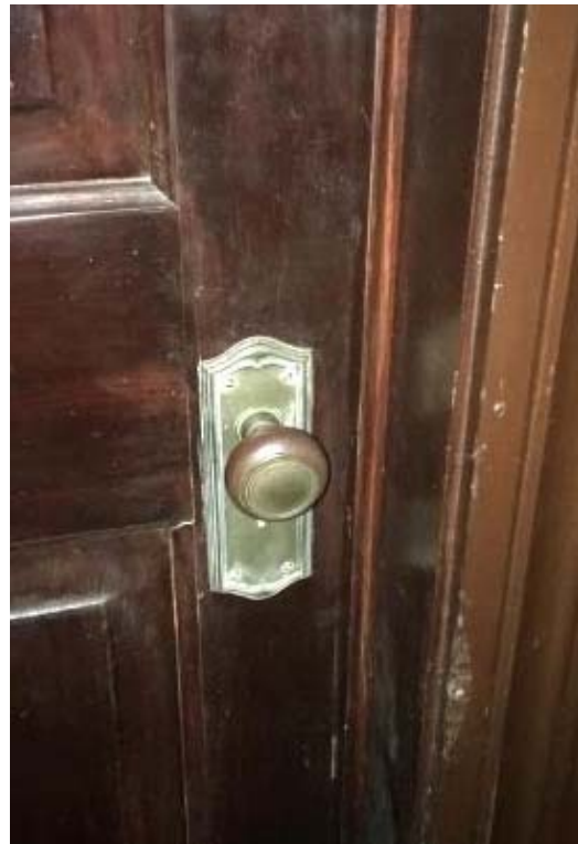
FIGURE 155. Detail of typical latch set.
