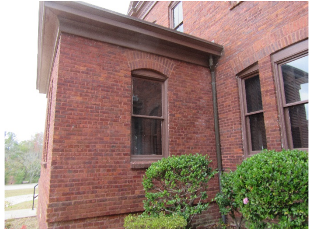
FIGURE 32. North elevation of the dining room addition.
