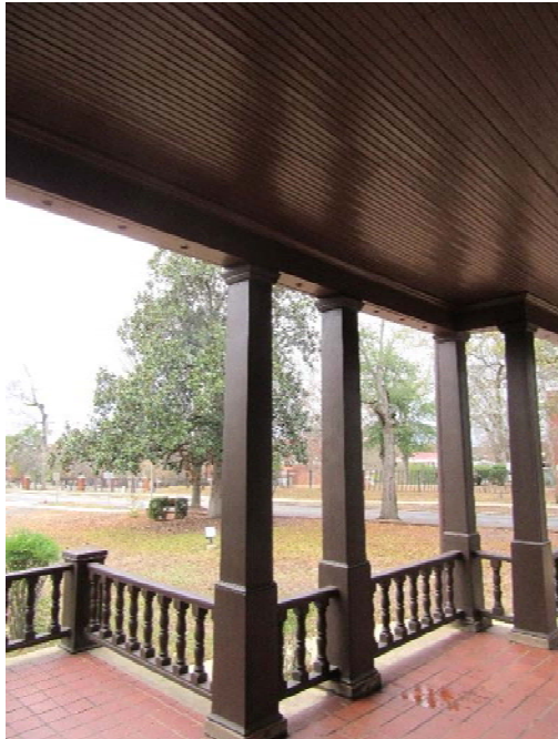
FIGURE 49. Porch columns, balustrade, encased beam, and bead board ceiling.
