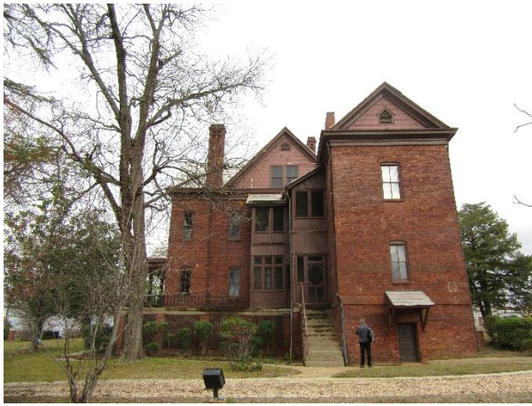
FIGURE 35. The Oaks, south elevation, looking north.
