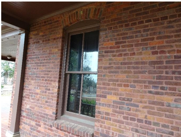
FIGURE 59. Typical masonry window.
