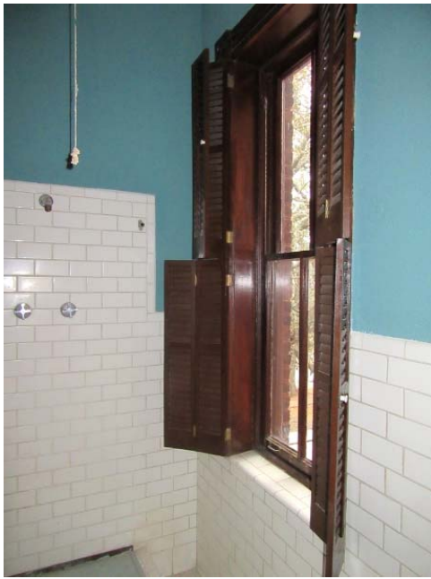
FIGURE 174. Ceramic tile wainscot in Portia's shower room.
