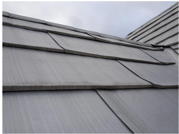
FIGURE 76. Detail of pressed sheet-metal roofing with grooved pattern, giving the appearance of a wood shingle.
