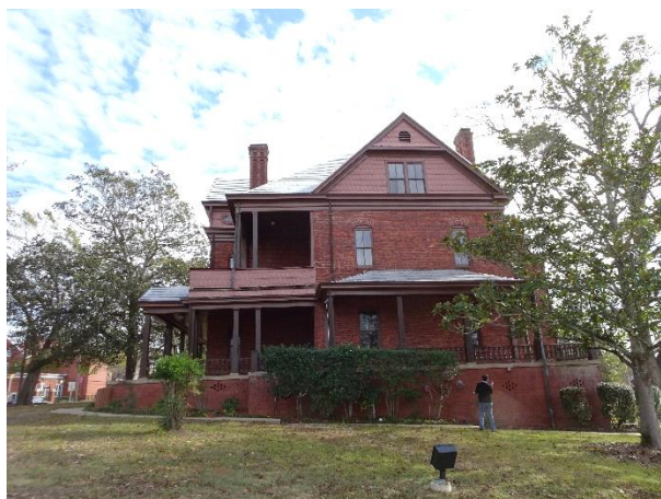
FIGURE 33. The Oaks, west elevation, looking east.
