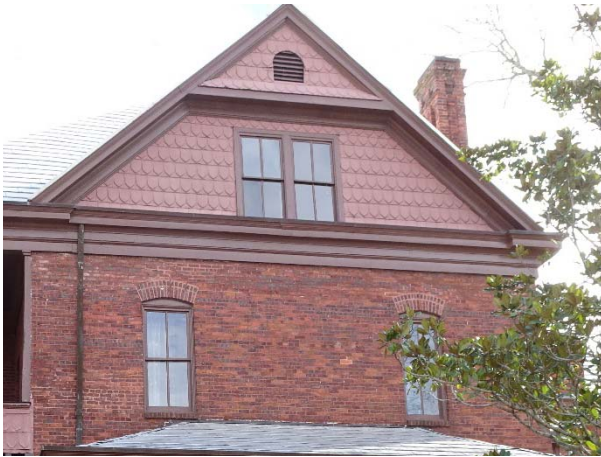
FIGURE 44. Overview of end gable with pressed sheet-metal cladding.
