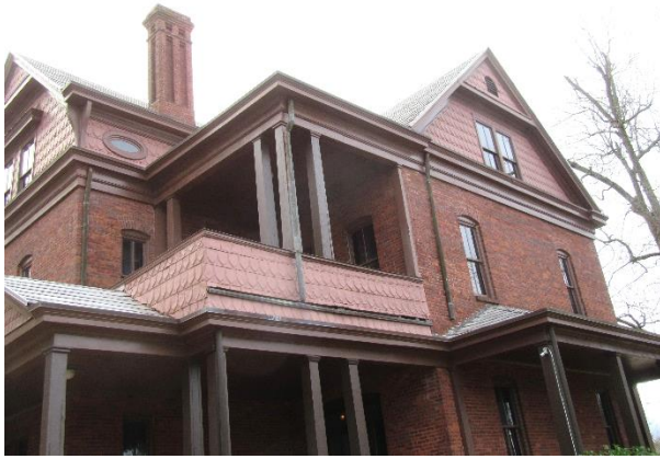
FIGURE 53. The Oaks, second-floor balcony.
