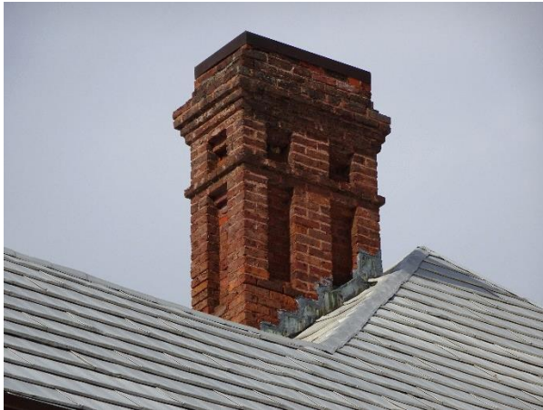
FIGURE 79. Typical brick chimney with corbelled brick details.
