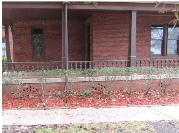
FIGURE 46. Diamond-shaped brick detailing found on the north elevation.
