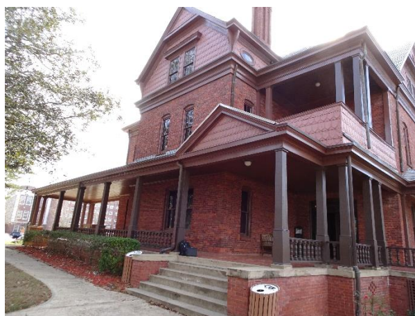
FIGURE 29. The Oaks, north elevation, looking southeast.
