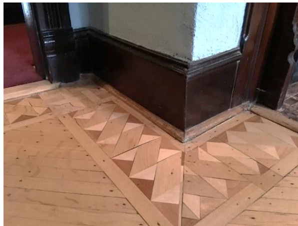
FIGURE 181. Detail of parquet border at second floor.
