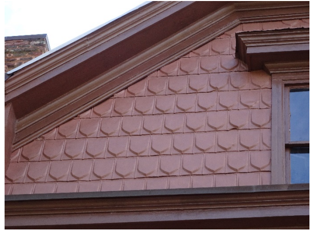
FIGURE 42. Pressed sheet-metal cladding at end gable.
