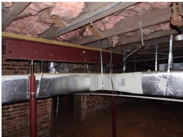
FIGURE 231. Supplemental non-original framing at southwest corner of the crawl space.
