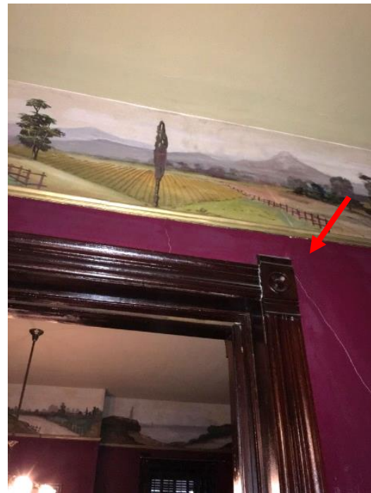
FIGURE 150. Typical first-floor door casing without transom.
