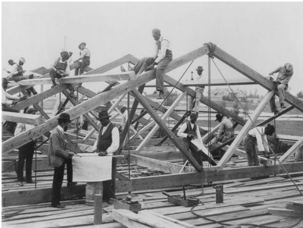
FIGURE 6. Roof construction of building by Tuskegee Students in 1902. (Source: Francis Benjamin Johnson Collection, Library of Congress LC J694-99)
