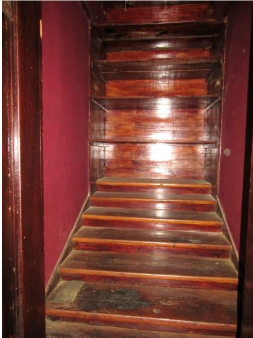
FIGURE 160. A rear wall of shelves terminates the stair inside a second-floor closet.
