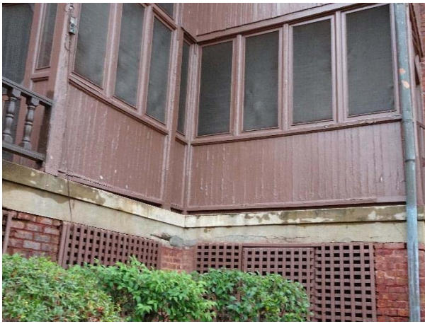
FIGURE 57. The vertically oriented wood cladding at the two-story screen porch.
