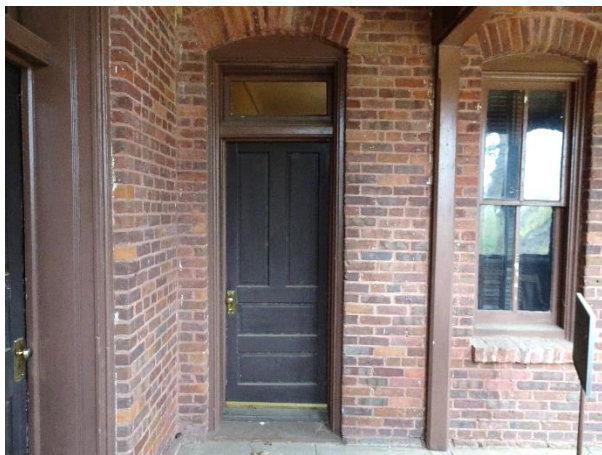
FIGURE 69. Typical side door with four solid panels.
