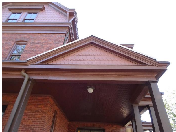
FIGURE 51. North elevation entrance porch gable.
