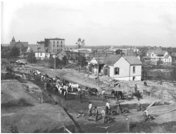
FIGURE 5. Students digging the foundation for the C.P. Huntington Memorial Building. (Source: Francis Benjamin Johnson Collection, Library of Congress LC J694-99)
