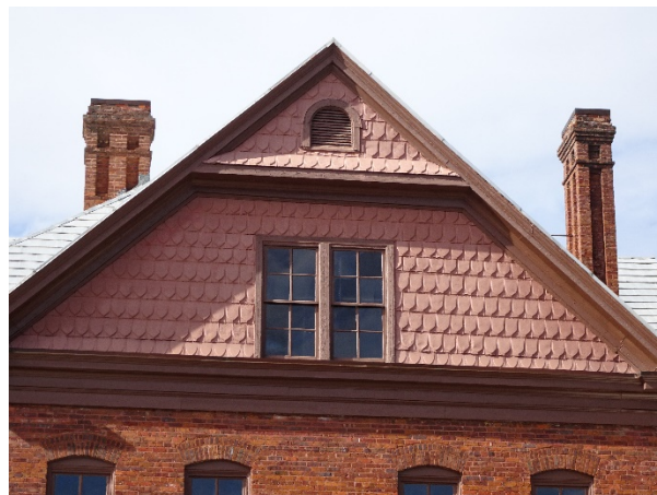
FIGURE 65. Typical third-floor window unit.
