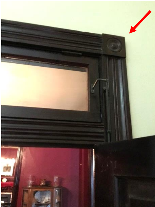
FIGURE 149. Typical door casing with transom.
