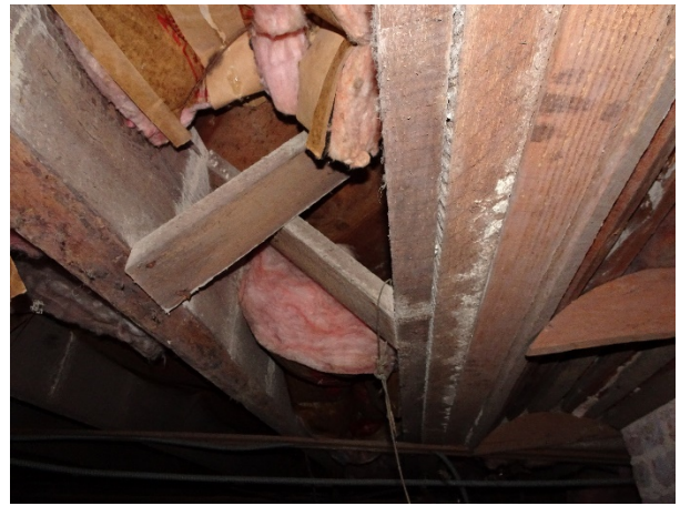
FIGURE 230. View of first-floor framing. Note bridging and insulation at joist pocket.
