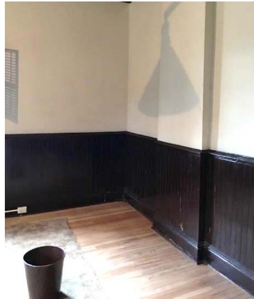
FIGURE 140. Stained wood wainscot.
