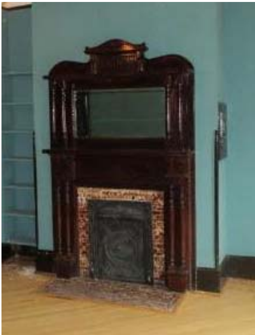
FIGURE 162. Detail of fireplace in Margaret Washington's bedroom.
