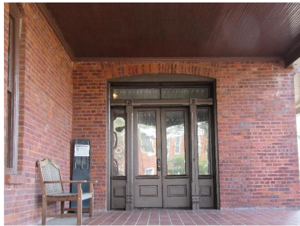
FIGURE 71. Main entrance door on the north elevation.
