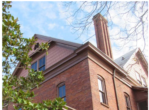
FIGURE 43. View of typical entablature detailing and the decorative depression found at a few of the gable ends.
