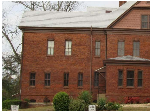
FIGURE 61. The Oaks, east elevation, showing the minor modifications made to the typical masonry window unit.
