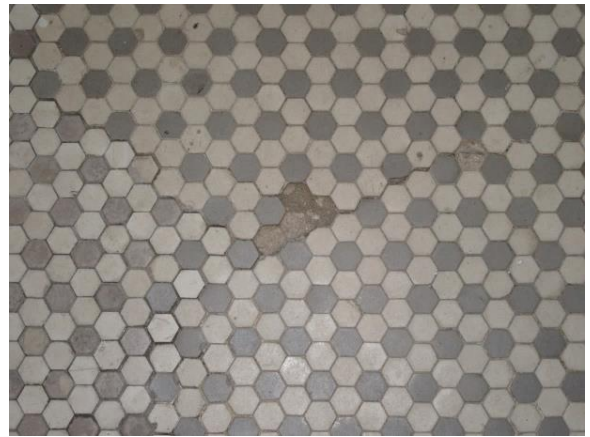
FIGURE 168. Detail of floor tile at bathroom.
