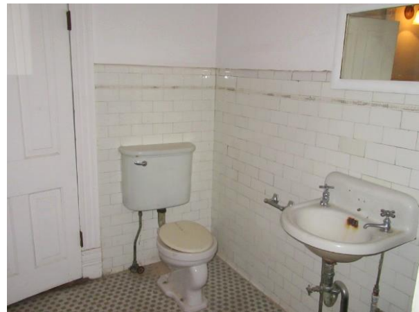
FIGURE 141. Ceramic tile at bathroom.
