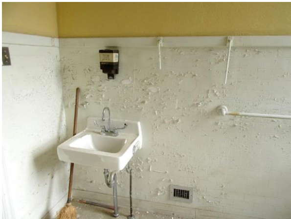
FIGURE 213. Lavatory and painted wainscot in third-floor bathroom.
