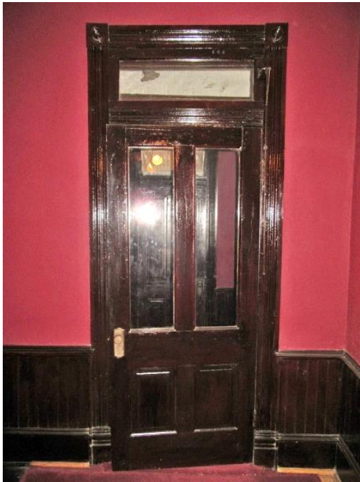
FIGURE 182. Typical door with transom.
