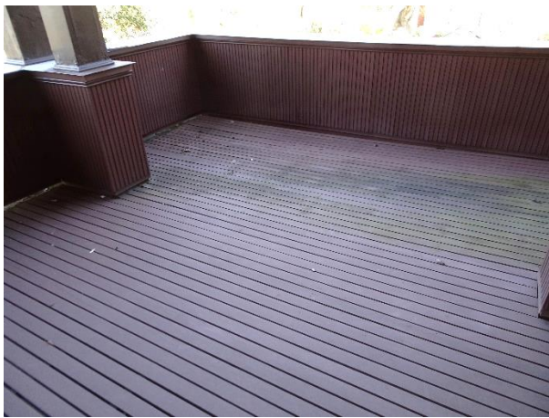
FIGURE 54. The balcony at the second floor.
