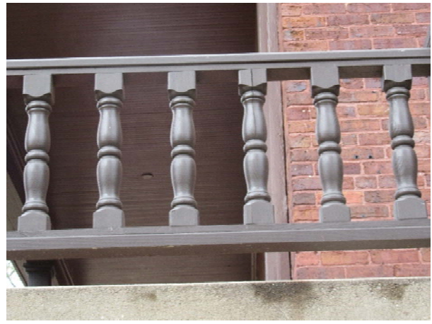
FIGURE 48. Typical painted brown wood railing.
