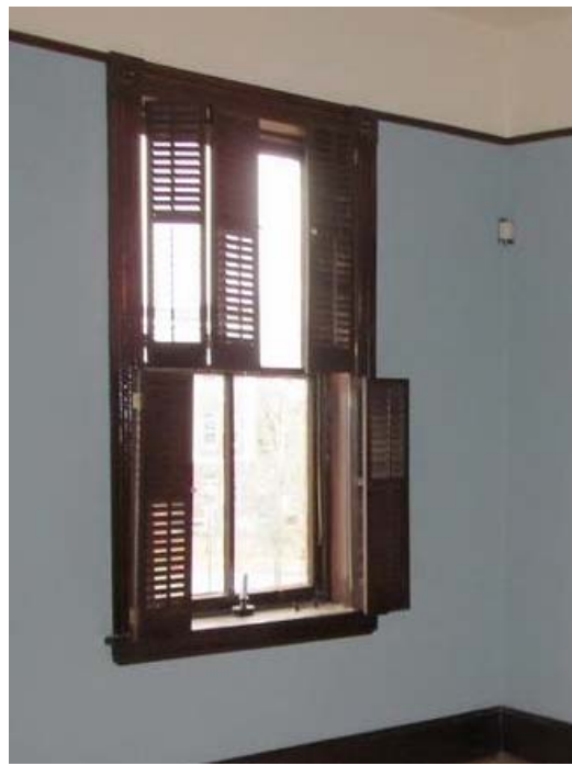
FIGURE 153. Typical window shutters.
