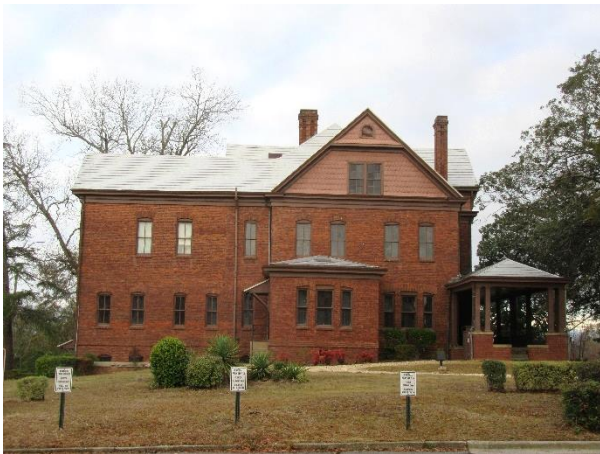
FIGURE 38. The Oaks, east elevation, looking west.
