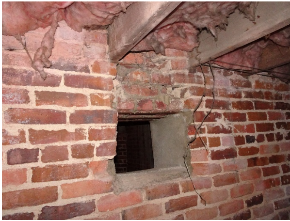
FIGURE 228. Load-bearing masonry wall at interior of basement / crawl space.
