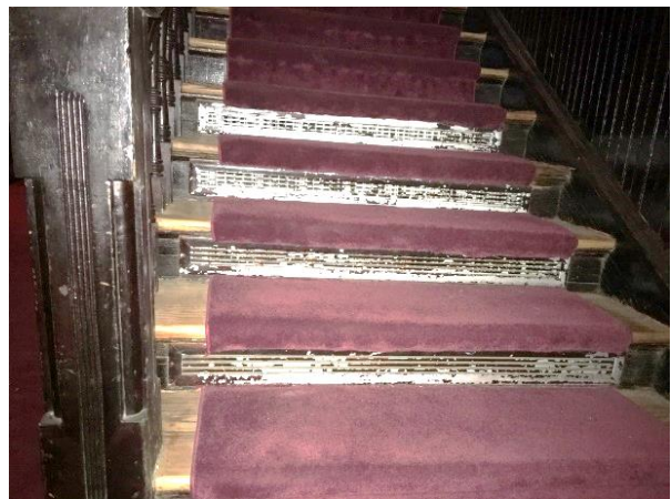
FIGURE 148. Carpet and grilles at stair.
