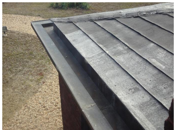
FIGURE 78. Gutters and downspouts on the east addition.
