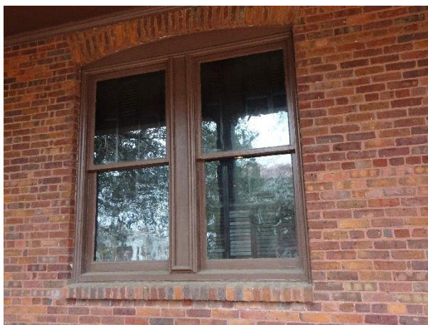
FIGURE 63. One-over-one paired window unit located at the wrap-around porch on the north elevation of the building.
