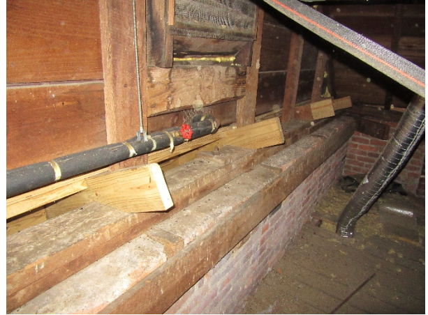
FIGURE 235. Replaced structural kickers at south wing roof.
