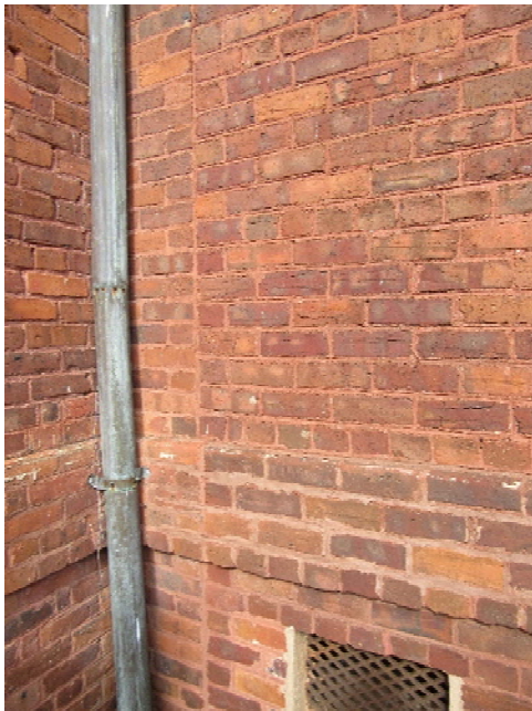
FIGURE 41. The corner where the dining room addition abuts the main structure.
