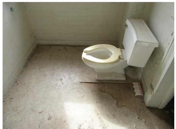
FIGURE 199. Floor in third floor bathroom.
