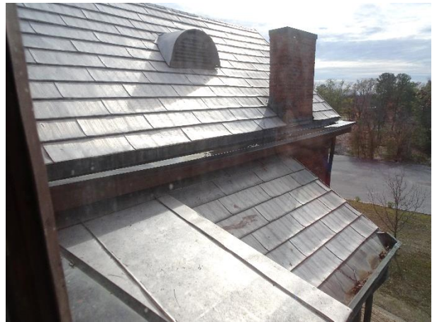
FIGURE 77. The typical roofing material, plus the standing seam panel and aluminum roof vent.
