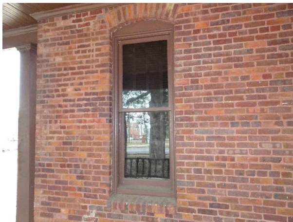
FIGURE 62. Typical one-over-one window type at the wrap-around porch.
