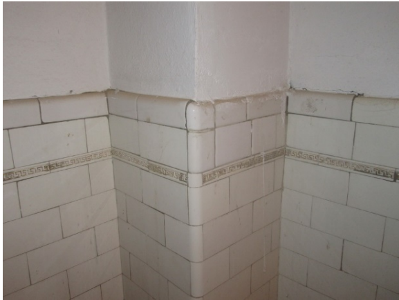
FIGURE 167. Detail of wall tile at bathroom.
