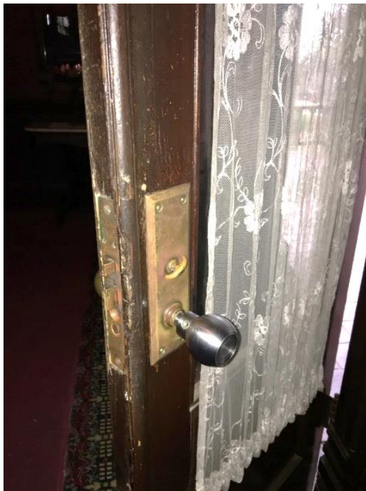
FIGURE 157. Non-original hardware.
