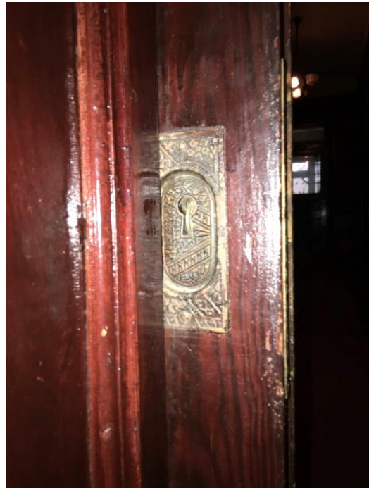
FIGURE 156. Detail of pocket door hardware.
