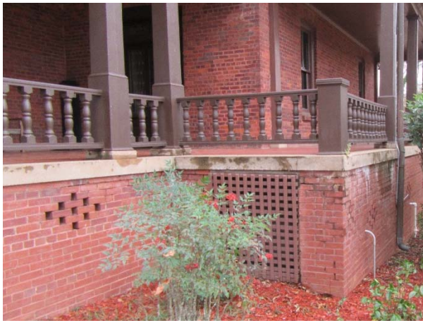
FIGURE 47. Wood lattice visible on main porch, visible from the north elevation.
