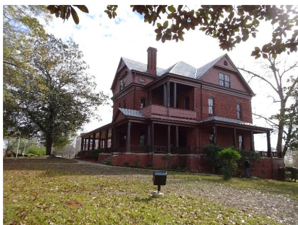
FIGURE 28. The Oaks, looking southeast. (Source: All photographs by authors unless otherwise noted)
