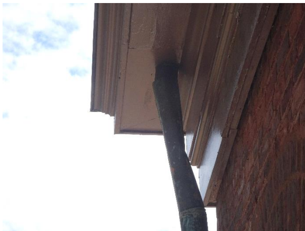
FIGURE 117. Damaged downspout.
