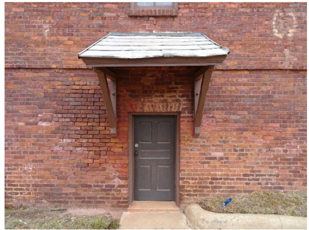
FIGURE 74. Basement entrance at the south elevation of the south wing.
