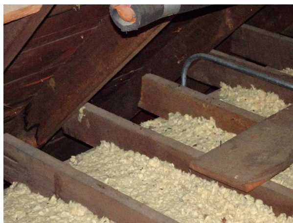
FIGURE 232. Ceiling joists as viewed from the attic.
