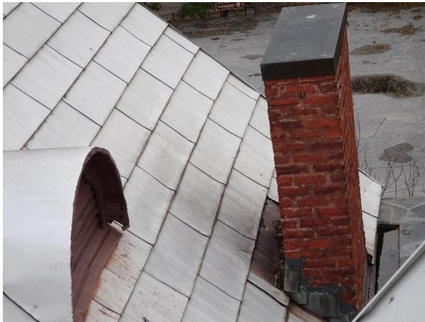
FIGURE 80. Non-original brick chimney at the west elevation of the south wing of the building.
