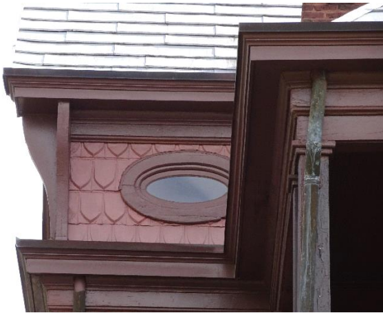
FIGURE 67. An elliptical window, looking east toward the west return wall elevation of the projecting gable.
