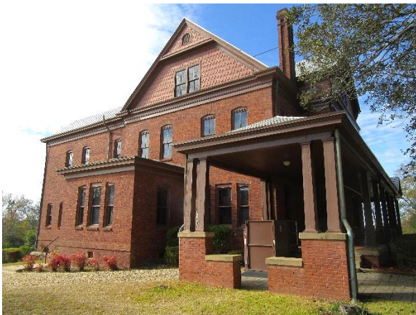
FIGURE 39. The Oaks, east elevation, looking southwest.
