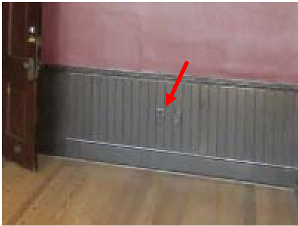
FIGURE 203. East bedroom – new receptacles in wainscot.
