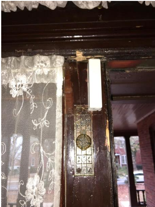
FIGURE 154. Hardware at entry door.
