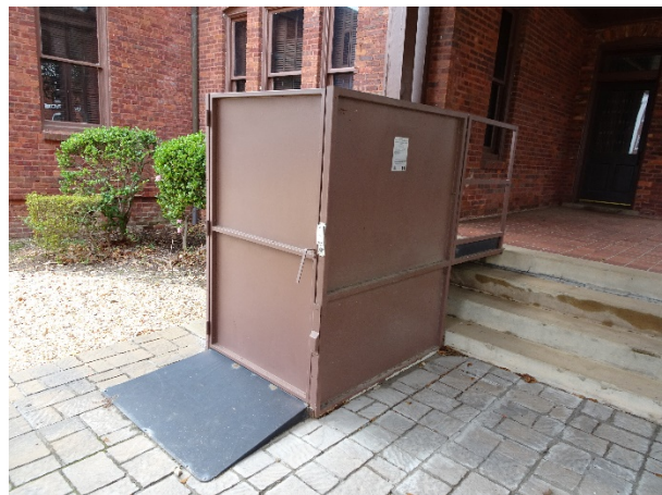
FIGURE 52. Wheelchair lift located at the staircase within the porte-cochère.
