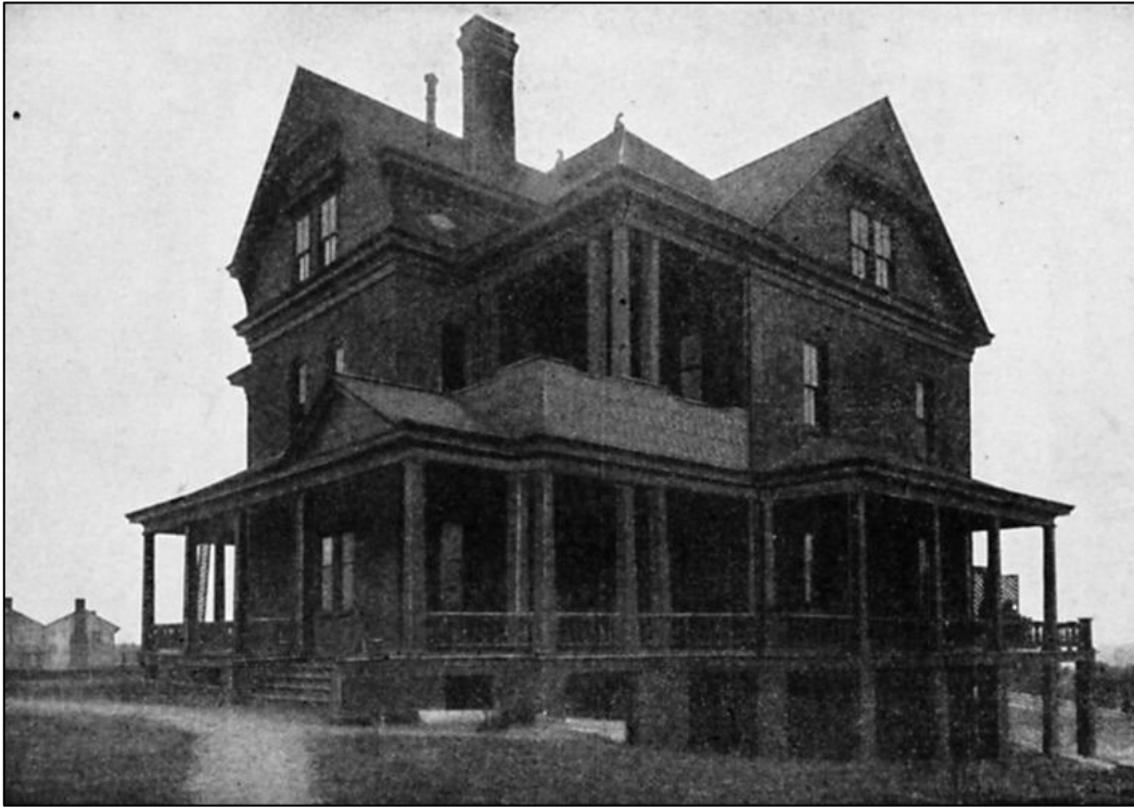
Fig 6-1. Circa 1900 view of the north and west elevations of the Oaks. Note that none of the landscaping had been installed. The historic circulation pattern of the front walkway appears to be in place, though it is more formalized in later views (see Figure 6-5). (Schomburg Center for Research in Black Culture, Jean Blackwell Hutson Research and Reference Division, New York Public Library Digital Collections. http://digitalcollections.nypl.org/items/510d47df-7576-a3d9-e040-e00a18064a99 ).
