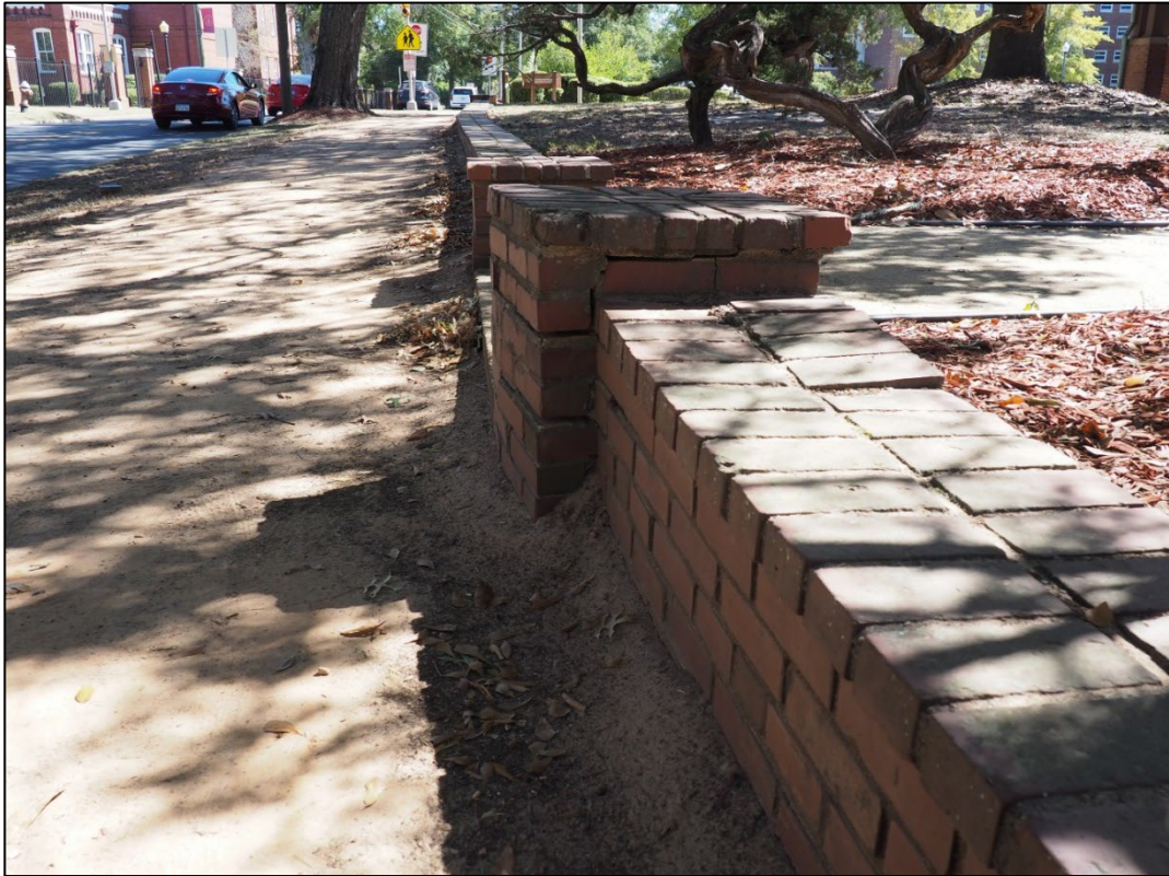
Fig 8-21. Front retaining wall, photo by author
