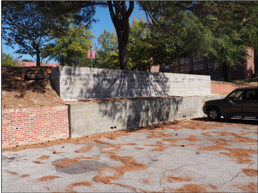
Fig 8-20. Brick retaining wall adjacent to concrete block retaining wall in south parking lot, photo by author
