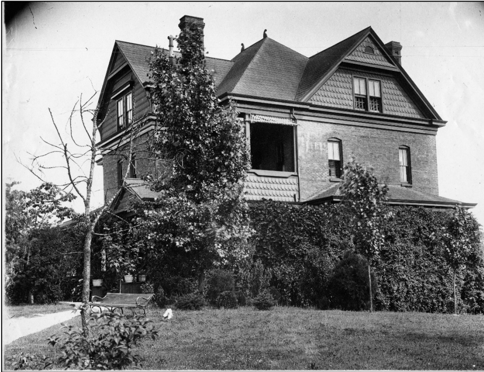
Fig 6-18. The Oaks, circa 1925 taken from the northwest corner of the property. The front walkway still exists, vines cover the house, but the fencing between the front lawn area and the rear yard appears to have been removed. (Tuskegee University Archives, Special Collections, Digital Files)
