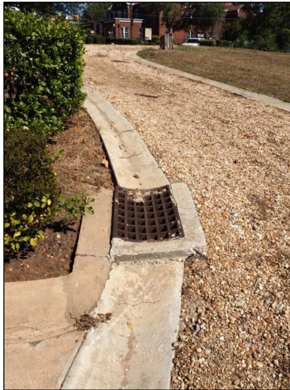
Fig 8-16. Gravel carriage trail with concrete valley gutter and drain inlet, photo by author
