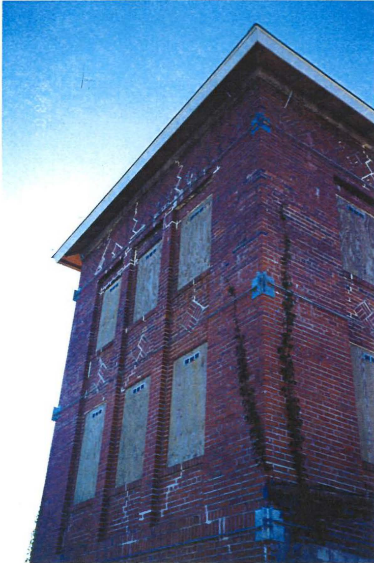
Photo 2. Control Tower Building – West Face
