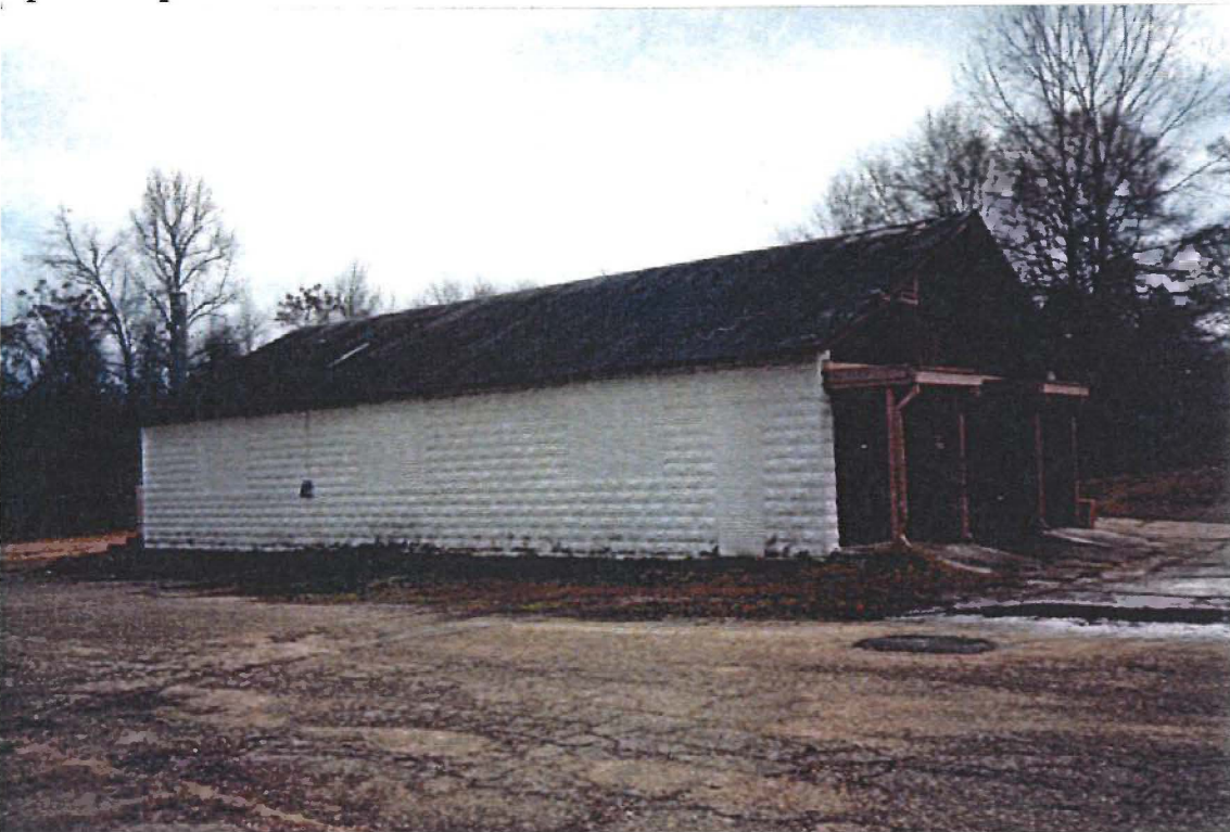
Figure 9: North facade of the Warehouse/Vehicle Storage Building as it looks today. Former window and door openings were infilled with smooth-faced block. Pond & Company.
