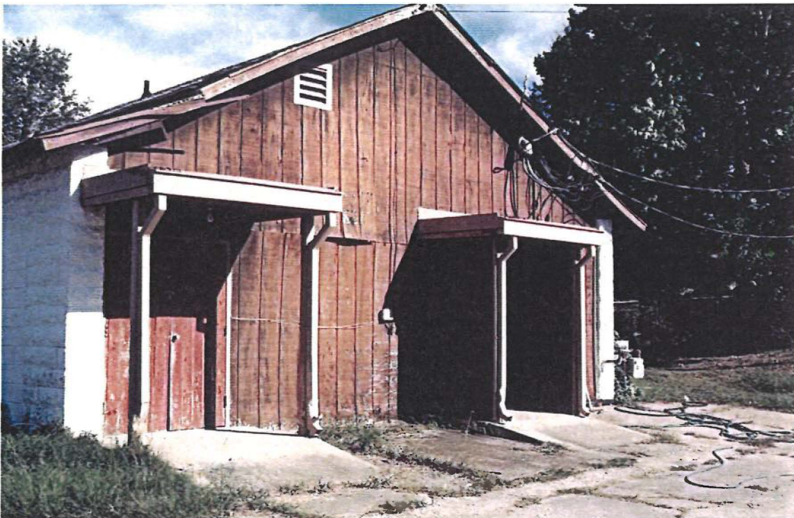
Figure 8: West facade as it looks today. Both the east and west facades were completely replaced as part of the 1974 renovation.
