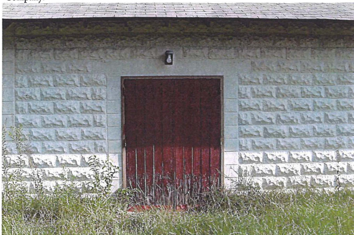
Figure 7: A door opening on the south façade created during the 1974 renovation. Smooth-faced replacement block matches original courses. The original window lintel remains.
