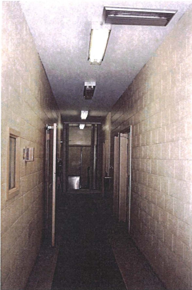
Figure 10: South interior hallway of the Warehouse/Vehicle Storage Building looking east. The walls, ceiling, and concrete floor were added during the 1974 renovation.
