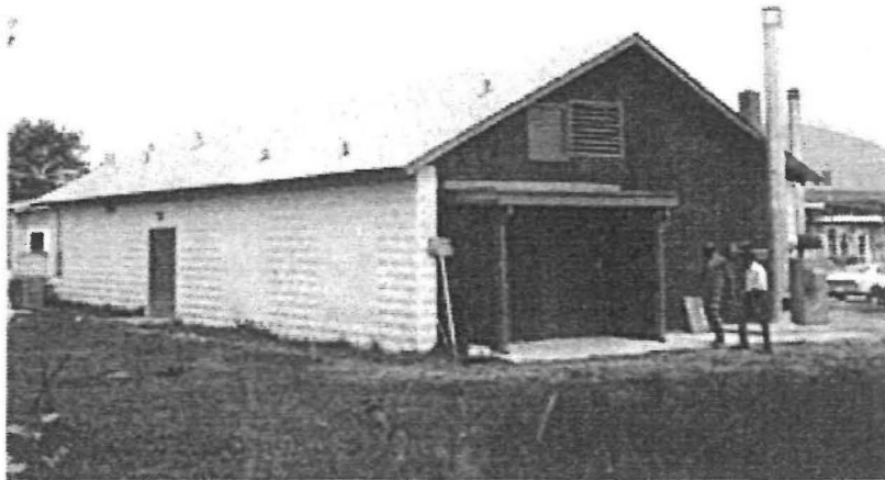
Figure 5: The Warehouse/Vehicle Storage Building as it looked shortly after the Veterinary School's renovation. Booker Conley's Files, Physical Plant, Tuskegee University.
