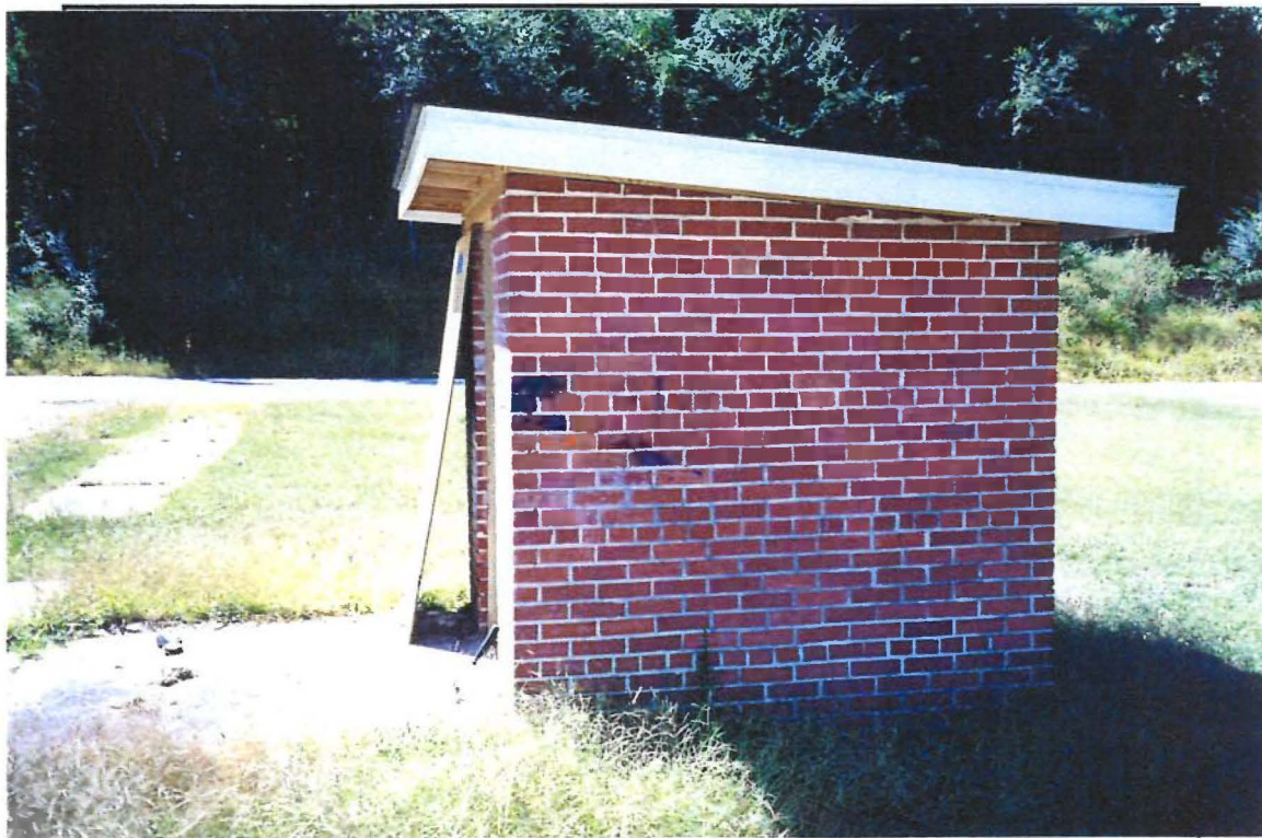
Photo 14. Fire Protection Shed – East Face
