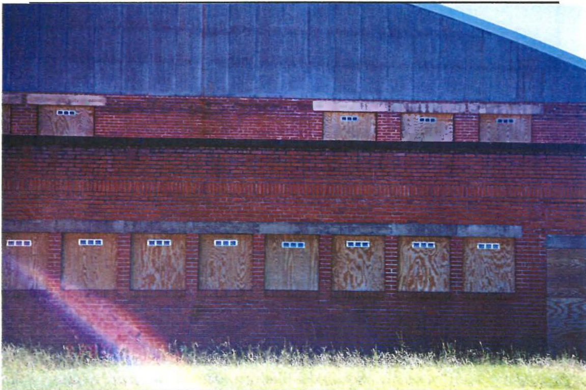
Photo 8. Hangar No. 1 – West Face
