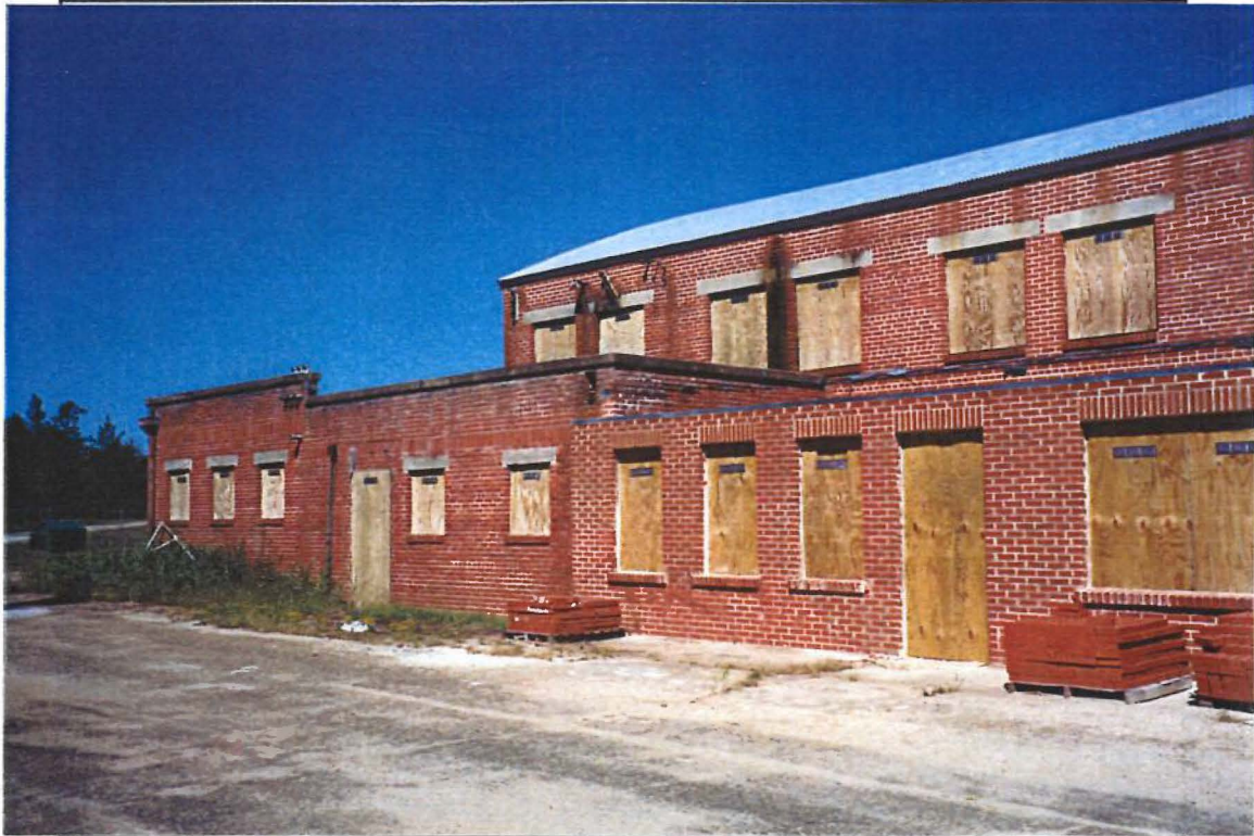
Photo 9. Hangar No. 1 – South Face
