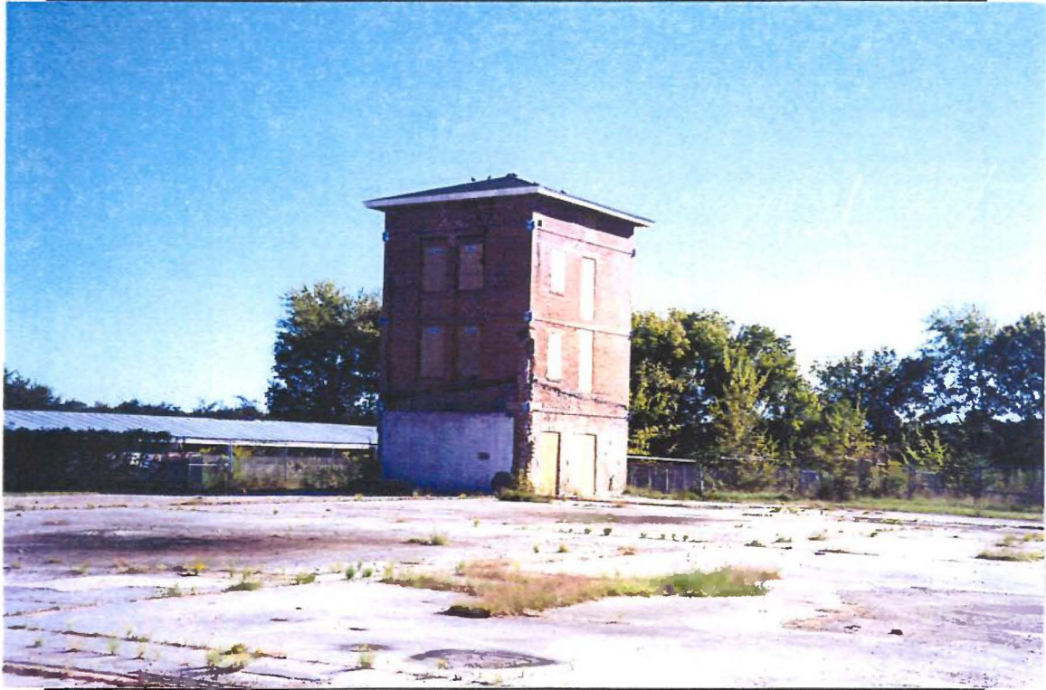
Photo 1. Control Tower Building
