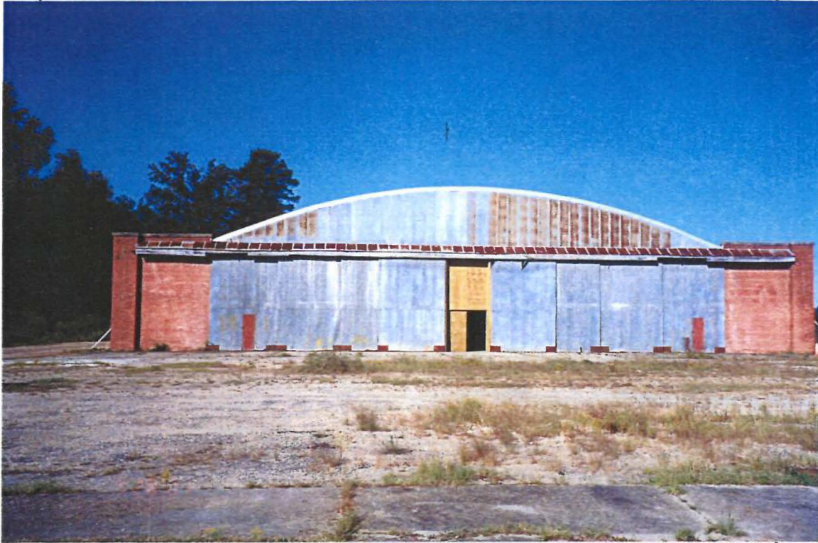
Photo 7. Hangar No. 1 – East Face
