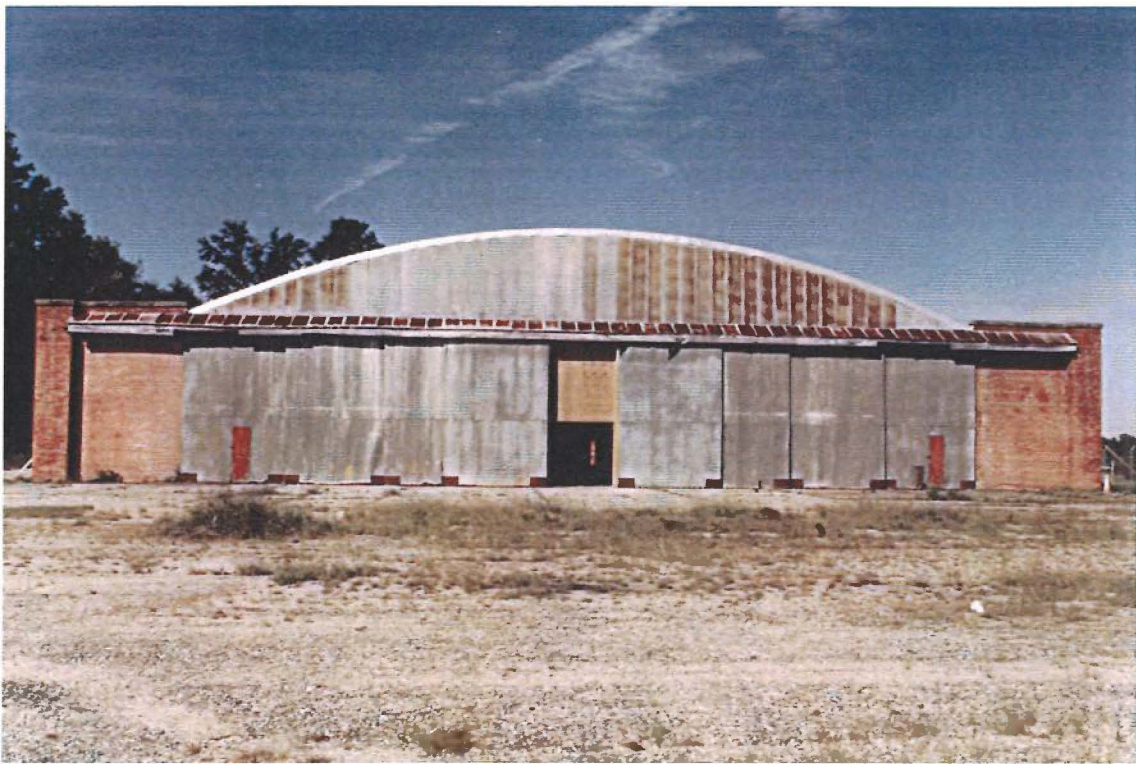
Figure 14: Existing east front facade.
