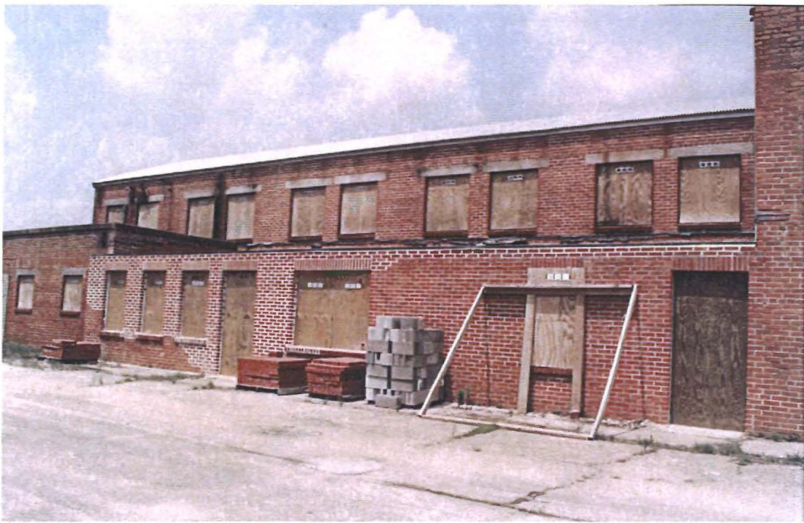
Figure 16: Existing south side facade showing rebuilt wall of lunch/tea room addition.
