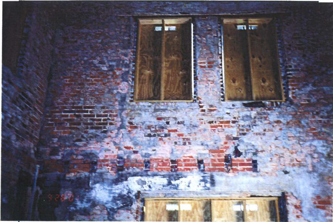
Photo 3. Control Tower Building – Interior North Face
