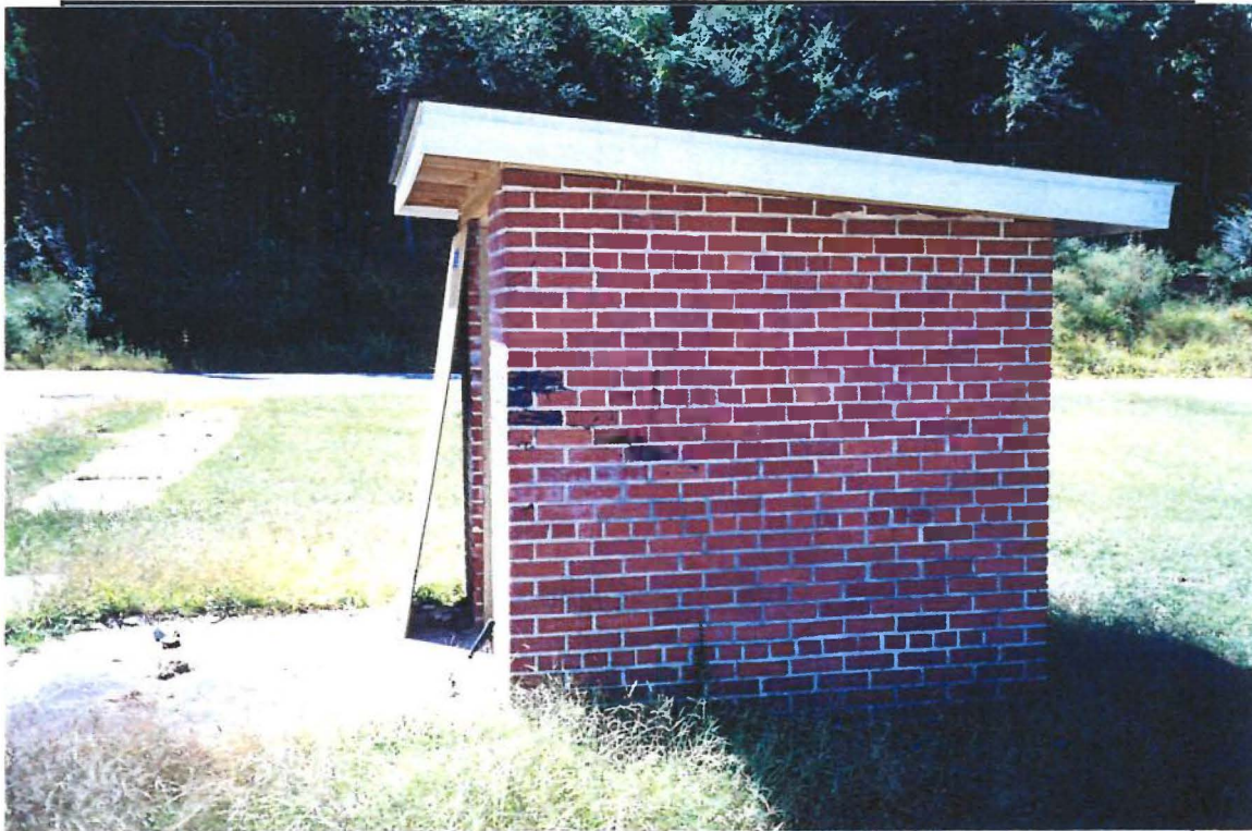
Photo 14. Fire Protection Shed – East Face
