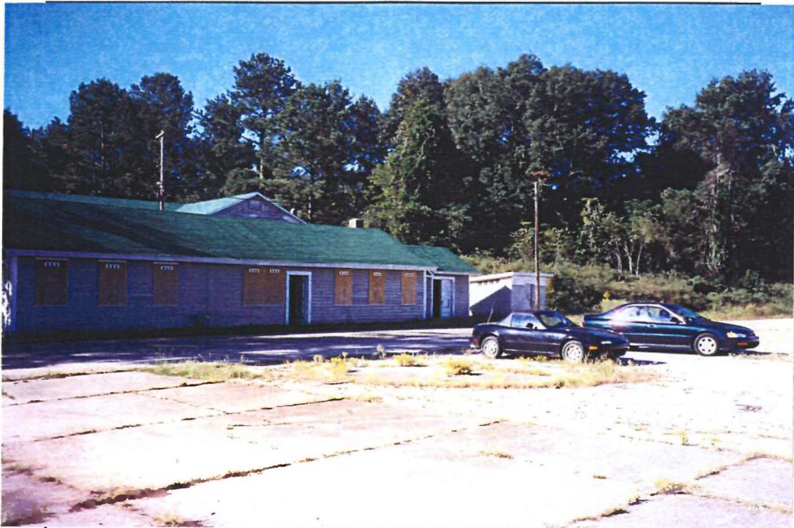
Photo 18. Bath and Locker House – East Face
