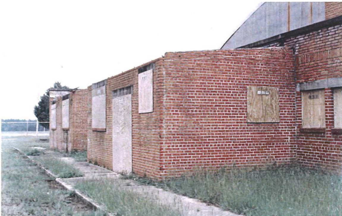
Figure 19: Existing office addition on west rear facade.
