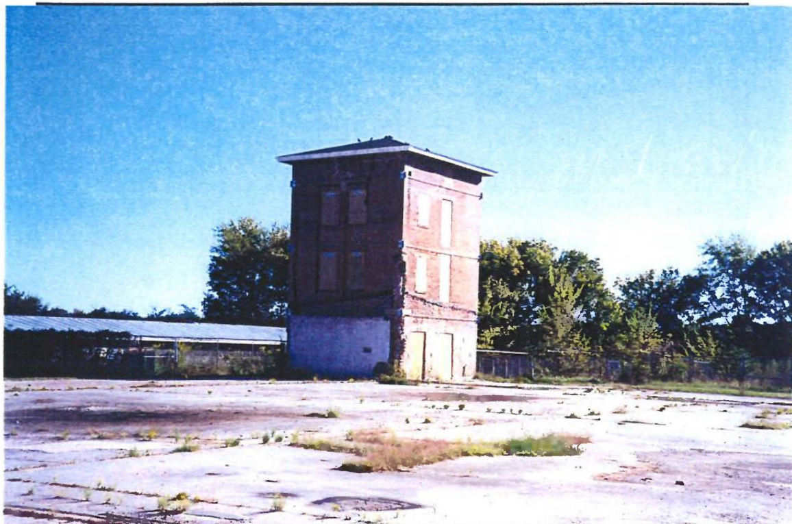
Photo 1. Control Tower Building
