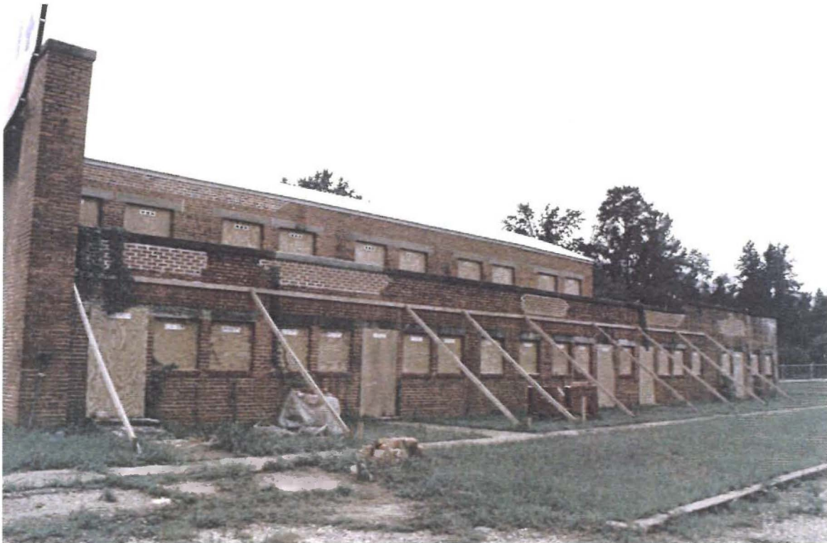
Figure 17: Existing north side facade with temporary shoring.
