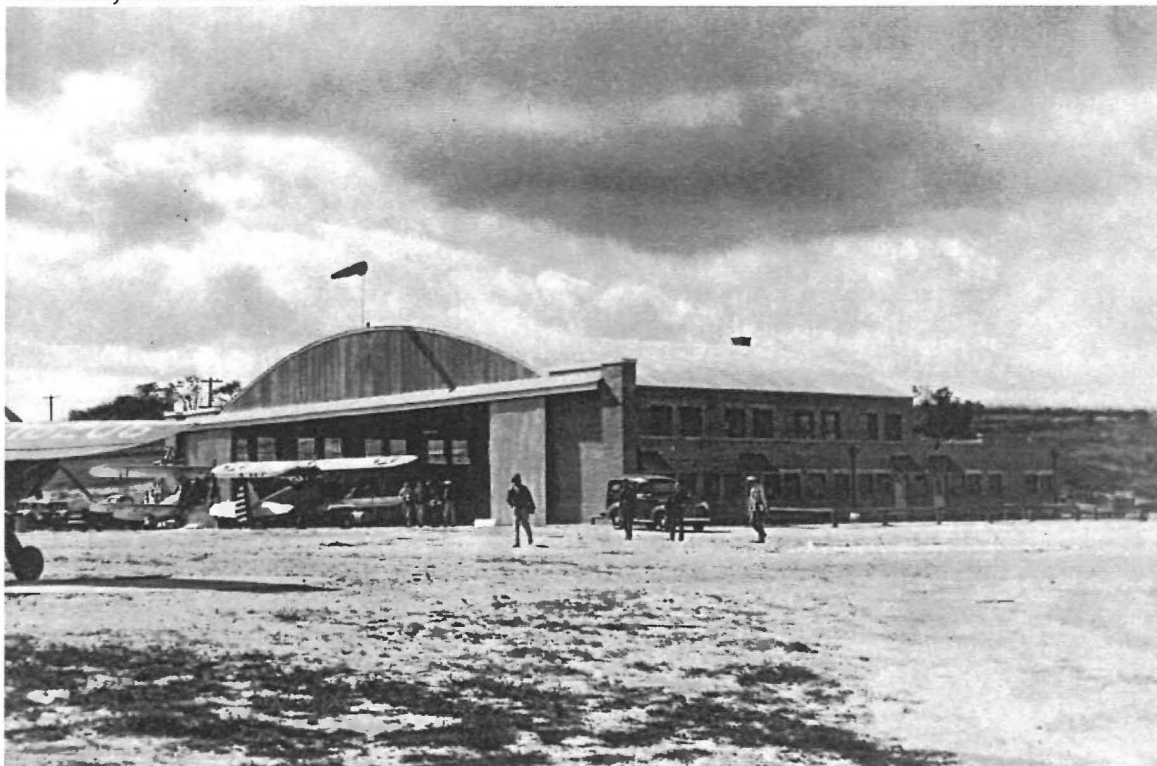
Figure 2: Photo of Hangar Number One in use before the 1943-1944 office addition. Historic Photograph Collection, Howard University.
