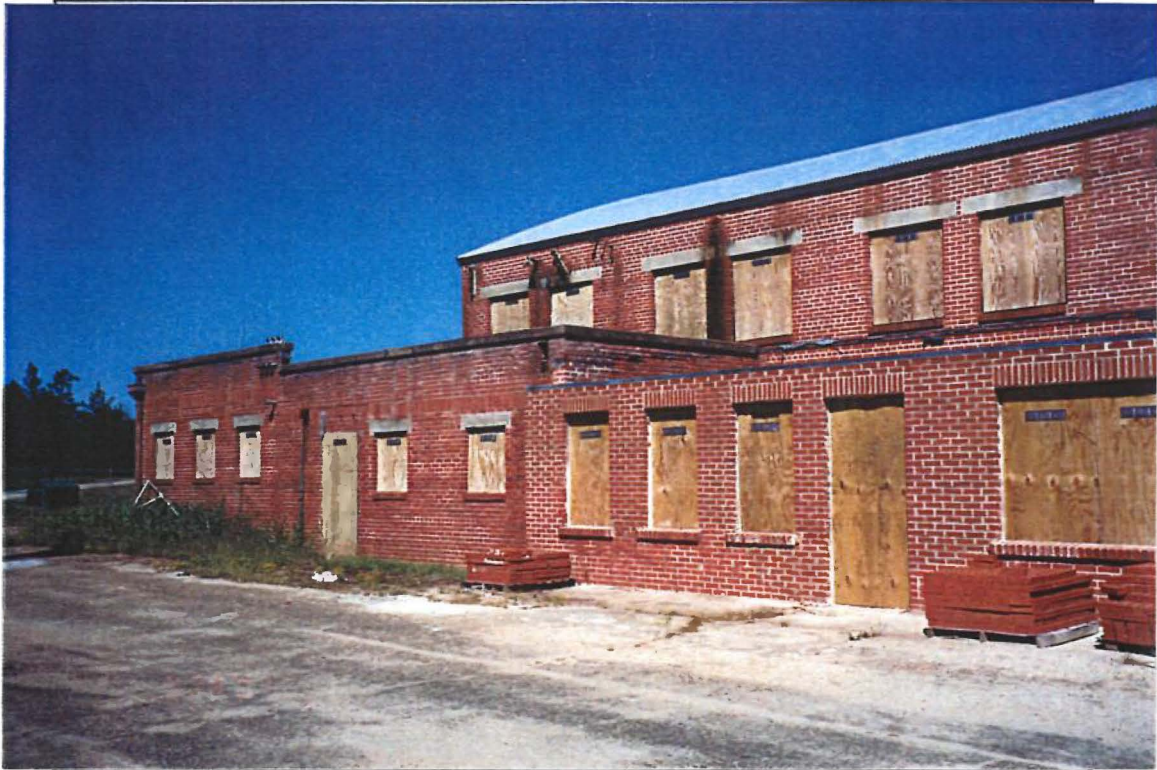
Photo 9. Hangar No. 1 – South Face
