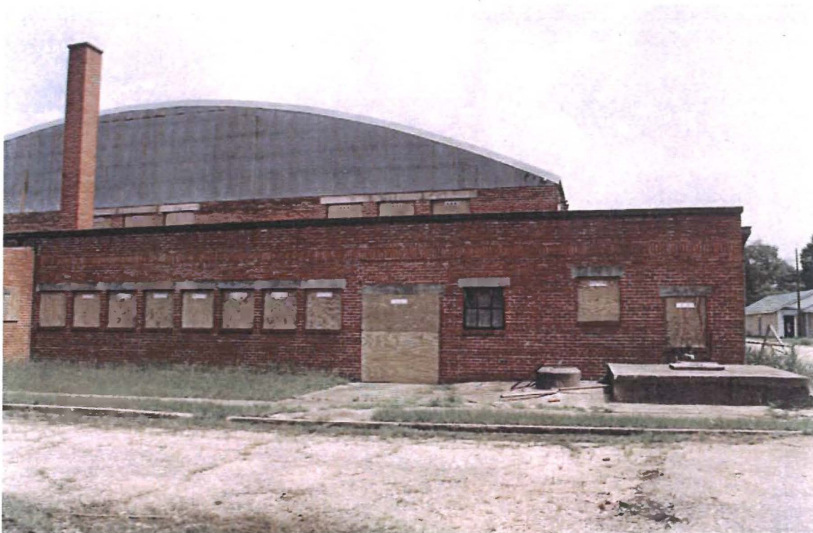
Figure 18: Existing west rear facade with water cistern.
