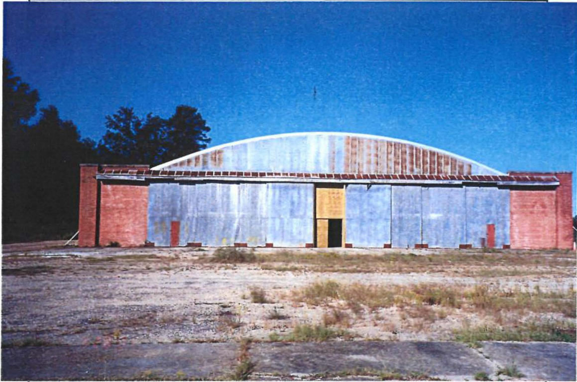
Photo 7. Hangar No. 1 – East Face
