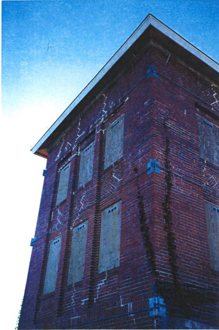
Photo 2. Control Tower Building – West Face
