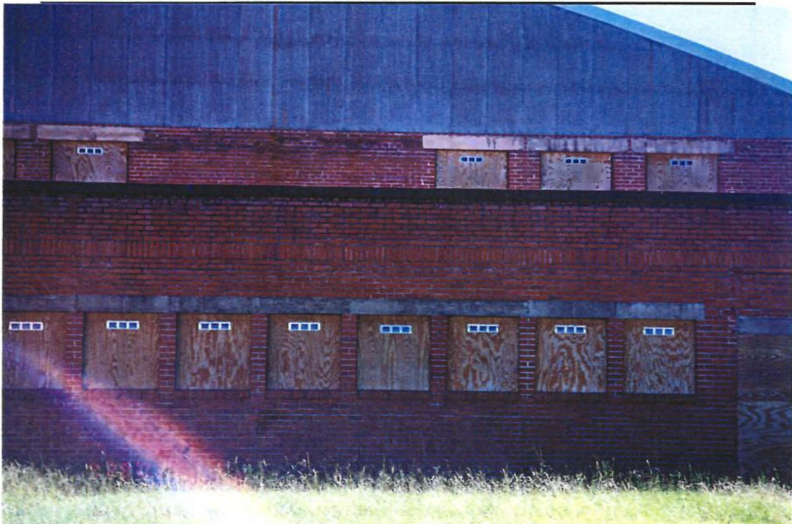
Photo 8. Hangar No. 1 – West Face
