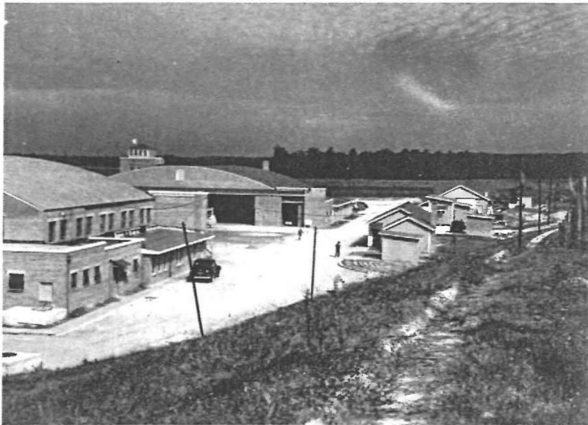
Figure 8: Photo showing the lunch/tea room addition on the south facade of Hangar Number One. Historic Photograph Collection, Howard University.
