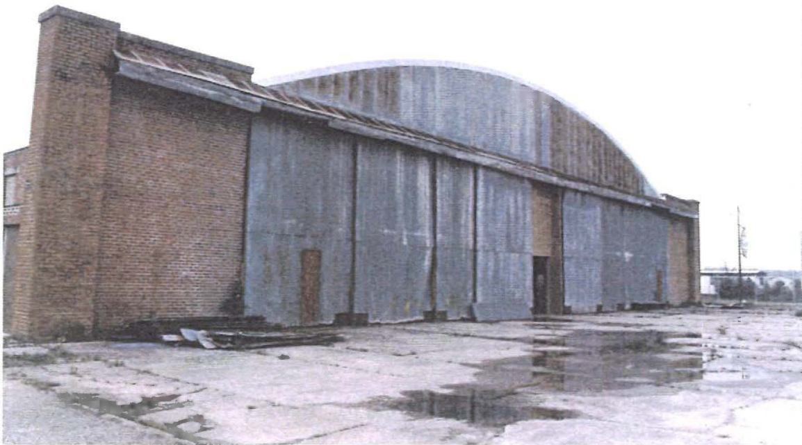
Figure 15: Existing sliding hangar doors.
