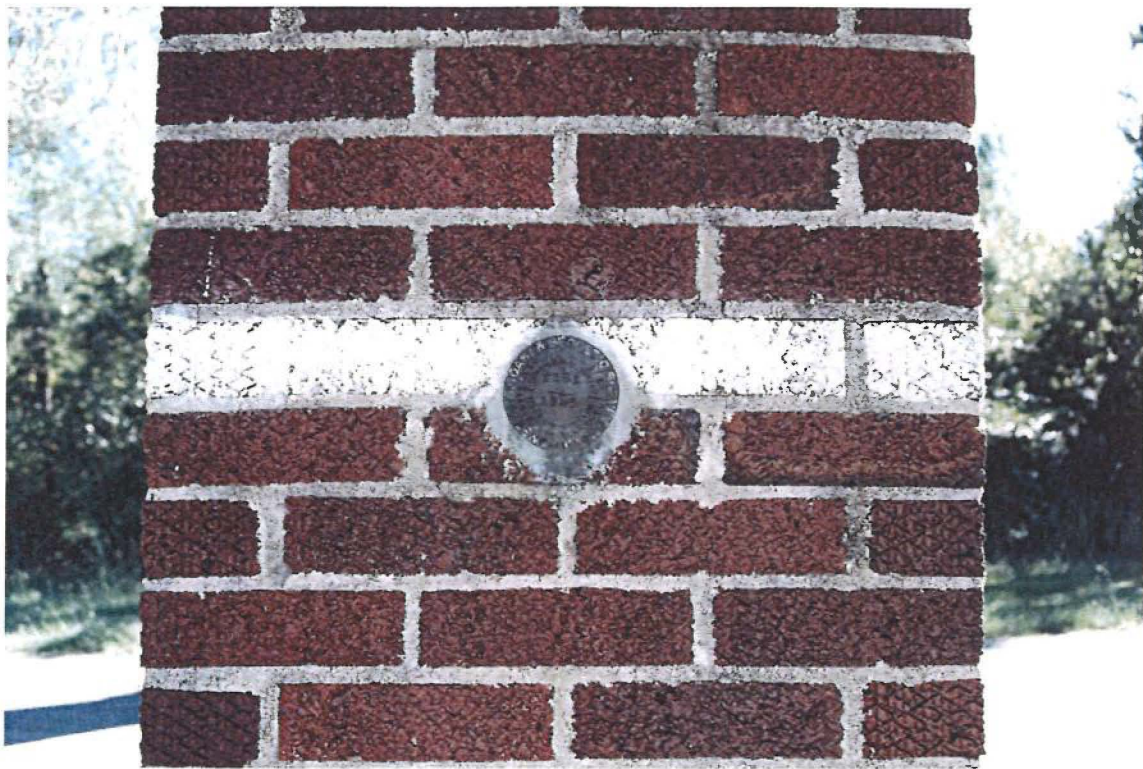
Figure 3: United States Coast and Geodetic Survey Bench Mark installed in 1945.
