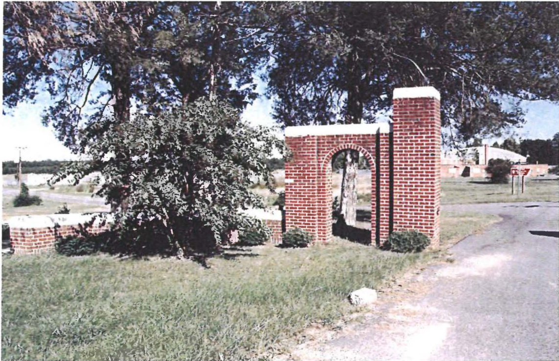
Figure 5: North Wall of Entrance Gate.
