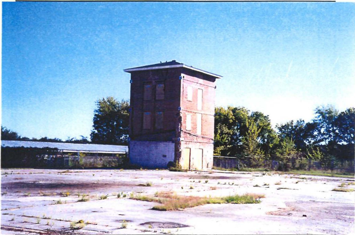
Photo 1. Control Tower Building
