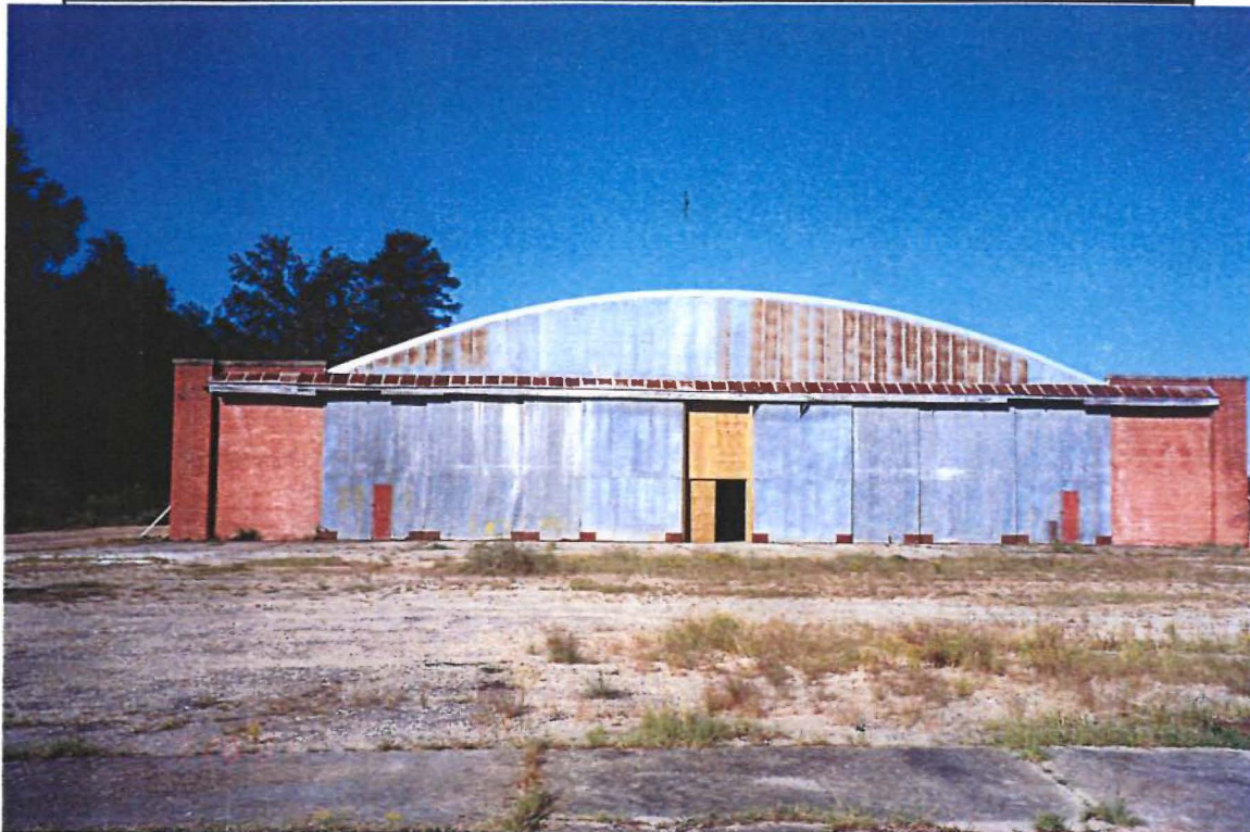
Photo 7. Hangar No. 1 – East Face
