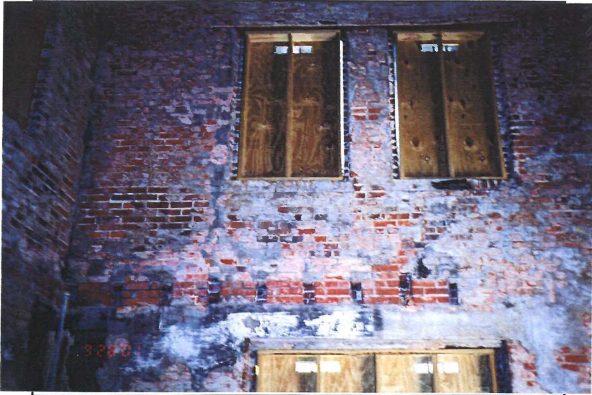
Photo 3. Control Tower Building – Interior North Face
