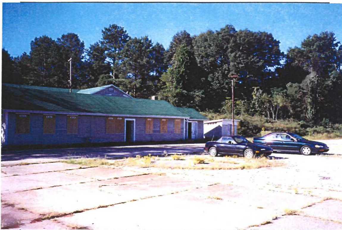
Photo 18. Bath and Locker House – East Face
