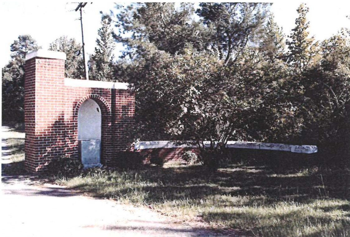
Figure 7: South Wall of Entrance Gate.
