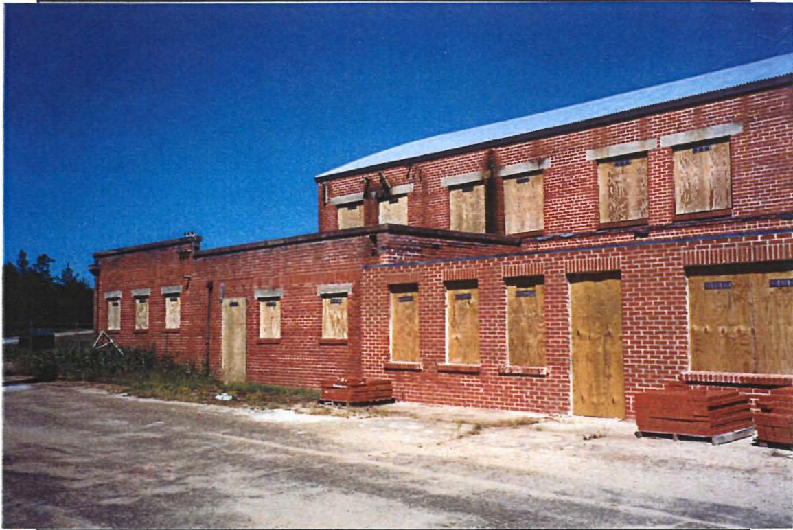
Photo 9. Hangar No. 1 – South Face
