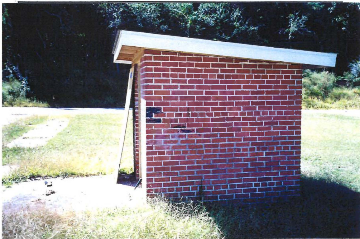
Photo 14. Fire Protection Shed – East Face
