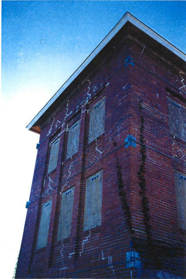
Photo 2. Control Tower Building – West Face
