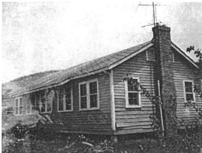
Figure 8: 1977 photograph of the west rear and north side facades of the Cadet Class and Waiting Room when it was used as a residence. Booker Conley's Files, Physical Plant, Tuskegee University.
