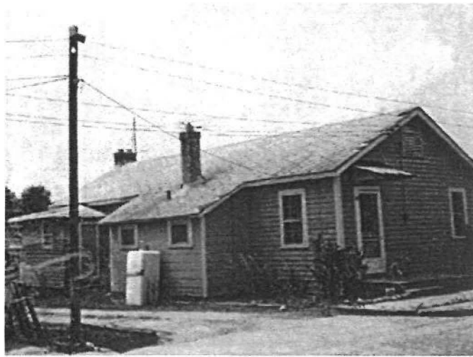
Figure 7: 1977 photograph of the east front and south side facades of the Cadet Class and Waiting Room when it was used as a residence. Booker Conley's Files, Physical Plant, Tuskegee University.
