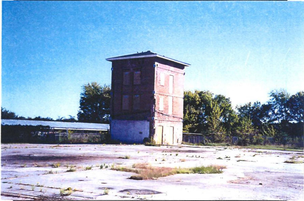
Photo 1. Control Tower Building
