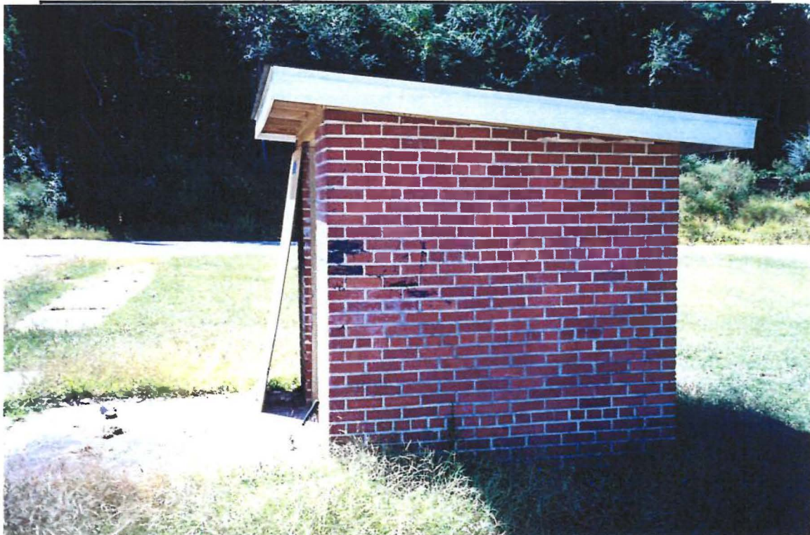
Photo 14. Fire Protection Shed – East Face
