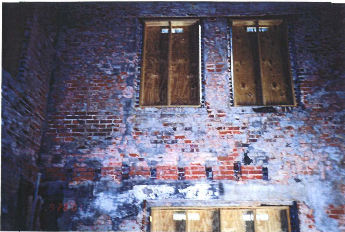
Photo 3. Control Tower Building – Interior North Face
