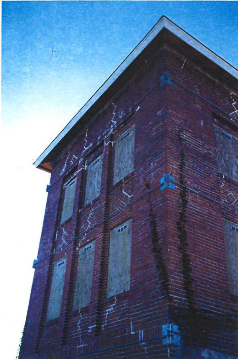
Photo 2. Control Tower Building – West Face
