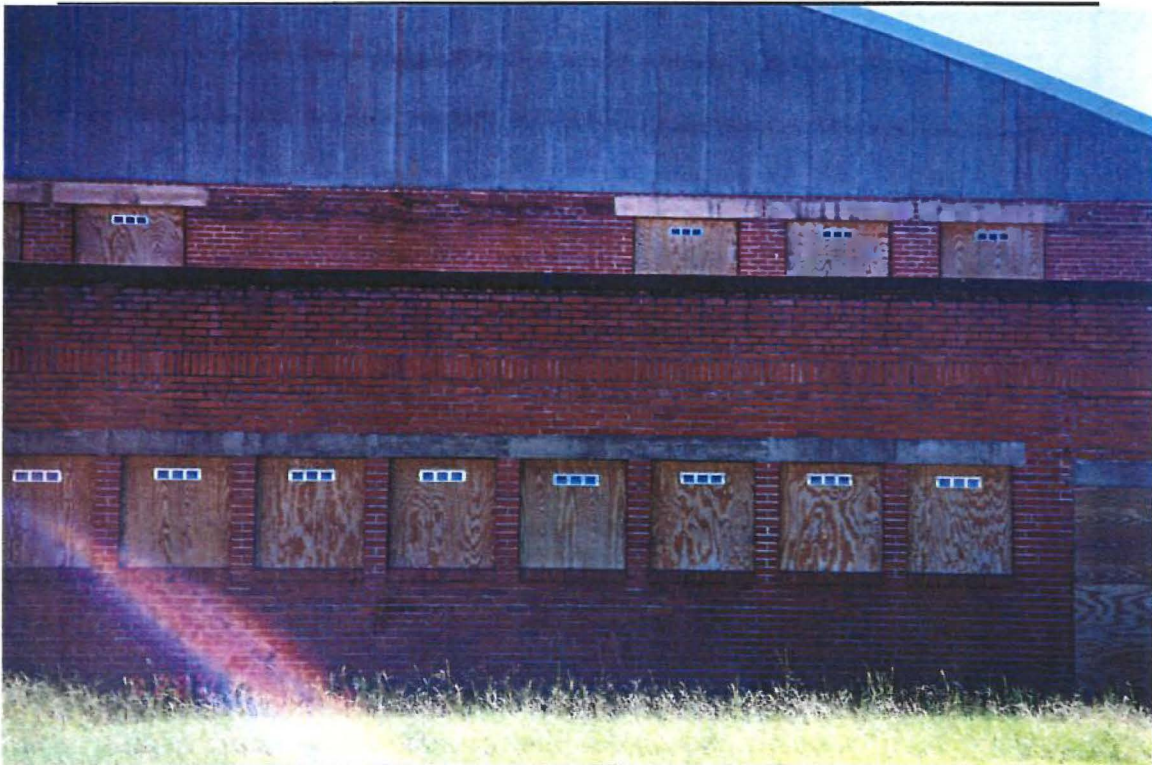
Photo 8. Hangar No. 1 – West Face
