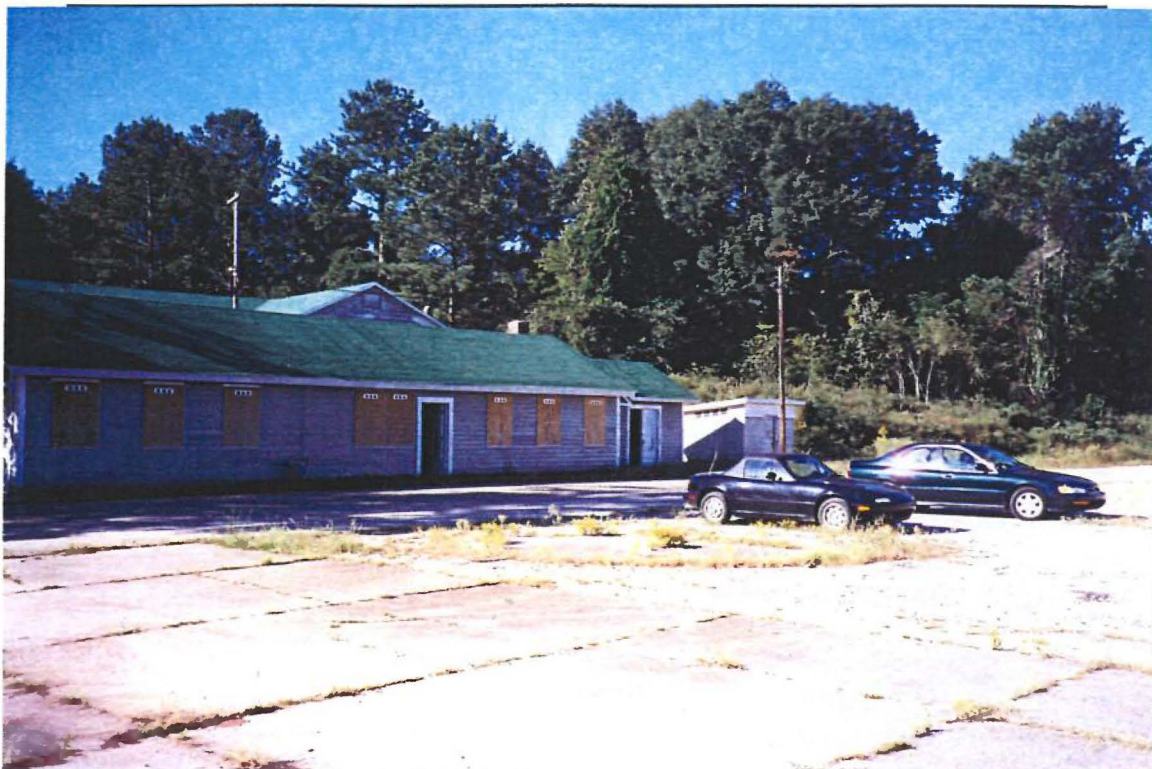
Photo 18. Bath and Locker House – East Face
