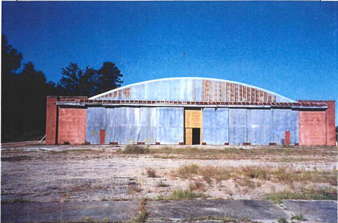
Photo 7. Hangar No. 1 – East Face
