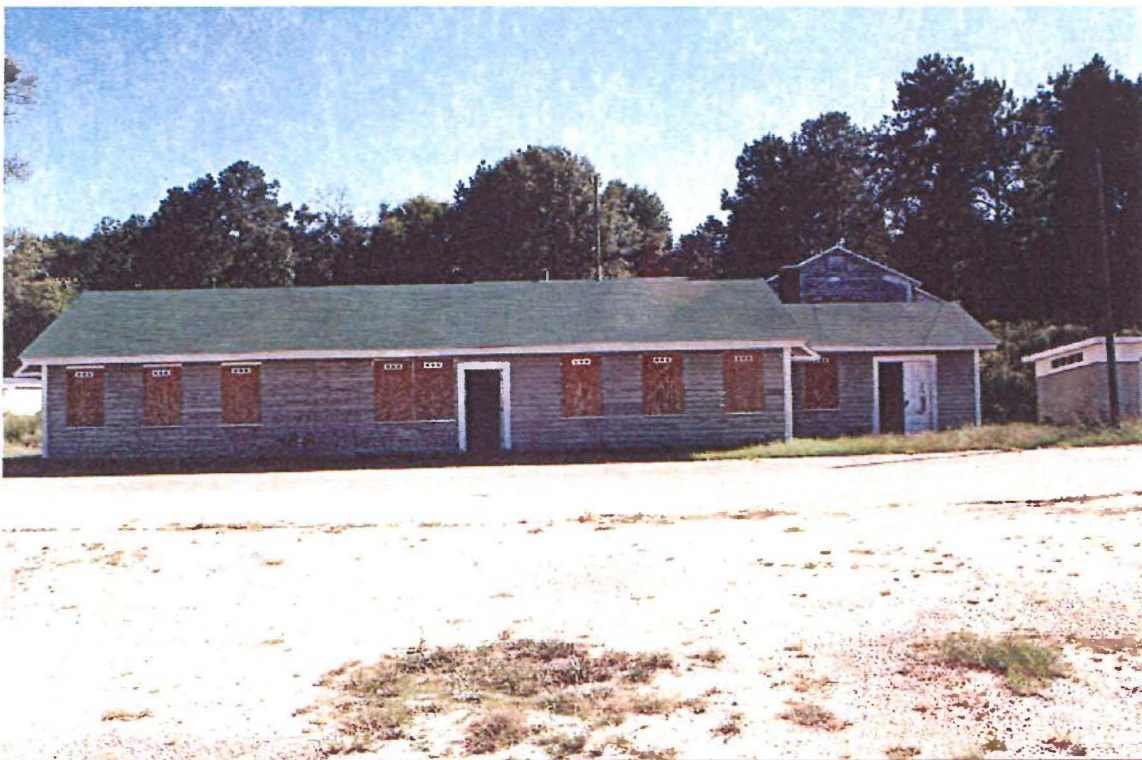
Figure 8: Existing north front facade.
