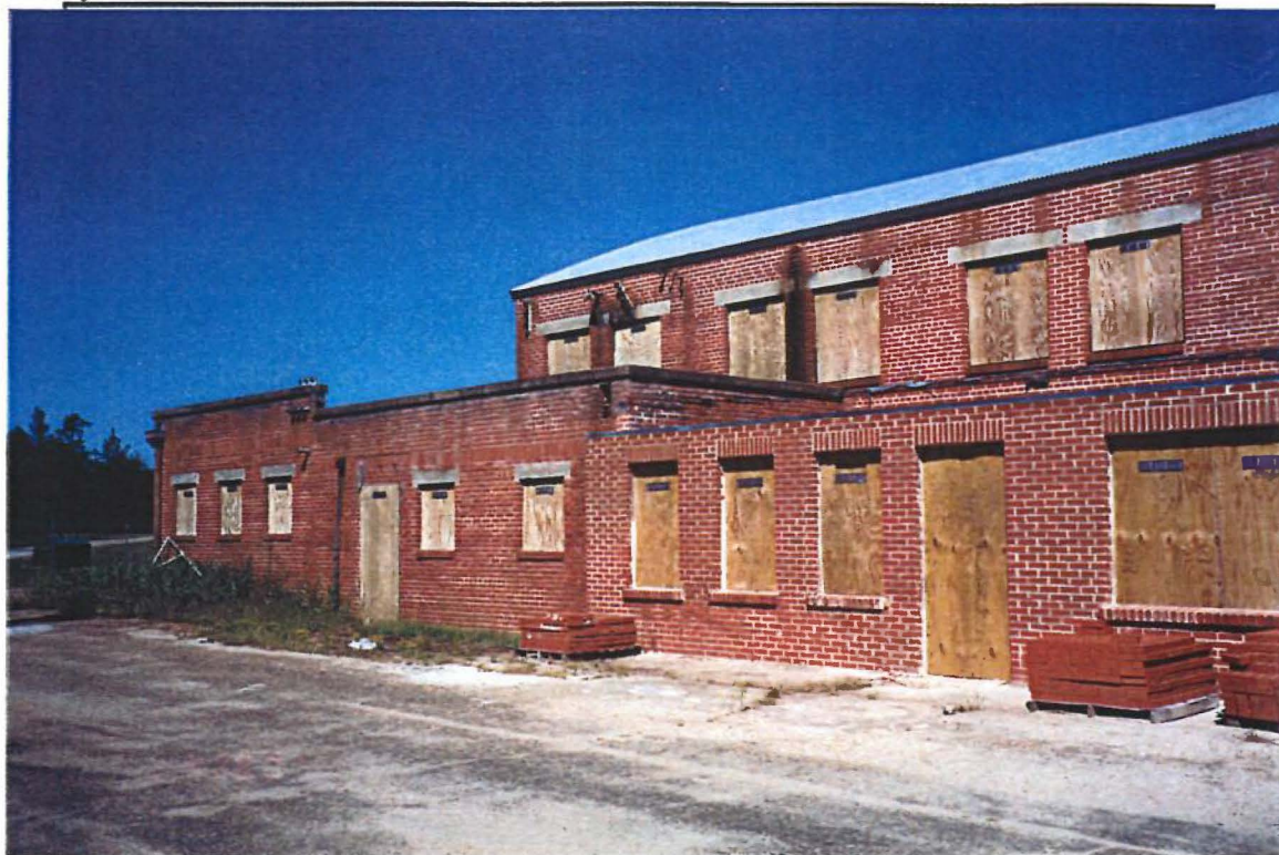
Photo 9. Hangar No. 1 – South Face
