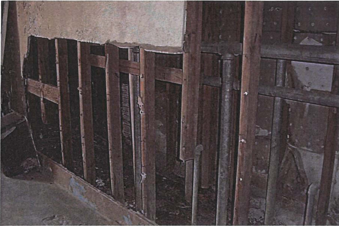
Figure 11: View of the plumbing chase that separates the men's and women's facilities.
