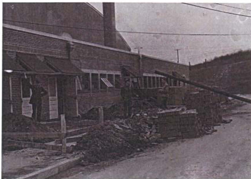
Figure 5: Construction of office addition to Hangar Number One c.1943/1944. From Moorland-Spingarn Research Center, Howard University.
