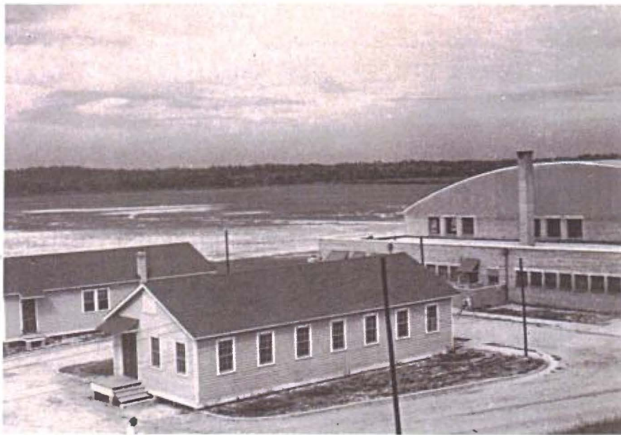
Figure 7: View of Army Supply Building, Flight Commanders Office, and Hangar Number One with curbing and utilities evident. From Moorland-Spingarn Research Center, Howard University.
