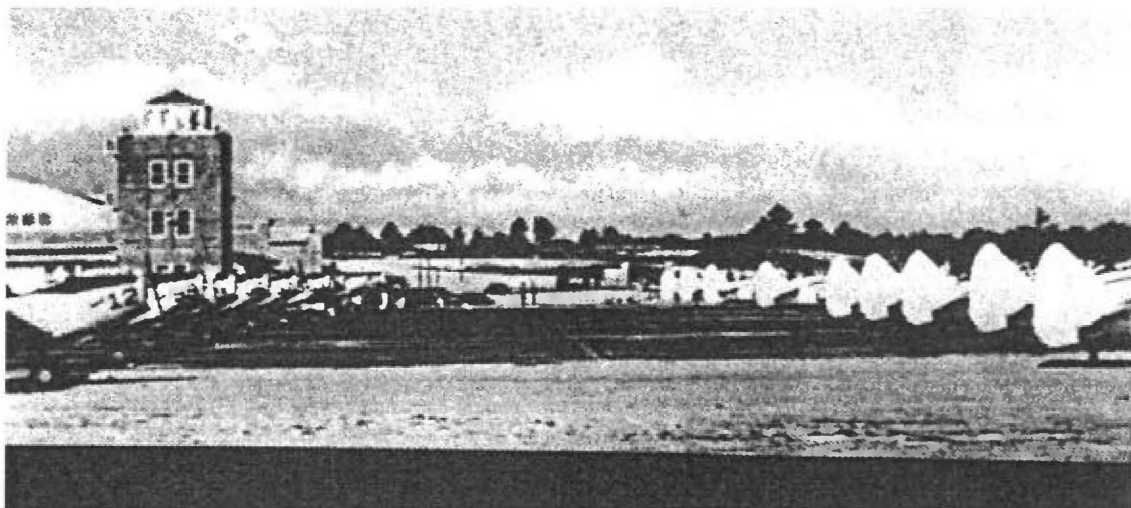
Figure 13: Parking Mat for plane Tie Downs North and East of Hangar Two c.1945. From Pilot Training School, Tuskegee Institute, Tuskegee Institute, Alabama. U.S. Army Air Forces Training Edition. May 1944. AFRHA, Maxwell AFB.
