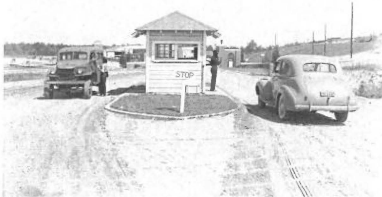
Figure 9: Guard Booth (looking east). Brick Entrance Gate in background, May 1944. From Pilot Training School, Tuskegee Institute, Tuskegee Alabama . U.S. Army Air Forces Training Edition, May 1944. AFHRA, Maxwell AFB.
