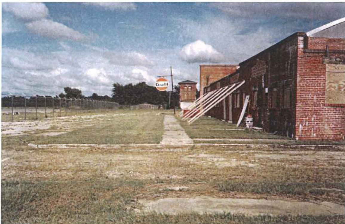
Figure 49: Historic Sidewalks and Curbing on north side of Hangar Number One.
