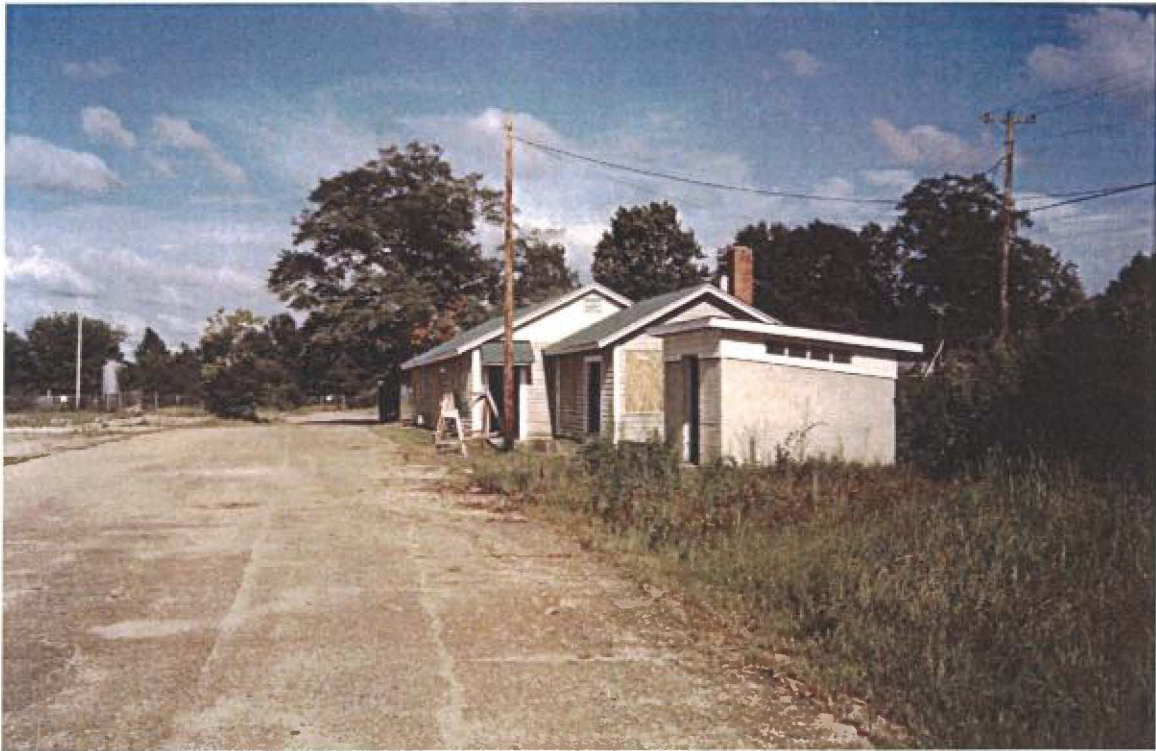
Figure 39: Utility Poles and Lines.
