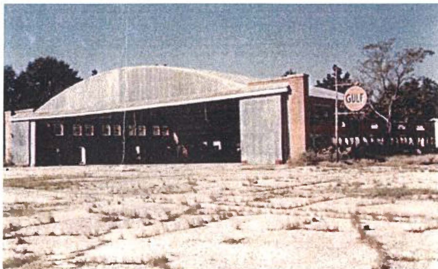
Figure 21: Original Gulf Sign at Northeast corner of Hangar Number One. (Current sign is a replacement version.) From Booker Conley's Photograph Collection.
