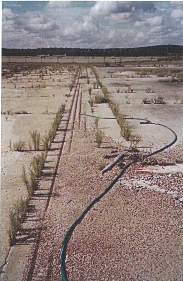
Figure 47: Metal Tracks for Sliding Doors of Hangar Number Two.
