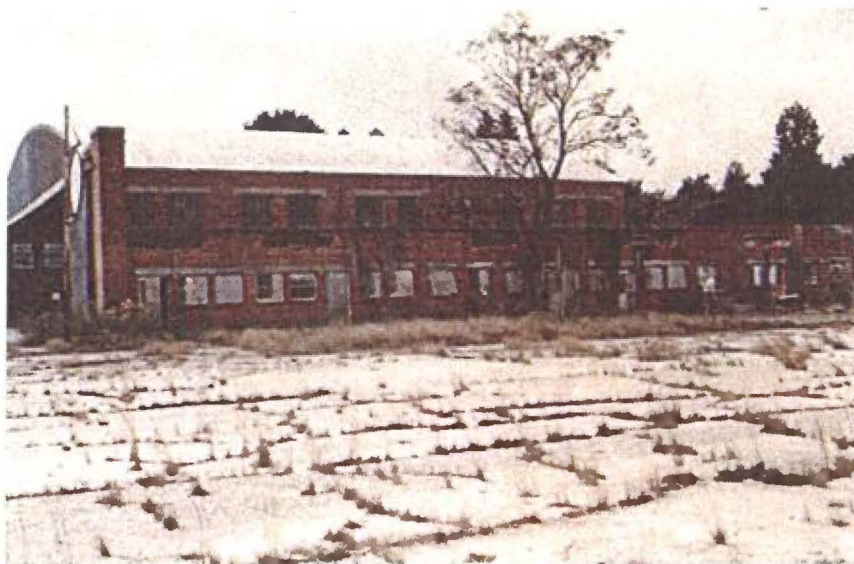
Figure 23: Post-War Deterioration of Hangars and Landscape features. From Booker Conley's Photograph Collection.
