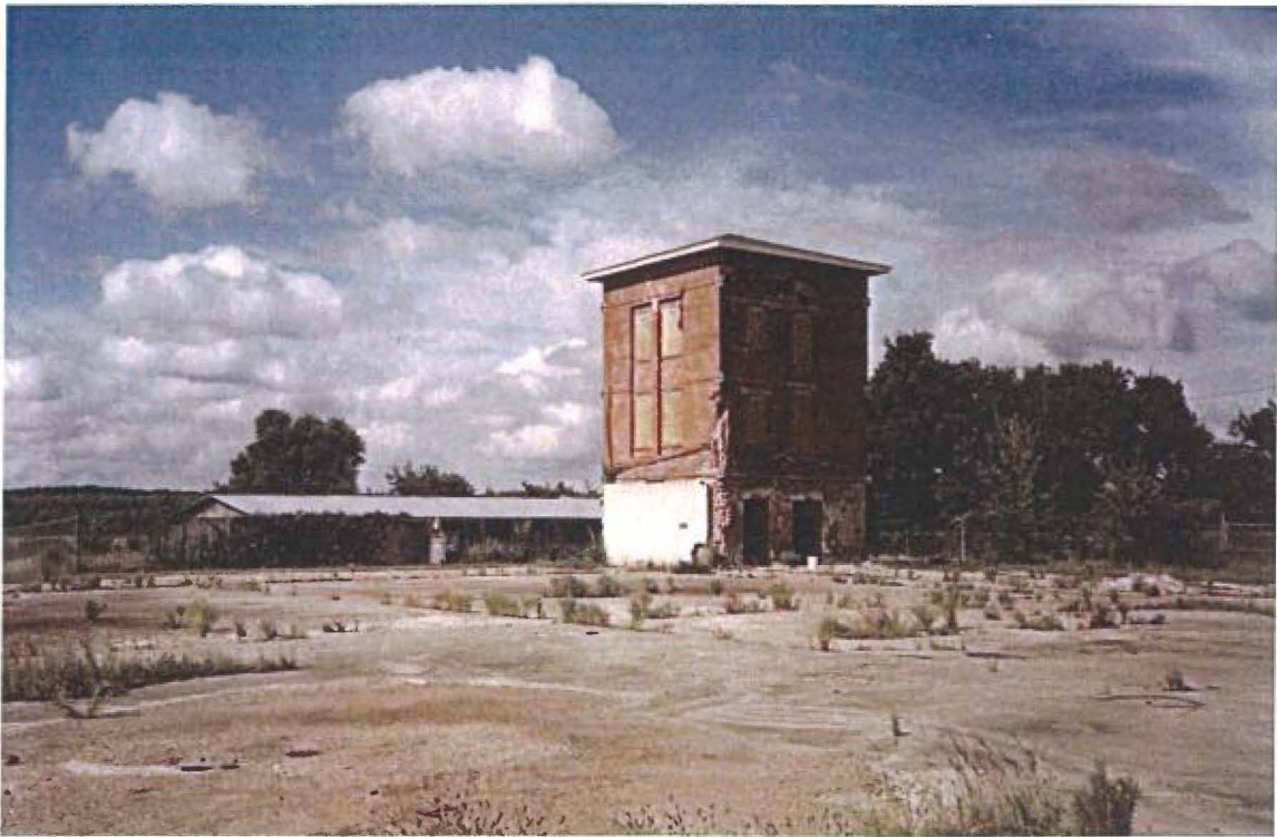
Figure 45: Vet School Facilities, Fencing.
