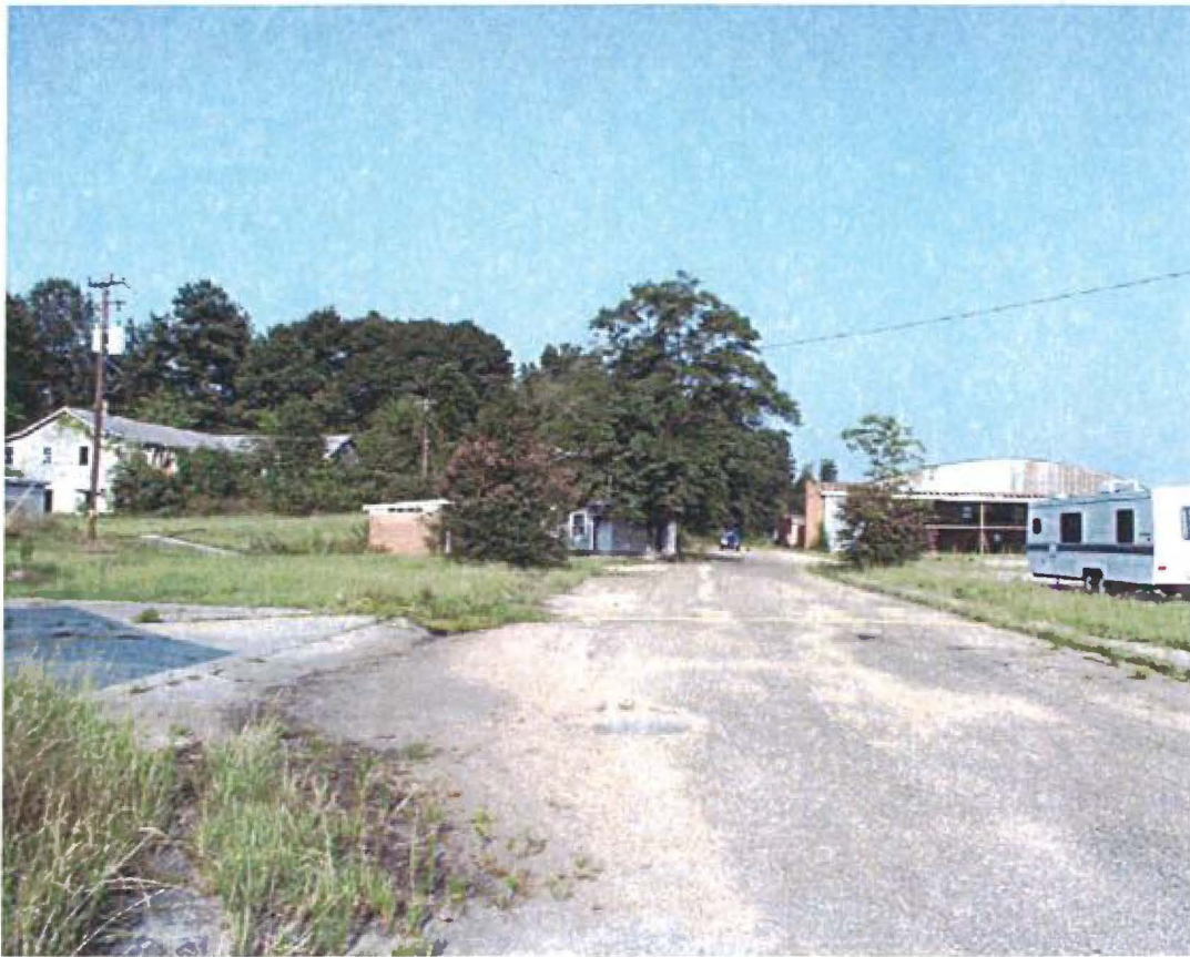
Figure 60: View of Site Pre-Stabilization.
