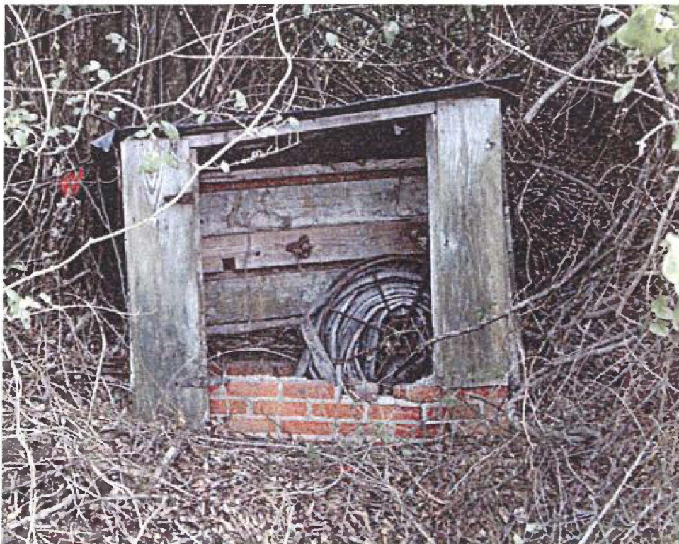
Figure 58: Fire Hose and Reel.
