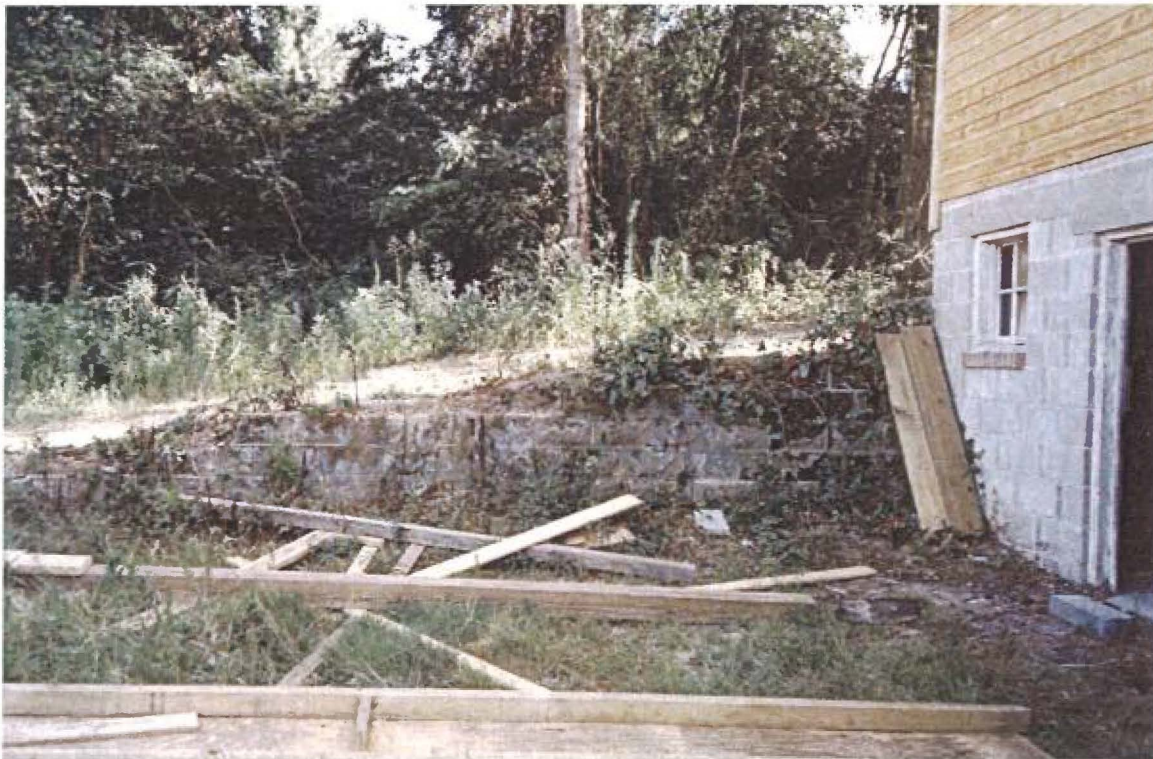
Figure 42: Skyway Club Block Retaining Walls.
