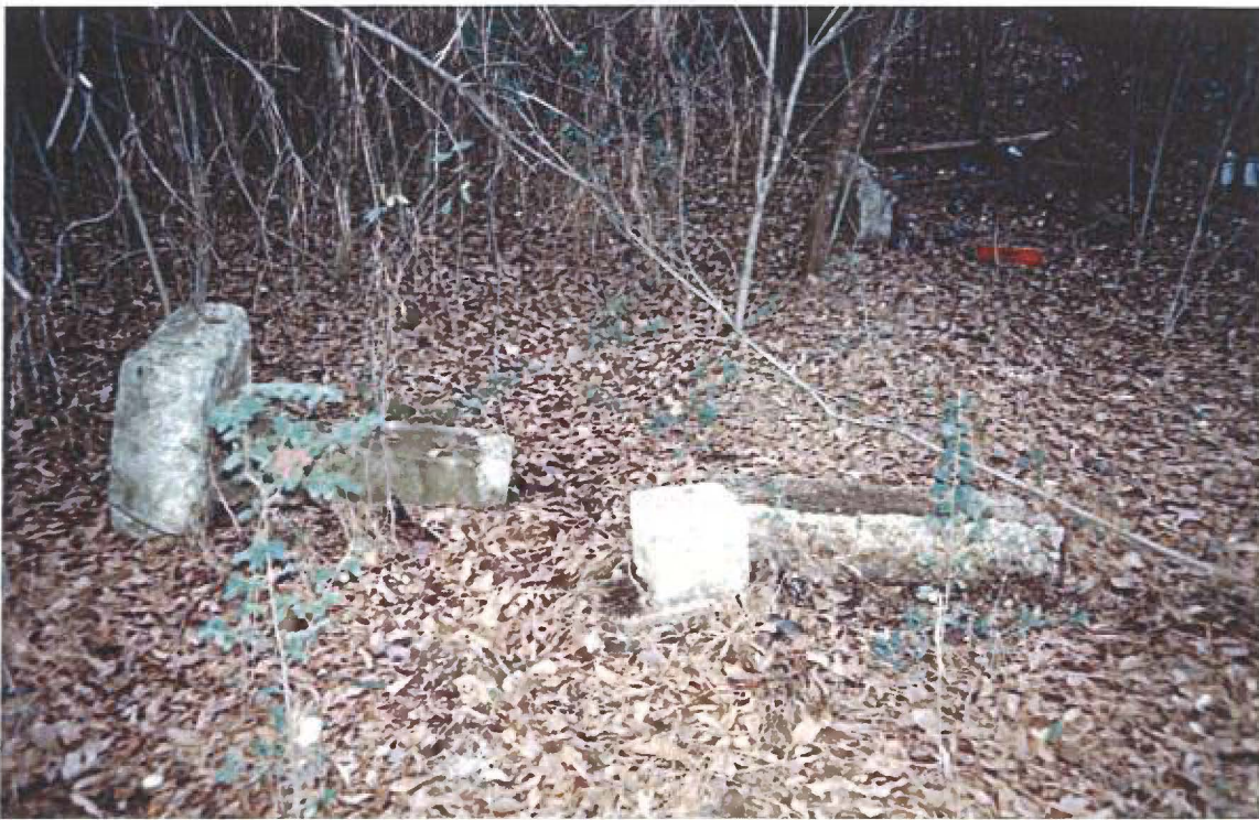
Figure 55: Concrete Stanchion; near Tennis Court, believed part of Spectator Seating.
