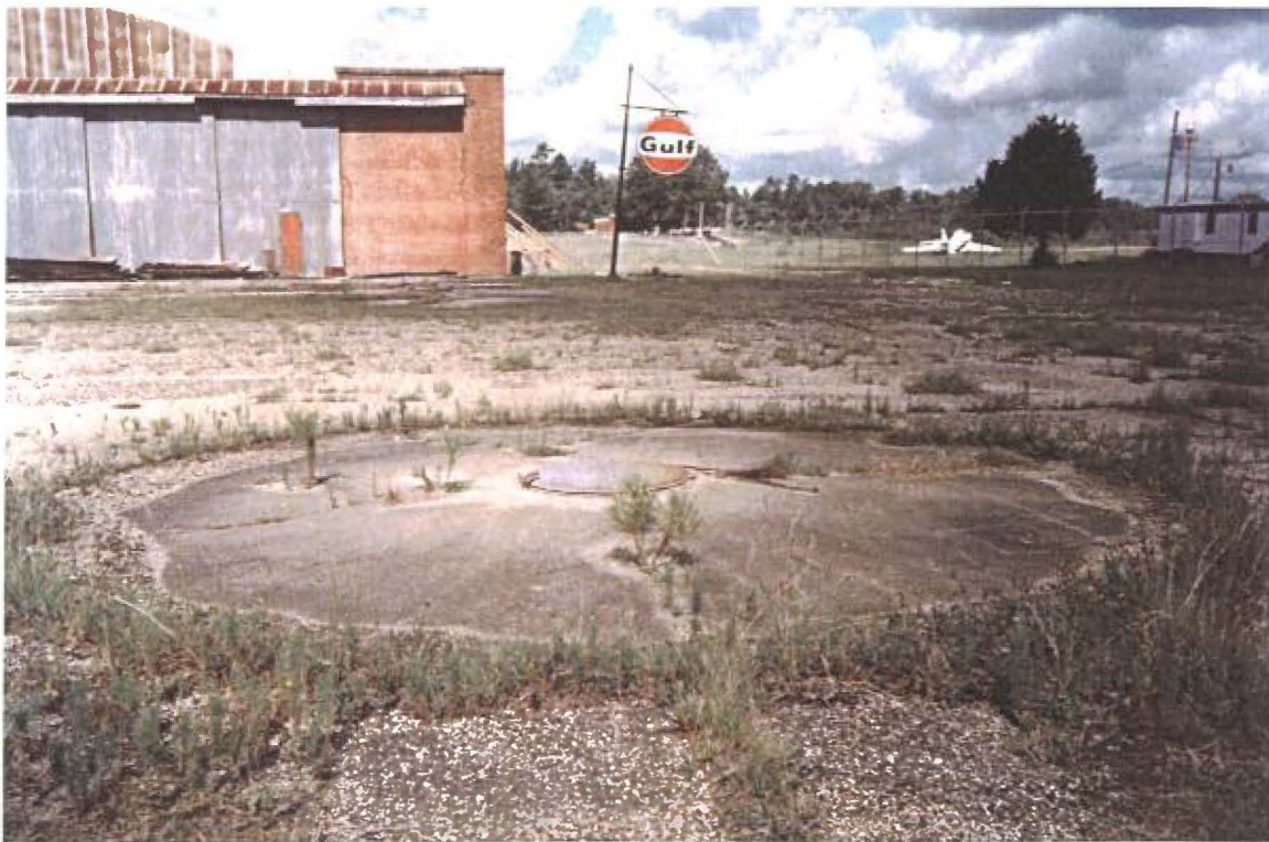
Figure 48: Underground Fuel Tank.
