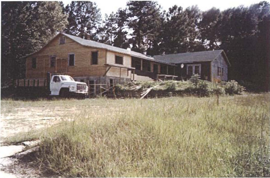
Figure 41: Skyway Club during stabilization, Historic Light Pole.
