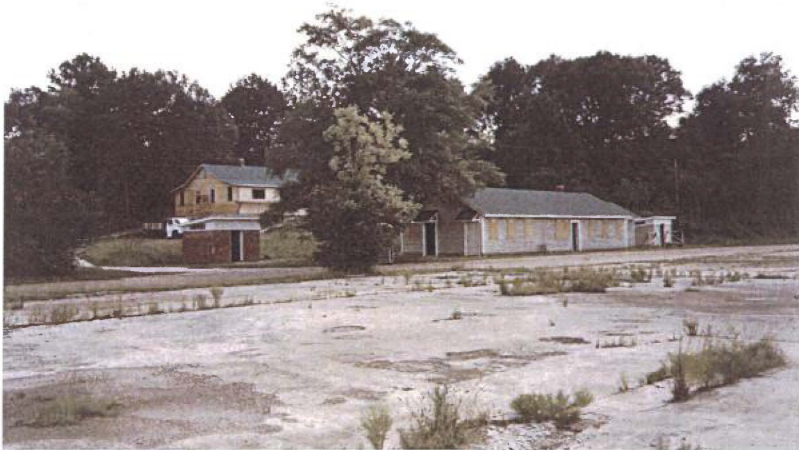
Figure 56: Heavily Vegetated Slope behind Skyway Club.
