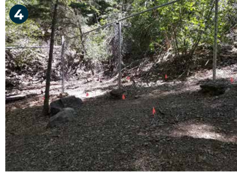
Existing fence to be removed.
