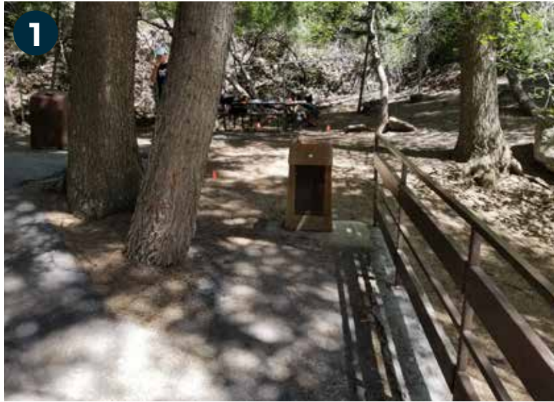
Existing drinking fountain to be removed.
