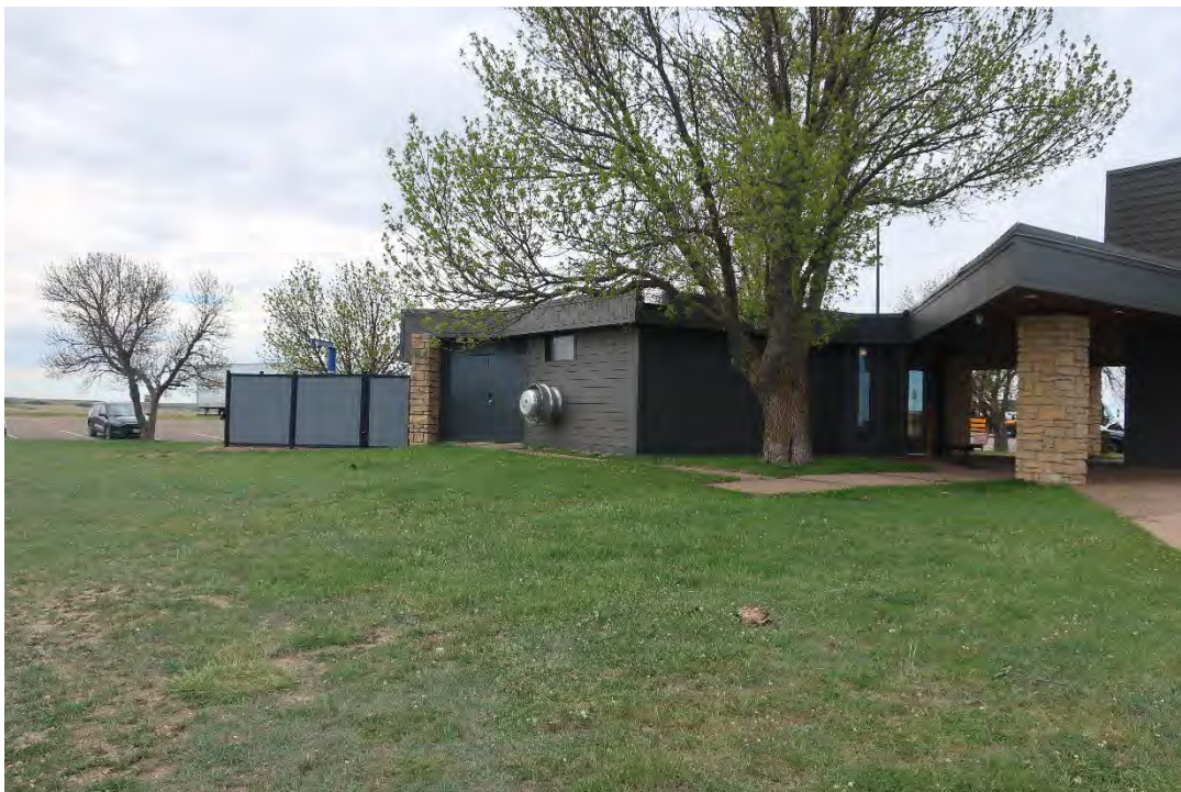
North elevation, Painted Canyon Comfort Station and Canopy, Theodore Roosevelt National Park. NPS photograph, May 2026.
