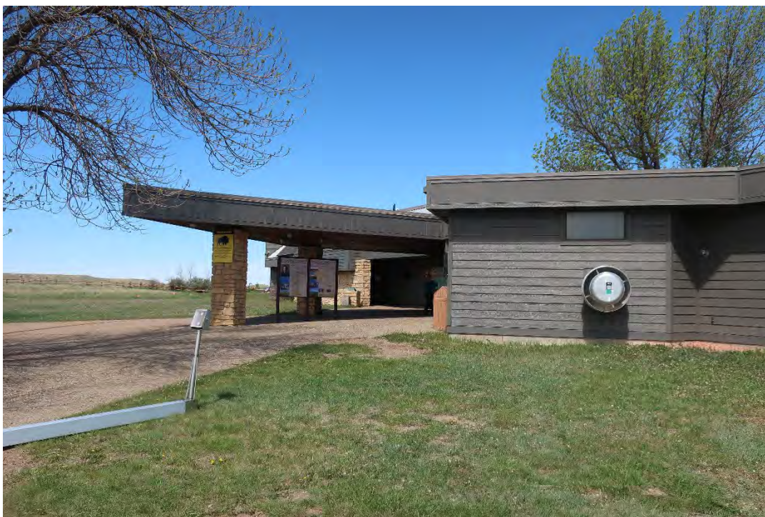
East elevation, Painted Canyon Comfort Station and Canopy, Theodore Roosevelt National Park. NPS photograph, May 2026.
