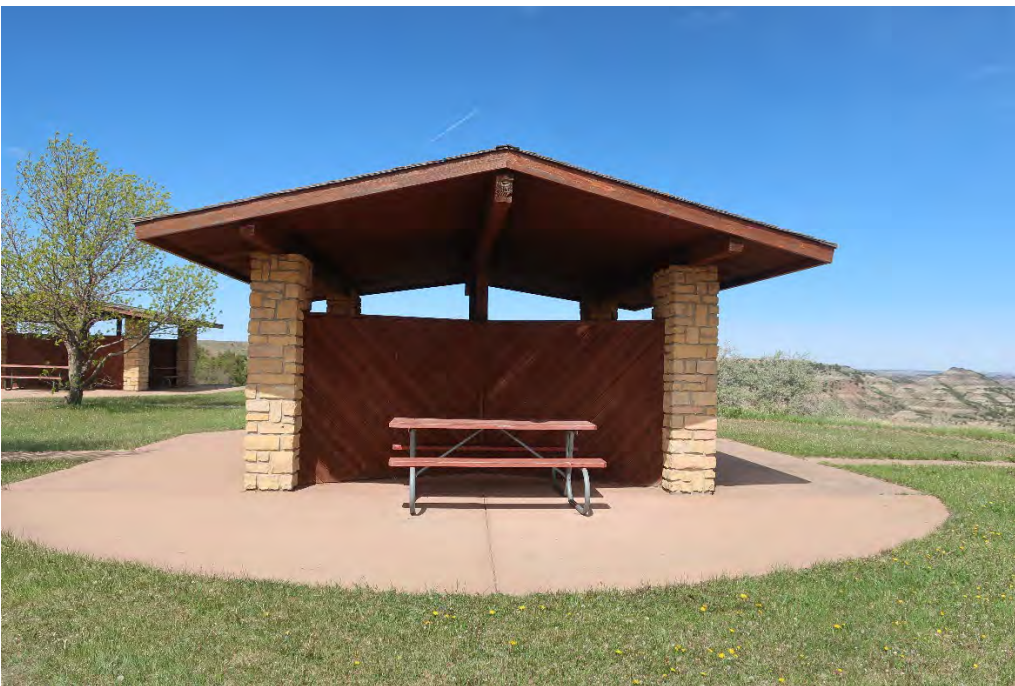
Facing west, West Elevation of Picnic Shelter with Second Shelter in Background, Theodore Roosevelt National Park. NPS, photograph, May 2026.
