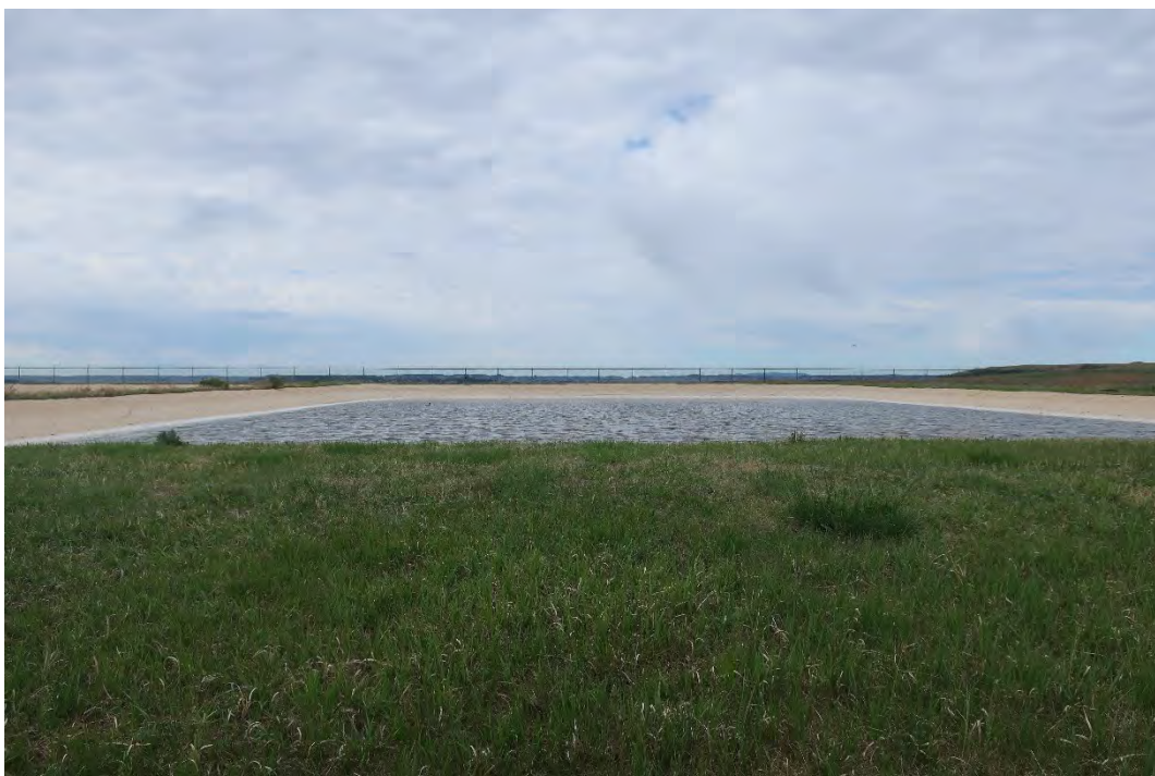
Facing south, Center Wastewater Lagoon, Theodore Roosevelt National Park, NPS photograph, May 2026.
