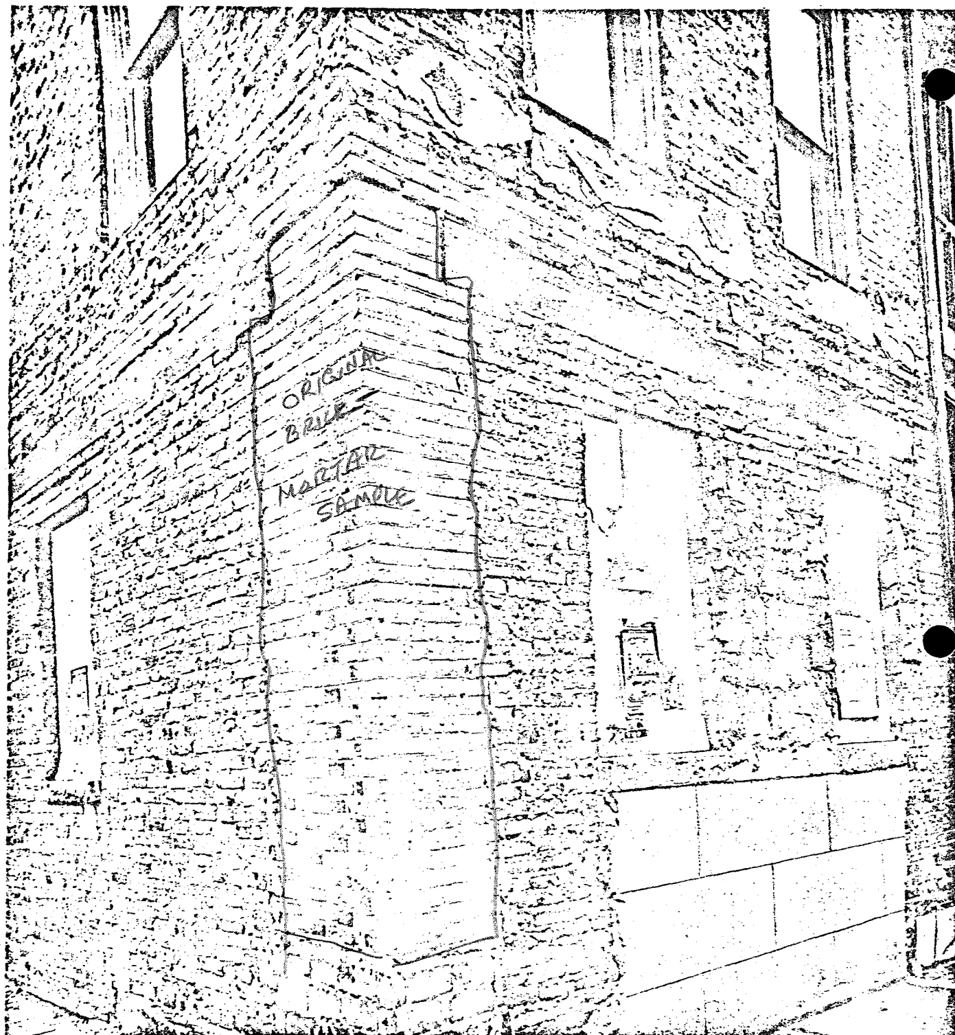
301 Pine Street, Exterior Corner: Pine Street is to the left, Third Street is to the right. Original brickwork starts at about two feet from the ground. Probably the first floor corner pier is original. The two wooden girders show where stone windows had once been. It is easily seen where "newer" brickwork has been filled into what had been the bulk window.
