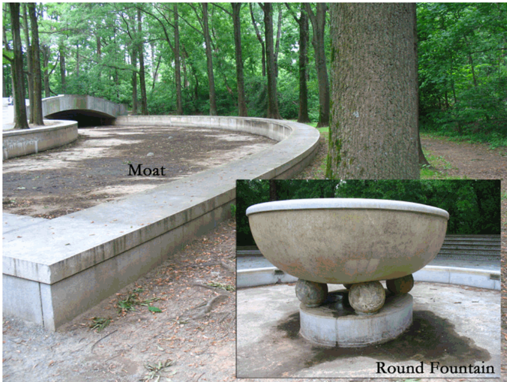
The two contributing constructed water features on the site are the large moats and the shallow round fountains (NCR CLP 2010).
