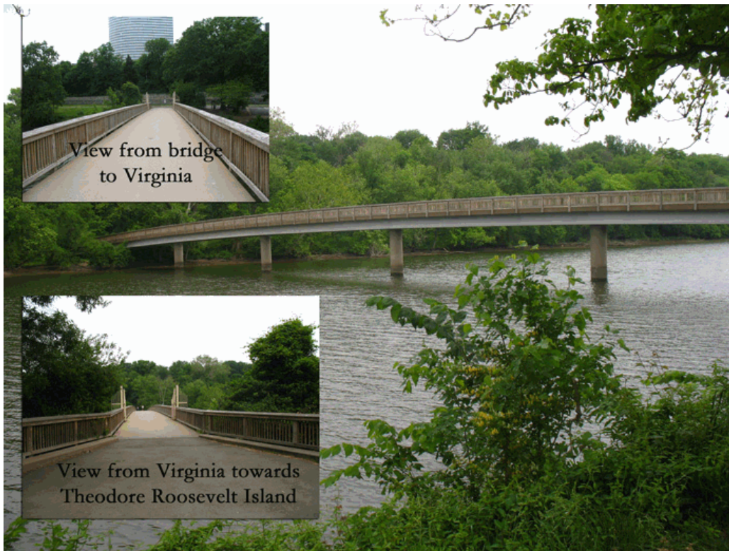
The pedestrian bridge, built in 1979, provides access to the island from the Virginia shore. Since it was built outside of the period of significance, it is considered a non-contributing resource (NCR CLP 2010).
