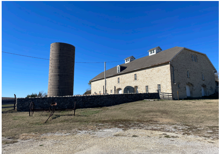
Figure 3-4. Overview of barn, silo, and corral looking northwest (QE, 2023).
