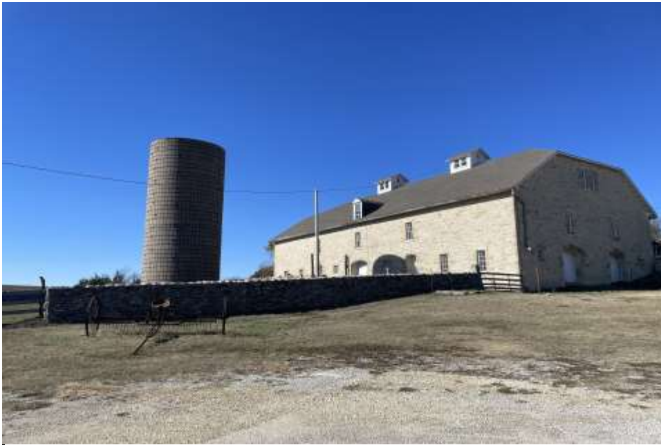
Figure 3. Overview of barn, silo, and corral looking northwest. October 31, 2023.
