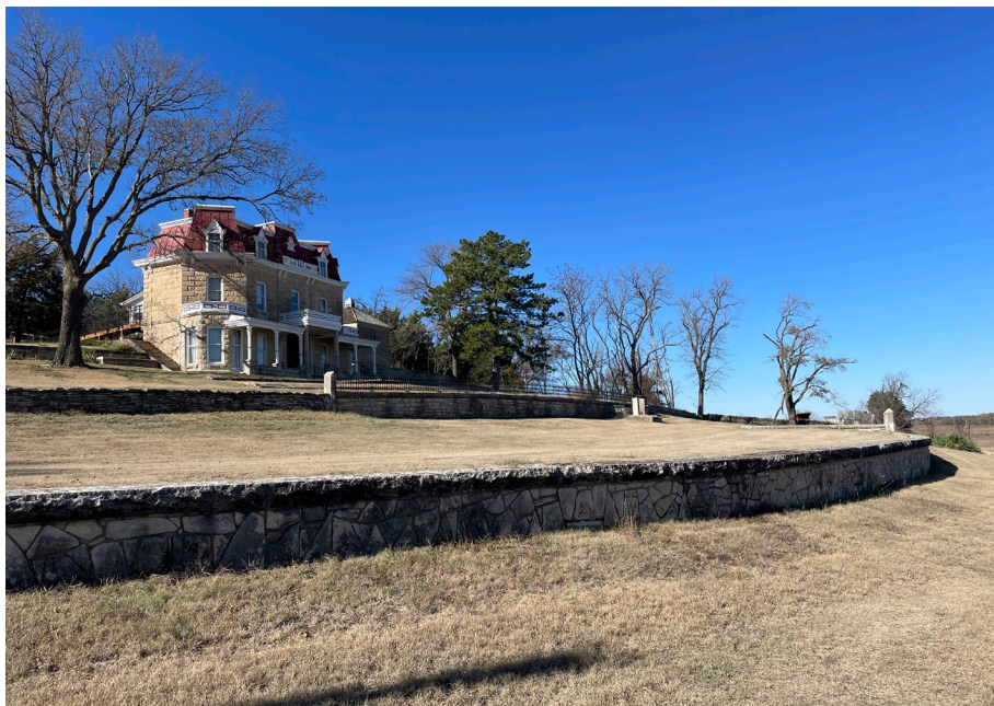
Figure 3-1. Overview of house and lawn, including stone fencing and terracing, looking northwest (QE, 2023).
