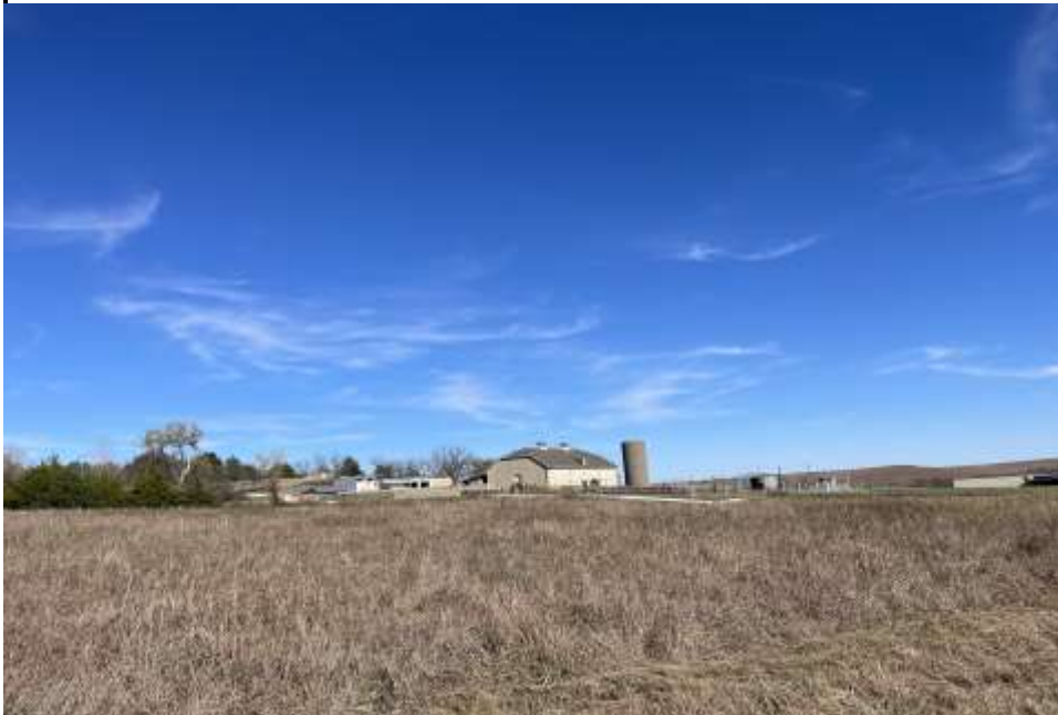
Figure 4. Overview of the ranch headquarters, looking northeast. October 31, 2023.
