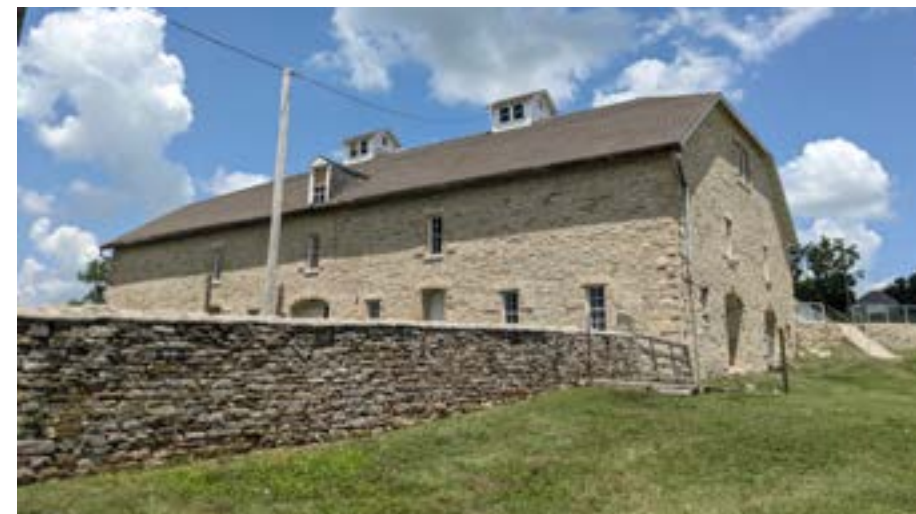
Figure 6-1. Eastern and southern facade of the Spring Hill Barn (Vireo, 2024).
