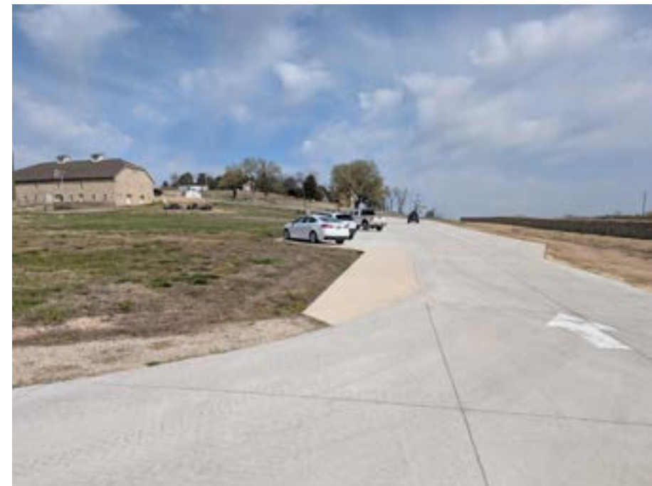
Figure 3-5. Paved parking lot, completed in 2020 (Vireo, 2024).
