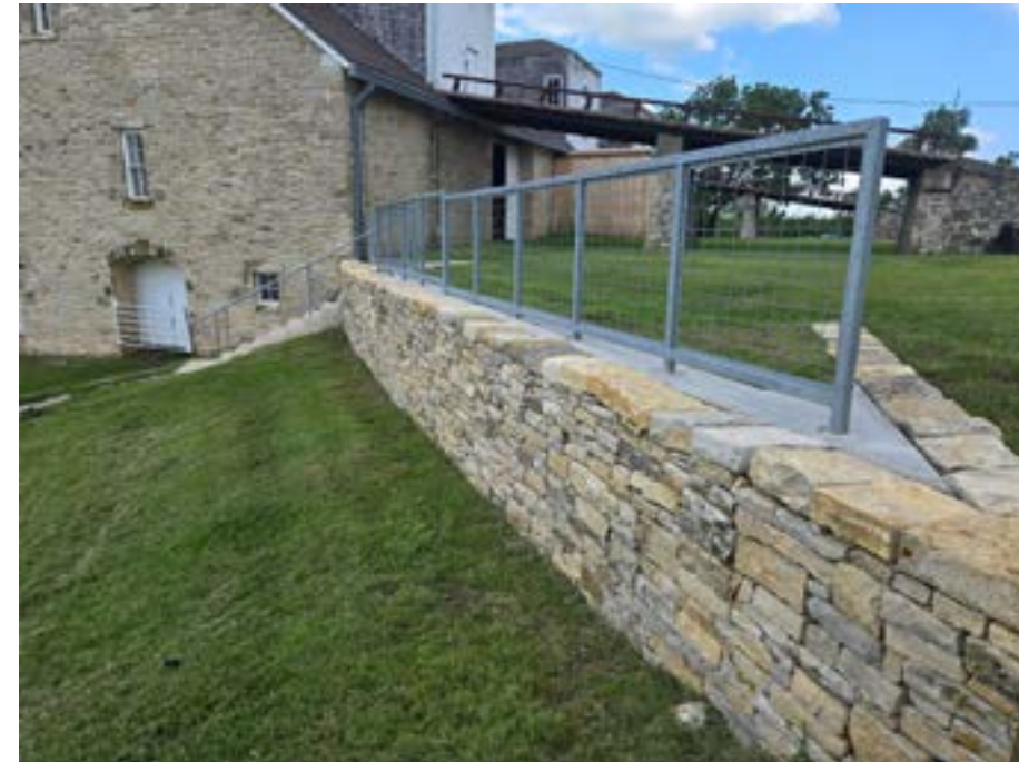
Figure 3-4. Reconstructed stone veneer retaining wall and steps, completed in 2020 (Vireo, 2024).
