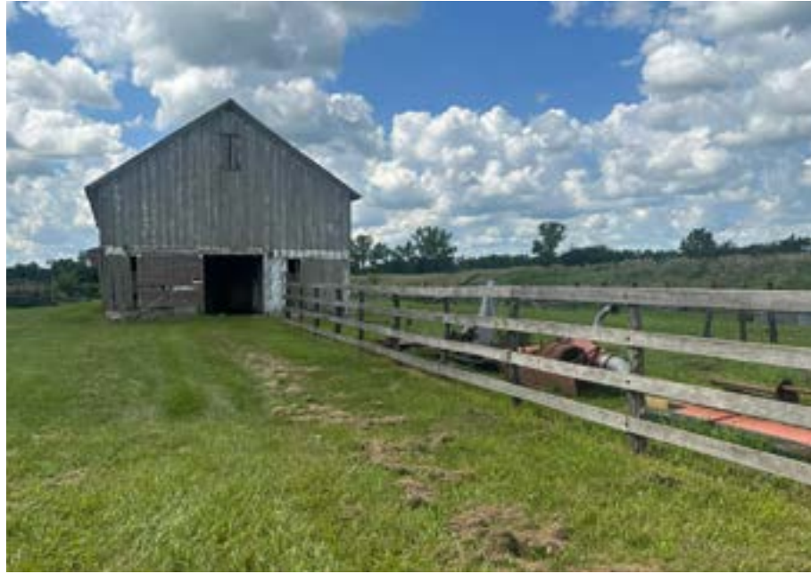
Figure 6-10. Existing four-rail fence to remain (Affinis, 2024).
