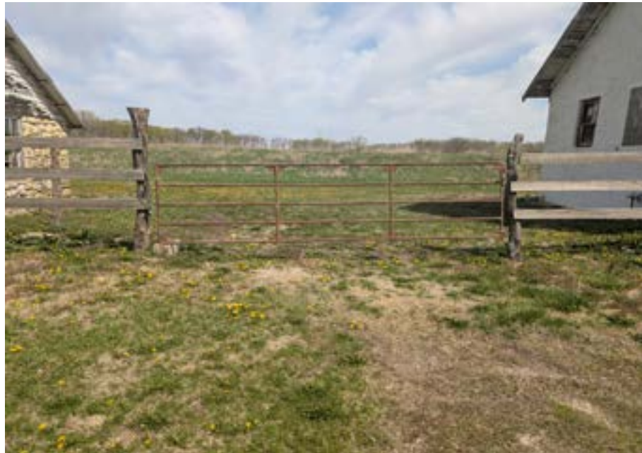
Figure 6-11. Existing steel gate to be replaced with custom swing gate (Vireo, 2025)
