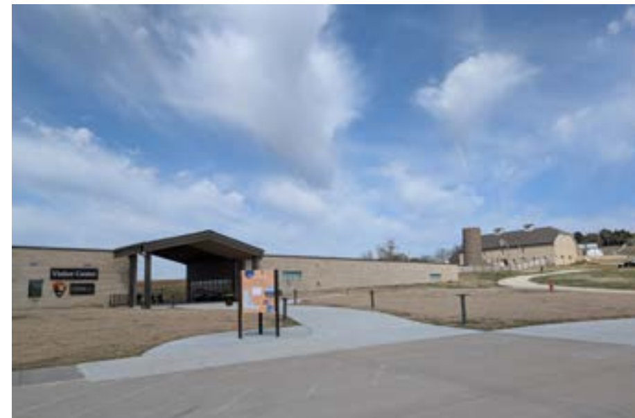
Figure 3-1. Visitor's Center and Park Headquarters, completed in 2012 (Vireo, 2025).
