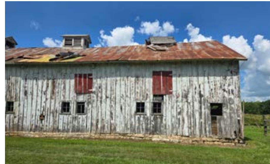
Figure 6-6. Deer Park Place Barn eastern facade (Vireo, 2024).
