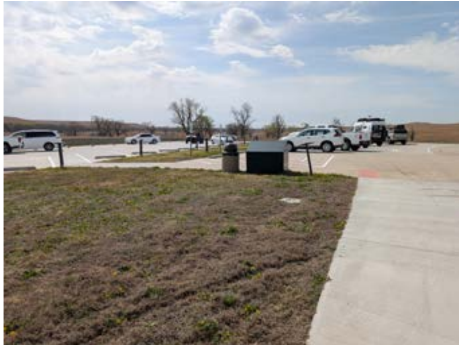
Figure 3-2. Paved Visitor's Center parking with accessible spots, completed in 2012. (Vireo, 2025).
