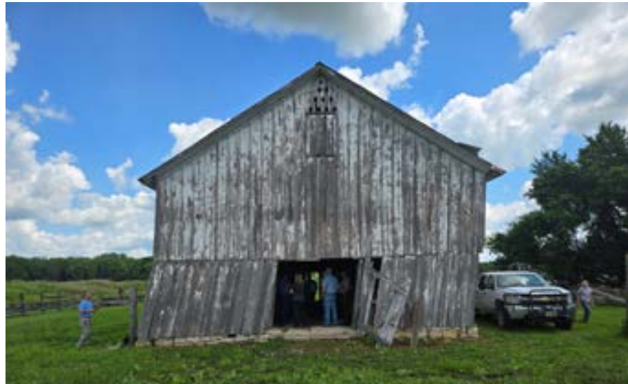
Figure 6-5. Deer Park Place Barn southern facade (Vireo, 2024).
