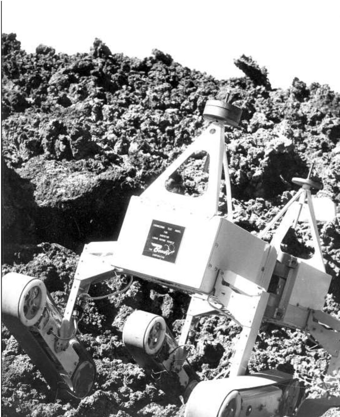
Fig. 75. Bendix prototype Surveyor Lunar Roving Vehicle on the Bonito Lava Flow, May, 1964. (Image from Schaber, open-file report, 2005.)
