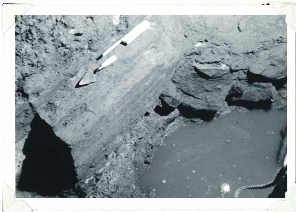
Figure 12. Stone and brick and boulder wall in east wall of excavation unit around column #8.
