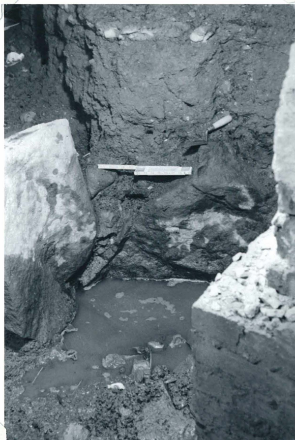
Figure 11. Detail of boulder portion of wall between columns # 13 and 29.
