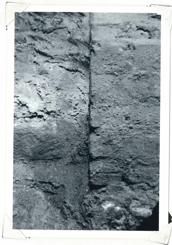
Figure 13. Detail of junction between stone and brick portions of wall in excavation unit around column #8 (eastern profile of wall; stone portion is 24 inches in height).
