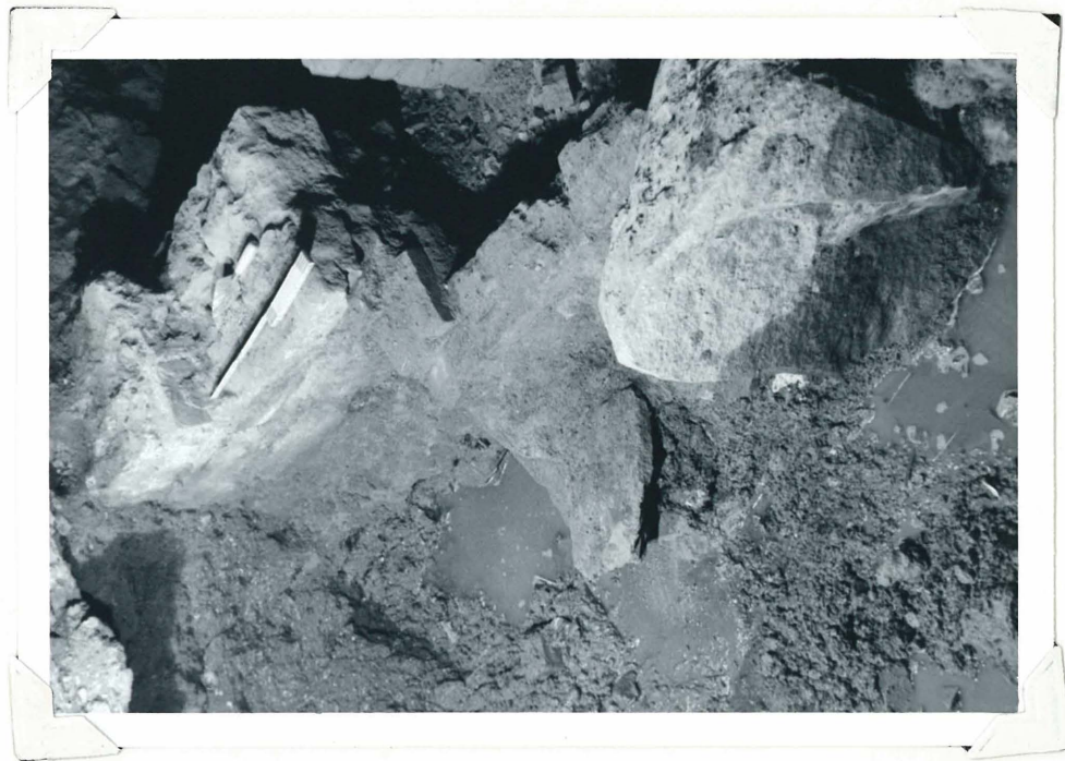
Figure 10. Stone and brick and boulder wall between columns # 13 and 29.
