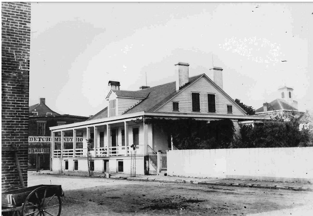
Figure 2. c. 1890s photograph of the Jean Baptiste Vallé House from the northeast, with the corner of the Lagrave Building (58 South Main Street) at left. (Source: Missouri Historical Society, https://mohistory.org/society ; a slightly cropped version also appears in Houck's History of Missouri , Vol. I, 350)
