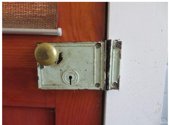
Figure 107. Interior rim lock and door knob for Door 108. (Source: RRJ, 2022)
