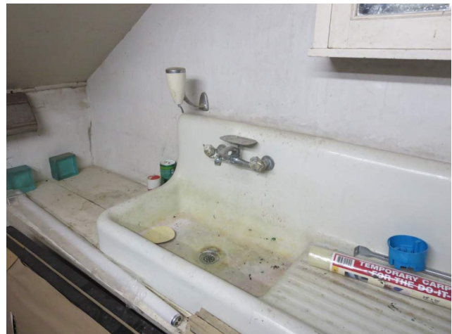
Figure 273. Existing old sink located at the basement level of the house. (Source: Alvine, 2022)
