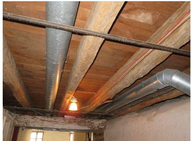
Figure 145. Overview of joists within Room 005. (Source: RRJ, 2022)
