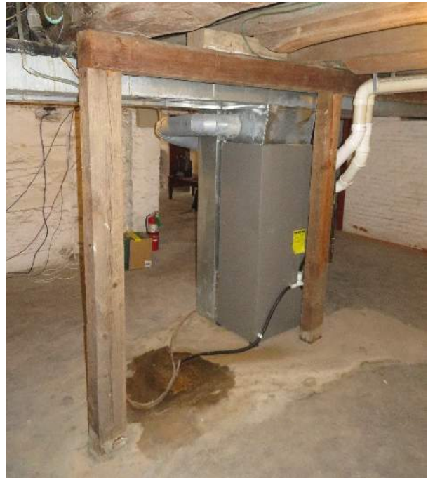
Figure 166. Supplemental framing. (Source: RRJ, 2022)
