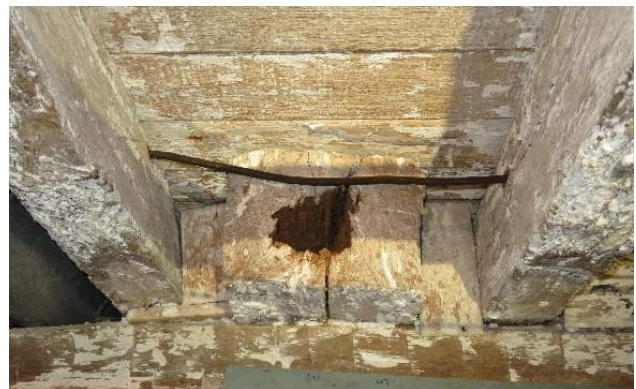
Figure 169. Hollow joist viewed from room 006. (Source: RRJ, 2022).
