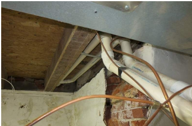
Figure 306. Existing flue and combustion air piping up high in basement level from northwest furnace. (Source: Alvine, 2022)
