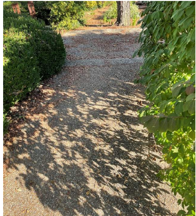
Figure 376. View to the connecting walkway that needs to be reached via an accessible ramp and level landing at grade. (Source: LSHLA, 2022).
