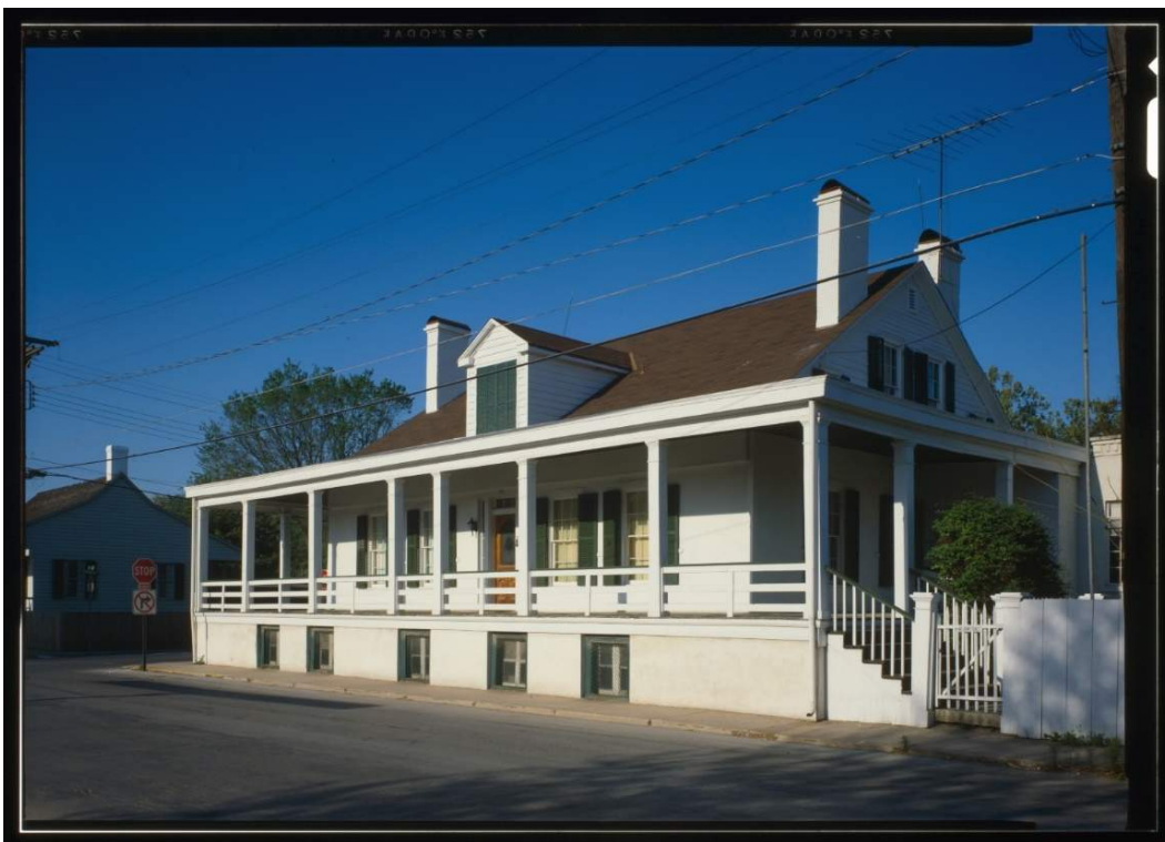
Figure 74. 1986, view of the house from the northeast on Main Street. (Source: Historic American Buildings Survey, Library of Congress, Call no. HABS MO,97-SAIGEN,1-). https://www.loc.gov/item/mo0360/ )
