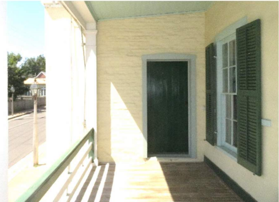
Figure 112. Exterior of Door 113B. The interior has been walled off and this door does not provide access to the house (Source: RRJ, 2022)
