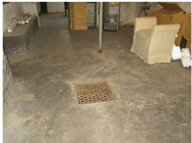
Figure 130. Slab-on-grade and floor drain in Room 003. (Source: RRJ, 2022).
