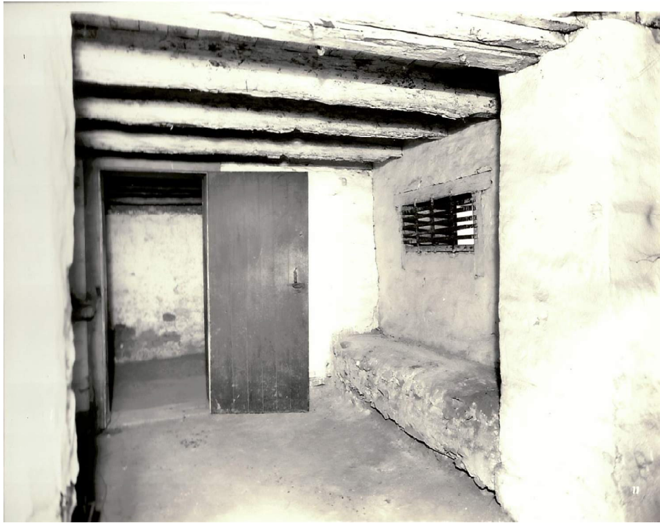
Figure 25. Undated (possibly before 1960s renovations), Room 001, looking north towards Door D002. Note the thickened stone masonry at the base of the foundation wall at right. (Source: Schram Collection, Felix Vallé State Historic Site)
