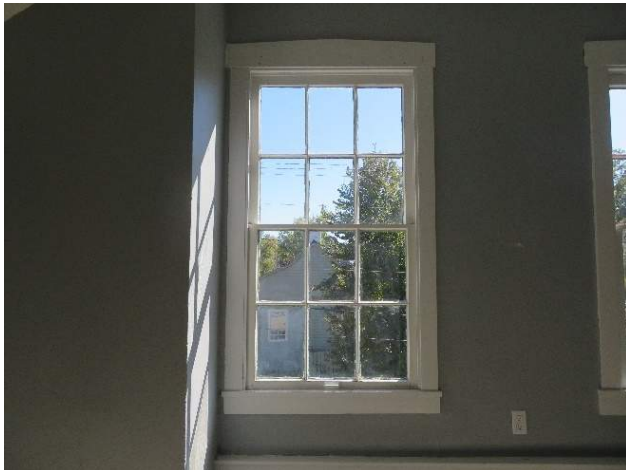
Figure 91. Interior view of Six-over-six double hung wood windows typical of first floor windows (Source: RRJ, 2022).
