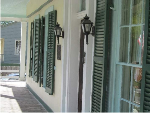
Figure 362. Incandescent wall-mounted sconces on the east porch. (Source: Alvine, 2022)
