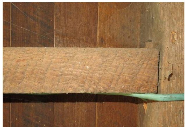
Figure 138. Pit saw marks at joist underside. (Source: RRJ, 2022).
