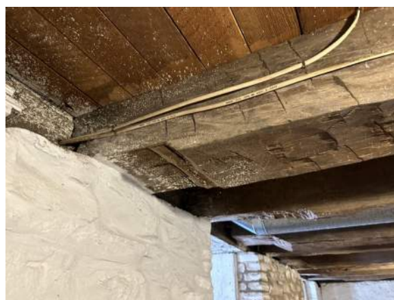
Figure 10. Samples 8, 9, and 10. Beams in Rooms 11, 11A, and 11B, white oak.
