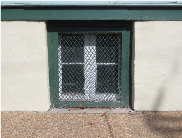
Figure 88. Exterior view of typical basement level Casement Window with metal mesh covering (Source: RRJ, 2022)
