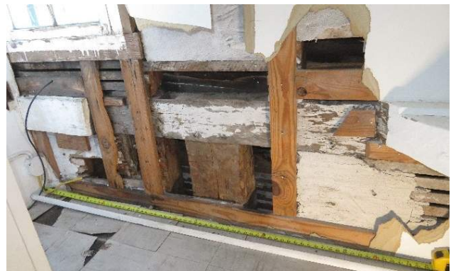
Figure 243. Exposed vertical logs in Room 208. (Source: RRJ, 2022).
