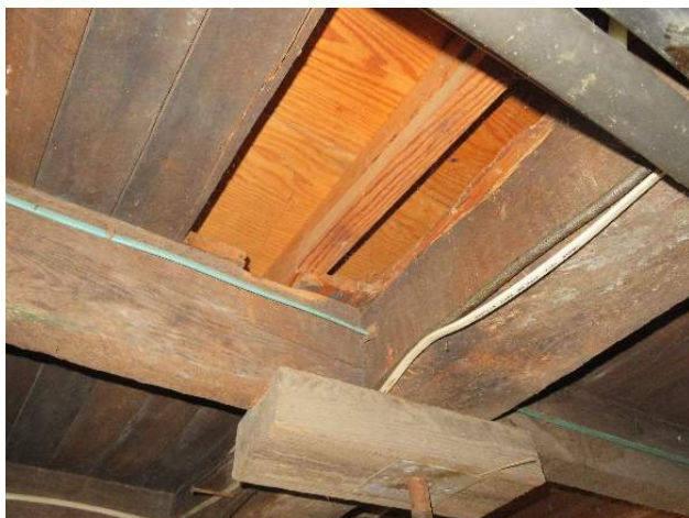
Figure 141. Additional decking and framing above subfloor. (Source: RRJ, 2022).
