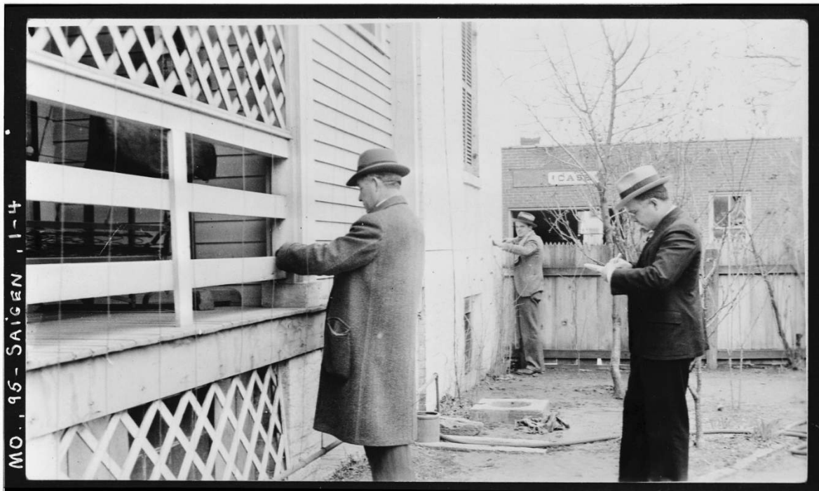
Figure 12. 1934, west exterior wall, looking south. (Source: Historic American Buildings Survey, Library of Congress, Call no. HABS MO,97-SAIGEN,1-). https://www.loc.gov/item/mo0360/ )
