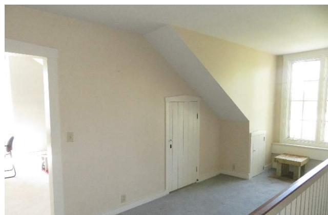
Figure 227. One of two small storage spaces that flank the area west of stairs in Room 201. (Source: RRJ, 2022).
