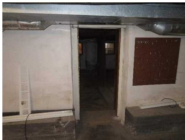
Figure 124. A Supplemental concrete foundation within Room 003. (Source: RRJ, 2022).
