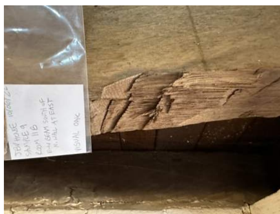
Figure 12. Sample 9. Room 11B, beam, white oak.
