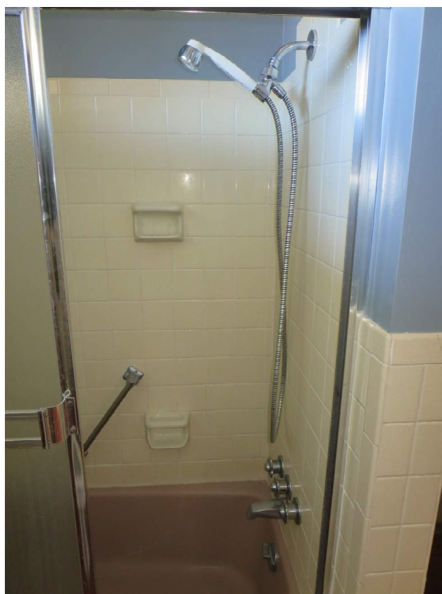
Figure 271. Existing shower at First level restroom. (Source: Alvine, 2022)
