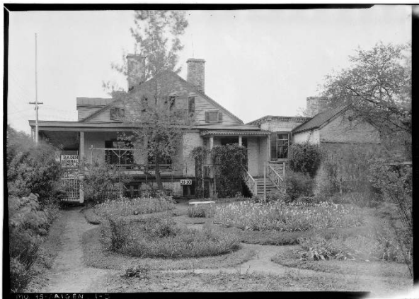
Figure 16. 1933 photograph of the Jean Baptiste Vallé House from the north. (Source: HABS)
