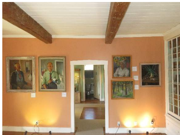
Figure 177. Exposed joists in Room 103, view looking west. (Source: RRJ, 2022)
