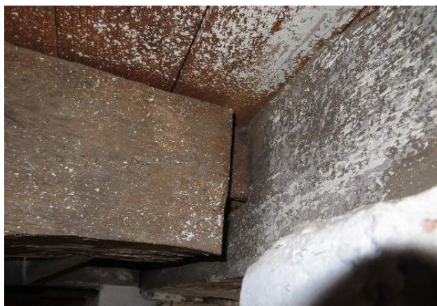
Figure 164. Half-dovetail lap joint at southeast corner. (Source: RRJ, 2022).
