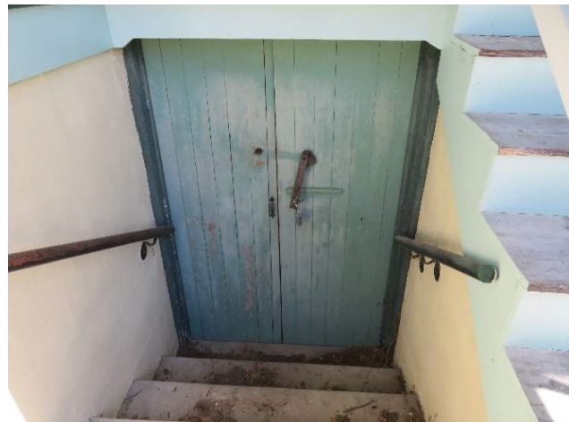
Figure 98. Exterior of basement entrance, Door D001. (Source: RRJ, 2022)
