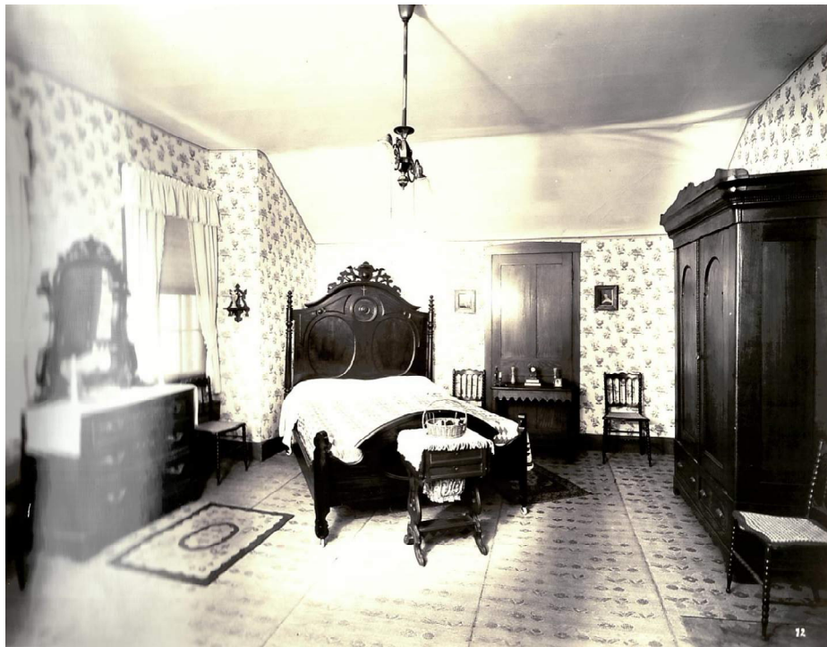
Figure 29. Undated (possibly before 1960s renovations), Room 207, looking east. (Source: Schram Collection, Felix Vallé State Historic Site)
