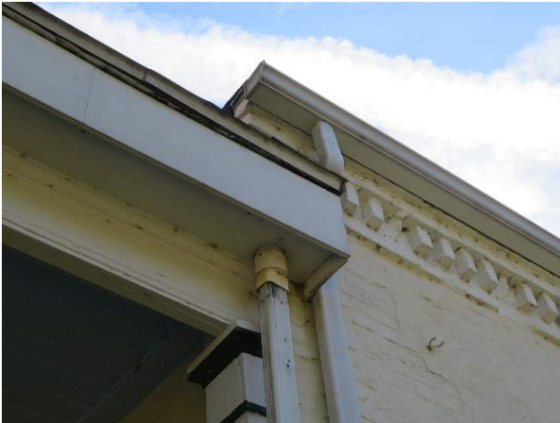
Figure 78. Downspout at roof eave. (Source: RRJ, 2022).
