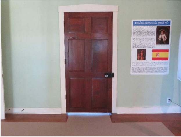
Figure 251. Door D104B seen from Room 104. (Source: RRJ, 2022)
