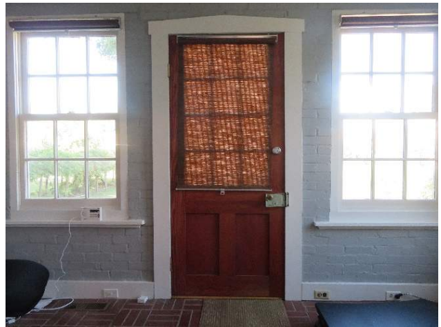
Figure 106. Interior of Door D108. (Source: RRJ, 2022)
