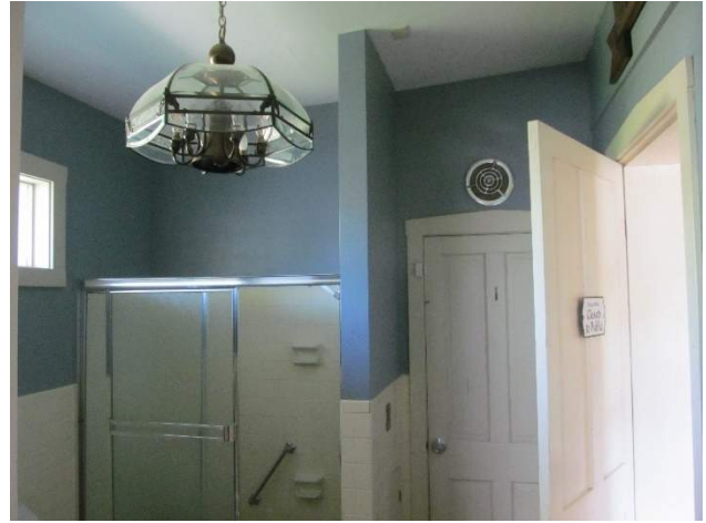
Figure 363. Incandescent pendant lighting fixture in bathroom on first floor. (Source: Alvine, 2022)
