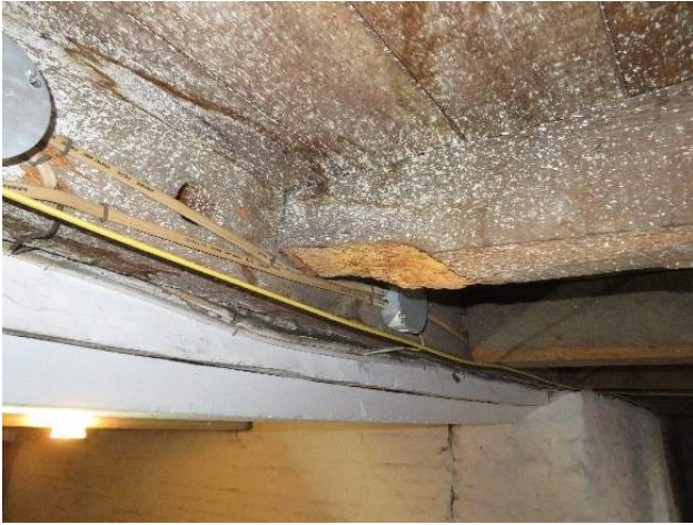
Figure 175. Bearing end of joists at shoring. (Source: RRJ, 2022).
