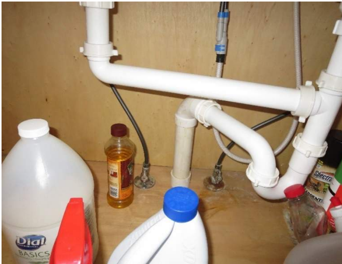
Figure 288. Existing sanitary waste piping below the kitchen sink is PVC. (Source: Alvine, 2022)
