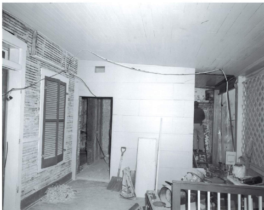
Figure 54. 1960s during renovations, Room 111 (west porch), looking south towards Room 112 (the bathroom), with the exterior plaster partially removed from the west wall at left. (Source: Schram Collection, Felix Vallé State Historic Site)
