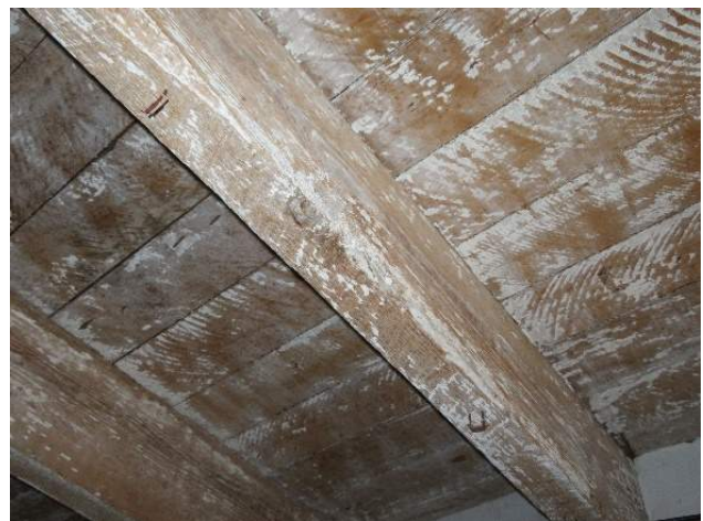
Figure 144. Circular sawn joist and decking. (Source: RRJ, 2022)
