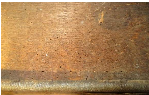
Figure 142. Evidence of powder post beetles. (Source: RRJ, 2022).
