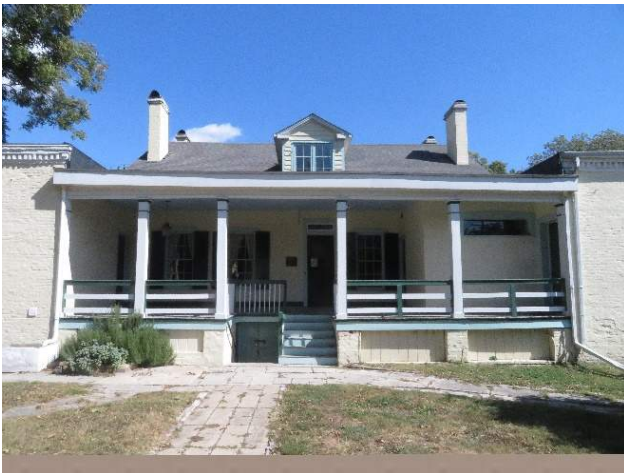
Figure 79. Gutter at eave at west gallery (Source: RRJ, 2022).
