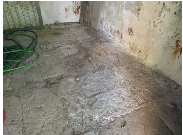
Figure 221. Stone flooring within Room 110. (Source: RRJ, 2022).
