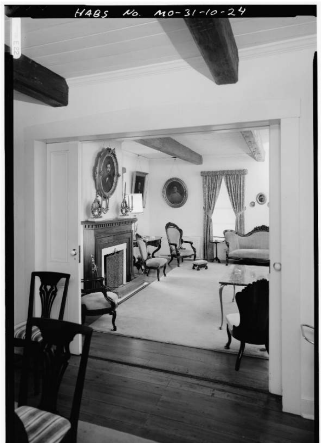
Figure 83. 1986, Room 106 (the dining room), looking east into Room 105 (the living room). Note that radiator heating system is still in place. (Source: Historic American Buildings Survey, Library of Congress, Call no. HABS MO,97-SAIGEN,1-). https://www.loc.gov/item/mo0360/ )
