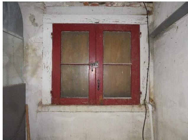
Figure 87. A basement casement window with exterior panel board behind (Source: RRJ, 2022).
