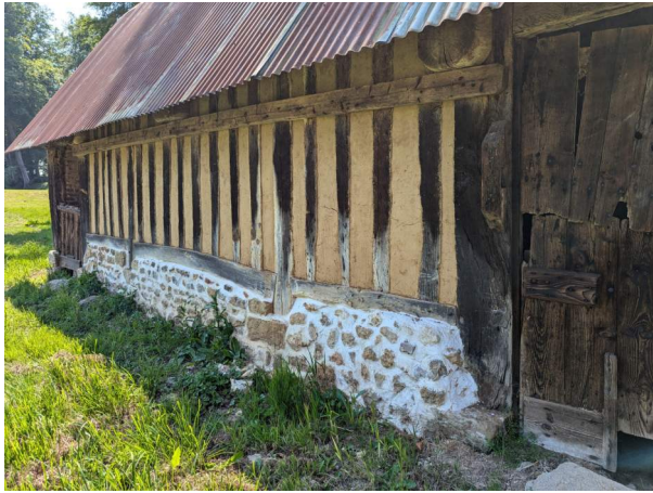
Figure 25. 18th or 19th century farm structure on the grounds of the Château de Bailleul in Picardy, France, with close-stud pan-de-bois construction. (Source: Lurita McIntosh Blank, 2024).
