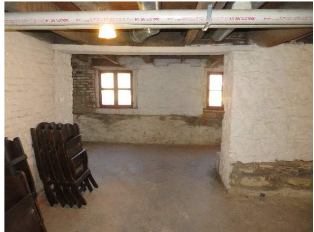
Figure 129. Slab-on-grade within Rooms 011B and 013 (Source: RRJ, 2022)
