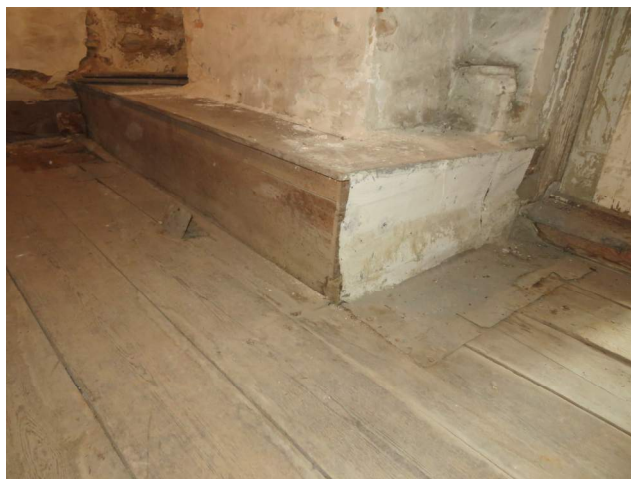
Figure 132. Floor planking observed in Room 009. (Source: RRJ, 2022).
