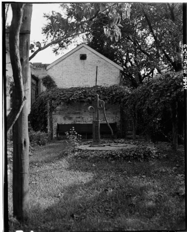
Figure 68. 1934 view of the well looking south toward the house, showing the stone lid and a metal pump set off center on top. (Source: HABS MO-31-10, Library of Congress Prints and Photographs Division, 1934)
