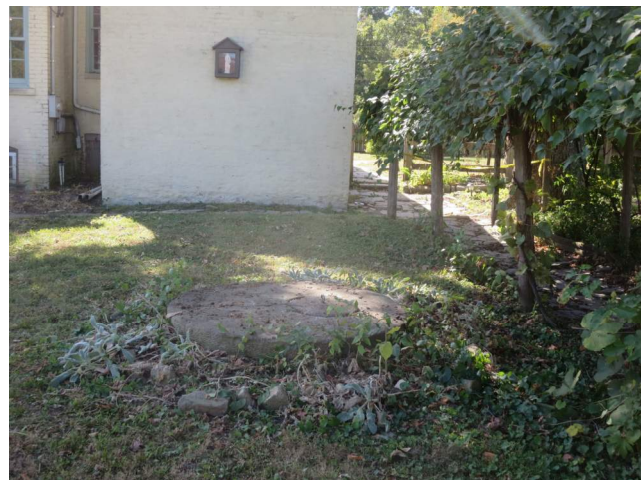
Figure 262. Photo of remaining well pump pad at rose garden. (Source: Alvine, 2022).
