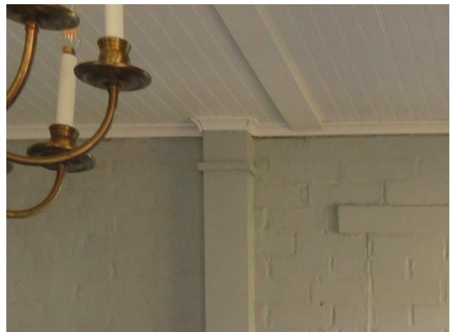
Figure 215. Room 108, looking north, showing detail of a portico column. The banding detail is the lower part of the column in the image below. (Source: RRJ, 2022)
