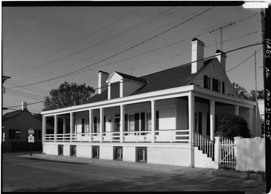
Figure 73. 1986, view of the house from the northeast on Main Street. (Source: Historic American Buildings Survey, Library of Congress, Call no. HABS MO,97-SAIGEN,1-). https://www.loc.gov/item/mo0360/ )
