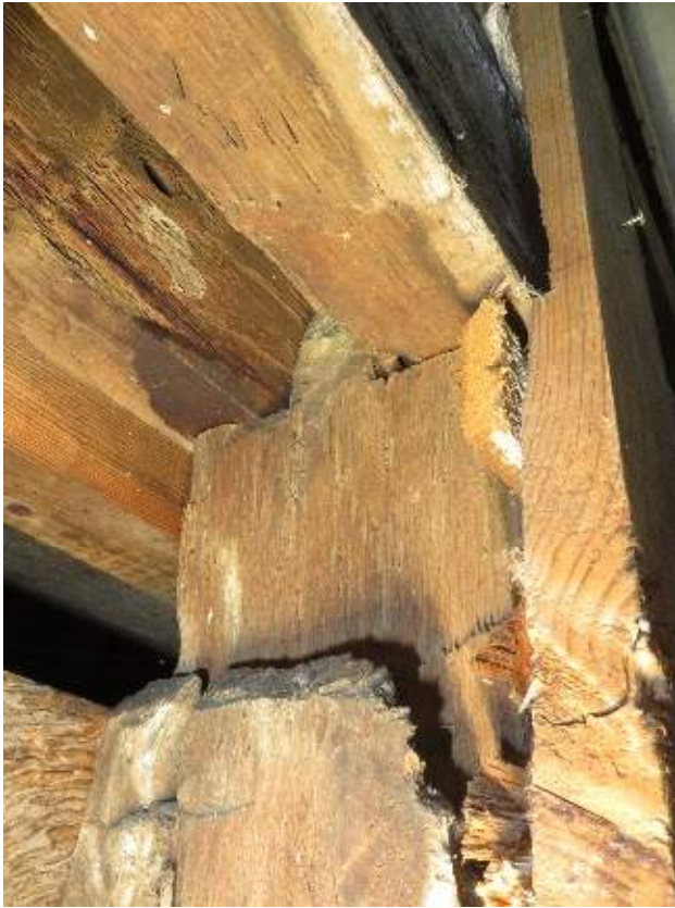
Figure 184. Portion of vertical log wall visible where finishes have been removed at the north wall within the northeast room at the second floor, showing the mortise connection of the vertical log to a continuous kerf at the top plate. (Source: RRJ, 2022)
