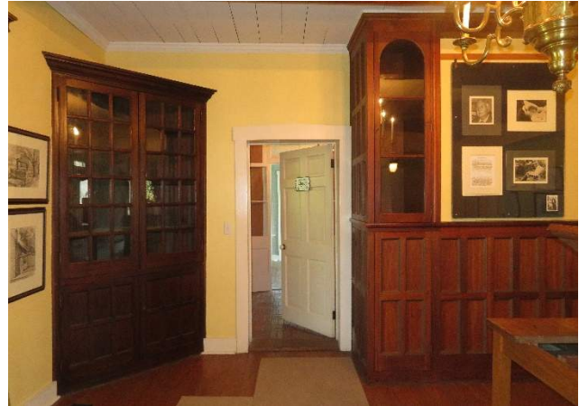
Figure 209. Room 106 facing north showing corner built-in (left) and portion of built-in concealing the former fireplace (right). (Source: RRJ, 2022).
