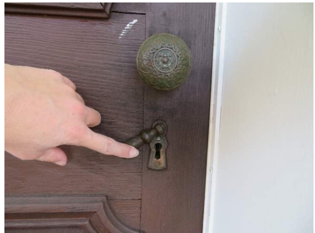
Figure 102. Exterior brass door knob with interlocking leaf and dart motif and key hole cover. (Source: RRJ, 2022)
