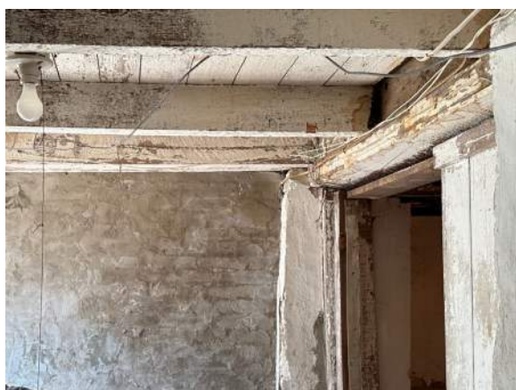
Figure 9. Sample 7. Room 10, beam, southern pine.
