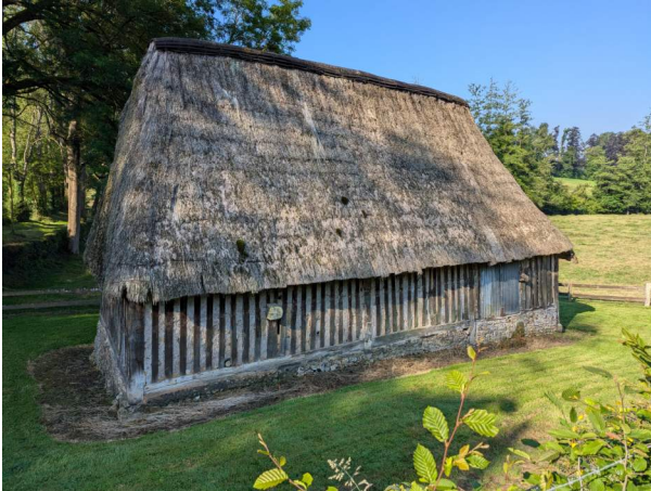
Figure 23. 17th century barn near Livet-sur-Authou, Normandy, France showing close-stud pan-de-bois construction technique that was the architectural antecedent to poteaux-sur-sole. (Source: Lurita McIntosh Blank, 2024)
