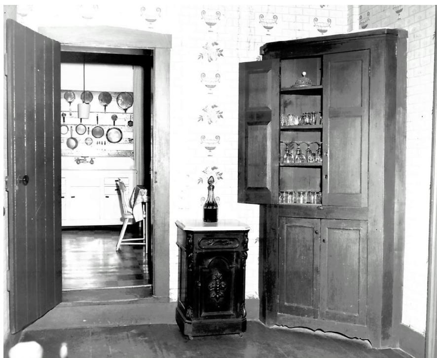
Figure 62. Undated (after the 1960s renovation), Room 107 (the pantry), looking west into the kitchen. This corner cabinet is believed to have been original to the house, although relocated in this photograph, and is now in private ownership in Ste. Genevieve. (Source: Schram Collection, Felix Vallé State Historic Site)
