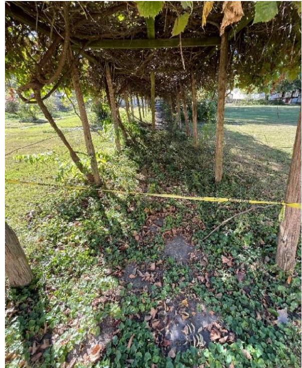
Figure 386. The pathway under the arbor (looking south) is paved with cut stones. It is overgrown with grass and groundcovers. The NPS has closed this path to visitors due to the condition of the arbor. (Source: LSHLA, 2022)
