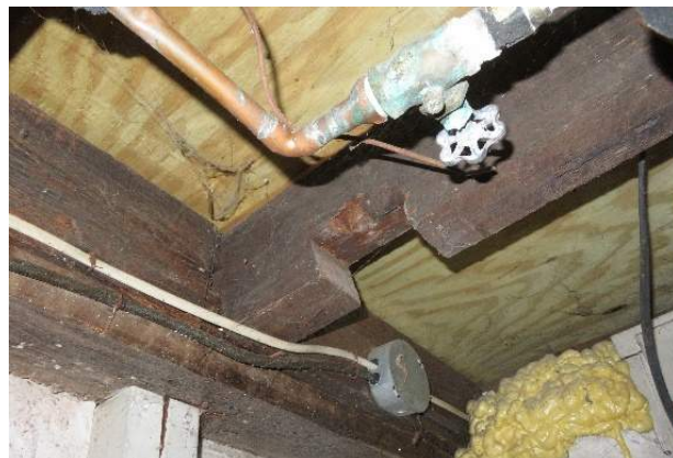
Figure 139. Plywood at room southwest. (Source: RRJ, 2022)
