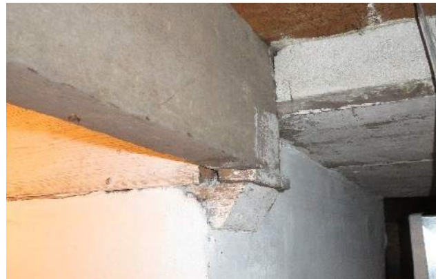
Figure 172. Timber haunch supporting joist. (Source: RRJ, 2022)
