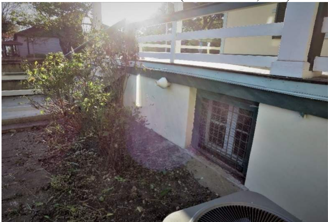
Figure 309. Existing combination flue exhaust and combustion air intake fitting at north exposure of house serving center basement furnace. (Source: Alvine, 2022)
