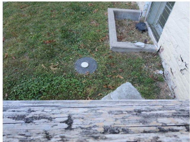
Figure 260. Existing water meter pit inside of property at south side. (Source: Alvine, 2022).
