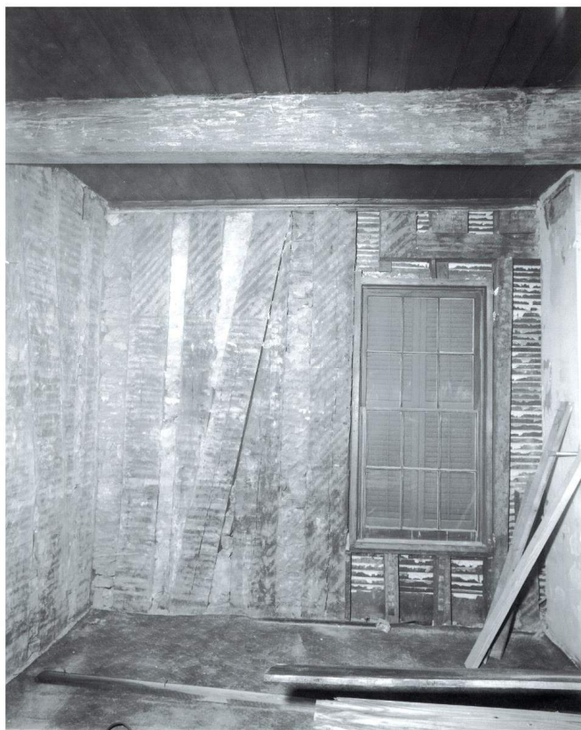
Figure 51. 1960s during renovations, southeast corner of Room 103, looking south. Note the wall framing alterations around the window and fireplace at right. (Source: Schram Collection, Felix Vallé State Historic Site)
