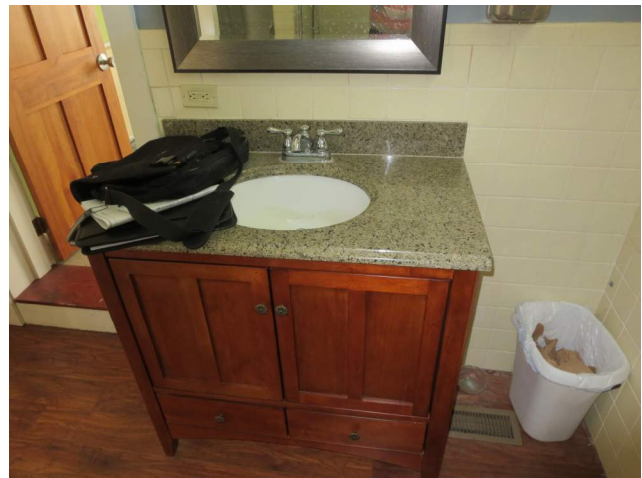
Figure 267. Existing under-mounted lavatory at First level restroom. (Source: Alvine, 2022).
