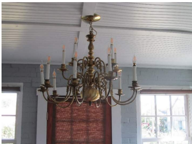
Figure 356. Incandescent pendant chandelier in living room on first floor. (Source: Alvine, 2022)
