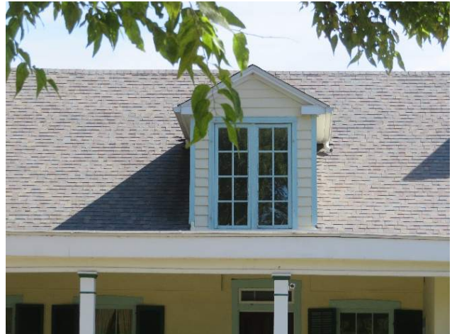
Figure 96. Exterior view of double casement window at second floor (Source: RRJ, 2022)
