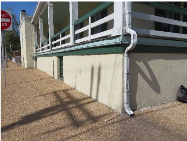
Figure 80. Downspouts at East Gallery, discharge at sidewalk. (Source: RRJ, 2022).
