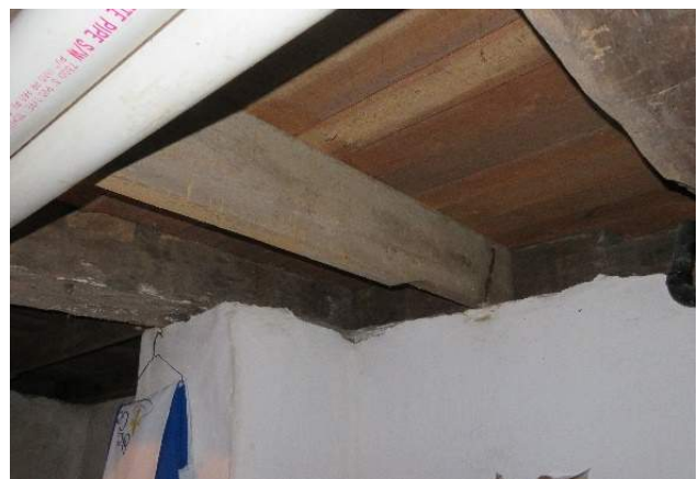
Figure 168. Joist end bearing on the limestone foundation. (Source: RRJ, 2022)
