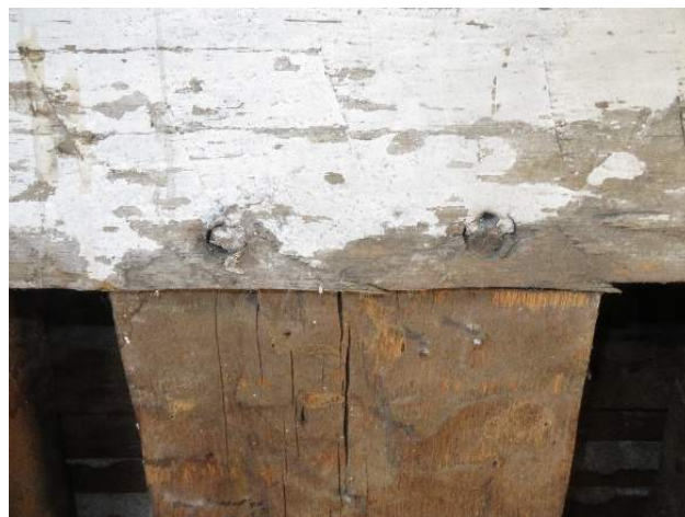
Figure 183. Two tenons observed at top of vertical log. (Source: RRJ, 2022)
