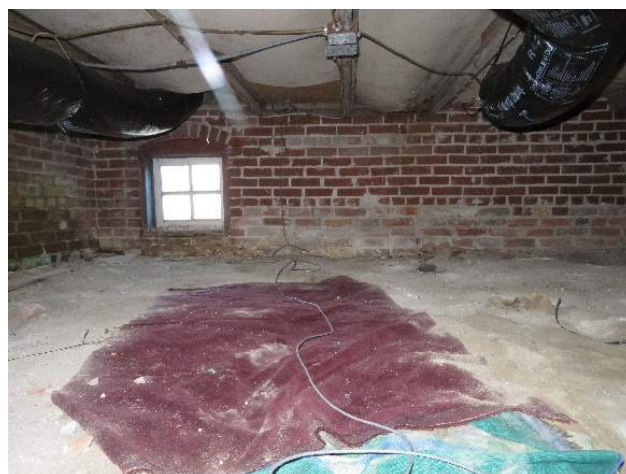
Figure 153. Overview looking north. (Source: RRJ, 2022)
