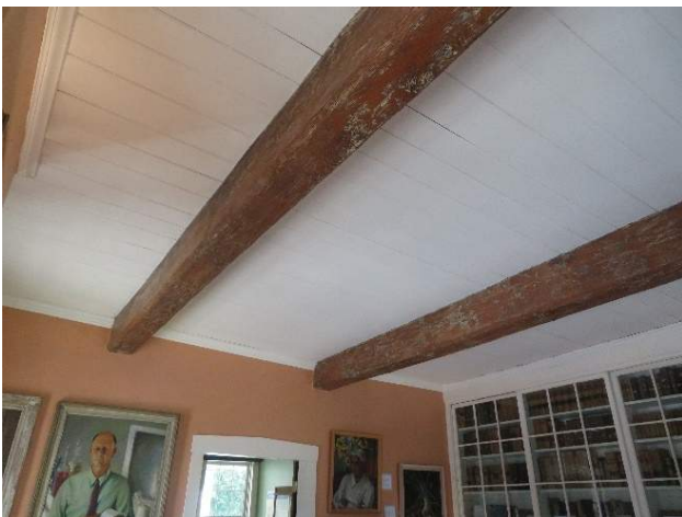
Figure 202. Exposed ceiling beams in Room 103. (Source: RRJ, 2022)
