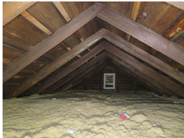
Figure 121. Overview of roof rafter framing and gable end wall. (Source: RRJ, 2022).
