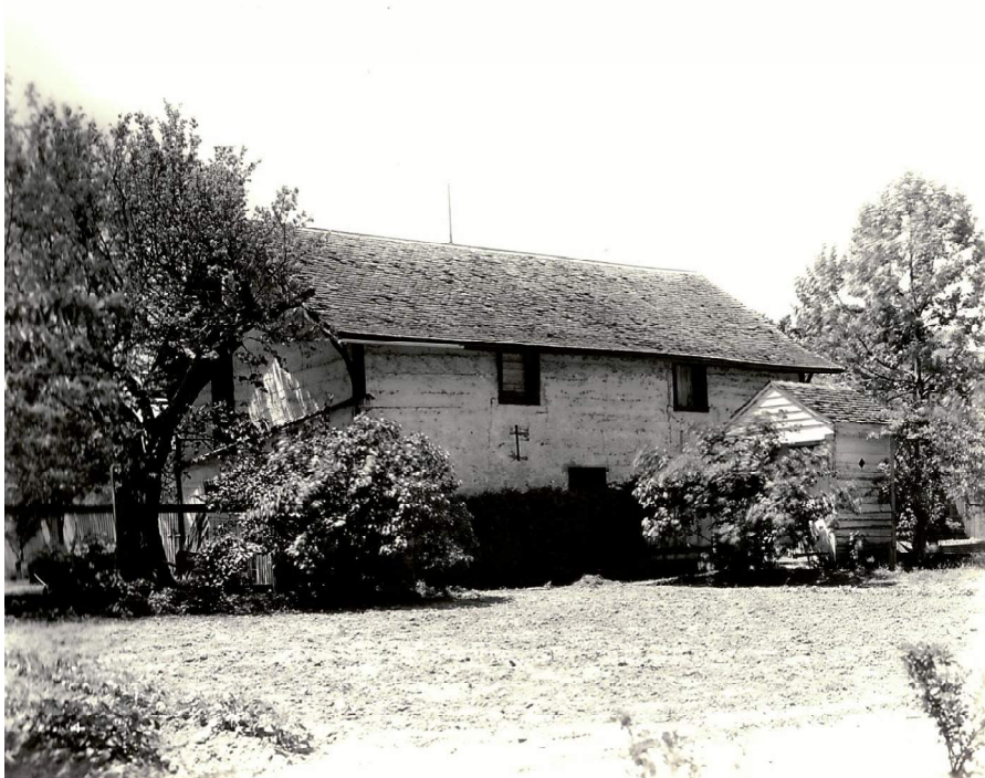
Figure 40. Undated, looking south to the garage (demolished in 1982). (Source: Schram Collection, Felix Vallé State Historic Site)
