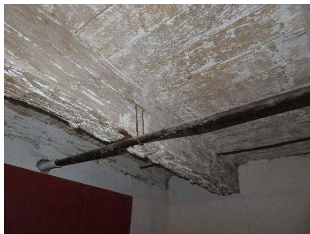
Figure 150. Checking at south-most joist. (Source: RRJ, 2022).
