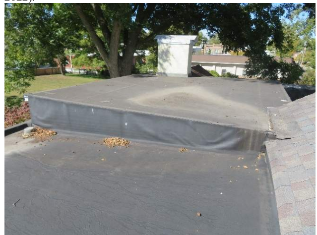
Figure 77. EPDM Roofing above room 109 and West Gallery (Source: RRJ, 2022).
