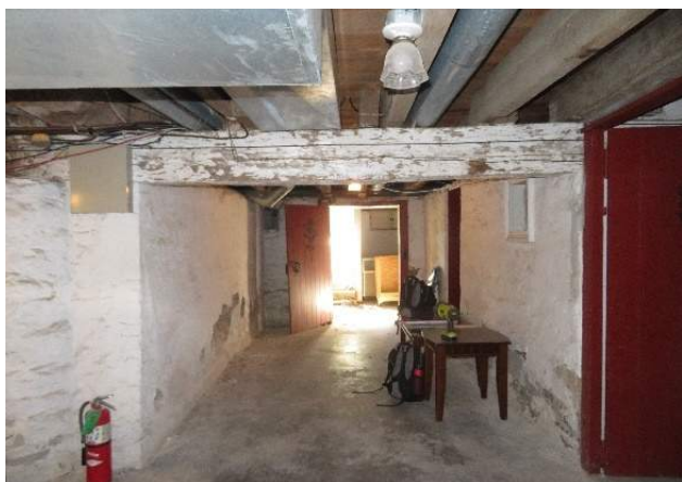
Figure 161. Overview looking west into Room 5. (Source: RRJ, 2022).
