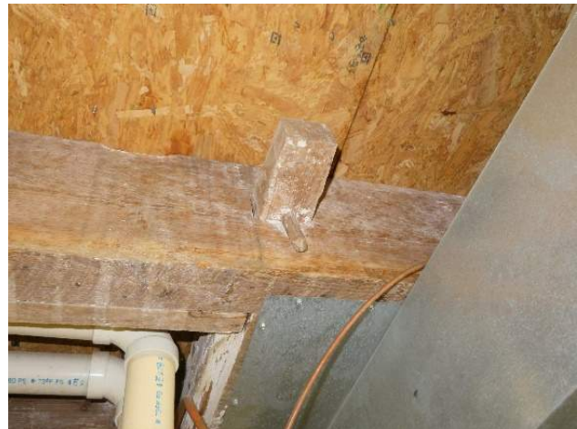
Figure 135. Pinned tenon joint. (Source: RRJ, 2022).
