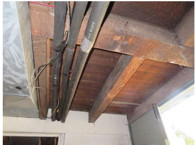
Figure 133. Beam near descending staircase. (Source: RRJ, 2022)
