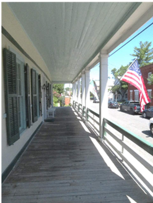
Figure 114. East gallery facing north (Source: : RRJ, 2022)
