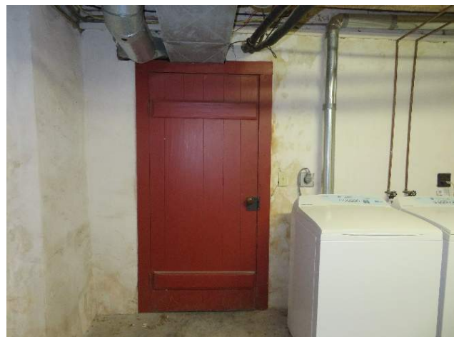
Figure 244. Door D002 viewed from within Room 002. (Source: RRJ, 2022)
