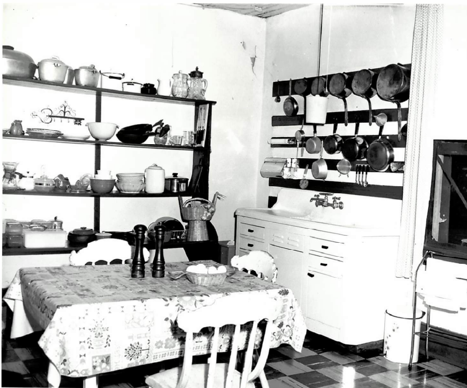
Figure 60. Undated (after the 1960s renovation), Room 109 (the kitchen), looking west. (Source: Schram Collection, Felix Vallé State Historic Site)
