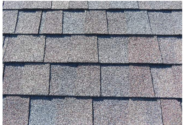
Figure 76. Laminated asphalt shingle roofing. (Source: RRJ, 2022).
