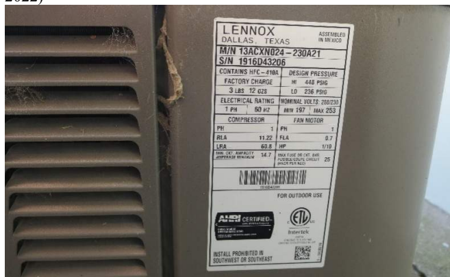
Figure 316. Existing 3-ton condensing unit serving central basement level furnace. (Source: Alvine, 2022)
