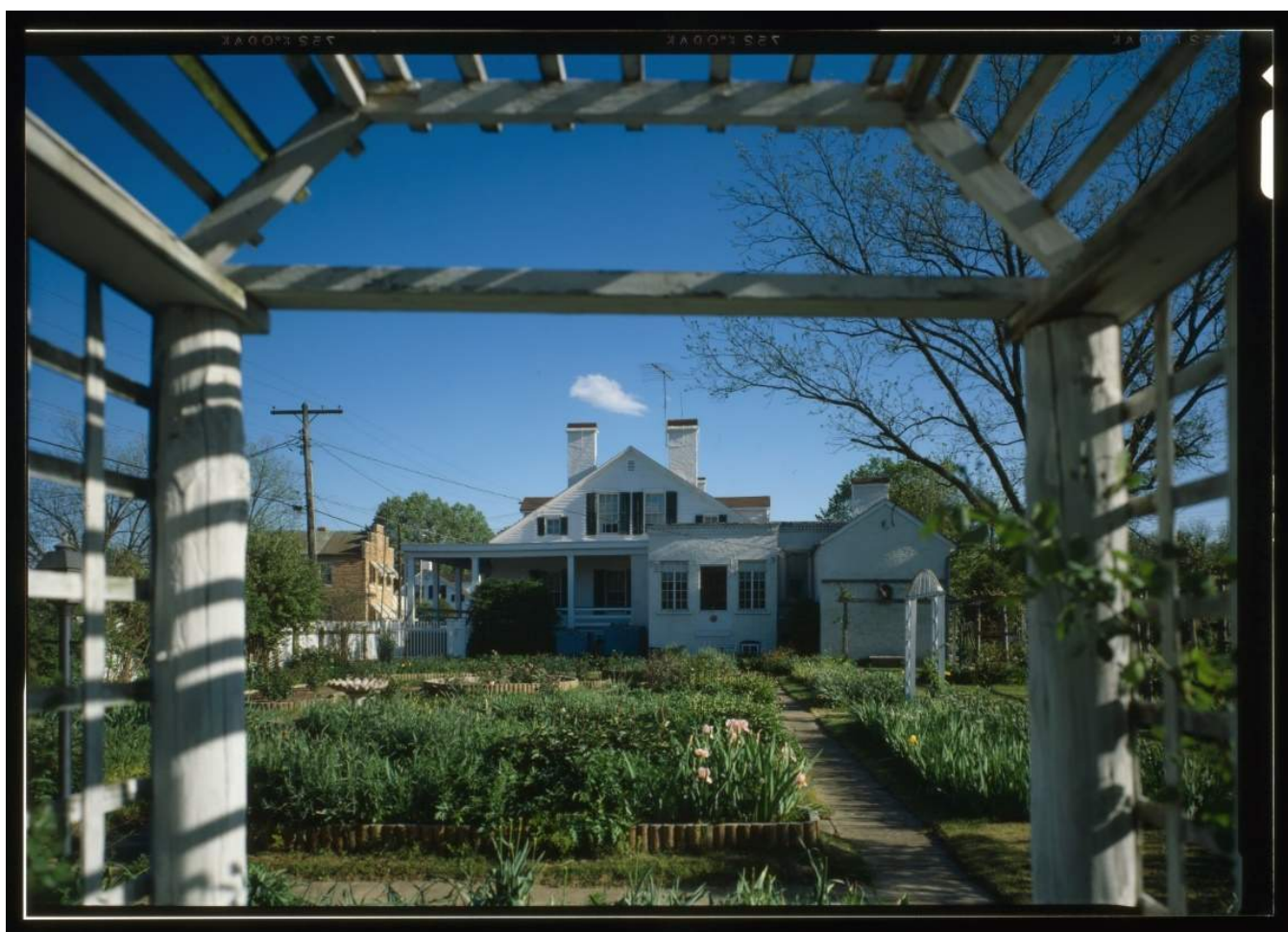
Figure 81. 1986, looking south across the parterre garden to the north exterior wall. Note that the door to the sunroom has not yet been reinstalled. (Source: Historic American Buildings Survey, Library of Congress, Call no. HABS MO,97-SAIGEN,1-) https://www.loc.gov/item/mo0360/ )
