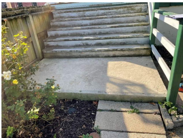
Figure 382. View of the 30-inch-wide pathway, raised concrete landing, and steps leading to the east entrance to the house. (Source: LSHLA, 2022)
