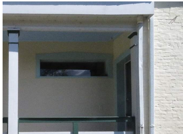
Figure 95. Exterior view of Window W112 (Source: RRJ, 2022).
