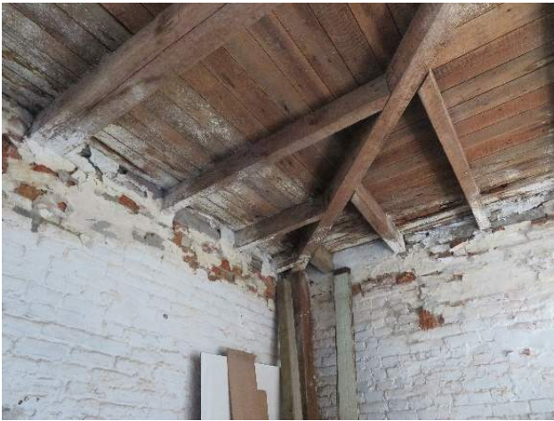
Figure 176. Overview of northeast gallery corner. (Source: RRJ, 2022)
