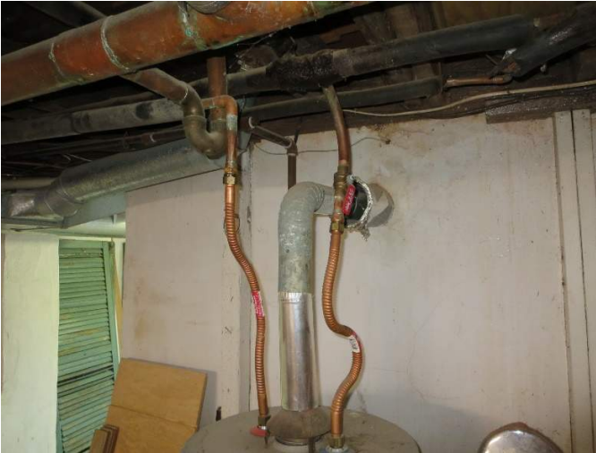
Figure 284. The water heater flue passes through the adjacent wall to the south. (Source: Alvine, 2022)
