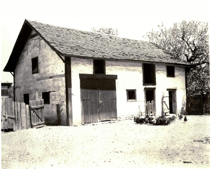
Figure 39. Undated, likely looking northeast to the garage (demolished in 1982). Note the ghosting and remnants of roll roofing on the left gable end, indicating that another structure may have previously been attached to this side of the structure. (Source: Schram Collection, Felix Vallé State Historic Site)
