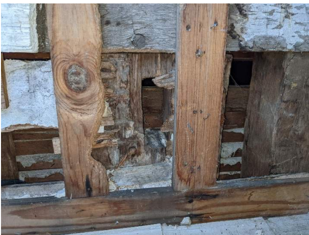
Figure 185. Notch in vertical log for c. 1792 (now missing) gallery framing. (Source: RRJ, 2022)
