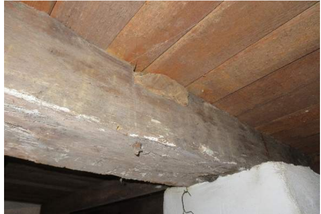
Figure 170. of previous half-dovetail lap joint belonging to a diagonal sill plate brace within the northmost timber joist. (Source: RRJ, 2022).
