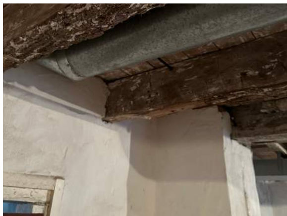
Figure 3. Sample 1. Room 6, beam, white oak.
