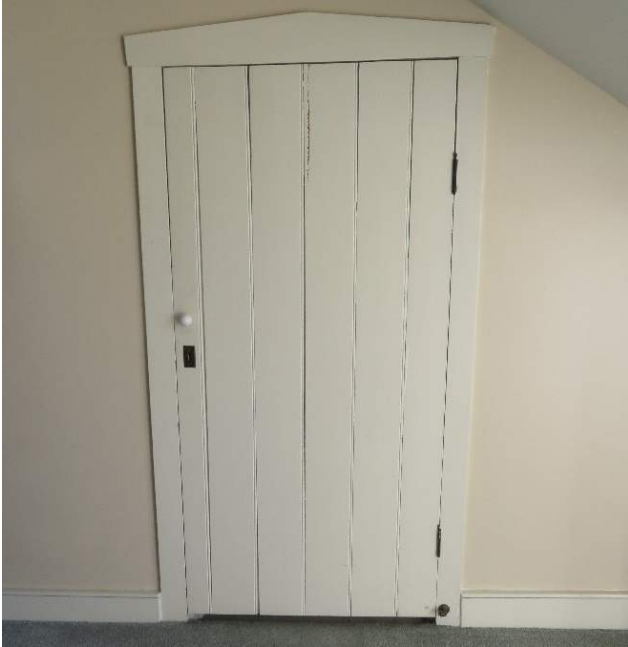
Figure 257. Door D201 seen from Room 201. (Source: RRJ, 2022)
