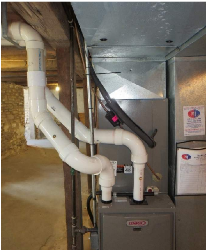
Figure 291. The gas piping serving each of the Basement furnaces is Schedule 40 black steel. (Source: Alvine, 2022)
