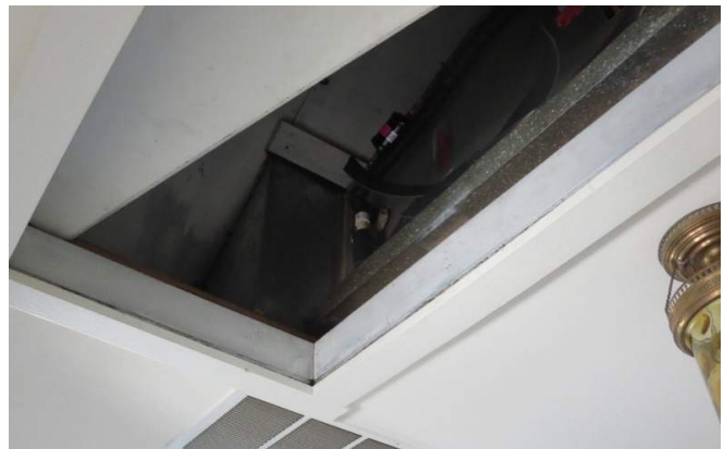
Figure 311. View up through the access opening in the ceiling to the Second level electric furnace. (Source: Alvine, 2022)
