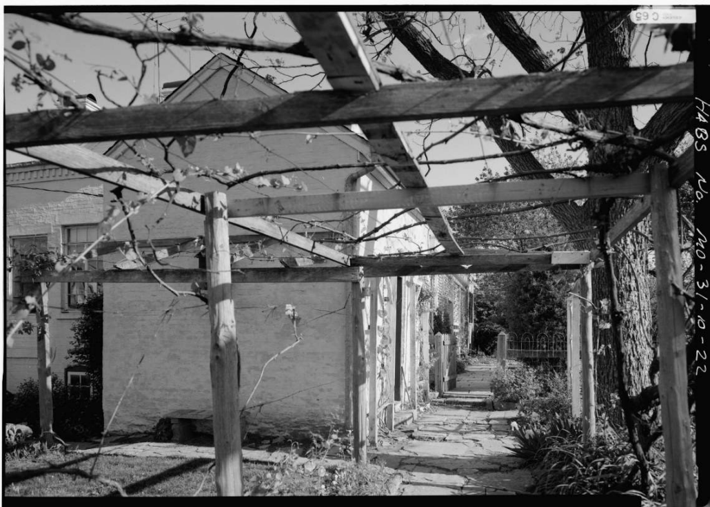
Figure 77. 1986, looking south from the grape arbor along the west exterior wall of the house. (Source: Historic American Buildings Survey, Library of Congress, Call no. HABS MO,97-SAIGEN,1-). https://www.loc.gov/item/mo0360/ )
