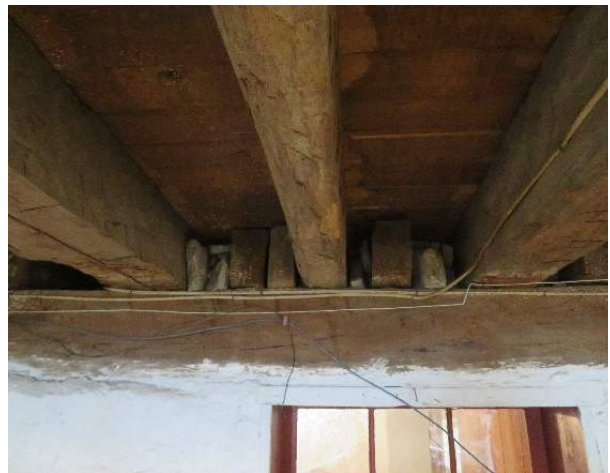
Figure 167. Joist ends and infill looking west. (Source: RRJ, 2022).
