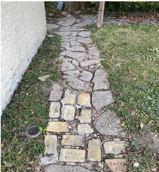
Figure 388. Irregular cut stone pavers with large open spaces between the stones are used on the pathway leading around the garage, west of the house. (Source: LSHLA, 2022).
