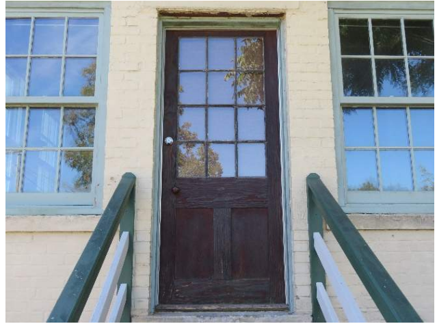
Figure 105. Exterior of Door D108. (Source: RRJ, 2022)
