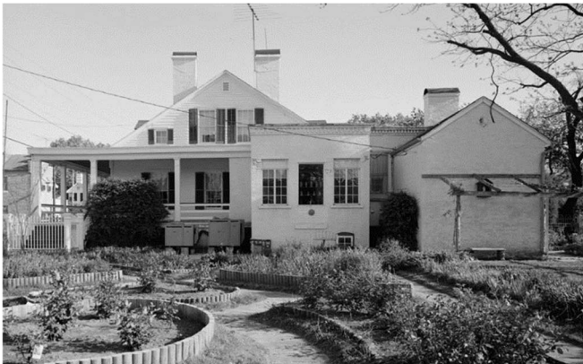
Figure 298. Vintage HVAC units which resided at the north side of the house have since been removed. (Source: HABS, 1933)
