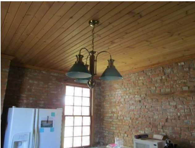
Figure 354.. Incandescent pendant lighting fixture in kitchen on first floor. (Source: Alvine, 2022)
