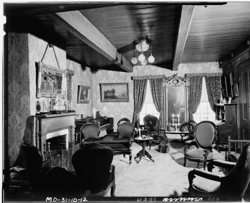
Figure 19. 1949, Room 105 looking east towards Main Street. Note the fireplace mantel at left is not the same mantel as is presently in place at the house. (Source: Historic American Buildings Survey, Library of Congress, Call no. HABS MO,97-SAIGEN,1-). https://www.loc.gov/item/mo0360/ )
