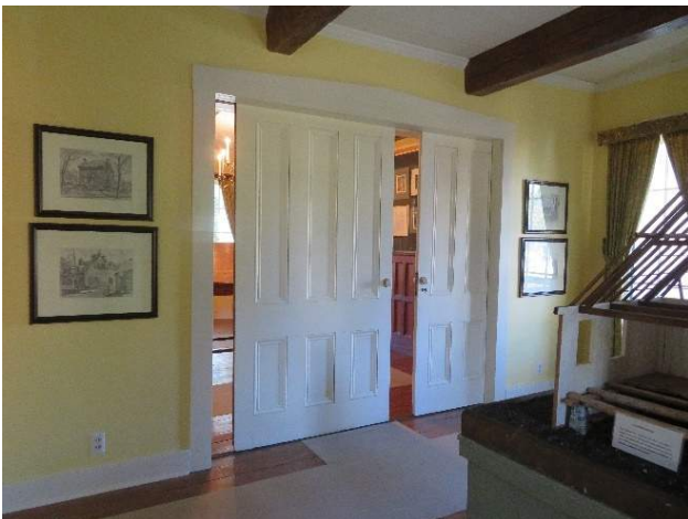
Figure 253. Semi-closed double pocket doors (D105B) seen from Room 105. (Source: RRJ, 2022)
