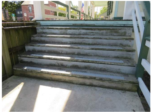
Figure 115. Stairs to east gallery at north wall (Source: RRJ, 2022)
