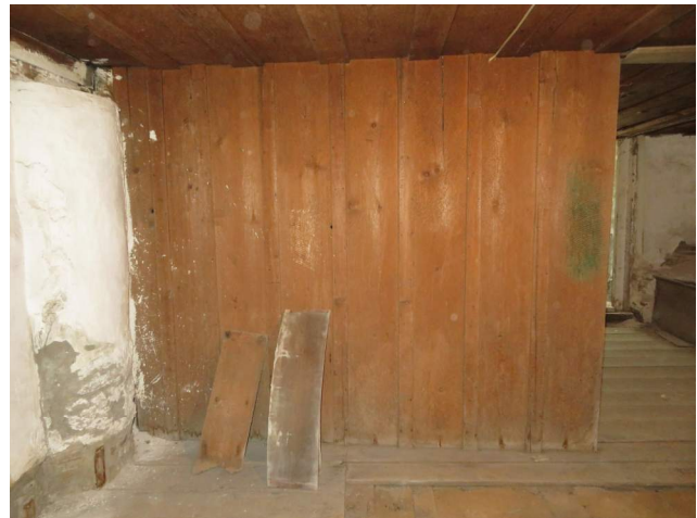
Figure 128. c. 1862 sawn lumber partition wall in room 009. (Source: RRJ, 2022).
