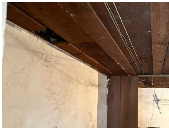
Figure 8. Sample 6. Room 9, beam, white oak.
