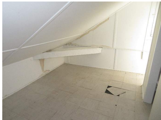
Figure 189. Top Plate Brace at Southeast (Room 203). (Source: RRJ, 2022).
