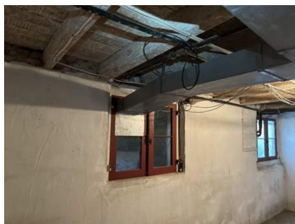
Figure 6. Sample 4. Room 7, beam, southern pine.
