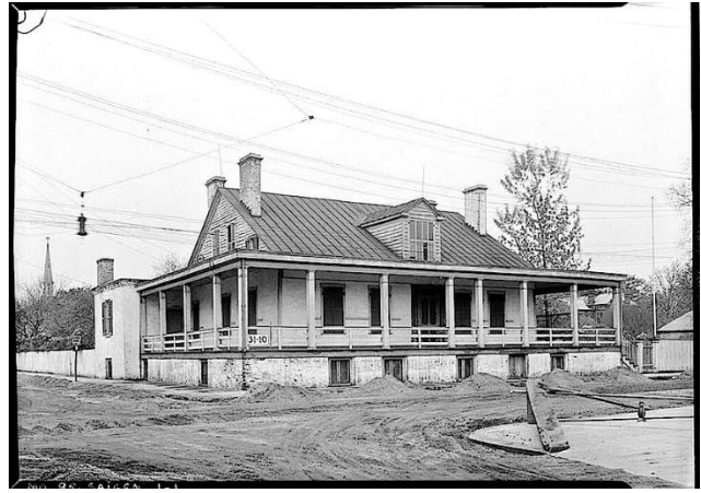
Figure 30. 1934 view northwest toward the east façade of the house from South Main Street, over newly constructed sidewalks. (Source: Alexander Piaget photograph, HABS MO-31-10, Library of Congress Prints and Photographs Division).
