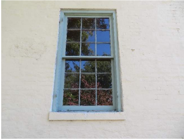
Figure 92. Exterior view of typical nine-over-nine double hung window (Source: RRJ, 2022)
