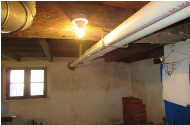
Figure 307. Existing flue and combustion air piping up high in basement level from central furnace. (Source: Alvine, 2022)
