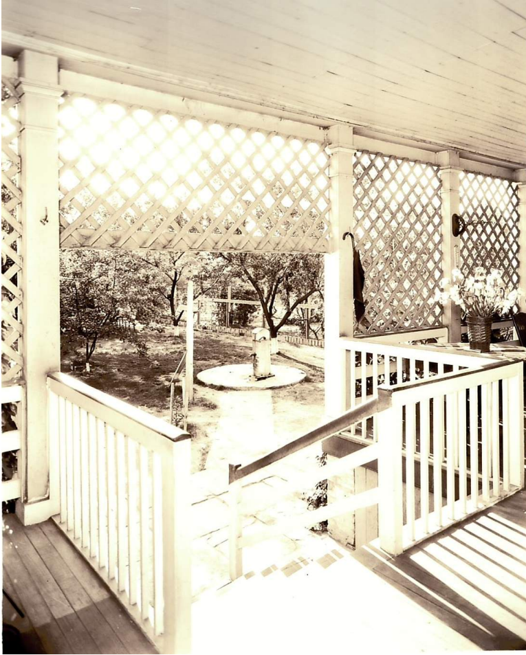
Figure 37. Undated, view from west porch, looking northwest towards the cistern and pump. Based on the diameter of the tree trunks and grapevines in the background, this photograph appears to be similar in date to the 1934 HABS photograph of the same view. (Source: Schram Collection, Felix Vallé State Historic Site)
