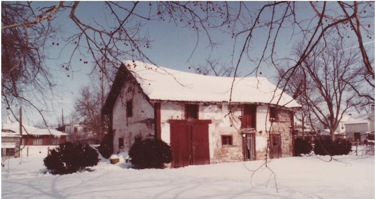
Figure 70. c. 1982, looking slightly northeast to the barn from Market Street, note the distress to the bar roof framing. (Source: Robert Mueller, private collection)
