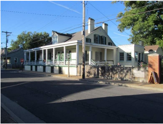
Figure 336. Citizen Electric Corporation overhead 240/120-volt, secondary electrical drop to building. (Source: Alvine, 2022)
