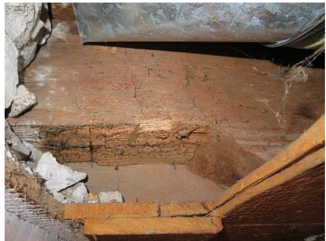
Figure 155. Side face of hewn joist at end. (Source: RRJ, 2022).
