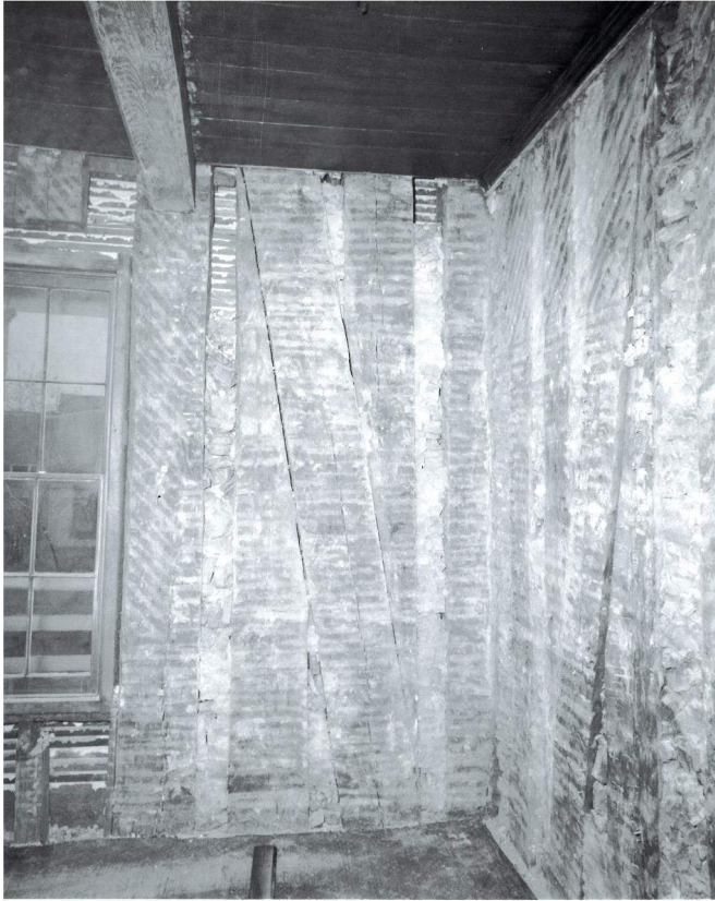
Figure 49. 1960s, photograph of the southeast corner of Room 103 taken during renovations, showing the exterior log walls from the interior. Note the alterations to the framing around the windows, indicating that the rough openings had been modified. Ghosting from plaster lath is visible; the diagonal lath marks may be from the original plaster. (Source: Schram Collection, Felix Vallé State Historic Site)
