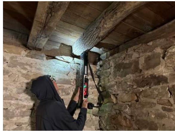
Figure 2. Use of a resistance drill to investigate the internal wood condition in a floor beam.
