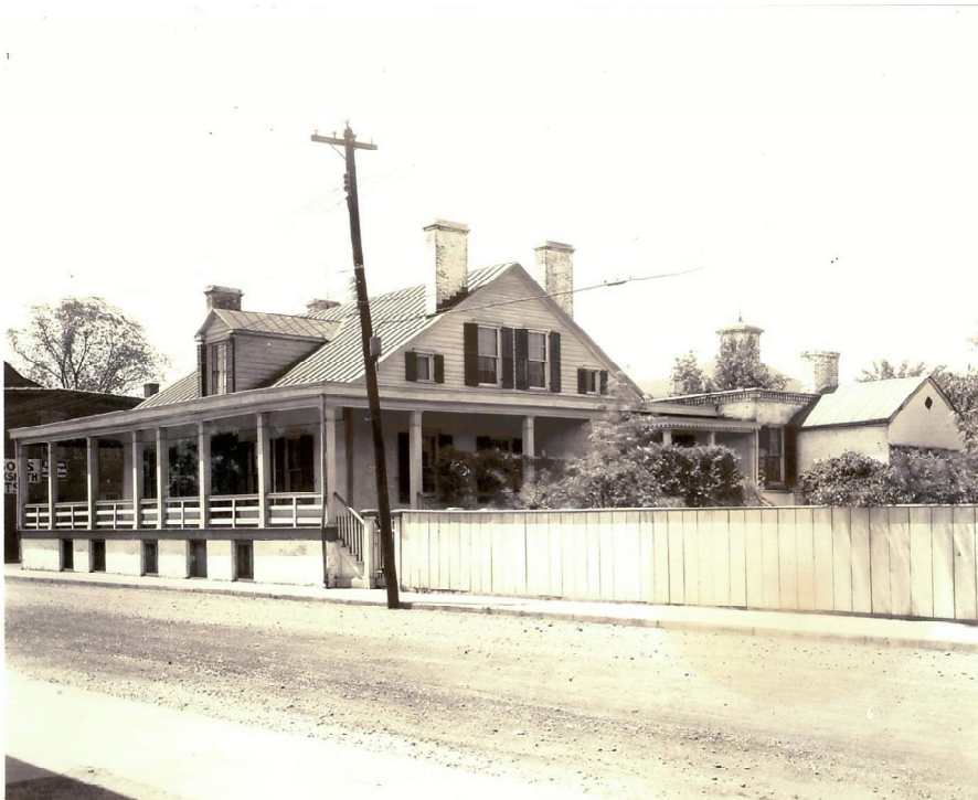
Figure 43. Undated (possibly 1930s), looking southwest from the corner of the Lagrave Building (58 South Main Street). (Source: Schram Collection, Felix Vallé State Historic Site)
