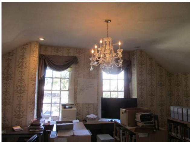
Figure 360. Incandescent chandelier and incandescent down lights in office on second floor. (Source: Alvine, 2022)
