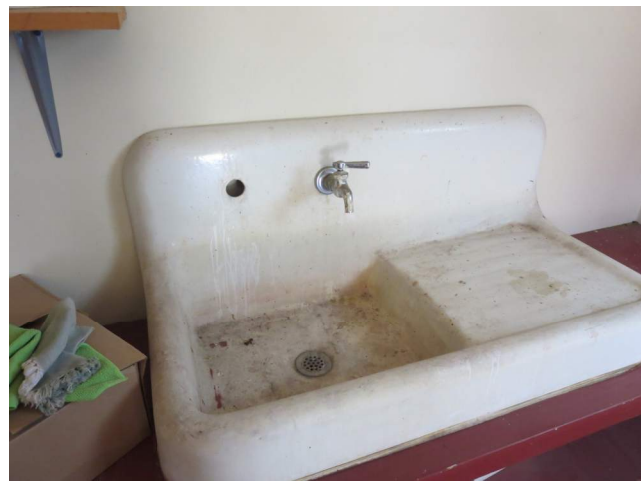
Figure 272. Existing old sink in the shop of the existing garage located west of the Vallé House. (Source: Alvine, 2022)
