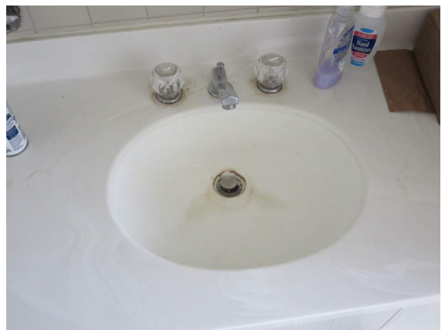
Figure 268. Existing molded, integral counter lavatory and faucet with crystalline handles at Second level restroom. (Source: Alvine, 2022).
