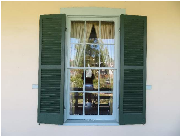
Figure 90. Six-over-six double hung wood windows typical of first floor windows located in original core of the house (Source: RRJ, 2022)
