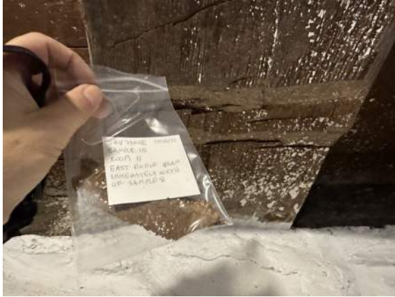
Figure 13. Sample 10. Room 11, beam, white oak.
