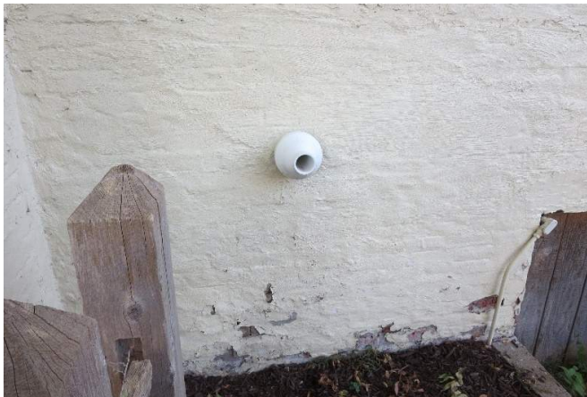
Figure 308.. Existing combination flue exhaust and combustion air intake fitting at west exposure of house serving NW basement furnace. (Source: Alvine, 2022)
