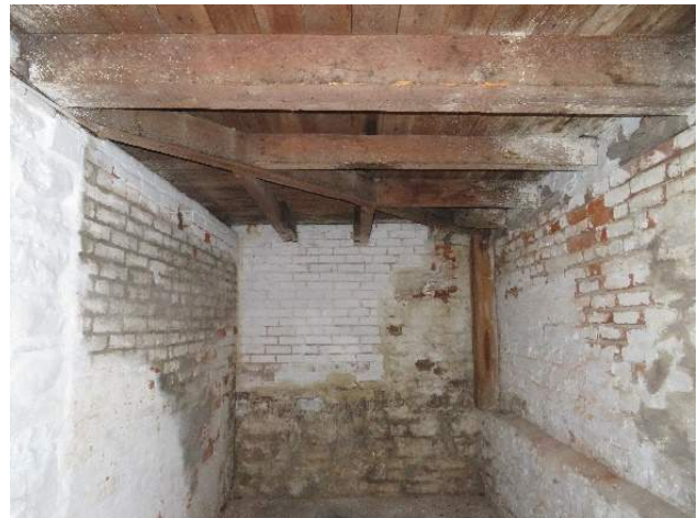
Figure 173. Overview of northeast gallery corner. (Source: RRJ, 2022)
