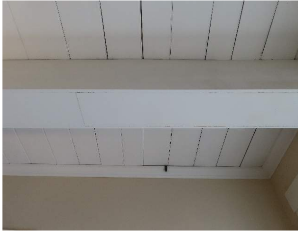
Figure 195. Painted ceiling boards in Room 101. (Source: RRJ, 2022)
