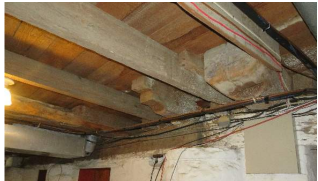
Figure 159. Overview looking south-southwest. (Source: RRJ, 2022).
