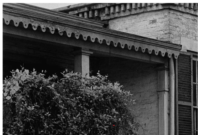
Figure 216. 1934 HABS photograph. The column at right is visible in the image above. (Source: HABS).
