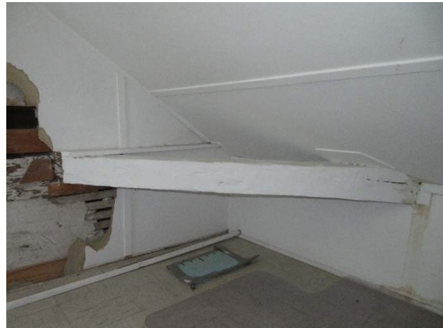
Figure 188. Top Plate Brace at Northeast (Room 208). (Source: RRJ, 2022)
