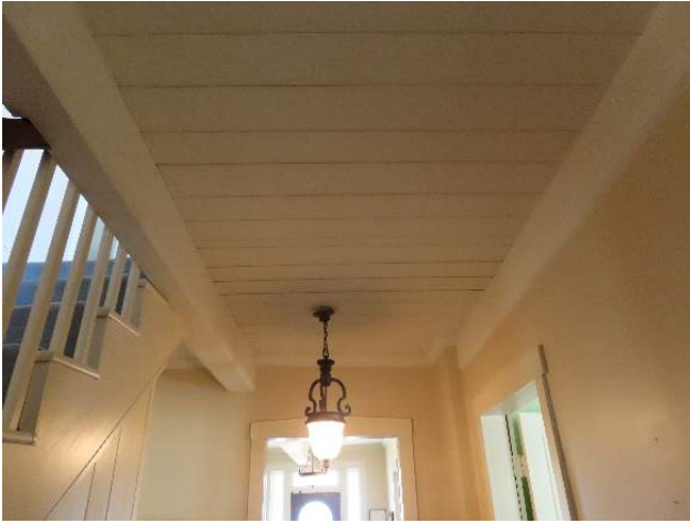
Figure 179. Covered joist viewed from Room 102, looking east. (Source: RRJ, 2022)
