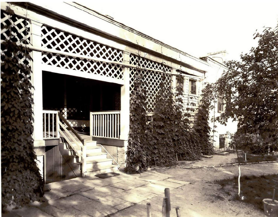
Figure 38. Undated (likely after 1934), view from yard towards the west porch, looking southeast. (Source: Schram Collection, Felix Vallé State Historic Site)
