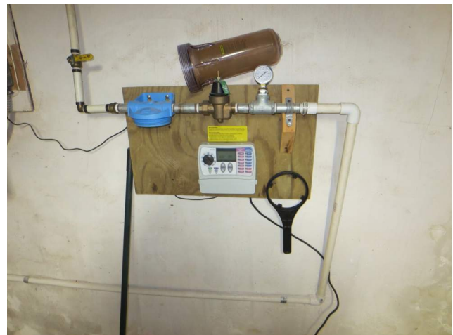
Figure 281. Existing PVC water piping serving lawn irrigation system. (Source: Alvine, 2022).
