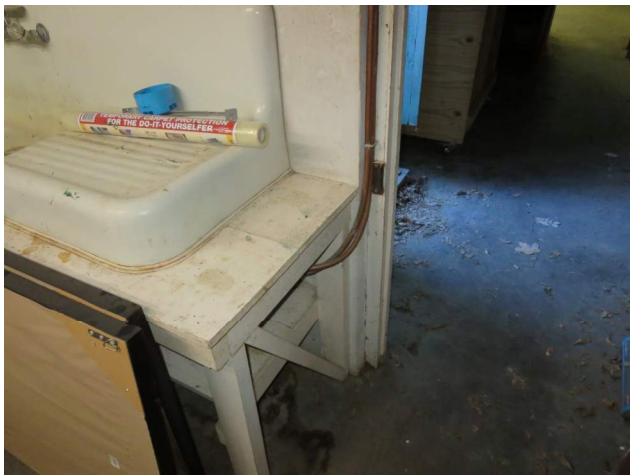
Figure 274. Existing hot and cold water supply piping routing down wall to below the sink wood counter. (Source: Alvine, 2022).
