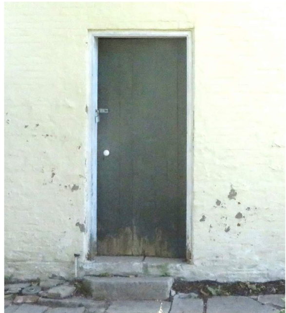
Figure 110. Exterior of Door D110 to tool shed. (Source: RRJ, 2022)
