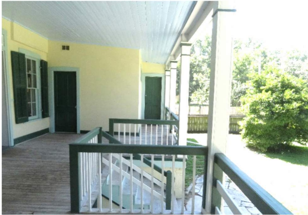
Figure 108. West porch showing Doors D112 (left) and D113A (right). (Source: RRJ, 2022)
