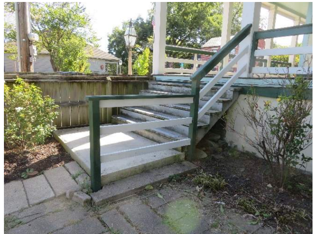
Figure 116. Railing at north stairs to east gallery (Source: : RRJ, 2022)
