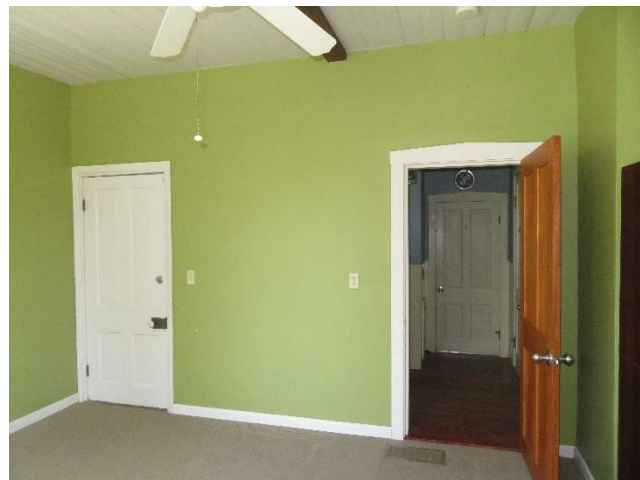
Figure 224. Room 113, looking north towards room 112. (Source: RRJ, 2022)
