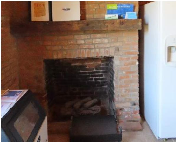
Figure 218. Masonry fireplace in northwest corner of Room 109. The mantel appears to be salvaged historic material but was likely installed in 2010s (Source: RRJ, 2022).
