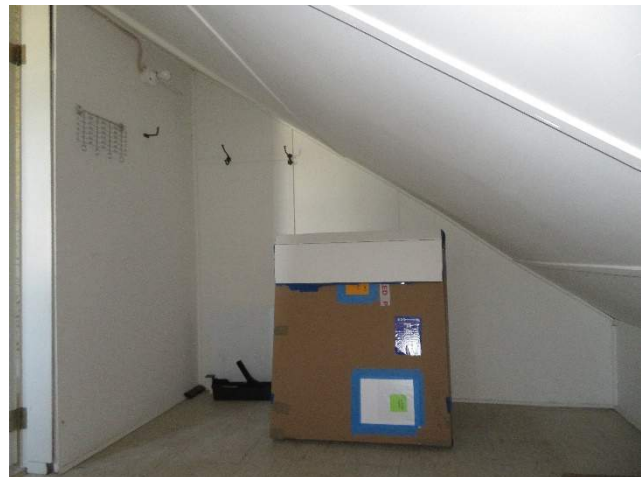
Figure 239. Debonded linoleum flooring in Room 206. (Source: RRJ, 2022)
