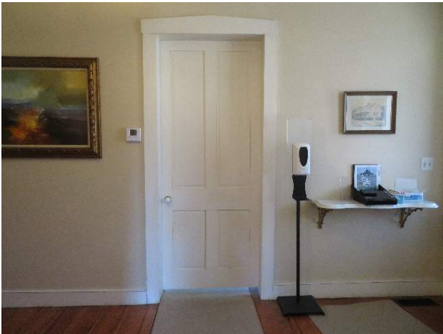
Figure 252. Door D105A seen from Room 101. (Source: RRJ, 2022)
