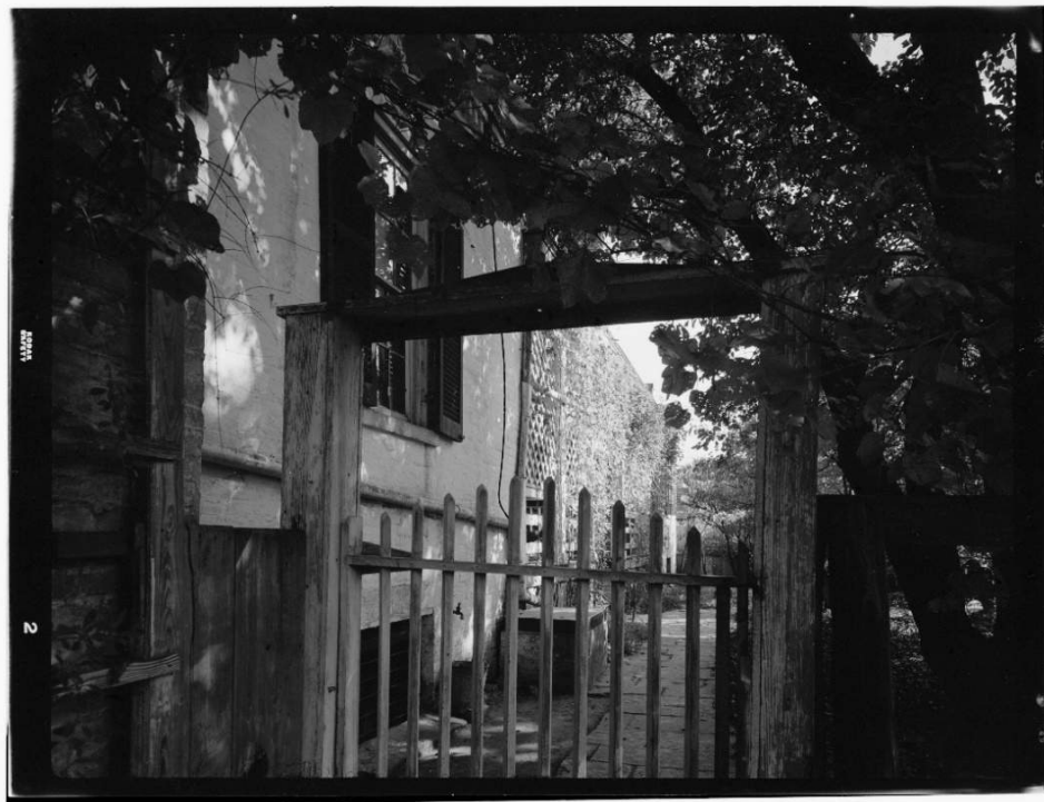
Figure 20. Undated (after 1934, possibly 1949), looking south towards Market Street along the west exterior wall. Note the vegetation growth on the west porch lattice. (Source: Historic American Buildings Survey, Library of Congress, Call no. HABS MO,97-SAIGEN,1-). https://www.loc.gov/item/mo0360/ )
