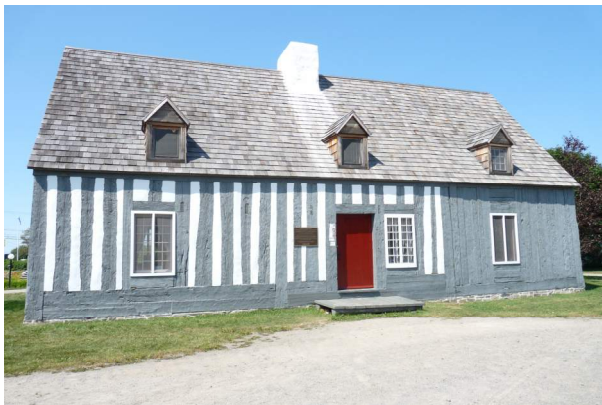
Figure 26. 18th or 19th century farm structure on the grounds of the Château de Bailleul in Picardy, France, with close-stud pan-de-bois construction. (Source: Lurita McIntosh Blank, 2024).
