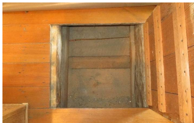
Figure 205. Concealed storage space below floor planks in Room 104. (Source: RRJ, 2022).
