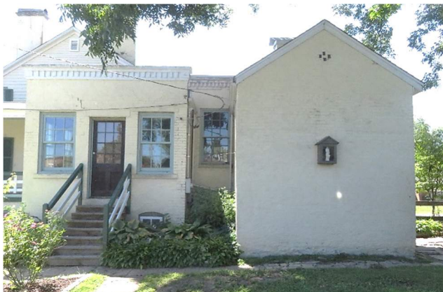
Figure 81. Masonry walls at tool shed and sunroom (Source: RRJ, 2022)
