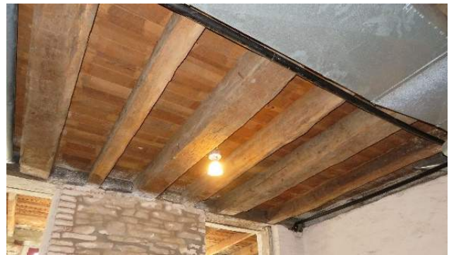
Figure 158. Overview looking east-southeast. (Source: RRJ, 2022)
