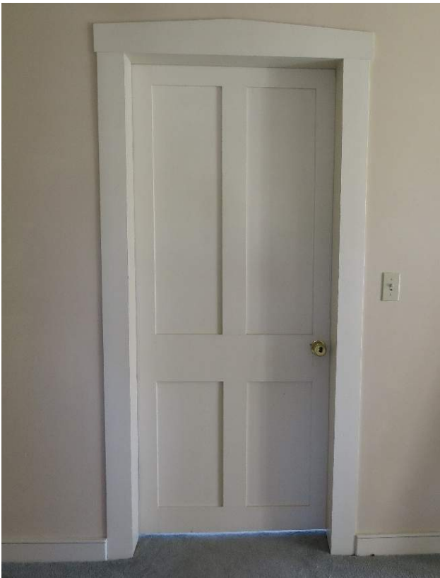
Figure 258. Door D204A seen from Room 201. (Source: RRJ, 2022)
