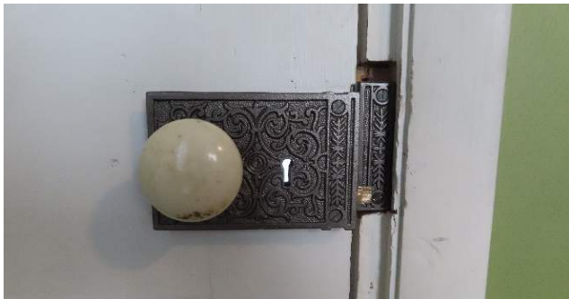
Figure 109. Interior door knob and rim lock form Door D113A. (Source: RRJ, 2022)
