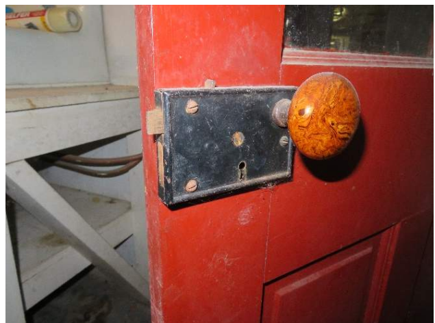
Figure 247. Door Hardware at Door D003. (Source: RRJ, 2022)
