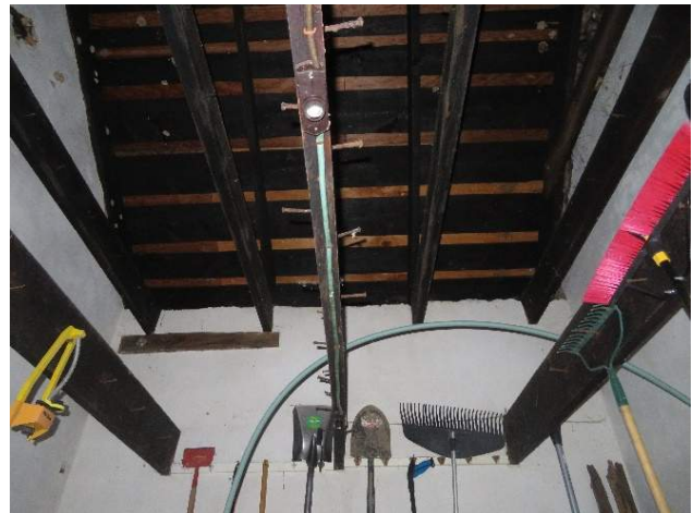
Figure 220. Exposed roof structure within Room 110. (Source: RRJ, 2022)
