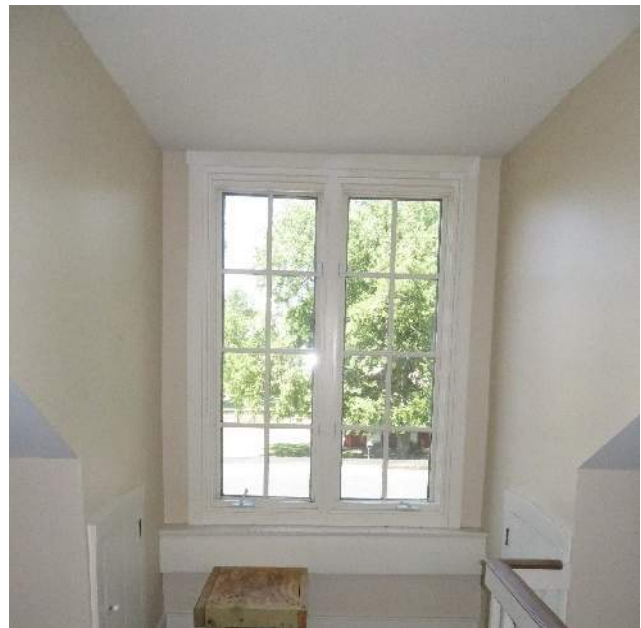
Figure 97. Interior view of double casement window at second floor (Source: RRJ, 2022).
