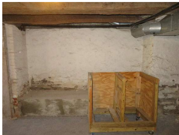
Figure 123. Supplemental concrete foundation within Room 011A (Source: RRJ, 2022)
