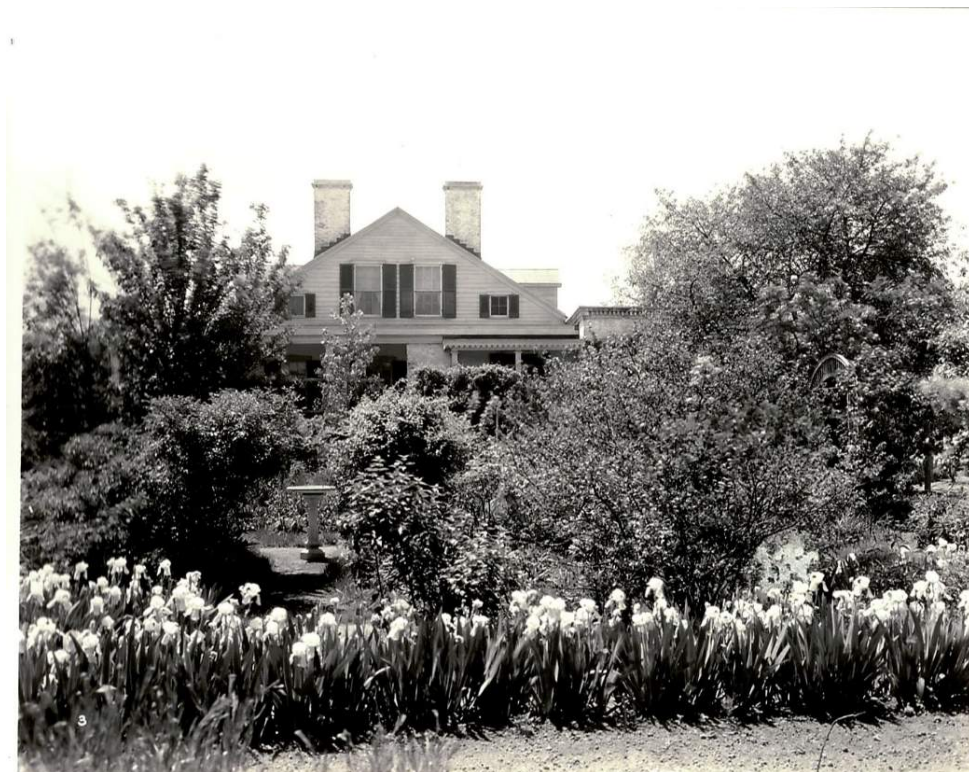
Figure 42. Undated (possibly 1930s), view of north exterior wall from the parterre garden. (Source: Schram Collection, Felix Vallé State Historic Site)
