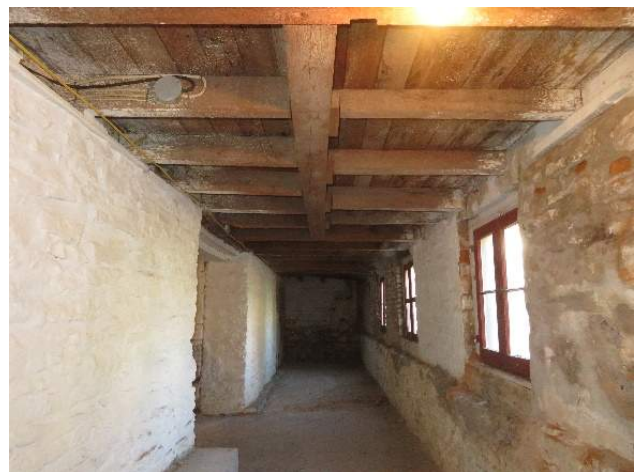
Figure 174. Overview of additional beam, looking north. (Source: RRJ, 2022).
