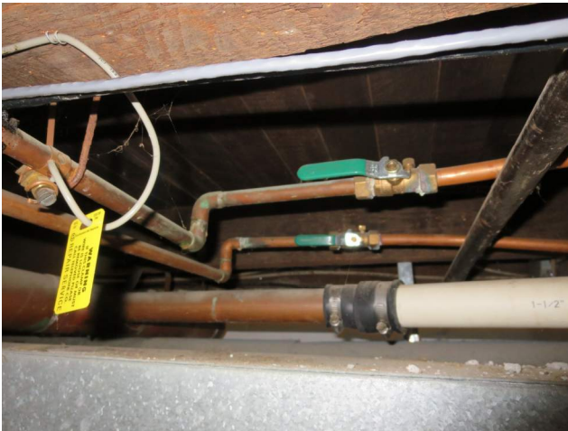
Figure 278. Existing copper piping in basement level. (Source: Alvine, 2022)
