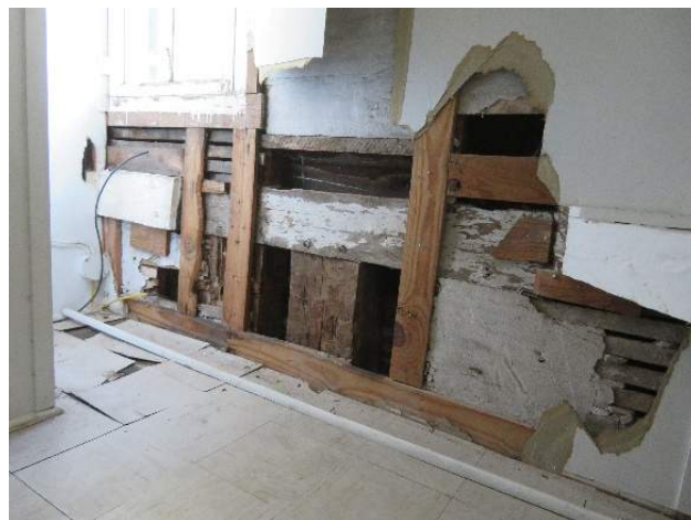
Figure 182. Portion of vertical log wall visible where finishes have been removed at the north wall within the northeast room at the second floor. (Source: RRJ, 2022)
