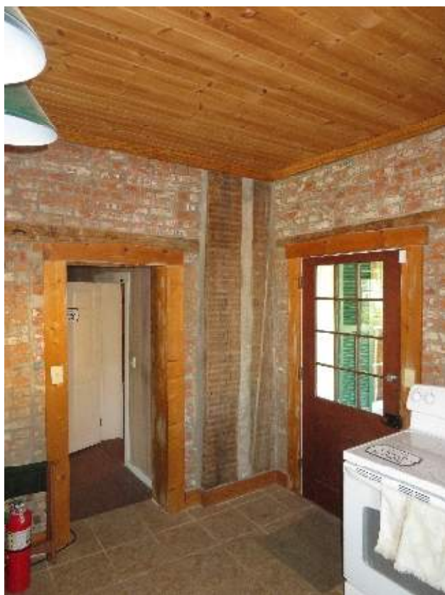
Figure 187. Two exposed vertical logs present within the first-floor kitchen. (Source: RRJ, 2022)
