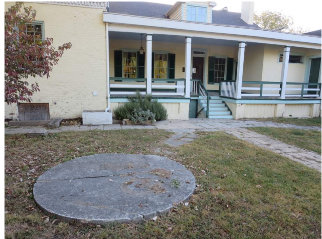
Figure 261. Photo of remaining cistern pump pad at courtyard. (Source: Alvine, 2022)
