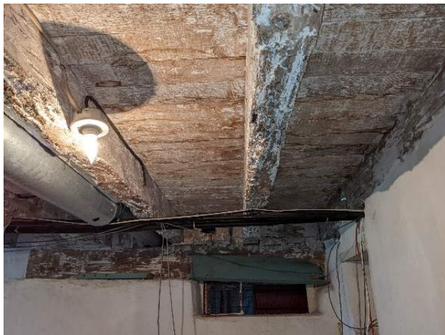
Figure 147. Overview of joists within room 006. (Source: RRJ, 2022)
