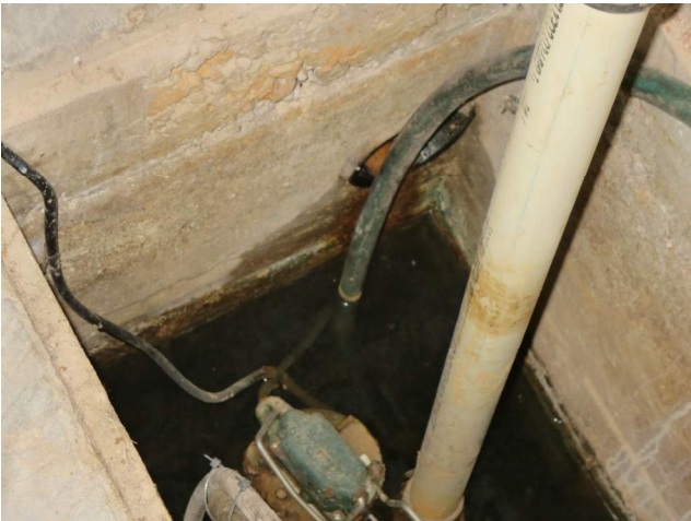
Figure 276. Existing below floor waste piping at the southwest corner of the sump pit where the waste pipe discharges into the pit (drain line with the green hose in front of it). (Source: Alvine, 2022).
