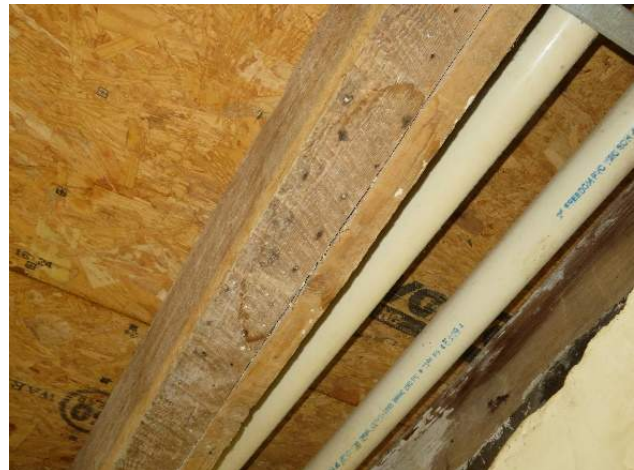
Figure 136. Underside of joist and plywood planking. (Source: RRJ, 2022)
