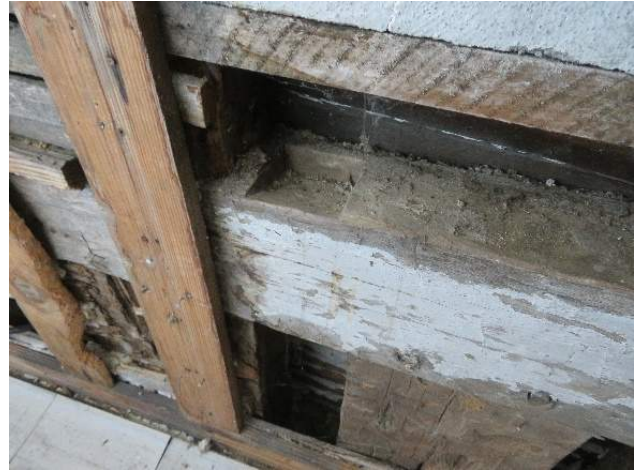
Figure 186. Notch within the top face of the timber top plate within the vertical log wall. This notch once received a hip rafter from the original roof. (Source: RRJ, 2022)
