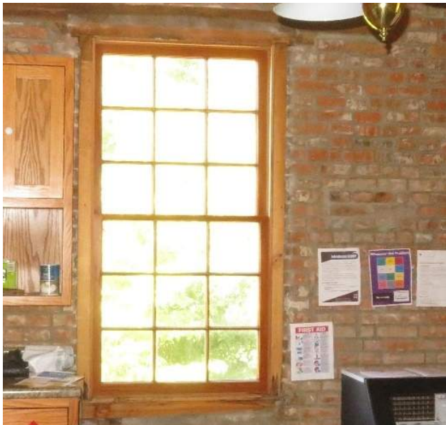
Figure 93. Interior view of typical nine-over-nine double hung window (Source: RRJ, 2022).
