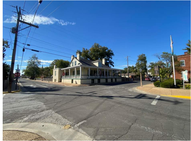
Figure 380. View of the intersection of Market and South Main Streets where the curb cuts need evaluation in order to ensure accessible routes are available to visitors from the accessible parking space at the welcome center to the Jean Baptiste Vallé House entrance. (Source: LSHLA, 2022)
