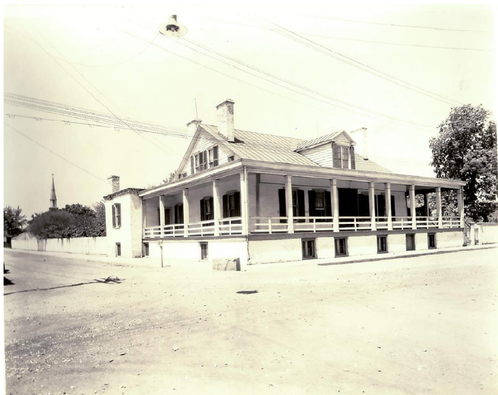
Figure 41. Undated (possibly 1930s), exterior from the southeast corner of Market and Main Streets. (Source: Schram Collection, Felix Vallé State Historic Site)
