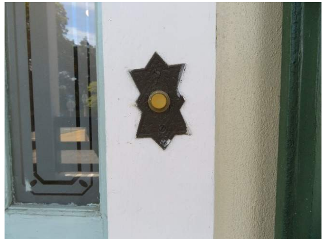
Figure 101. Press-button style doorbell with a cast brass octogram shaped plate at D101 (Source: RRJ, 2022)
