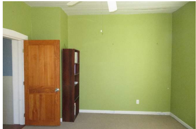
Figure 113. Interior view of Room 113 showing no exterior access at D113B location. (Source: RRJ, 2022)
