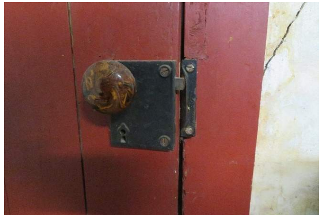
Figure 245. Door Hardware at Door D002. (Source: RRJ, 2022)
