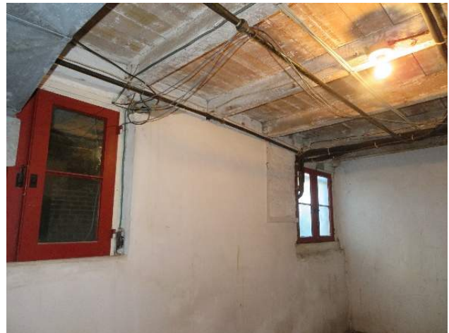
Figure 151. Overview of joists within room 007. (Source: RRJ, 2022)
