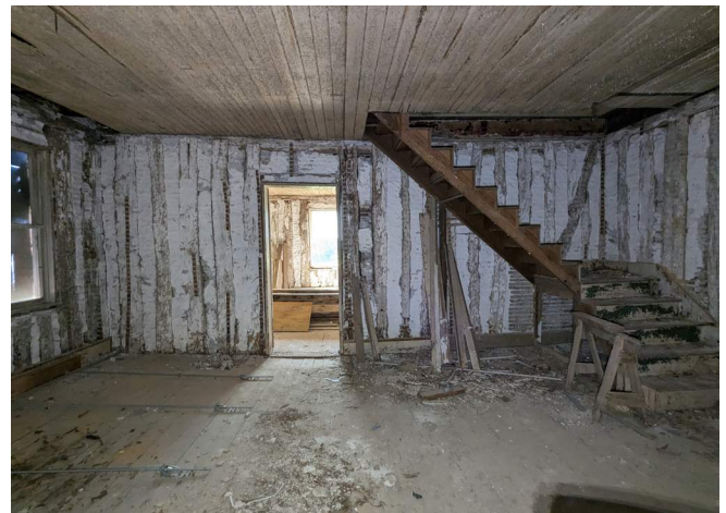
Figure 47. Room 105, looking south, showing the exposed vertical logs. (Source: RRJ 2023)
