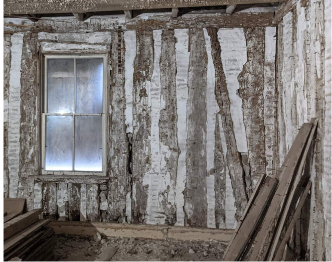
Figure 37. The east wall of Room 106 at the Delassus-Kern House. Note the steeply pitched brace on the right. (Source: MoDNR Felix Vallé House archives.)
