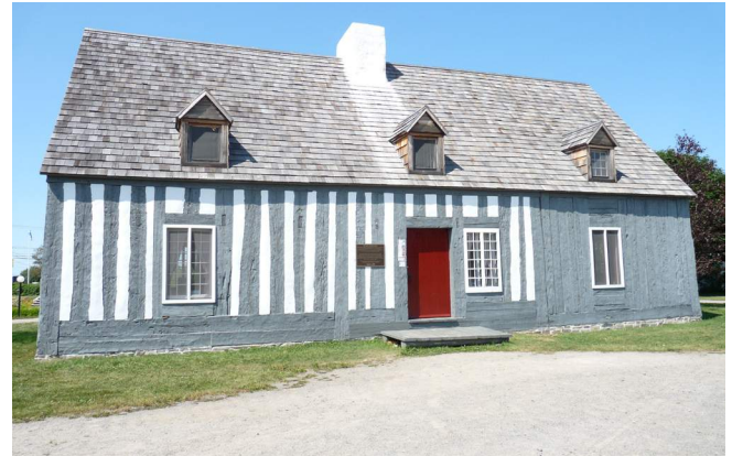
Figure 34. Maison Lamontagne, built in 1744 in Rimouski, Quebec, one of the oldest half-timbered structures in Quebec, following pan-de-bois building tradition. (Source: Site Historique de la Maison Lamontagne, https://maisonlamontagne.com )
