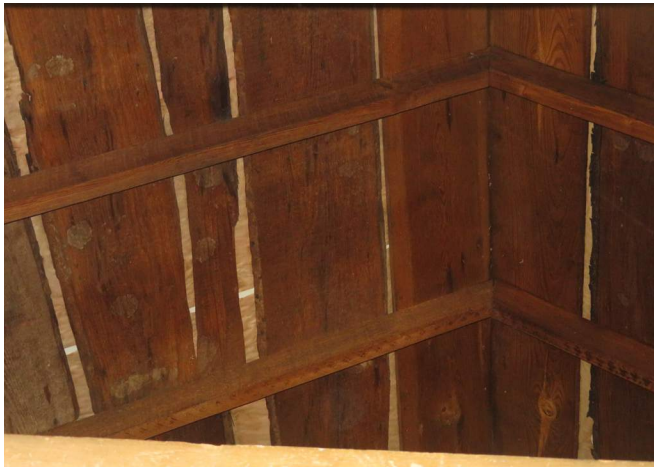
Figure 147. View of the underside of the roof sheathing, showing paired rafters and wany planks. (Source: RRJ 2023)
