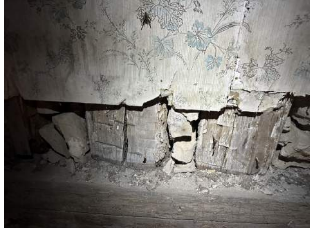
Figure 15. Vertical logs are resting on the sill.
