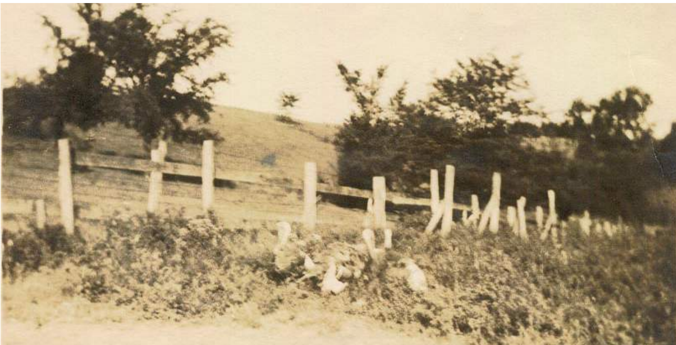
Figure 4. Undated photograph of the property, possibly looking west at the bluff, showing the post and rail fencing, turkeys, and possibly chickens. (Source: MoDNR Felix Vallé House archives.)
