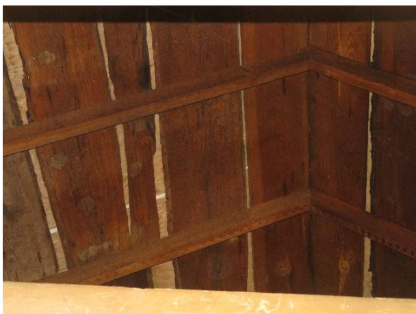
Photo 52. 2x4 dimensional lumber roof rafters spaced at 24 inches on center and planking (bark still in place).
