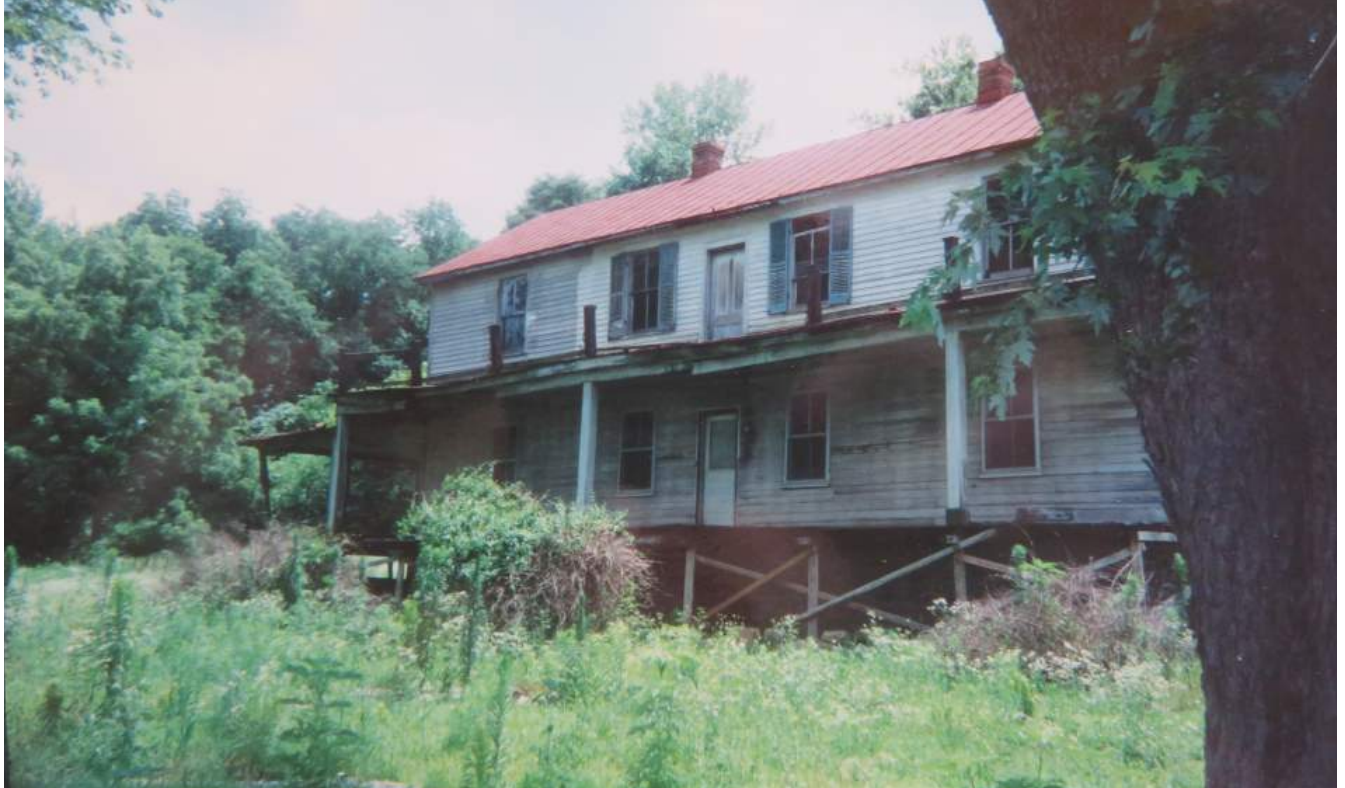
Figure 32. Photograph c. 1995, of the east exterior wall, showing the poor condition of the house and the collapsing double porch. (Source: MoDNR Felix Vallé House archives)
