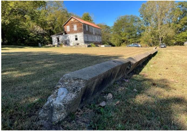
Photo 57. Concrete retaining wall at eastern edge of property
