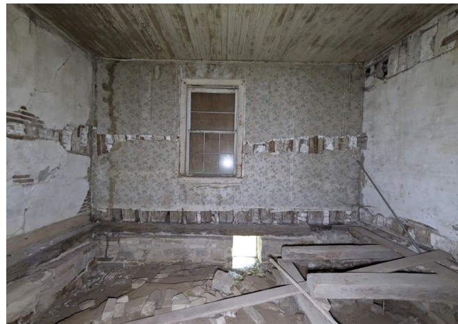
Figure 167. Room 103, looking north. (Source: RRJ 2023)
