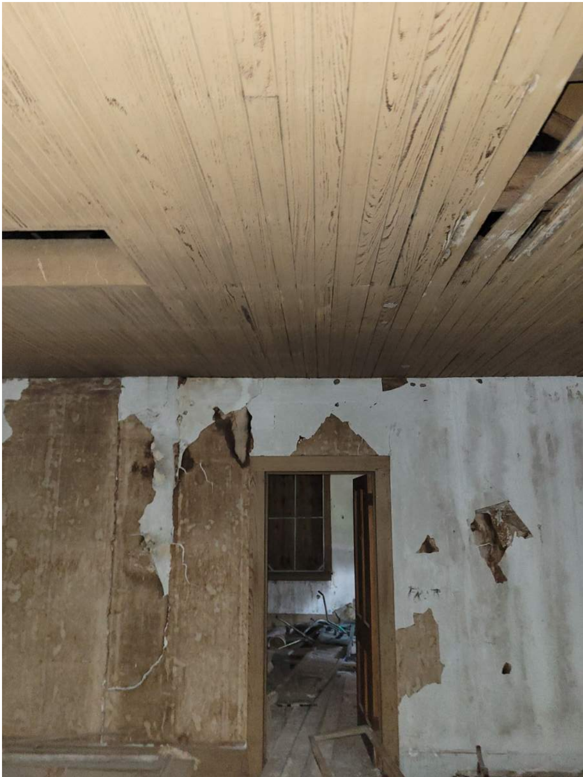
Photograph 19: LBP closet door frame Room 203.
