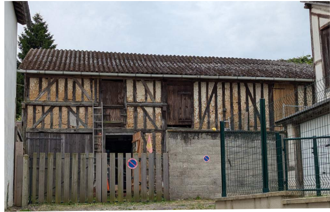
Figure 31. A stable, possibly 18th century, in Saint-Georges-du-Vieuvre, Normandy, France, with close-stud pan-de-bois construction. (Source: Lurita McIntosh Blank, 2024)
