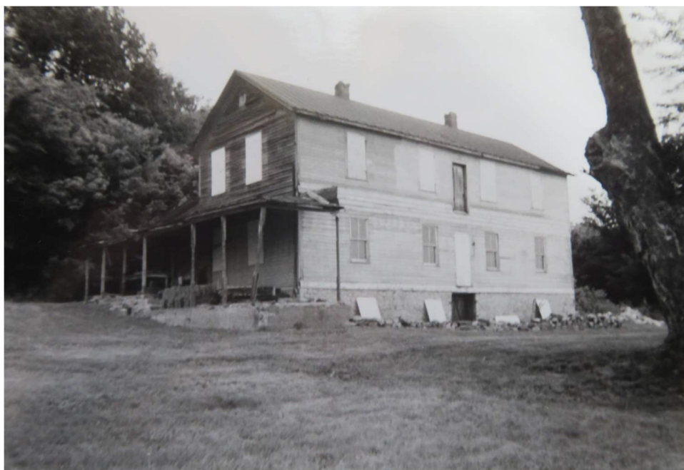
Photo 15. The house as it appeared in July 2000, after the removal of the porch on the east façade.
