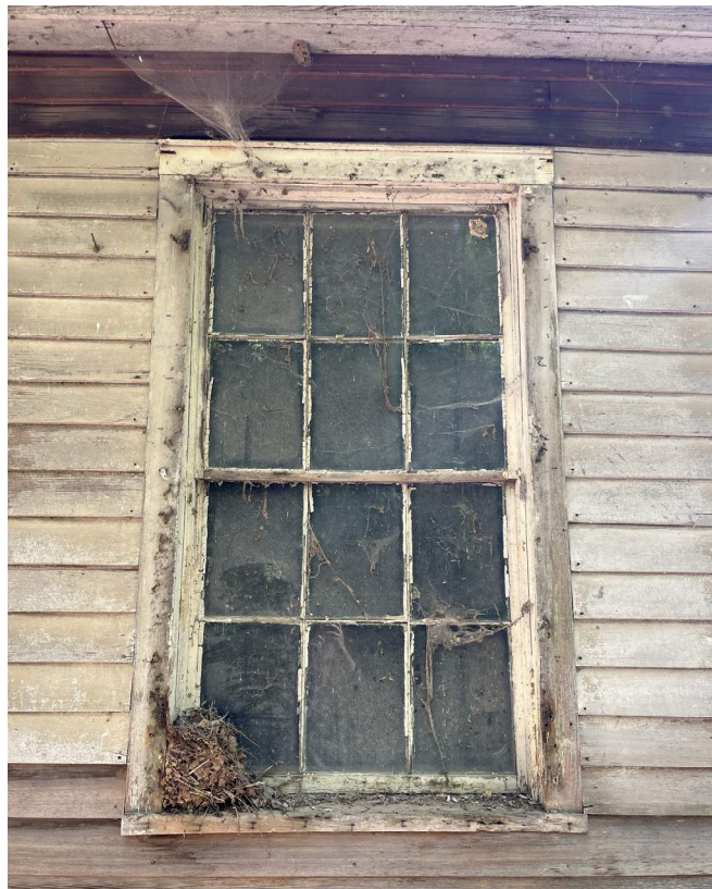
Figure 109. W102A, a first floor window on the west wall, likely a window unit that predates the 1903 alterations to the house. (Source: RRJ 2023)
