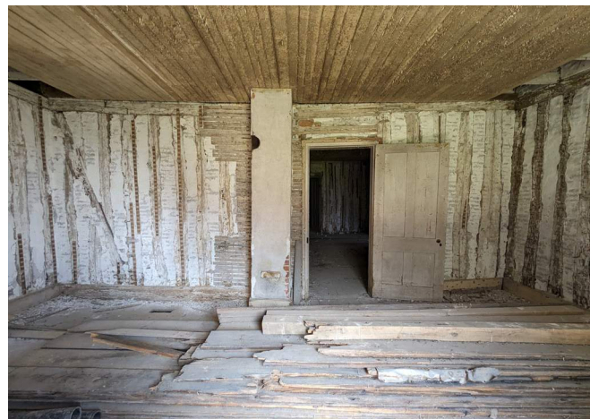
Figure 181. Room 106, looking north. (Source: RRJ 2023)
