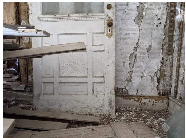
Photo 89. Ornamental panels and moulding on exterior door, with ornate hardware.
