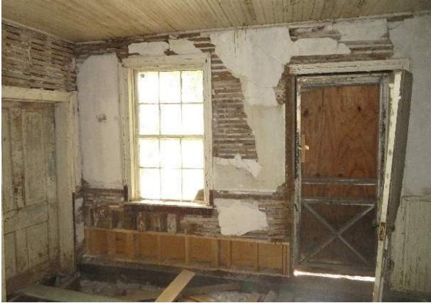
Photo 23. The west vertical log wall as viewed from within Room 102. The dimensional lumber knee wall and replaced bottom plate extend along approximately half of this wall between the south wall and the exterior door.
