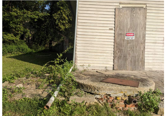
Figure 79. Kitchen cistern, located on the south porch, immediately outside the kitchen door. (Source: LSHLA 2023)
