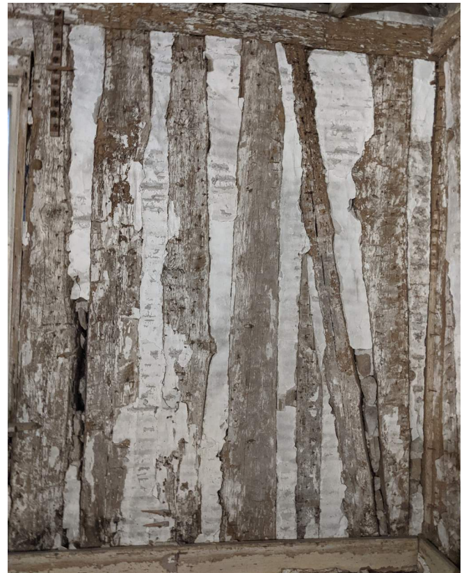
Figure 131. Vertical log walls with corner bracing in Room 106. (Source: RRJ 2023)
