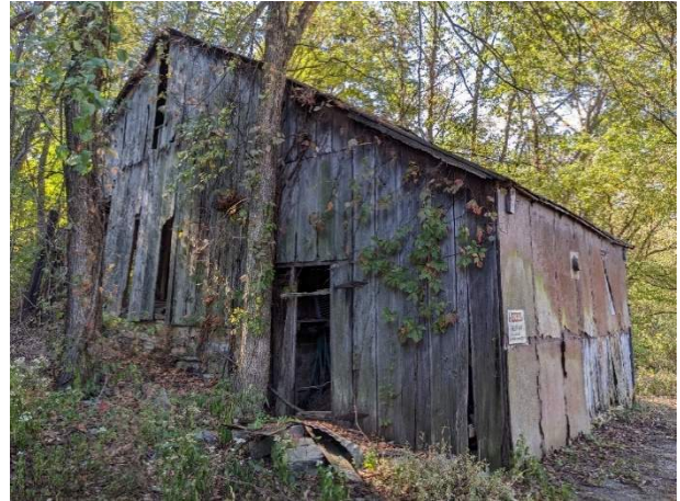
Photo 67. Wood shed exterior, south and east walls.
