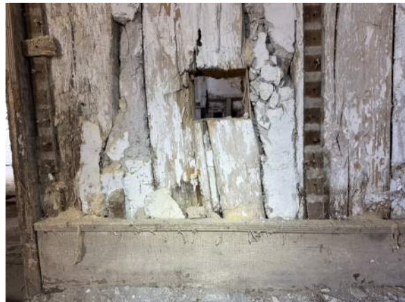
Figure 30. Opening in the interior wall log.
