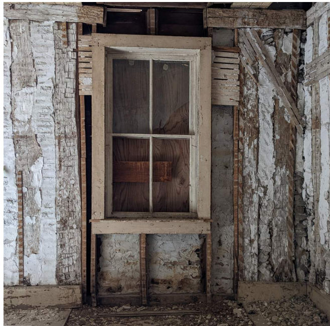
Figure 114. W106B, a first floor window on the south wall, showing the stud frame infill where the stone masonry chimney was removed. (Source: RRJ 2023)
