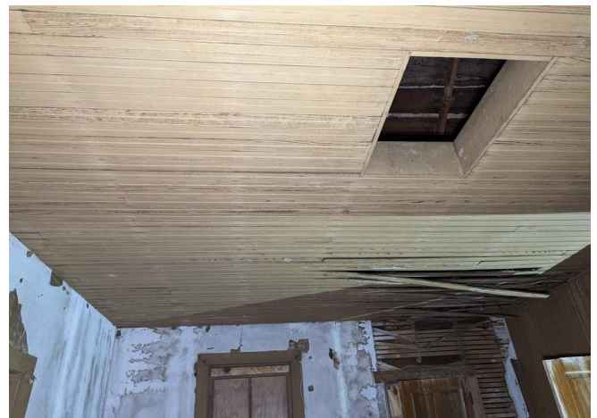
Figure 201. Beadboard ceiling with the attic access hatch in Room 203. (Source: RRJ 2023)
