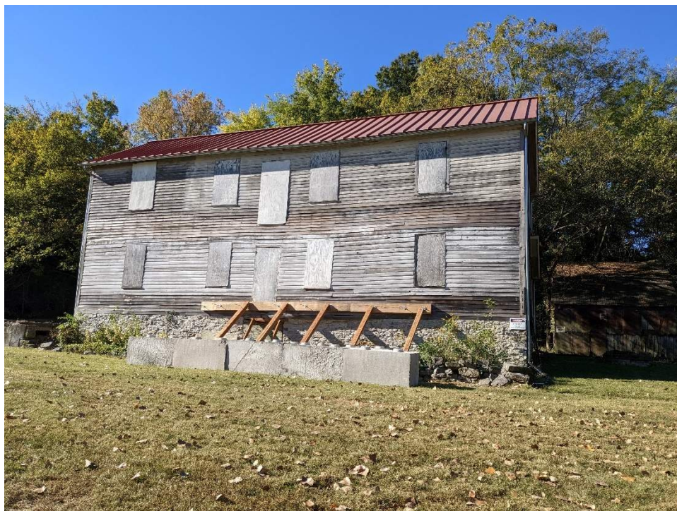
Photo 5. East (main) exterior wall of the Delassus-Kern House in October 2022, with first-floor shoring in place.
