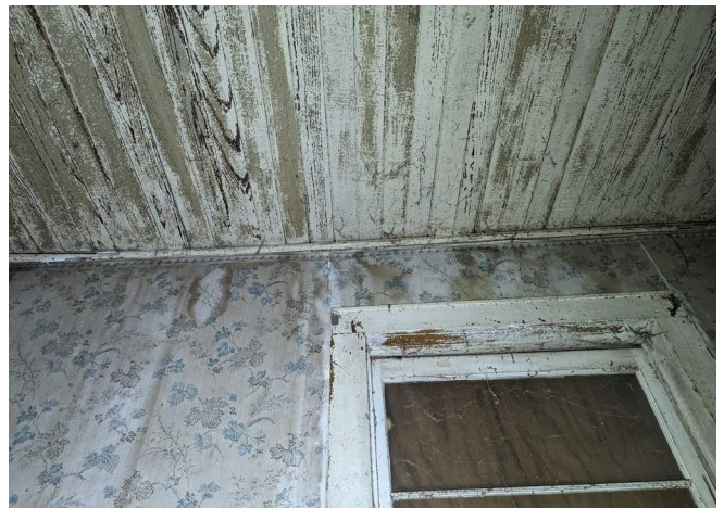
Figure 170. Detail of north wall and ceiling beadboard in Room 103. (Source: RRJ 2023)
