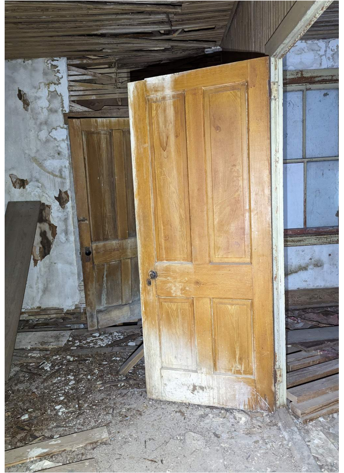
Figure 157. D204, showing faux graining on south face. (Source: RRJ 2023)
