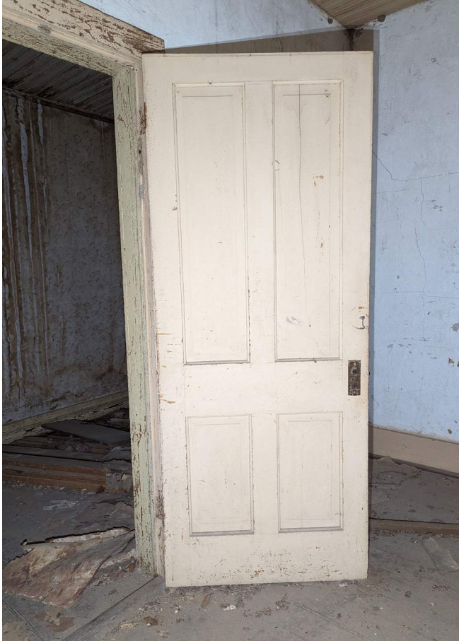
Figure 156. D201, showing the north face. (Source: RRJ 2023)
