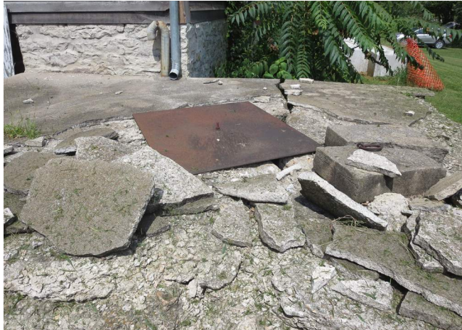
Figure 209. Second cistern located near the southeast corner of the house. (Source: Alvine 2023)
