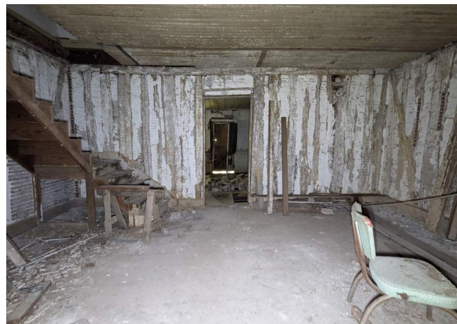
Figure 177. Room 105, looking west. (Source: RRJ 2023)
