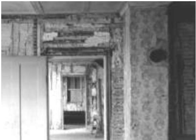
Figure 219. Existing first level on the other side of the same wall where a chimney exists where another round opening is present for a wood stove connection. (Source: Alvine 2023)
