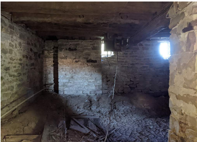
Figure 43. Room 001, looking north. (Source: RRJ 2023)
