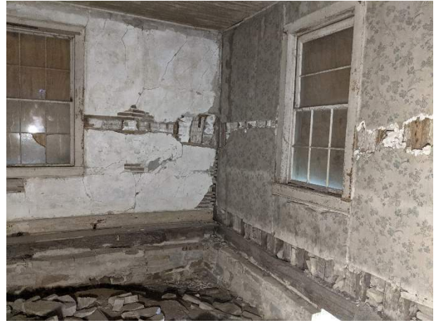
Photo 18. Remaining interior finishes at the west and north exterior walls of Room 103.
