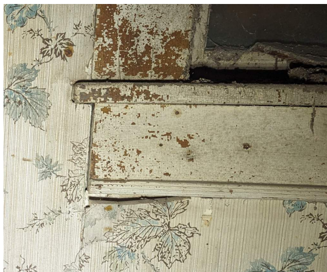
Figure 111. Applied moulding at the apron of W103A. (Source: RRJ 2023)
