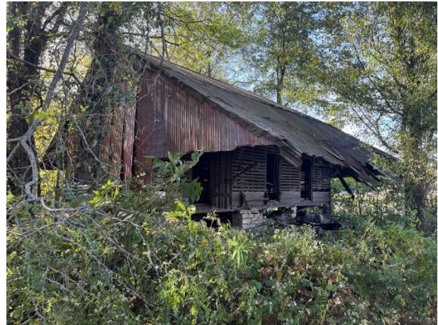
Photo 70. Exterior of corn crib.
