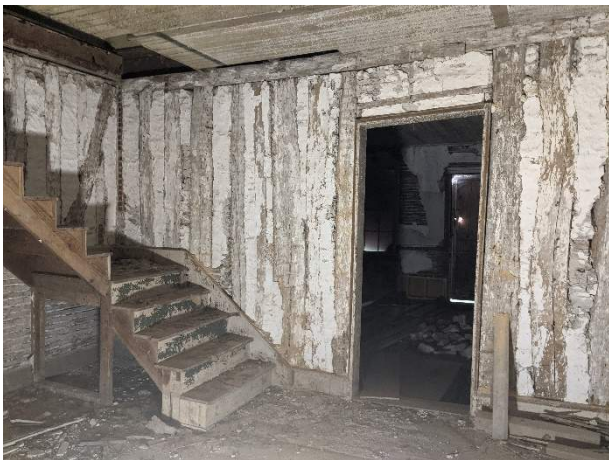
Photo 17. Vertical log walls on the south interior wall and west interior wall of Room 105.
