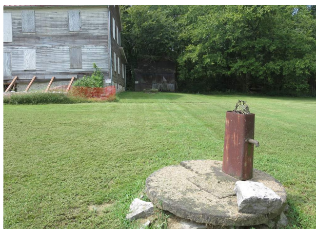
Figure 207. Existing well located 40-50 feet northeast of the house. (Source: Alvine 2023)
