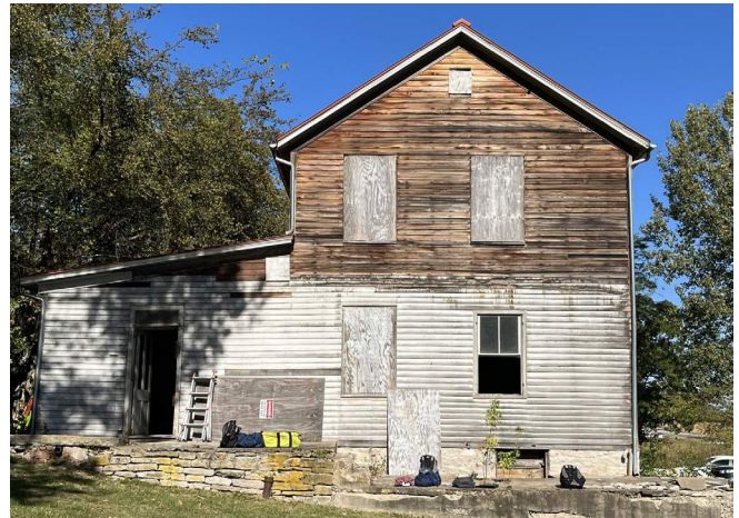
Figure 98. South exterior wall, showing localized replacement of siding at the upper level. (Source: RRJ 2023)
