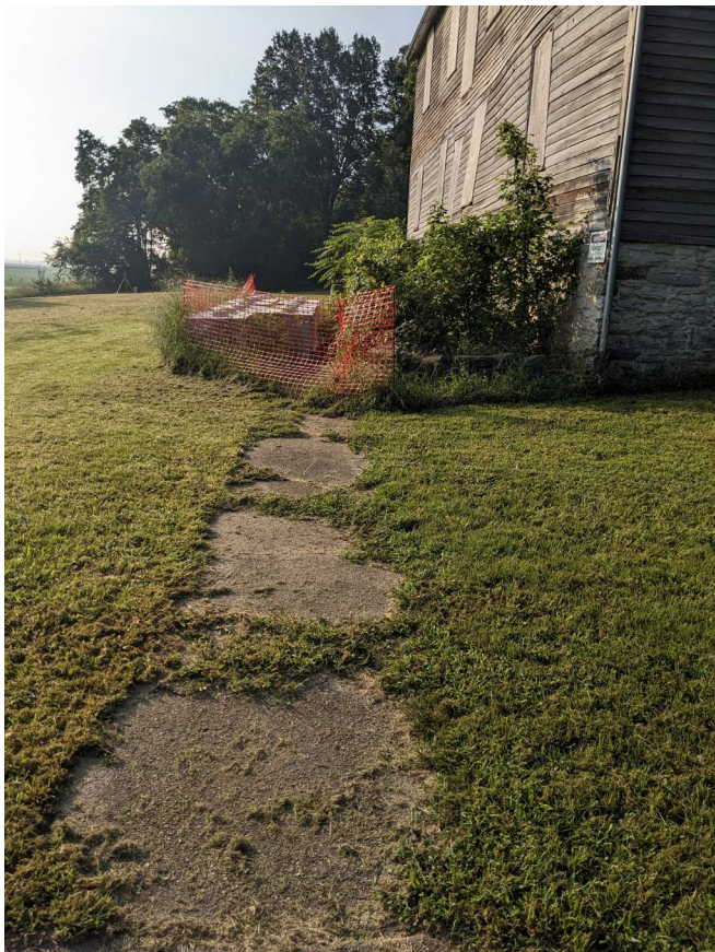
Figure 86. View southeast along the concrete walk connecting the driveway with the principal façade of the house. (Source: LSHLA 2023)
