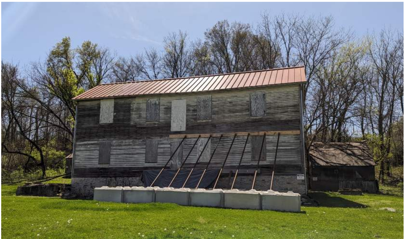
Figure 41. April 2024, after installation of the second floor bracing. (Source: RRJ 2024)
