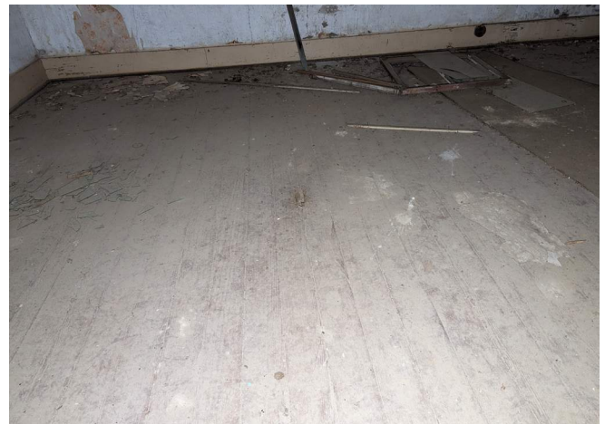
Figure 188. Wood flooring in Room 201; this flooring was typical throughout the second floor. (Source: RRJ 2023)
