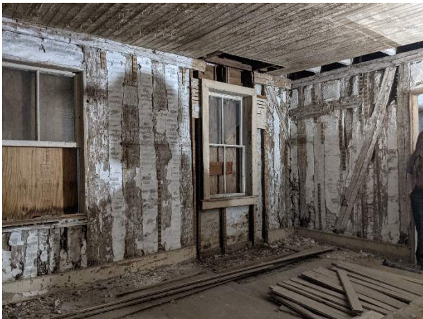
Photo 16. Vertical log walls on the south exterior wall and west interior wall of Room 104.
