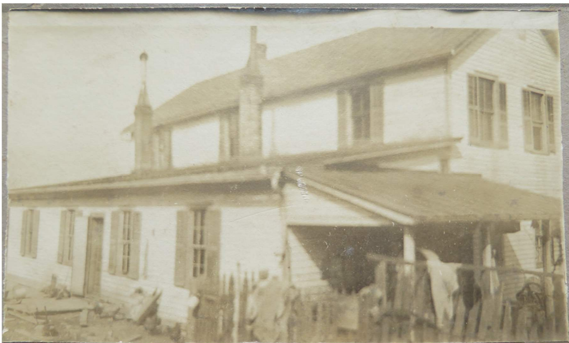
Photo 9. A c. 1900 photograph of the Delassus-Kern House from the southwest after the construction of the second story, showing the small, covered porch at the kitchen door. The roofing appears to be standing-seam metal panels. (MoDNR Archives, Felix Vallé House State Historic Site).
