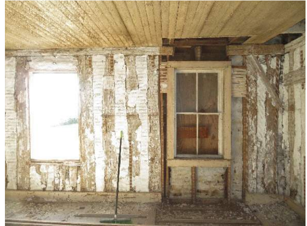
Photo 25. The south vertical log wall as viewed from within Room 106, showing dimensional lumber framing at the righthand window. This was the previous location of a stone masonry chimney. Note the original log framing at the lefthand window opening.
