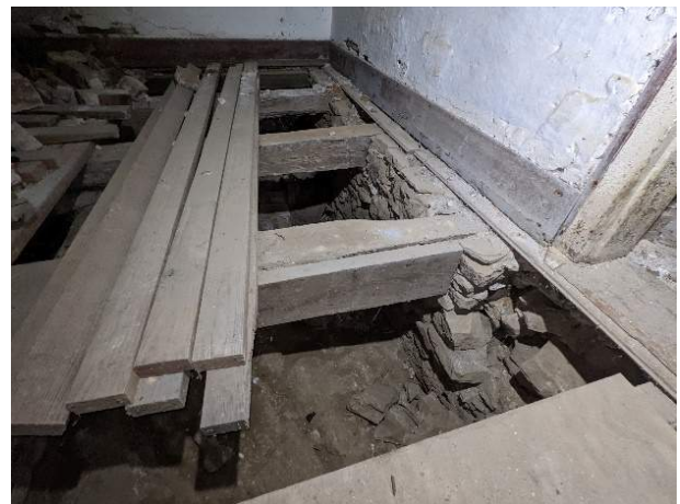
Photo 42. Joists within room 102.
