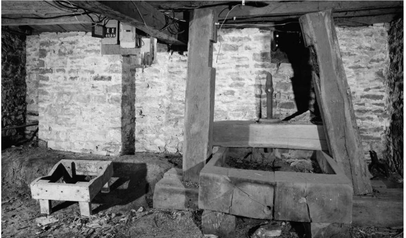
Figure 24. 1985 photograph of the basement, showing the historic wine press (now stored in the Ste. Genevieve NHP headquarters). (Source: HABS)
