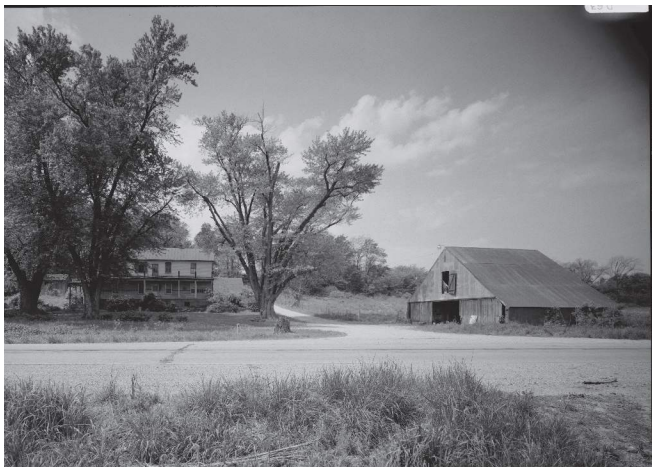
Figure 61. Photographs of the property from the parcel across the highway showing the driveway, house, and a utility shed that is no longer extant in. (Source: 1985 HABS)
