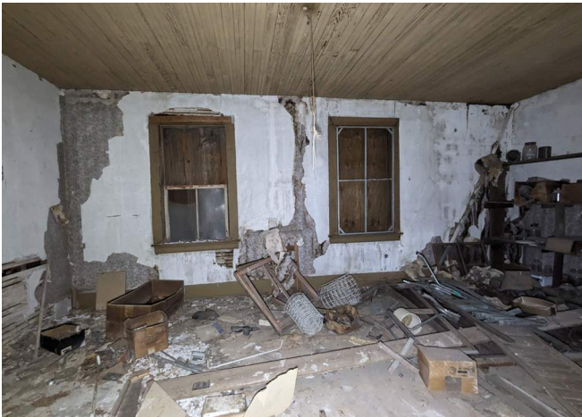
Figure 202. Room 204, looking north. (Source: RRJ 2023)
