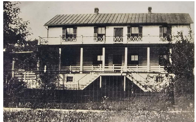
Figure 123. Undated photograph (possibly 1950s) of the east wall, showing the split staircase to the east porch and upper gallery railing. (Source: Volz, "Pierre Delassus de Luziere House (Kern House) Condition Assessment Report," original source not cited.)
