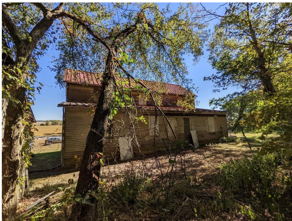
Photo 4. West (rear) exterior wall of the Delassus-Kern House in October 2022.
