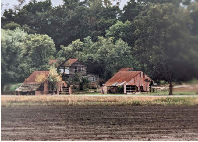
Figure 65. A 1993 photograph of the property showing the condition of the grounds and outbuildings immediately after the flood. (Source: Ste. Genevieve NHP archives)
