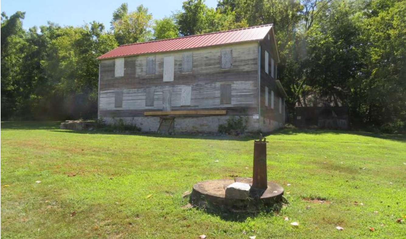
Figure 39. August 2022, view of the east exterior wall during installation of the first floor bracing. (Source: RRJ 2022)
