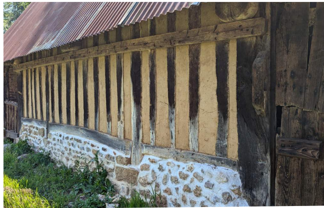
Figure 32. 18th or 19th century farm structure on the grounds of the Château de Bailleul in Picardy, France, with close-stud pan-de-bois construction. (Source: Lurita McIntosh Blank, 2024)
