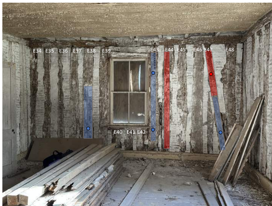
Figure 24. Section of the east wall. Room VI.
