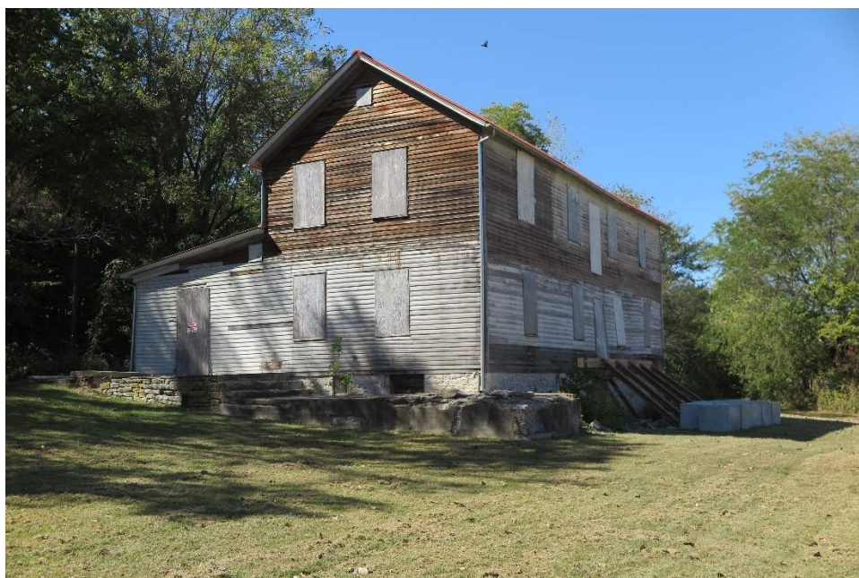
Photo 6. Southeast corner of the Delassus-Kern House in October 2022, with first-floor shoring in place.
