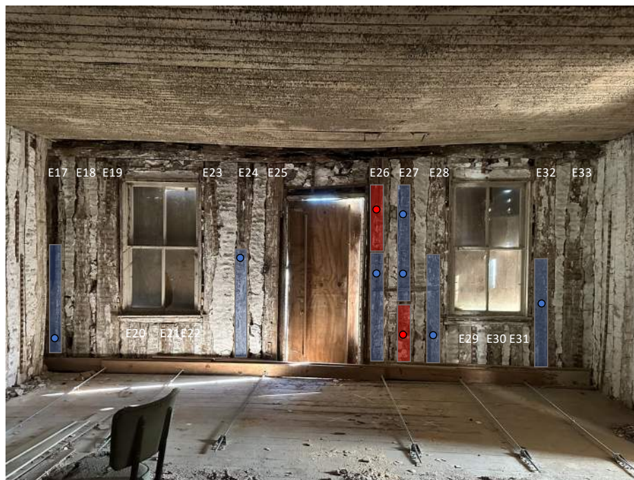
Figure 23. Section of the east wall. Room V.
