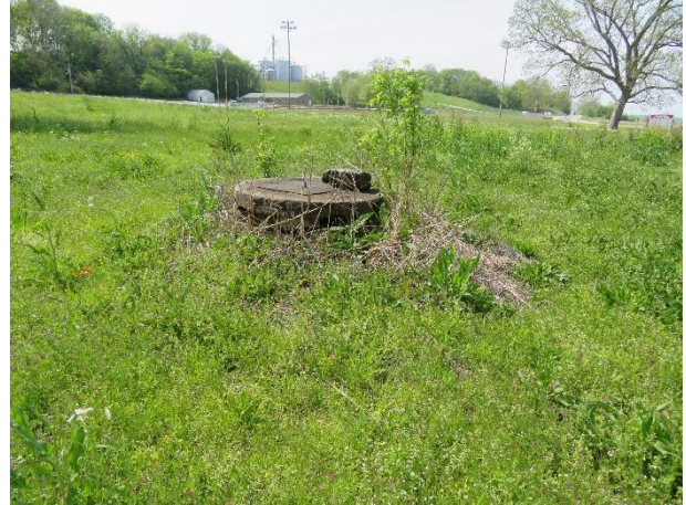
Photo 63. Well in the field to the north of the corn crib with a stone cap. The well had not been backfilled.
