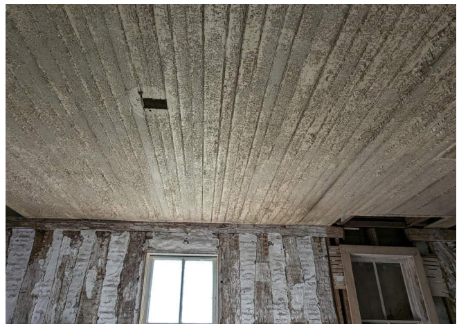
Figure 184. Beadboard ceiling in Room 106. (Source: RRJ 2023)
