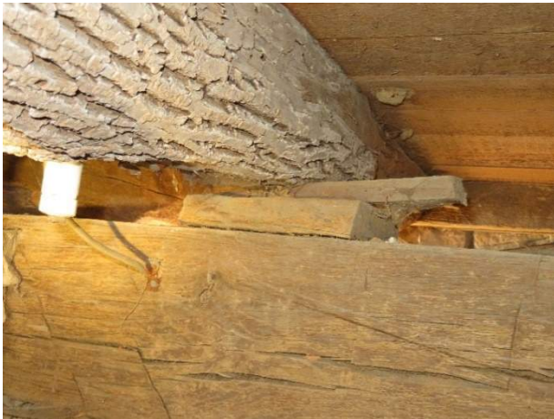
Photo 45. Shims present between joist 21 and girder.
