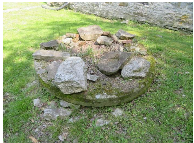
Photo 60. Cistern on the north side of the house. This cistern has also not been backfilled.
