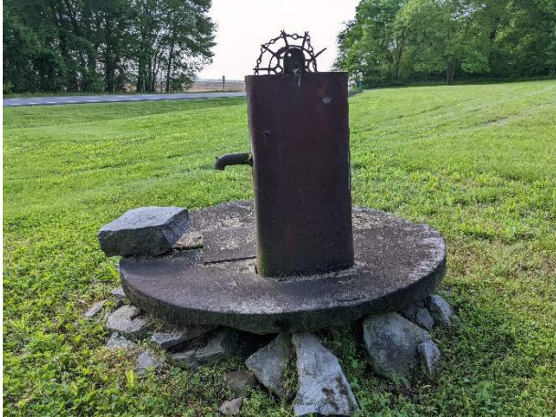
Photo 61. Cistern on front lawn is distressed. The cistern has not been backfilled and is partially filled with water.
