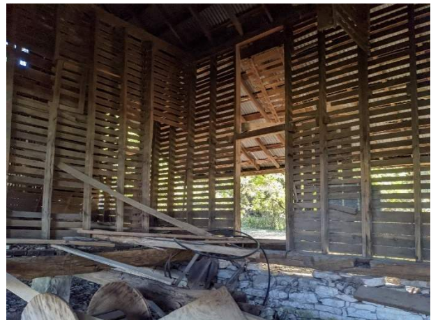
Photo 72. Interior of corn crib including slatted walls, masonry foundation, and access opening
