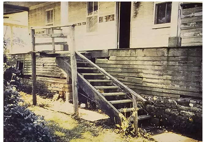
Figure 124. 1990s photograph of the east porch stairs. (Source: Volz, "Pierre Delassus de Luziere House (Kern House) Condition Assessment Report,")
