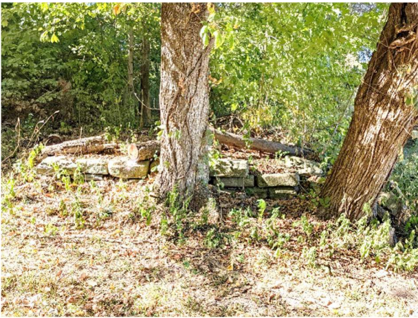
Photo 73. Foundation of former smoke house.
