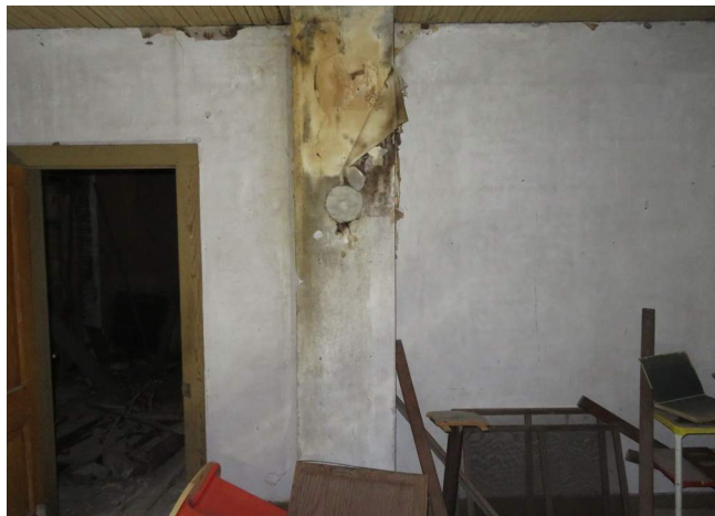
Figure 121. Chimney in Room 204, showing capped opening for the stove flue. (Source: RRJ 2023)
