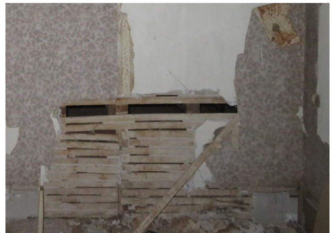
Figure 138. Exposed wall framing in Room 204, west wall, looking into the attic space of the lower roof. (Source: RRJ 2023)
