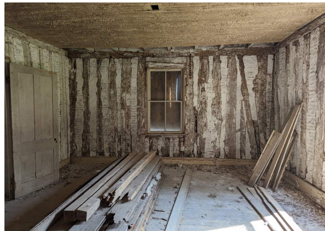
Figure 180. Room 106, looking east. (Source: RRJ 2023)
