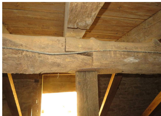
Figure 142. Splice in north-south girder at the wood post. (Source: RRJ 2023)
