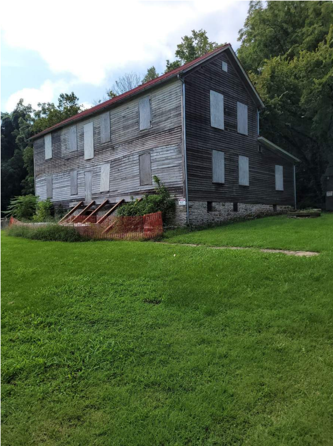
Photograph 1: Facing toward the north and east exterior (LBP lap siding and windows).
