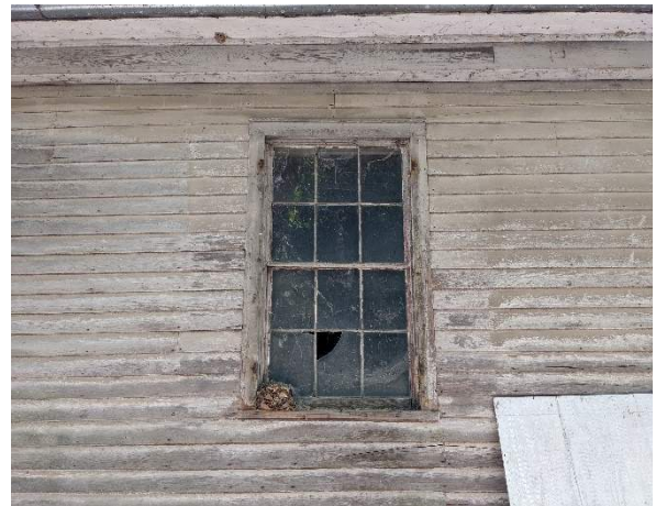
Photo 83. Window 103A on west wall, showing 6-over-6, double hung sash.
