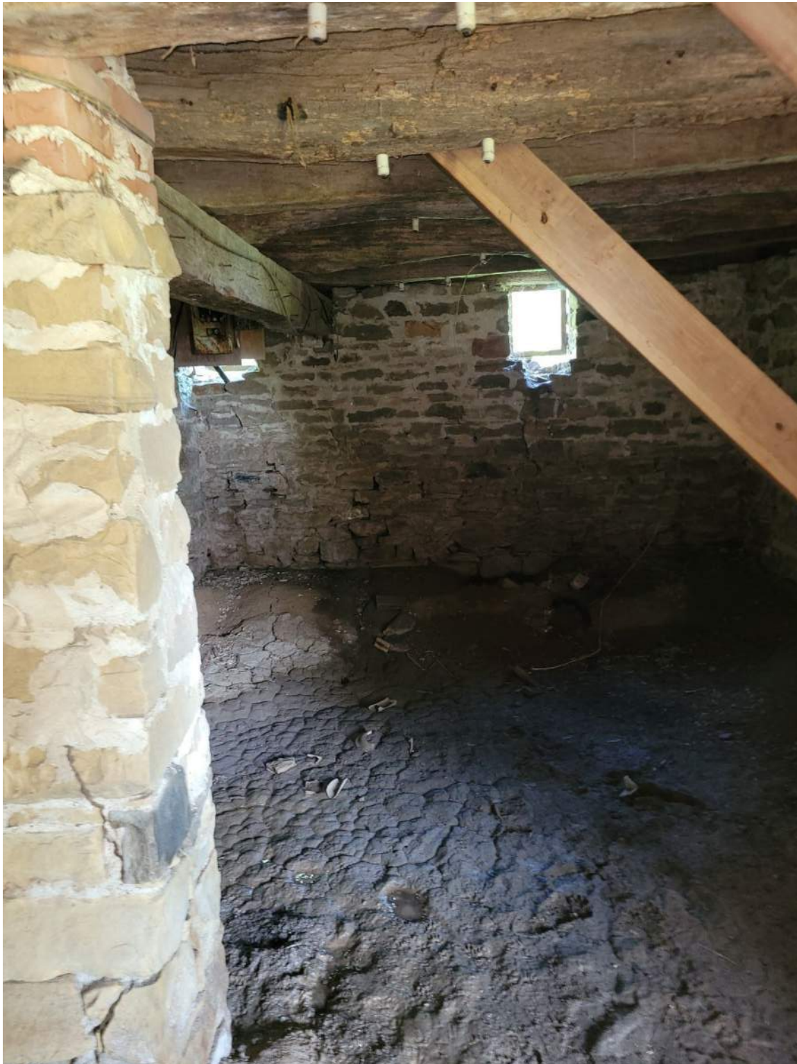
Photograph 22: View of basement no suspect hazardous materials observed.
