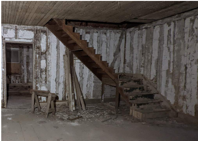
Figure 125. Stairs in Room 105, looking south. (Source: RRJ 2023)
