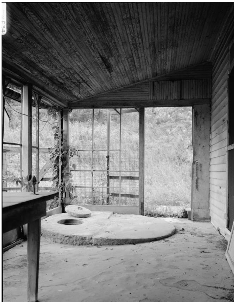
Figure 23. 1985 view looking west of the interior of the screened-in porch next to the kitchen door, showing the cistern with no pump. (Source: HABS)
