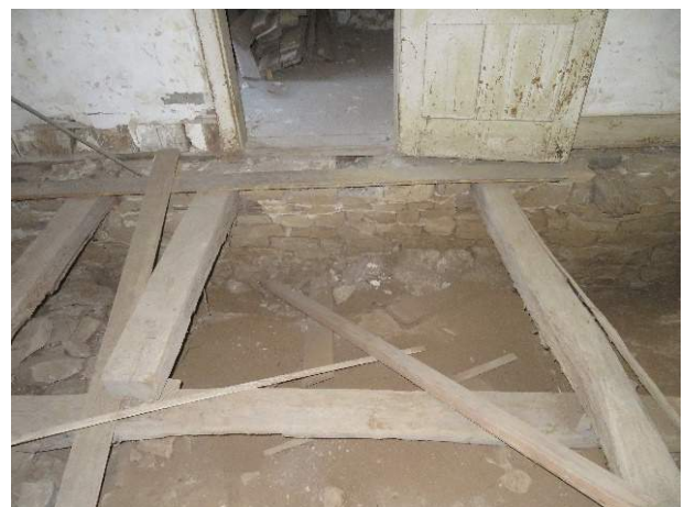
Photo 43. Framing joists and girder resting on ground within room 103.
