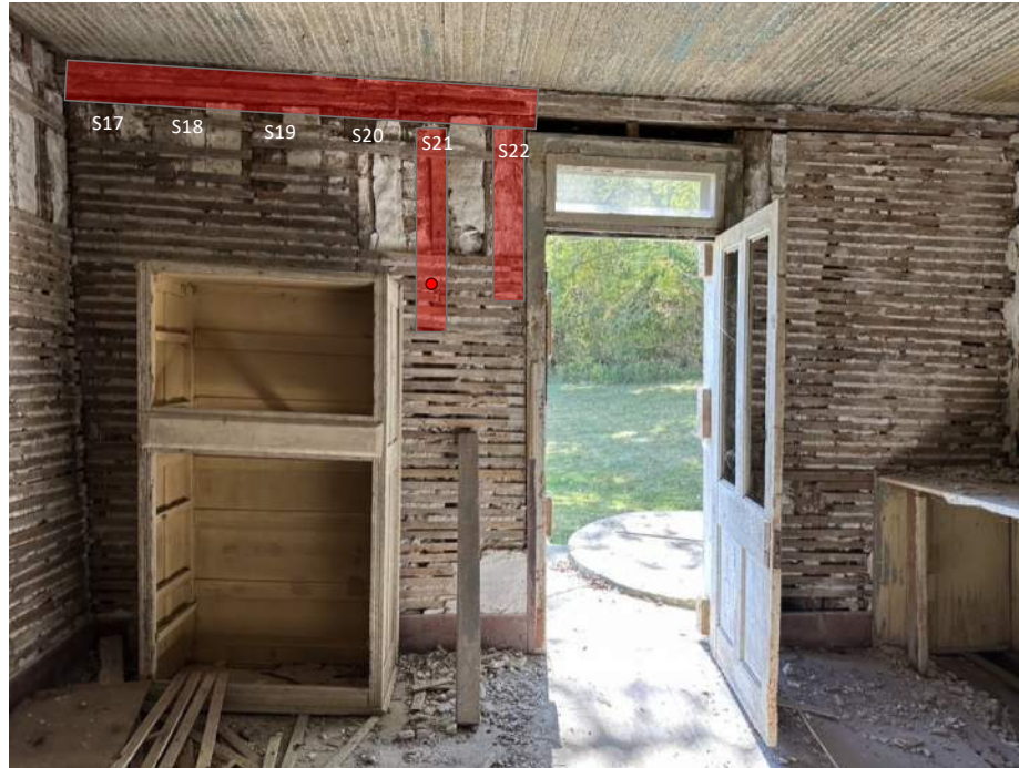
Figure 26. Section of the south wall. Room I.
