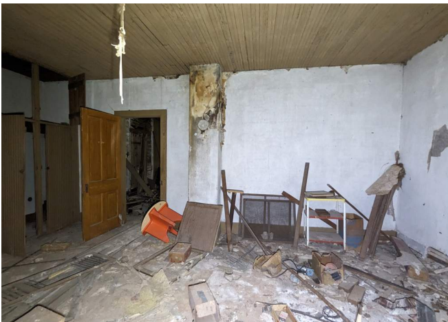
Figure 203. Room 204, looking south. (Source: RRJ 2023)
