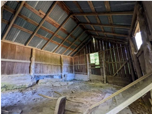
Photo 66. Interior and roof framing of chicken house.
