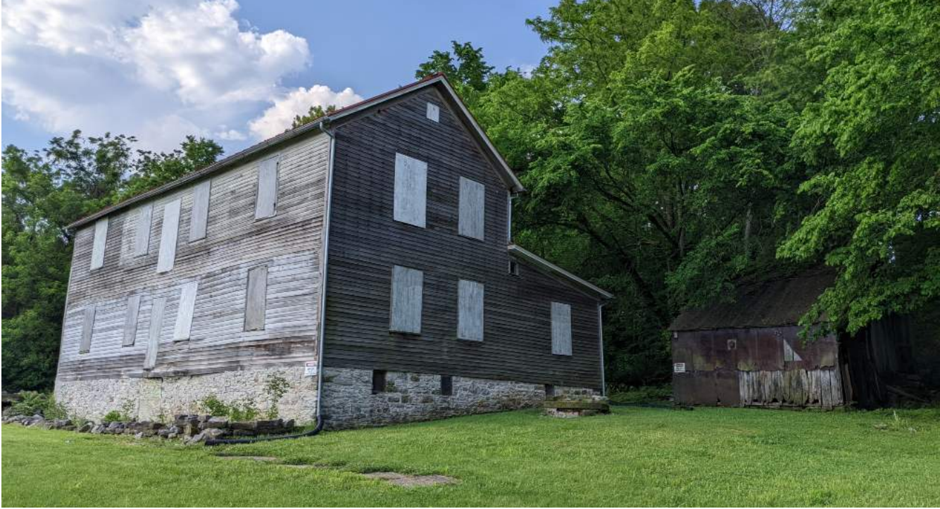
Figure 38. May 2002, view of the north and east exterior walls, with the wood shed at right. (Source: RRJ 2022)
