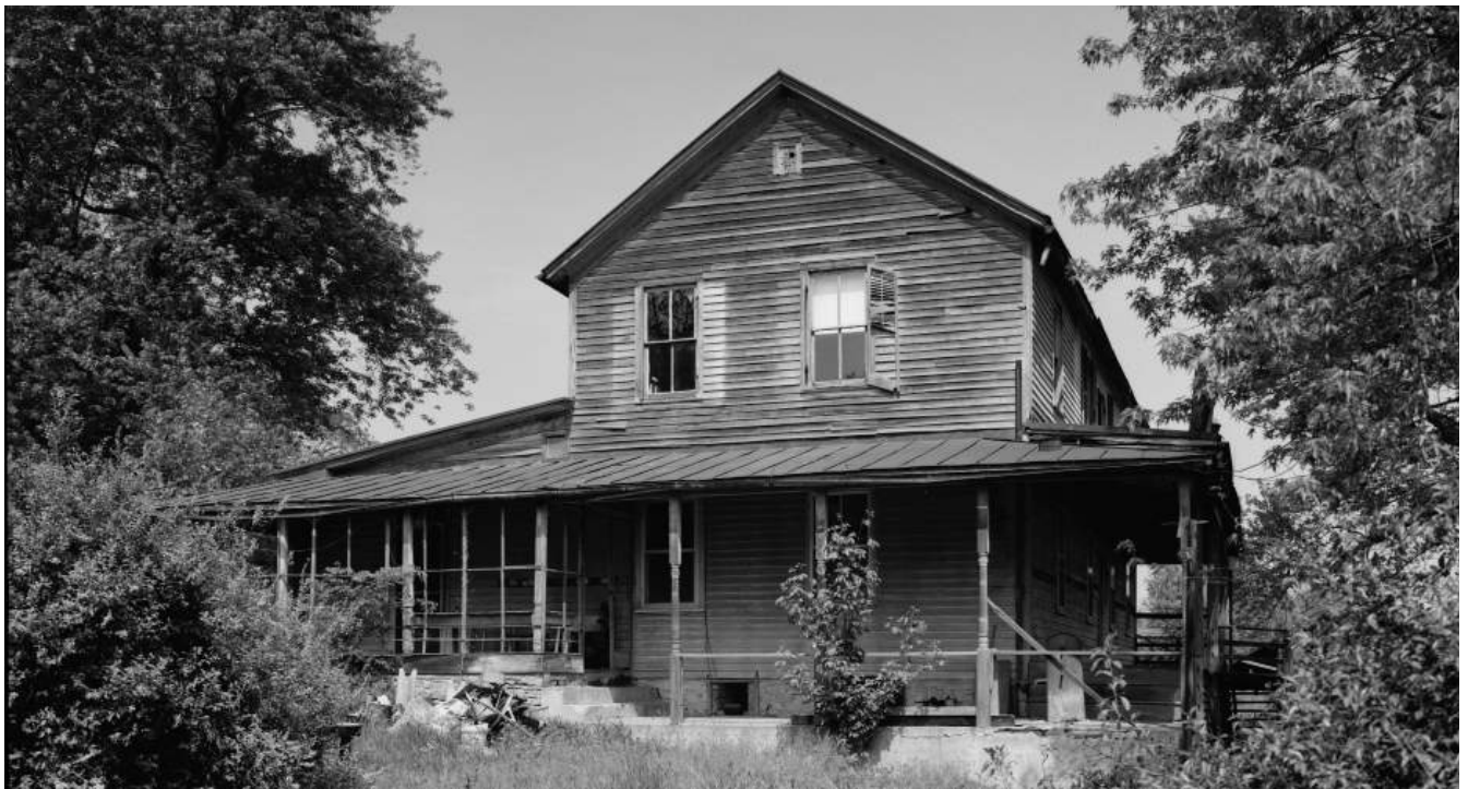
Figure 22. 1985 view of the south wall of the main house, showing the south porch and screened-in area next to the kitchen door. Note the pump housing on the southeast cistern (Source: HABS)
