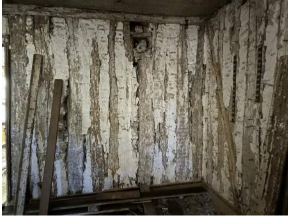
Figure 27. Interior partition wall showing similar construction techniques as for the exterior walls.
