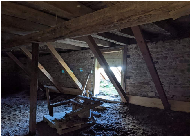
Figure 44. Room 001, looking northeast, showing the shoring in the basement. (Source: RRJ 2023)
