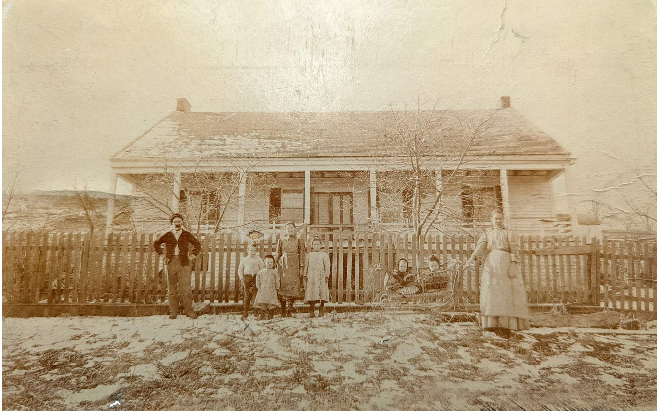
Figure 16. The earliest known photograph of the Delassus-Kern House, c. 1895, before the addition of the second story, with members of the Kern family. Note the gabled roof shape and the single gallery or porch on the front. The chimneys are brick, and the position of the chimneys in relation to the roof ridge suggests that the first floor is two rooms deep. (Source: MoDNR Felix Vallé House archives.)
