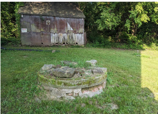
Figure 78. North yard cistern, adjacent to north exterior wall of house. (Source: LSHLA 2023)
