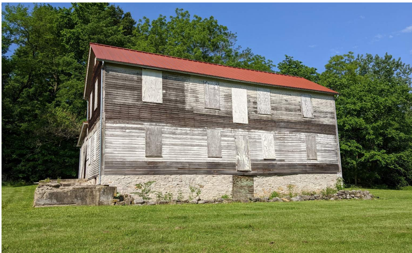
Delassus-Kern House, east facade.
