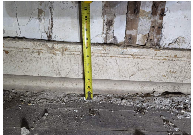
Figure 174. Baseboard with quarter round moulding. (Source: RRJ 2023)
