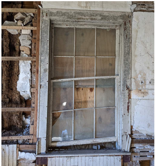
Figure 108. W101, showing the rectangular casing with the applied perimeter trim. (Source: RRJ 2023)
