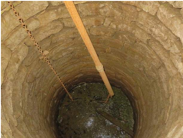
Photo 62. View into cistern.
