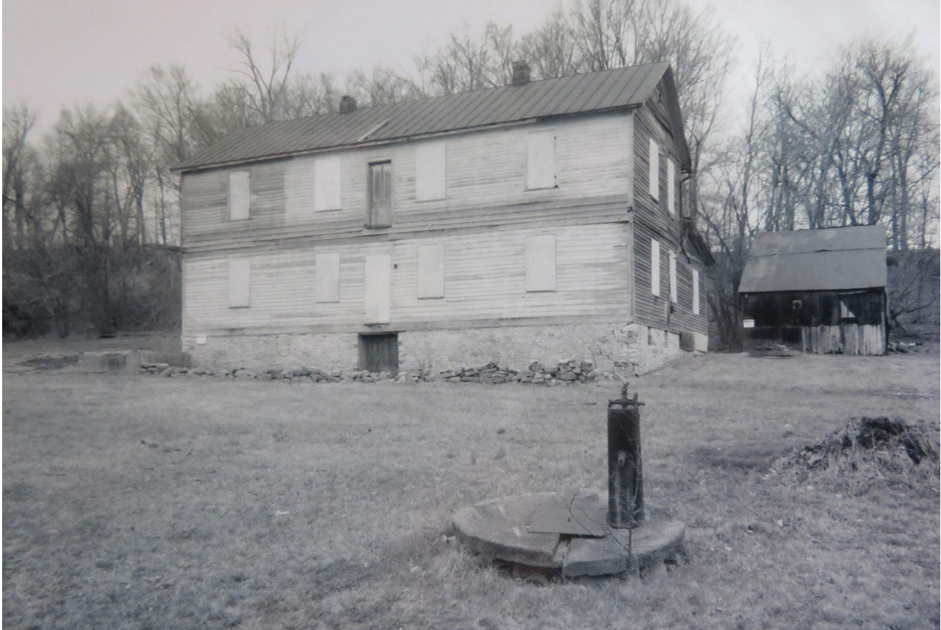
Figure 30. Photograph taken in July 2000, looking west, after the porches have been removed. (Source: MoDNR Felix Vallé House archives)
