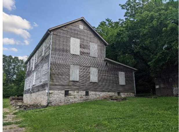
Photo 34. The masonry foundation walls, as viewed from northeast. The height of masonry walls increases from west to east, as the ground level slopes down toward the Common Field.
