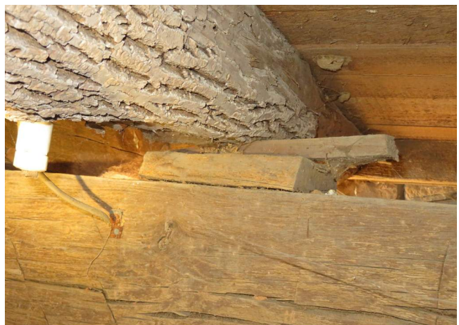
Figure 145. Shims between girder and floor joist. (Source: RRJ 2023)
