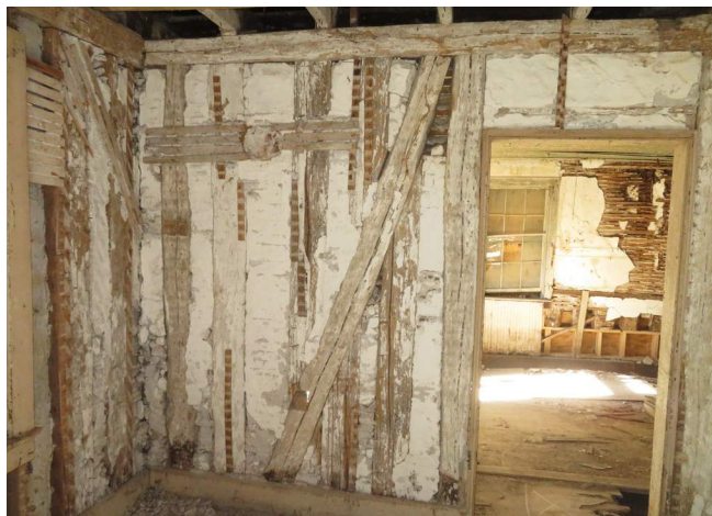
Figure 134. Log wall construction on the west wall of Room 106, looking into Room 101. (Source: RRJ 2023)
