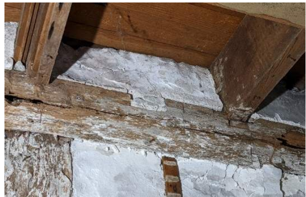
Photo 22. Vertical log top plate at the east exterior wall within room 104. Second-floor joists sit atop the existing top plate. Notches at the top of the top plate were likely created to receive the original roof framing members.
