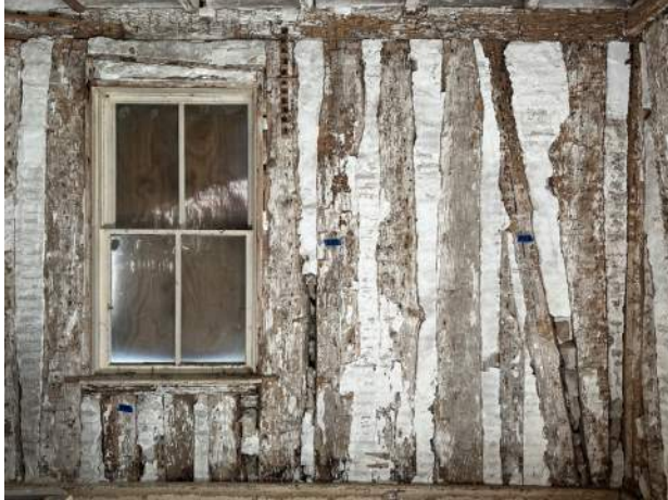
Figure 14. View of exterior wall showing hewn vertical logs and spaces between logs filled with pierrotage .
