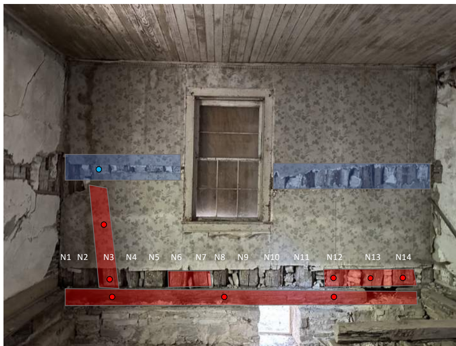
Figure 20. Section of the north wall. Room III.
