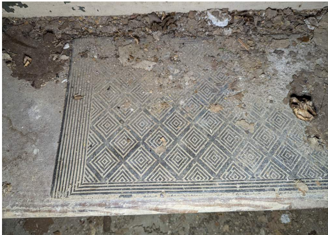
Figure 126. Linoleum tread cover. (Source: RRJ 2023)
