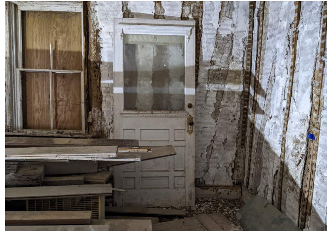
Figure 104. Unattached door in Room 106, likely Door D105. (Source: RRJ 2023)
