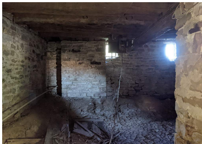
Figure 222. Fuse panel in basement, mounted to the floor structure in the upper right of the photograph. (Source: RRJ 2023)
