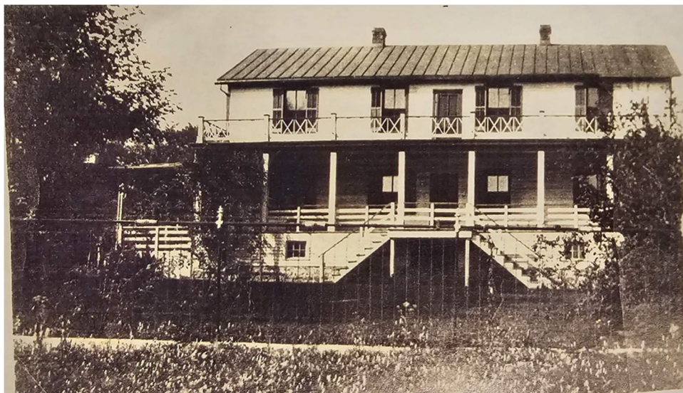
Photo 10. East façade of the house in the 1970s, before the porch, gallery, and front steps were removed. (Volz and Associates, "Pierre Delassus de Luziere House (Kern House) Condition Assessment Report," 1990.)
