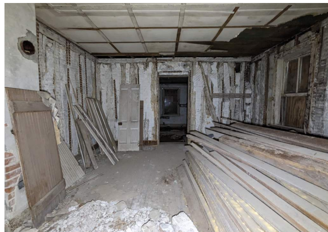
Figure 172. Room 104, looking west. (Source: RRJ 2023)
