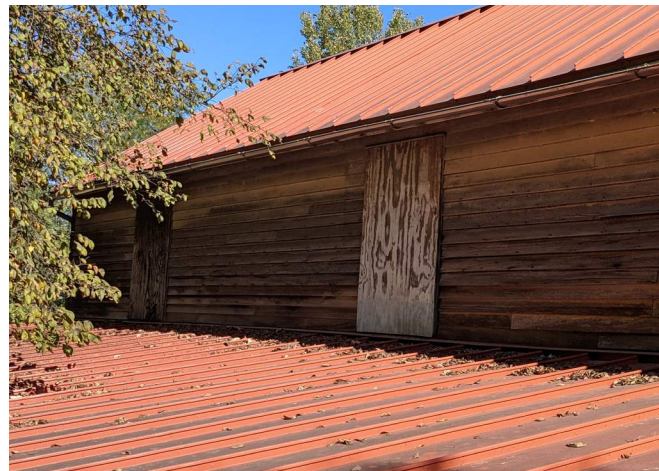
Figure 95. View of the standing seam metal panel roofing from the west. (Source: RRJ 2023)
