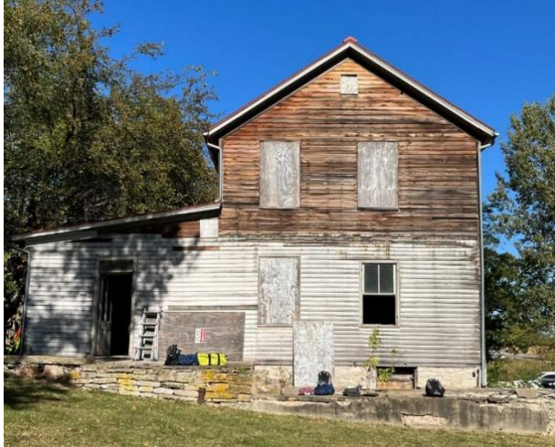
Photo 80. South wall showing whitewashed older siding at first floor and later aged replacement siding at second floor.
