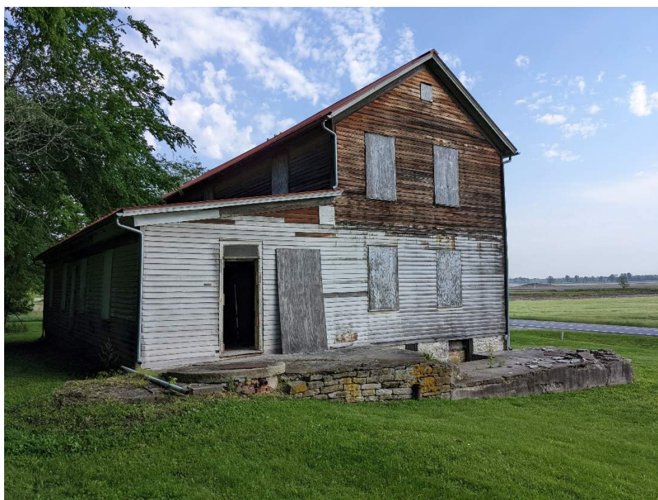
Photo 2. South (side) exterior wall of the Delassus-Kern House in May 2022.
