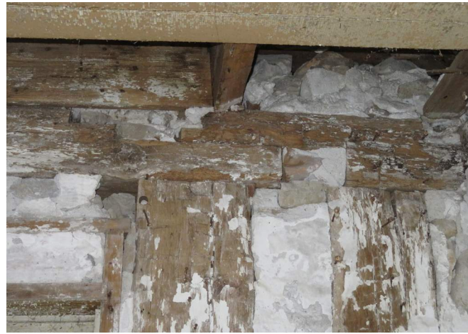
Figure 139. Open half-lap splice at top plate in Room 105. (Source: RRJ 2023)
