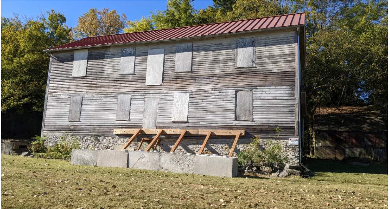
Figure 40. October 2022, after installation of the first floor bracing. (Source: RRJ 2022)
