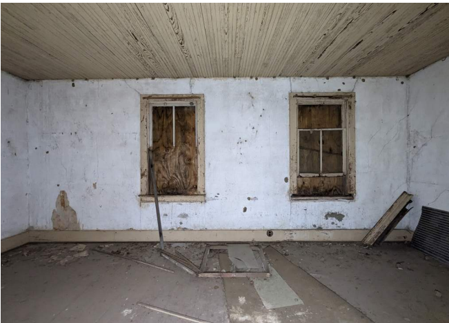
Figure 49. Room 201, looking south. (Source: RRJ 2023)
