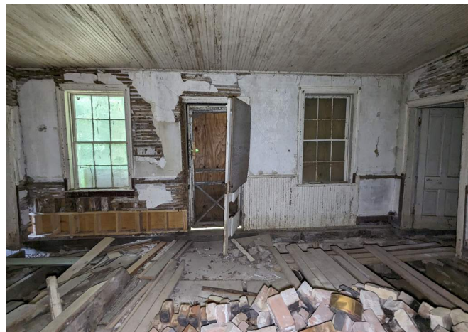
Figure 163. Room 102, looking west at the back door. (Source: RRJ 2023)
