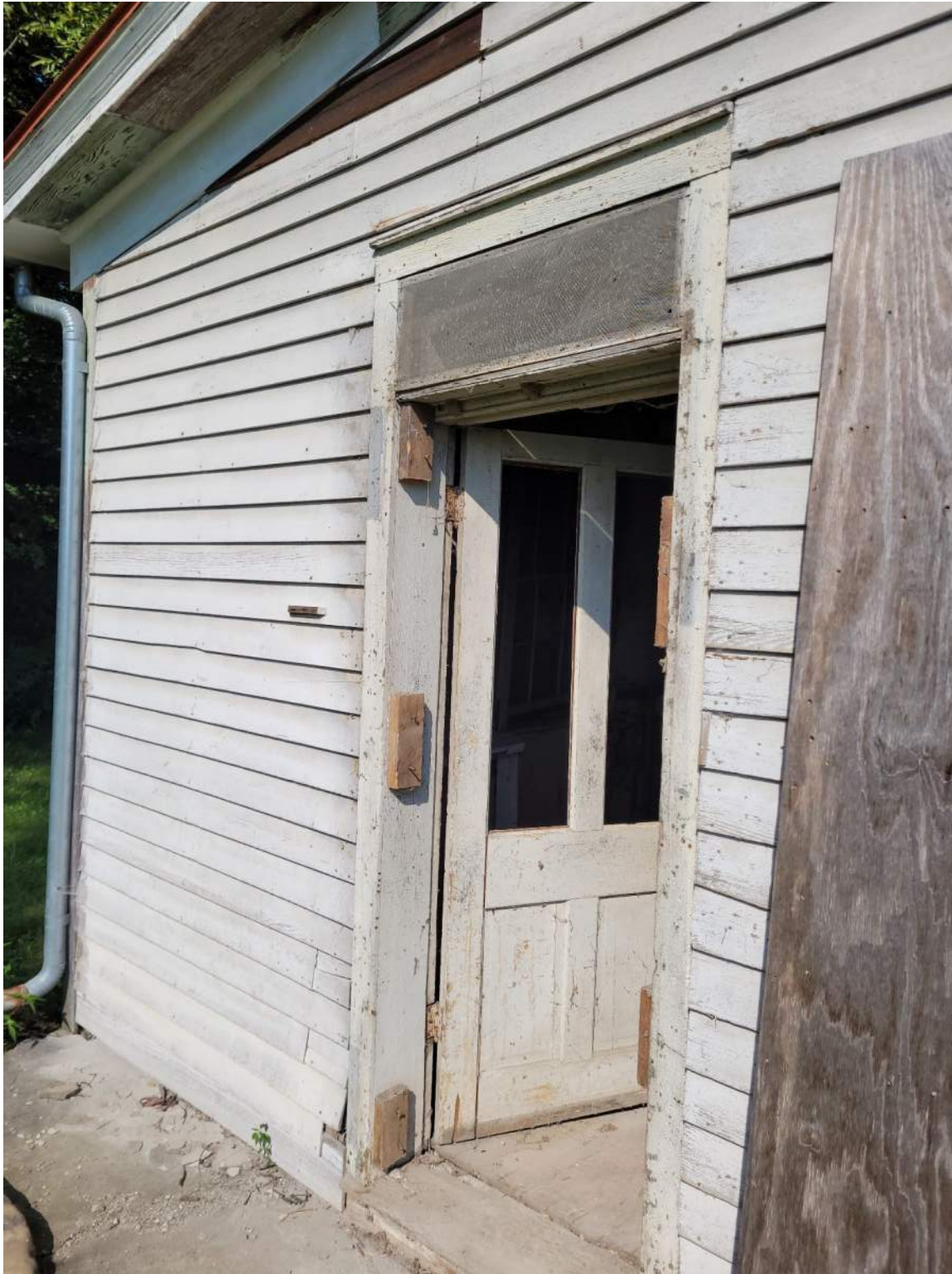
Photograph 2: Facing toward the south exterior (LBP lap siding, door, door frame and transom).
