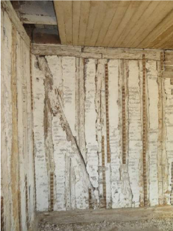
Photo 20. Typical interior vertical log wall with diagonal member within room 106.
