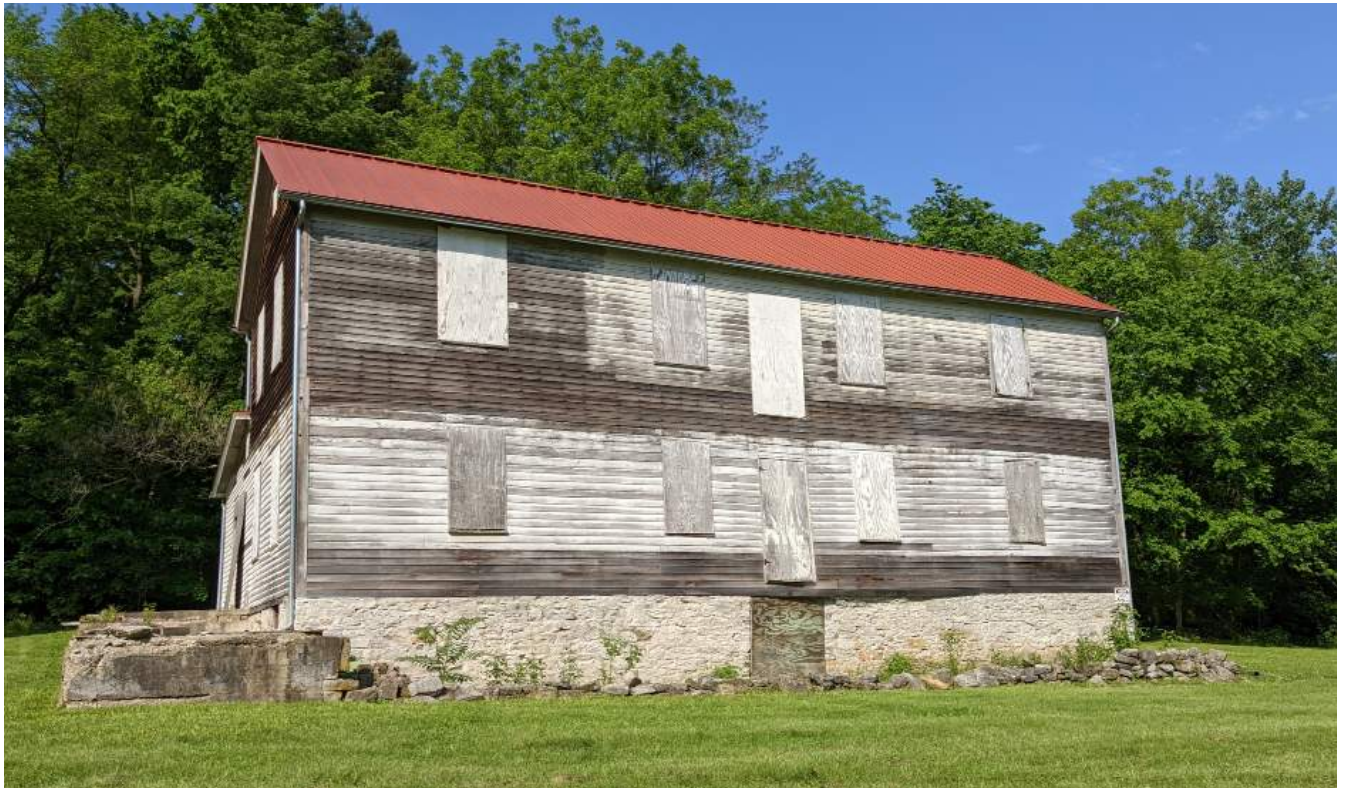
Figure 37. May 2022, view of the east exterior wall. (Source: RRJ 2022)
