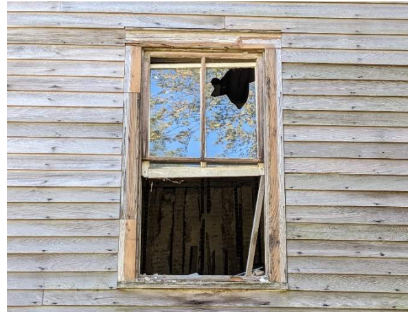
Photo 82. Window 104A on north wall, showing typical 2-over-2 windows installed after the second floor was added.
