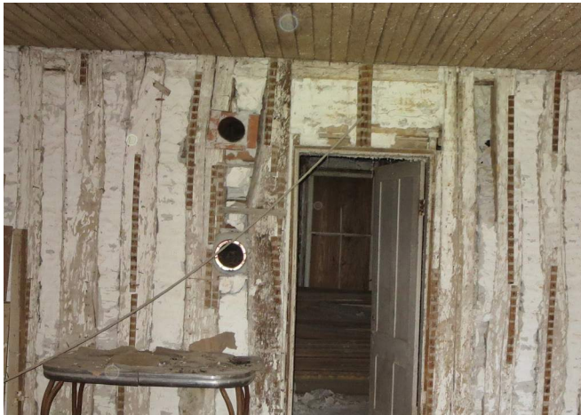
Figure 218. Existing round openings in the north wall of Room 105 indicate where wood stoves were connected to the chimney in the room to the north. (Source: Alvine 2023)
