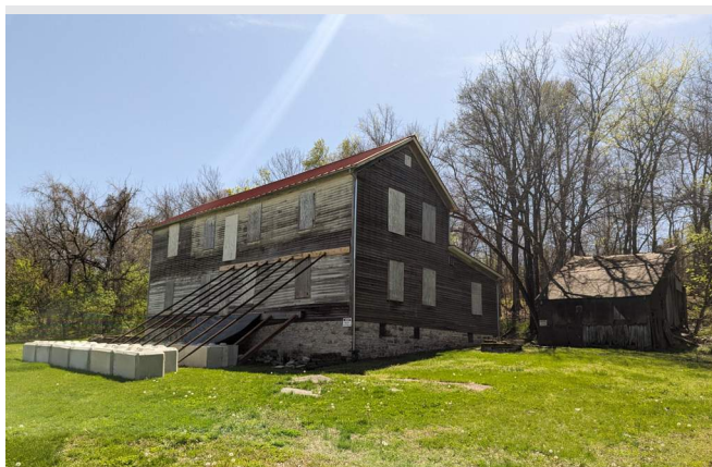
Figure 132. Exterior bracing at east wall. (Source: RRJ 2024)
