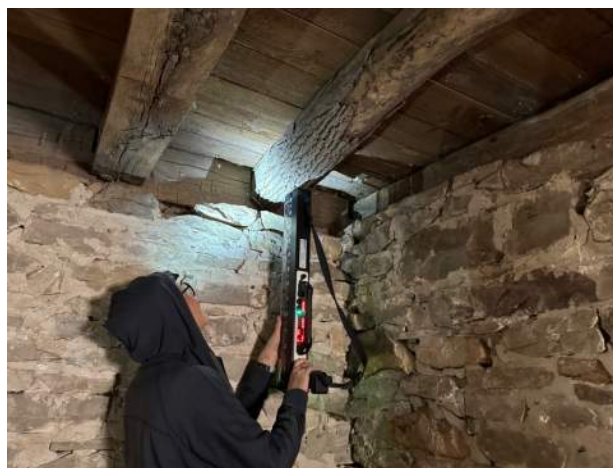
Figure 4. Use of a resistance drill to investigate the internal wood condition in a floor beam.
