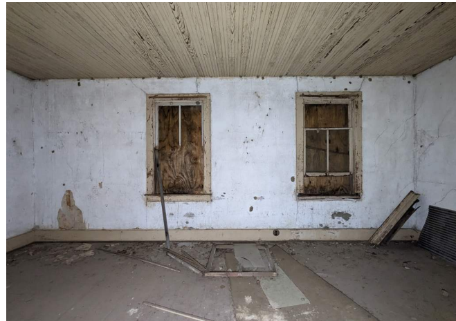
Figure 185. Room 201, looking south, showing remnants of wallpaper in the lower left corner. (Source: RRJ 2023)
