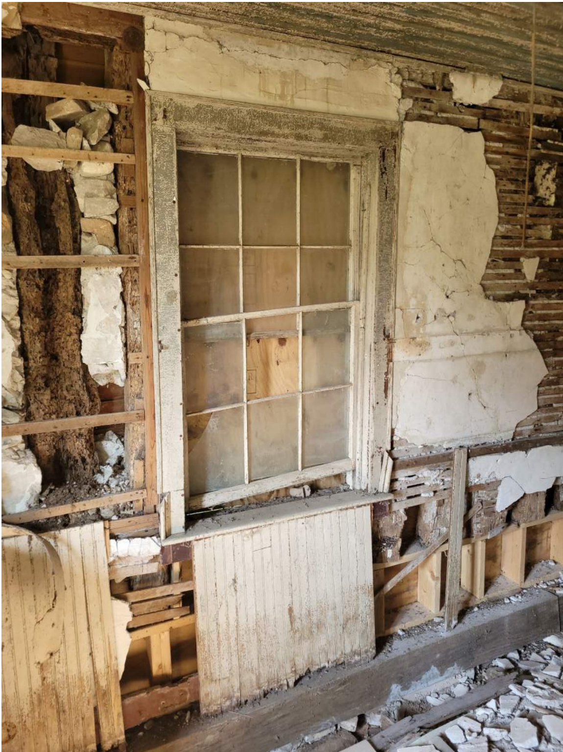
Photograph 4: LBP window and window frame Room 101.
