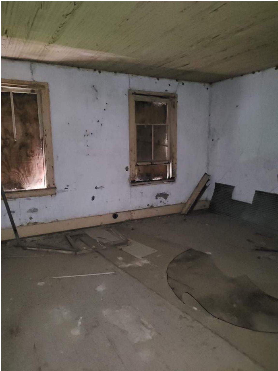
Photograph 15: LBP baseboard, window, and window frame Room 201.
