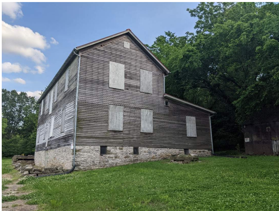
Photo 3. North (side) exterior wall of the Delassus-Kern House in May 2022.
