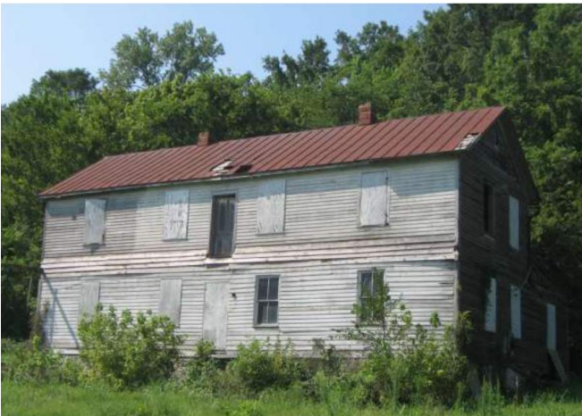
Figure 220. Photograph of Kern house c. 2011 when the chimneys existed at the roof (Source: Alvine 2023)
