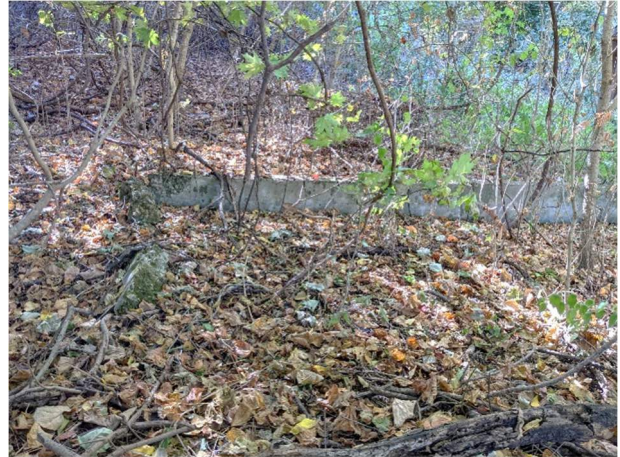
Photo 74. Remaining foundation of former chicken house.
