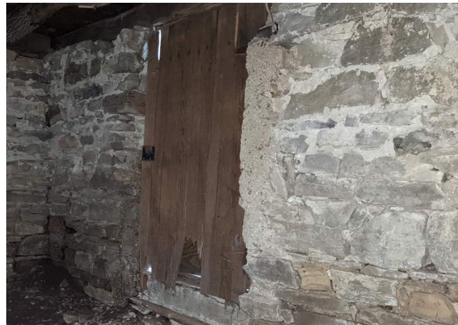
Figure 99. D001B, a batten style door. (Source: RRJ 2023)
