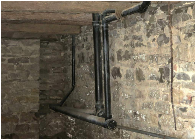
Figure 215. Existing 4-inch sanitary piping located at the west wall of the Basement routing south through the south Basement wall. (Source: Alvine 2023)
