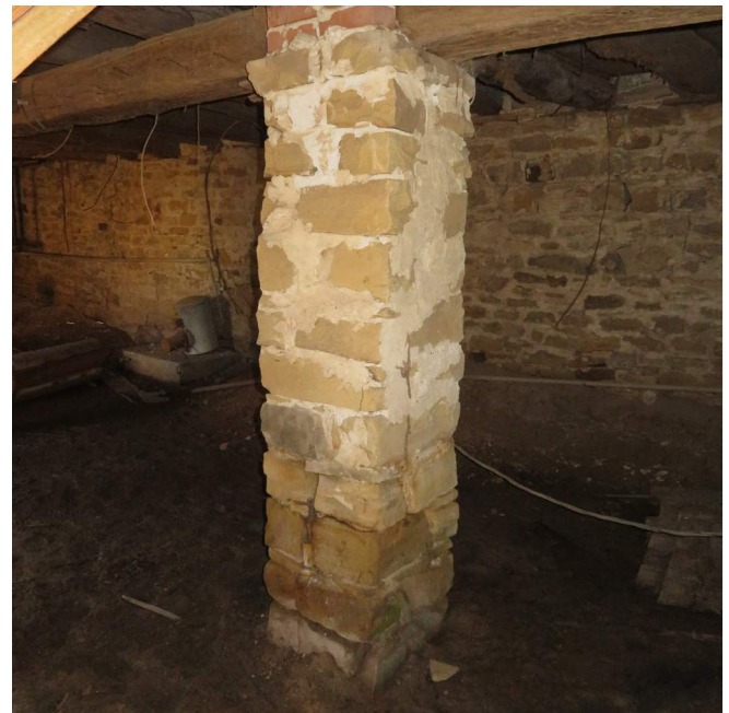
Figure 127. Stone masonry pier supporting the wood floor girders (Source: RRJ 2023)
