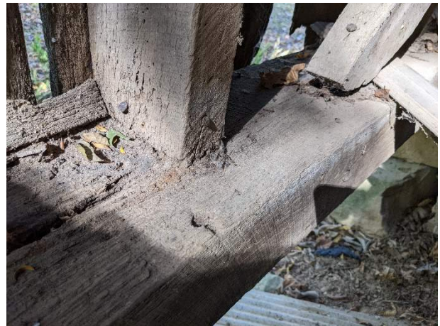
Photo 69. Detail of sill framing at the Wood shed.
