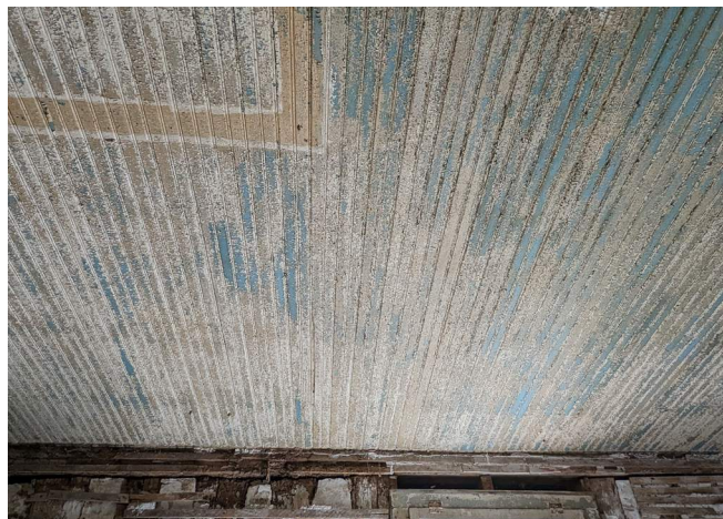
Figure 162. Ceiling beadboard in Room 101. (Source: RRJ 2023)
