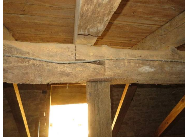
Photo 46. Splice within girder at center of full-height basement.
