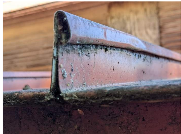
Photo 78. Standing seam of sheet metal roof.
