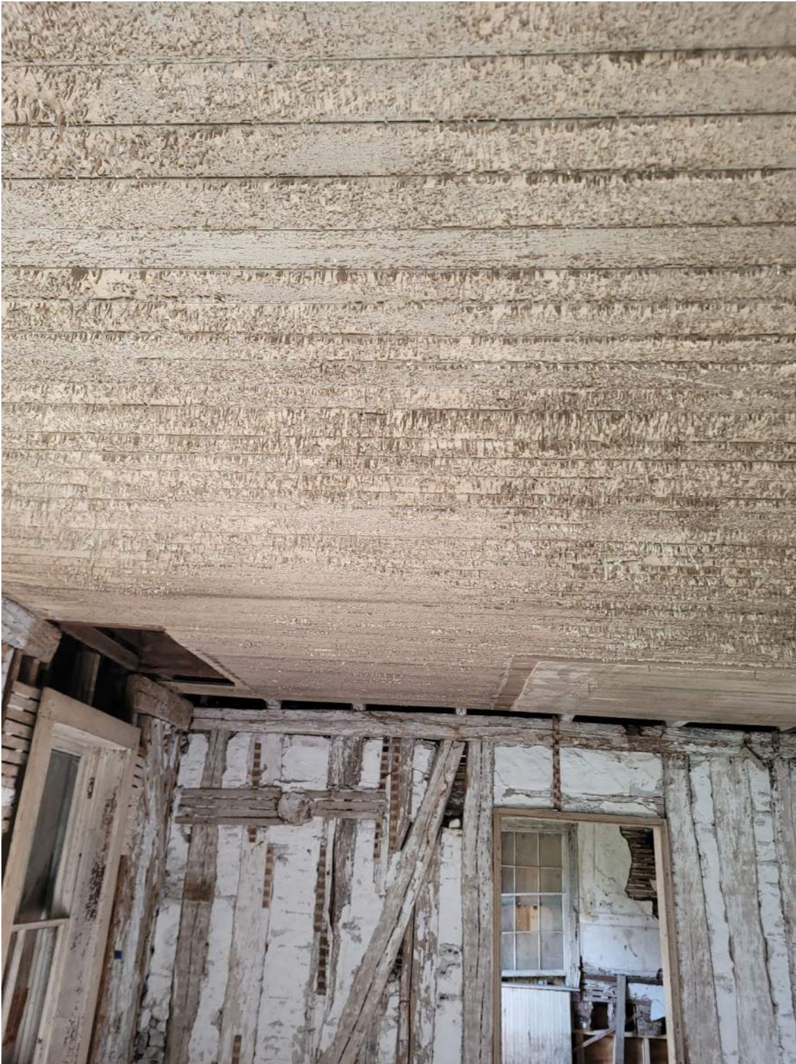
Photograph 7: LBP ceiling, window, window frame, and door frame Room 104.
