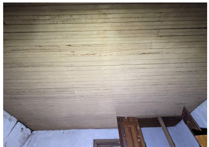
Figure 206. Beadboard ceiling in Room 204, looking east. (Source: RRJ 2023)
