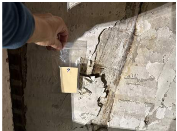
Figure 10. Sample 9. Diagonal brace, Room 4. White oak.
