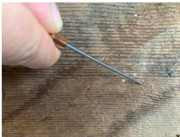
Figure 2. Probing of the wood using an awl.
