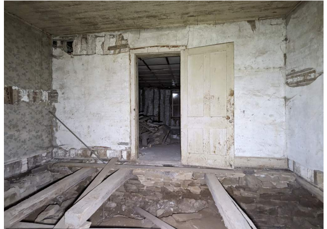
Figure 169. Room 103, looking east. (Source: RRJ 2023)
