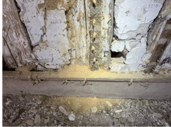
Figure 28. Lightly colored powderpost beetle frass from the interior wall logs.
