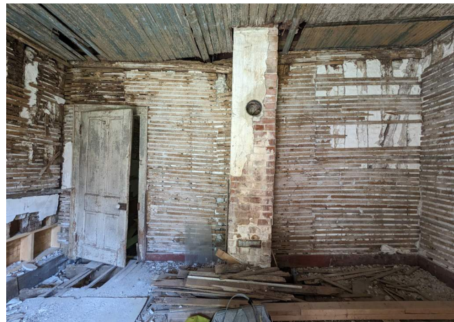
Figure 158. Room 101, looking north. (Source: RRJ 2023)
