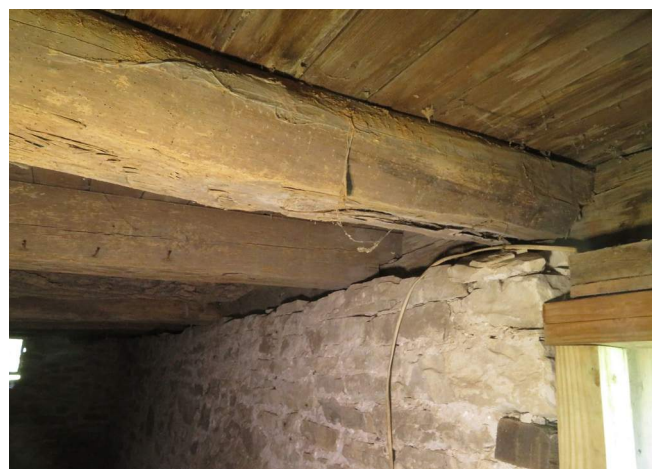
Figure 141. Floor joist bearing on the east foundation wall. (Source: RRJ 2023)
