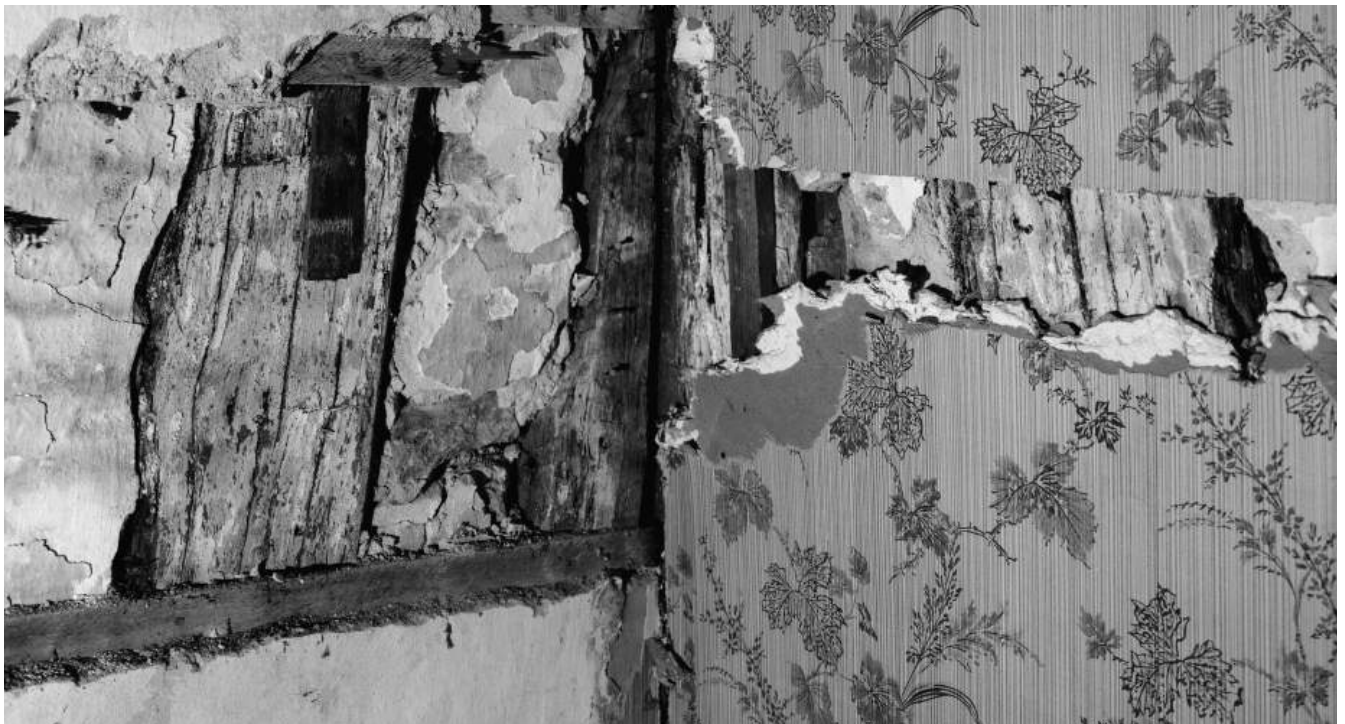
Figure 25. 1985 photograph of the northwest corner of Room 103, showing the vertical logs and pierrotage behind the plaster.. (Source: HABS)
