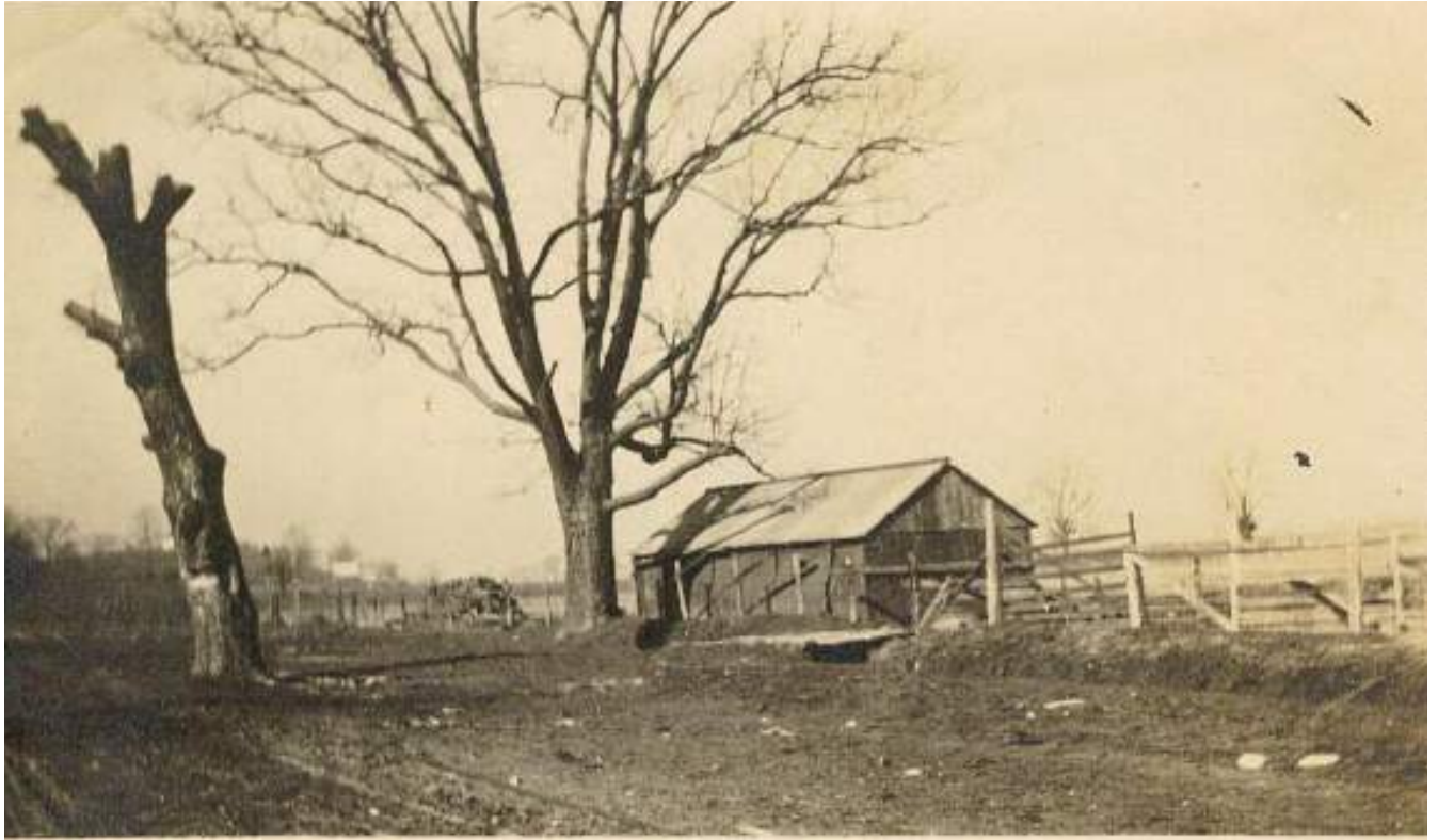
Figure 13. Undated photograph of the property (possibly 1920s), showing a small barn on the east side of the road. This photograph may date to before the 1920s improvements New Bourbon Road (now US-61). (Source: MoDNR Felix Vallé House archives.)
