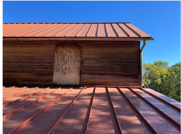
Photo 77. First and second story roofs at West wall.
