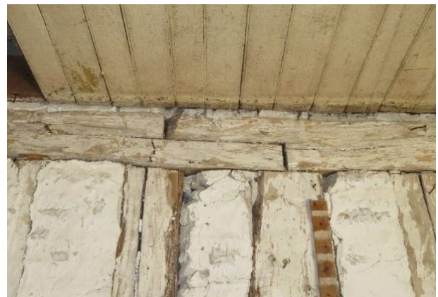
Photo 26. Typical top plate wall splice within north wall of room 106. Splices were observed to have one 1-inch wood trenail pinning the splice in place.
