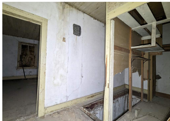
Figure 192. Room 202, looking southwest, showing the closet framing to the right and the stairwell. (Source: RRJ 2023)
