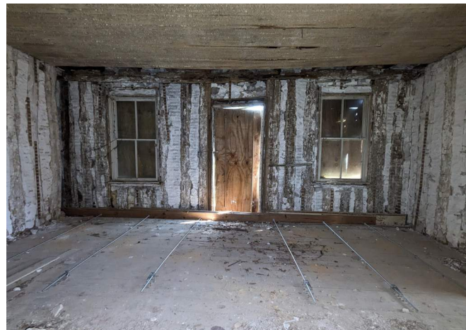
Figure 176. Room 105, looking east, showing the floor bracing that was installed before the 2023 shoring. (Source: RRJ 2023)
