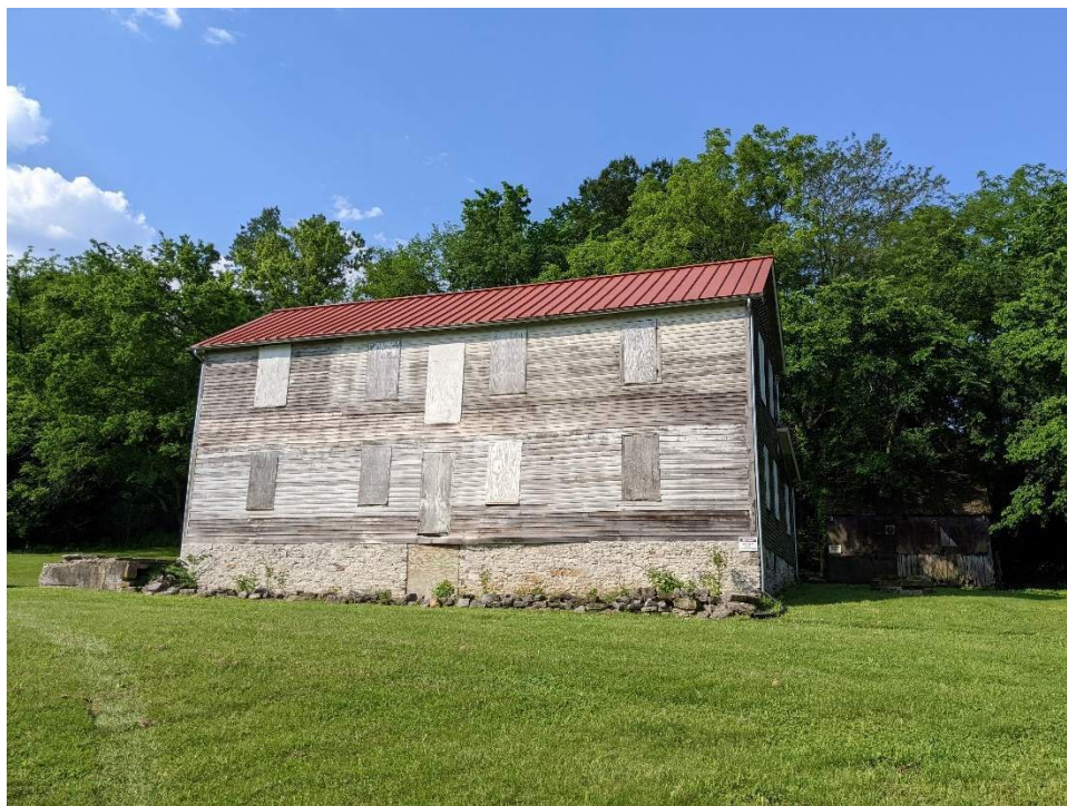
Photo 1. East (main) facade of the Delassus-Kern House in May 2022.
