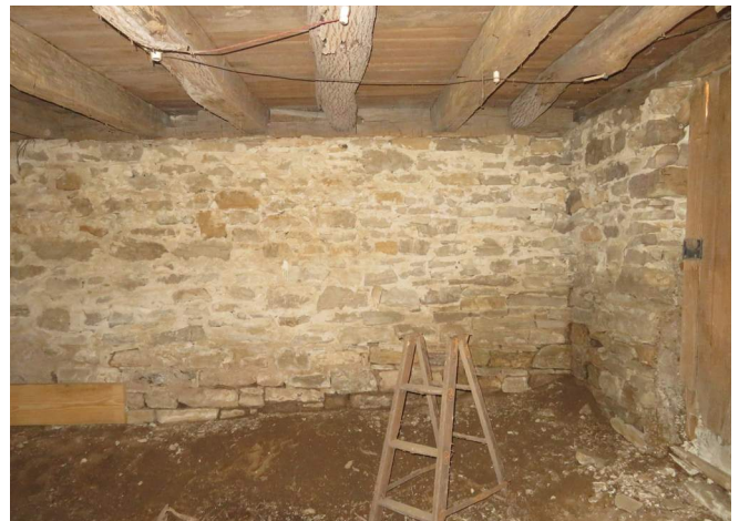
Figure 148. Basement interior, looking east. (Source: RRJ 2023)
