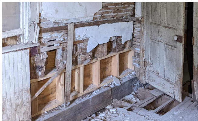
Figure 133. Stud wall construction at the west wall in Room 101. (Source: RRJ 2023)
