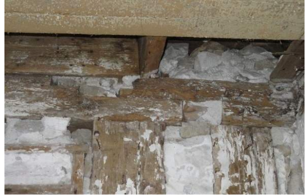
Photo 21. East wall top plate splice within room 105. The splice appears to have been constructed in this "open" position, with pierrotage infill placed between members.
