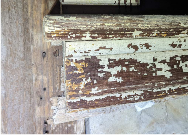
Figure 112. Apron of W104A. (Source: RRJ 2023)
