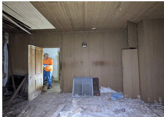
Figure 197. Room 203, looking south at the beadboard wall panels. (Source: RRJ 2023)
