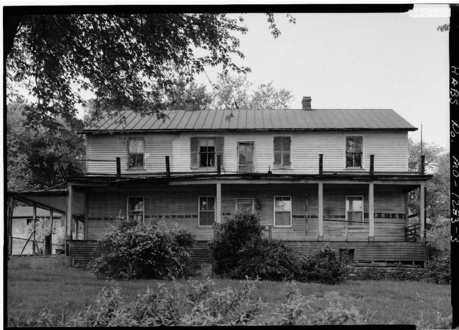
Photo 11. East facade of the house in 1985 (HABS).
