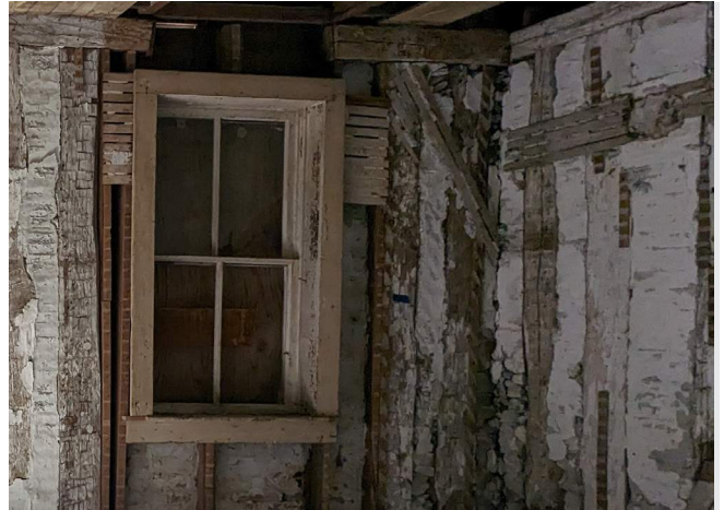
Figure 182. Diagonal lath applied directly to the logs in the southwest corner of Room 106. (Source: RRJ 2023)
