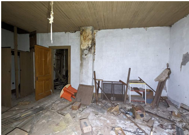
Figure 50. Room 204, looking south. (Source: RRJ 2023)
