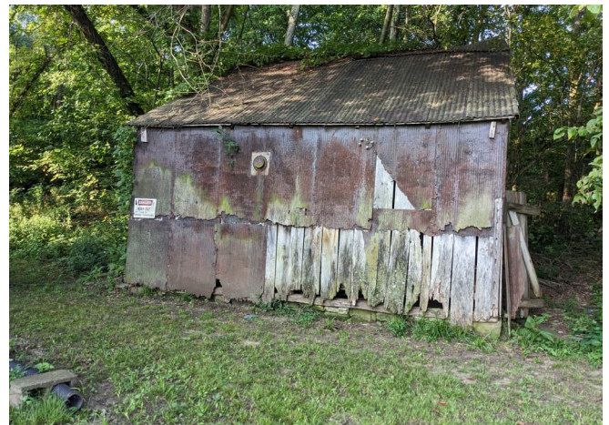
Figure 69. View west toward the wood shed. (Source: LSH-LA, 2023)
