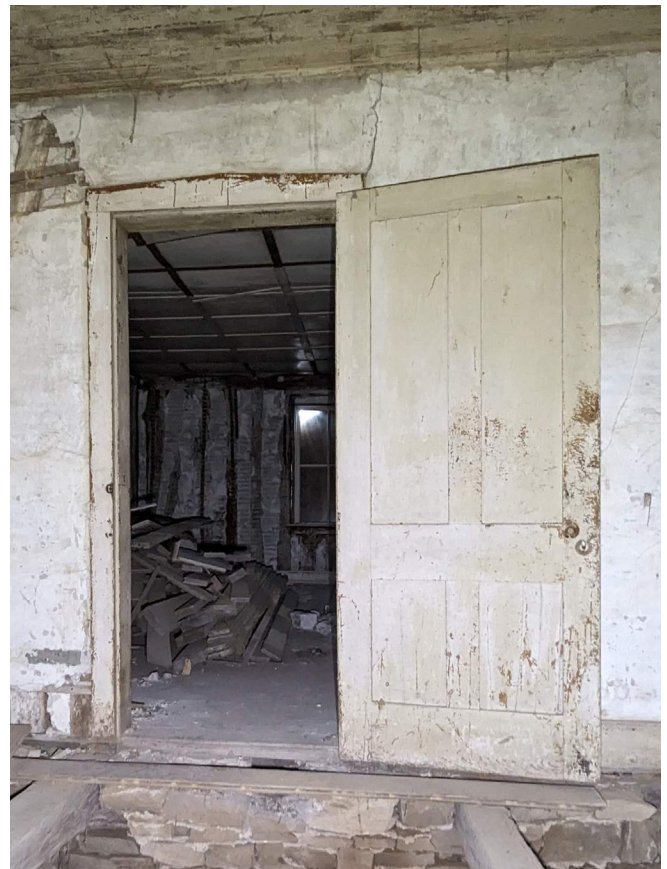
Figure 151. Door 103B, looking east, showing the pedimented casing. (Source: RRJ 2023)
