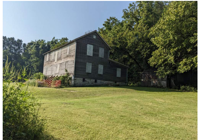
Figure 84. View south toward the house with the graded landform of the driveway visible. (Source: LSHLA 2023)
