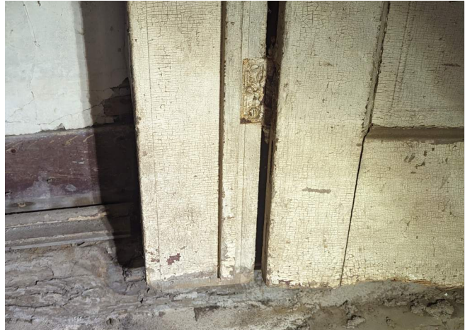
Figure 152. Jamb trim at D103A. (Source: RRJ 2023)
