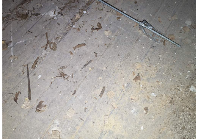
Figure 178. Typical hardwood floor boards in Room 105. (Source: RRJ 2023)
