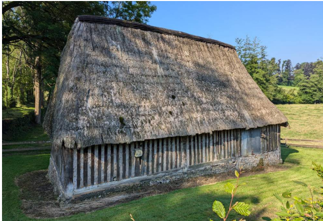
Figure 35. 17th century barn near Livet-sur-Authou, Normandy, France showing close-stud pan-de-bois construction technique that was the architectural antecedent to poteaux-sur-sole. (Source: Lurita McIntosh Blank, 2024)
