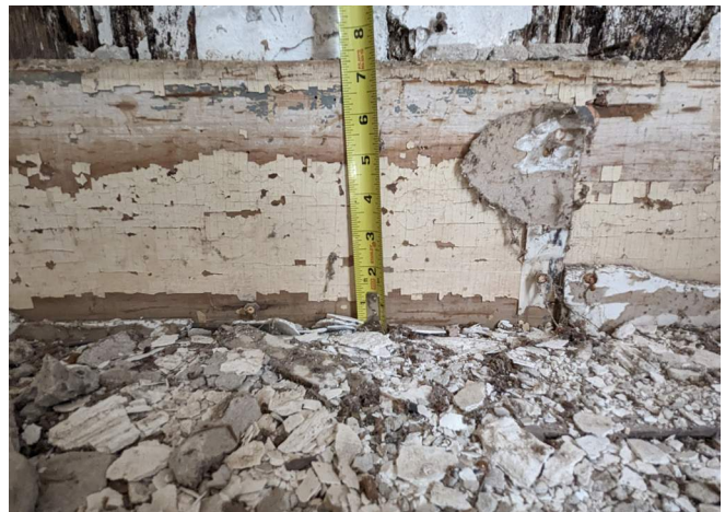
Figure 183. Baseboards in Room 106. (Source: RRJ 2023)
