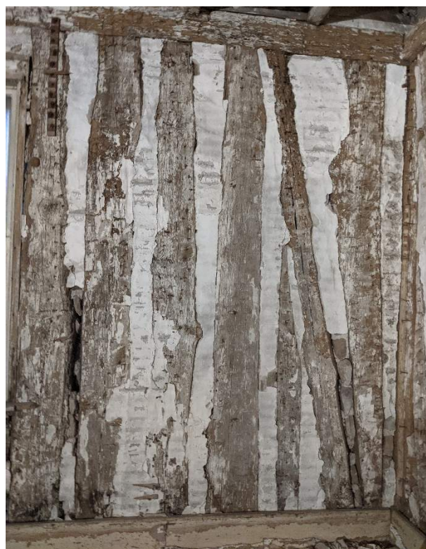
Photo 7. Exposed poteaux-sur-sole structure at the interior.
