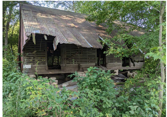
Figure 54. An outbuilding located north of the house that served as a corn crib. (Source: LSHLA, 2023)
