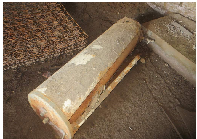
Figure 214. Photo of existing abandoned water heater lying on dirt floor next to concrete pad. The water heater may have located on the concrete pad at one time. (Source: Alvine 2023)
