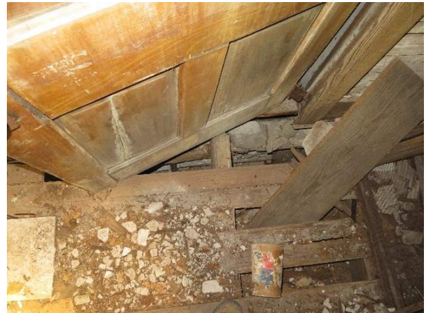
Photo 49. Second floor joists viewed from second floor at east wall.
