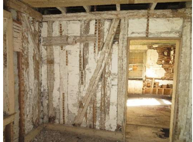
Photo 48. Second floor joists viewed from first floor at north-south interior wall within room 106.
