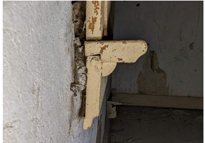
Figure 115. Profile of the stool and apron at W201B. (Source: RRJ 2023)
