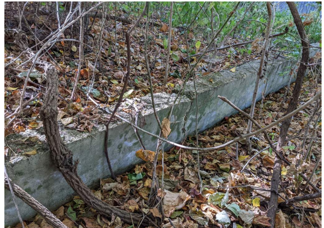
Figure 76. Ruins of the chicken house foundation. (Source: RRJ 2023)
