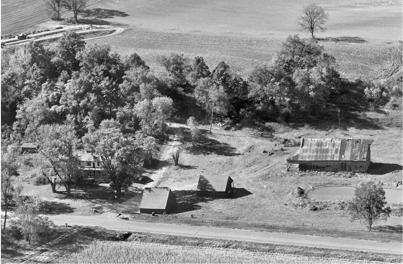
Figure 23. Aerial photograph from 1976, looking west, showing the large barn in very poor condition and a livestock pond that was not present in 1968. (Source: Vintage Aerial, Photo 4-FSTG-22, vintageaerial.com/photos/missouri/ste-genevieve/1976/FSTG/4 )
