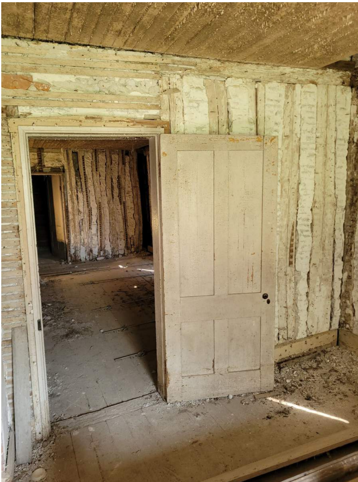
Photograph 8: LBP ceiling, baseboard, door, and door frame Room 104.
