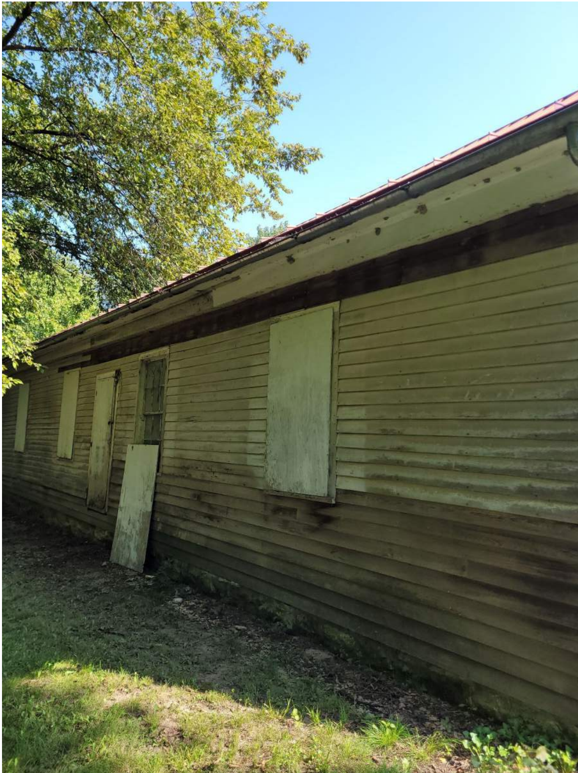
Photograph 3: Facing toward the west exterior (LBP lap siding, window, and window frame).
