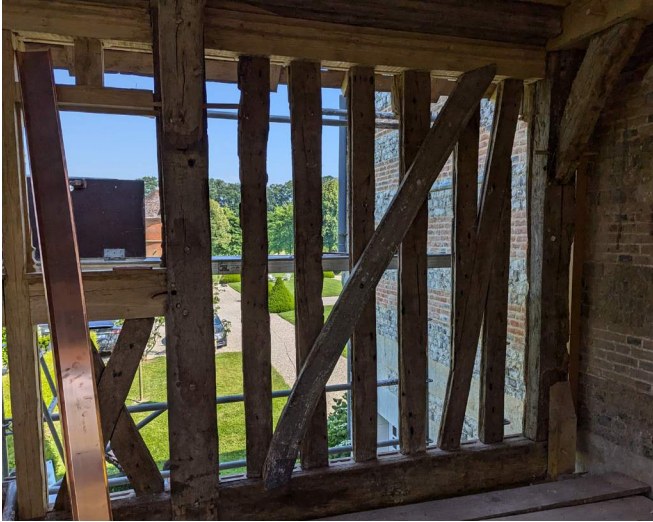
Figure 36. 18th century pan-de-bois structure under restoration in Terres-de-Caux, Normandy, France. Note the steeply pitched brace or décharge on the right. The brace set at a 45-degree angle was added at a later date. (Source: Lurita McIntosh Blank, 2024.)
