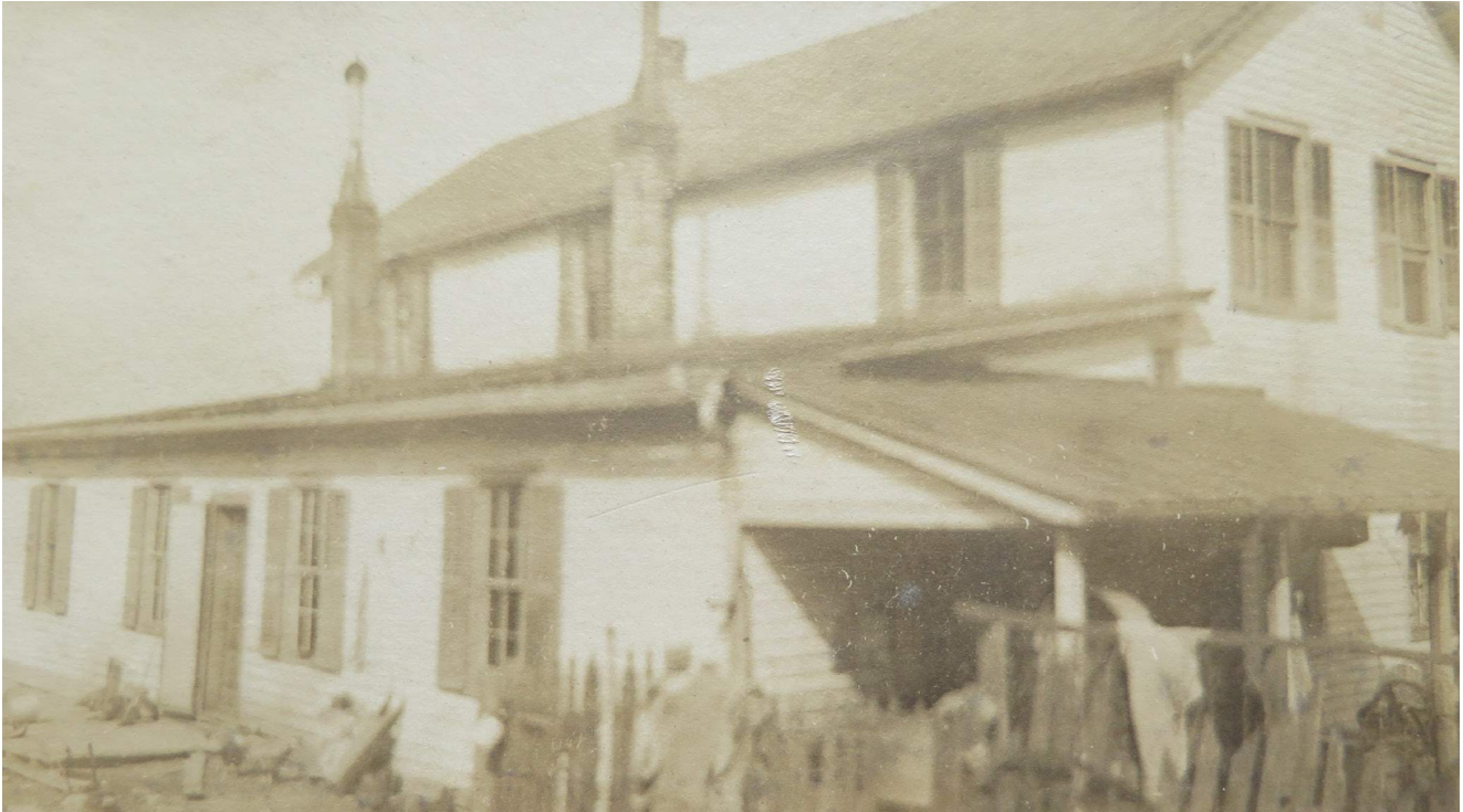
Figure 17. Undated (possibly 1910s) photograph of the rear west side of the house, showing the shed roof over the kitchen door and the new brick masonry chimneys. (Source: MoDNR Felix Vallé House archives.)
