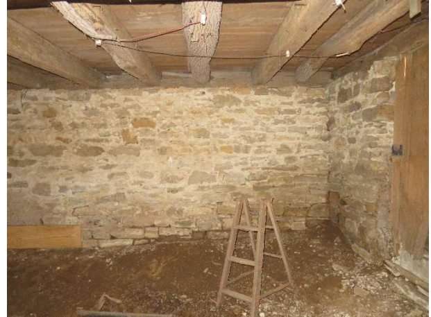
Photo 41. Overview of timber joists supporting the first wall, notched into the bottom plate of the east wall. The east wall at its south end is pictured.
