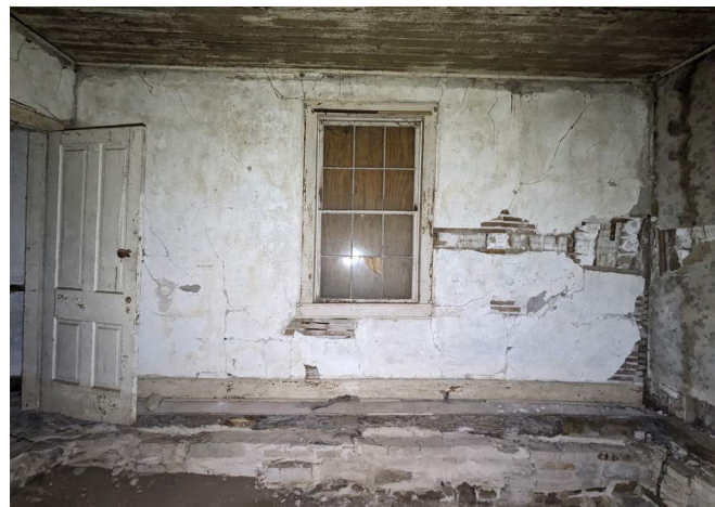
Figure 168. Room 103, looking west. (Source: RRJ 2023)
