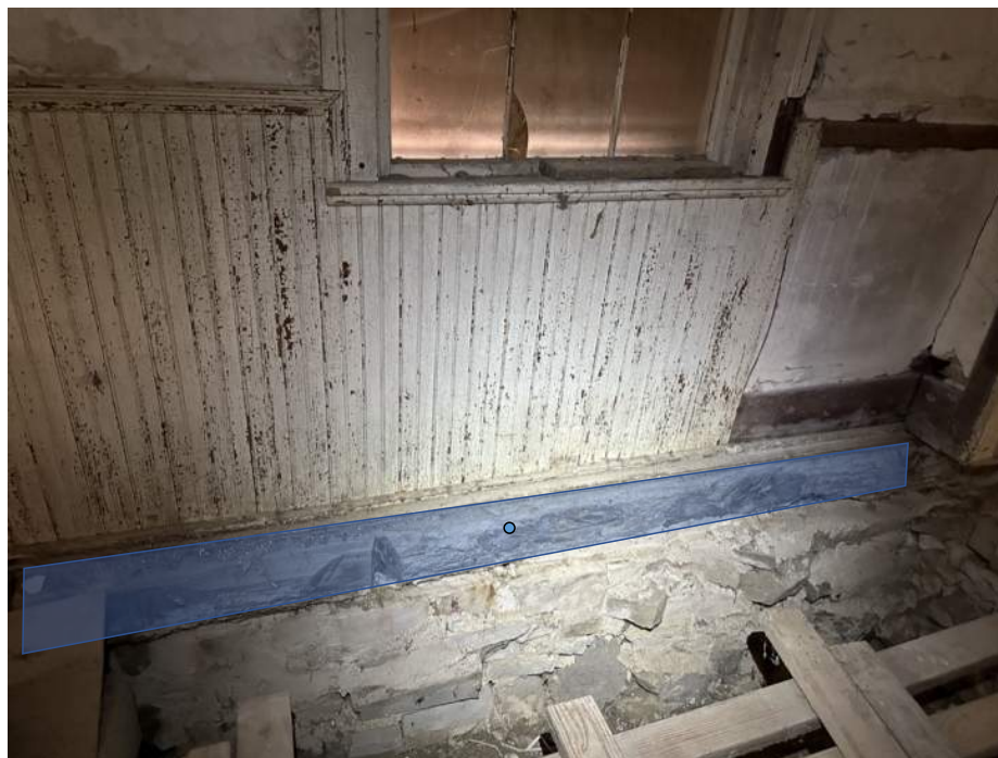
Figure 18. North section of the west wall. Room II.
