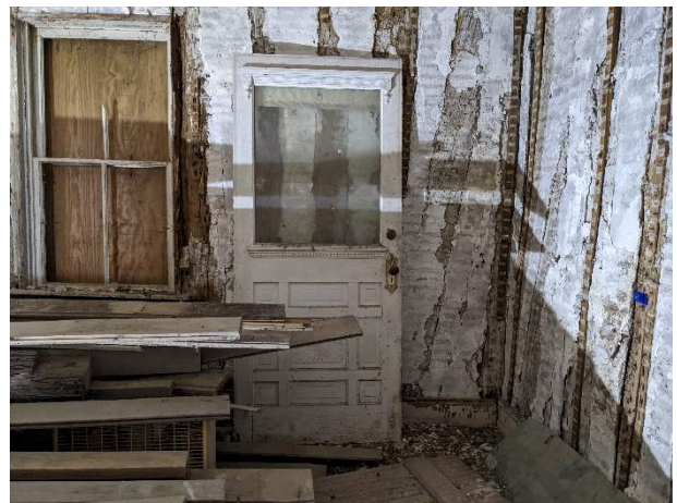
Photo 88. Exterior door stored in Room 106, similar to Door 101A but in better condition. Possibly the door from Room 104.
