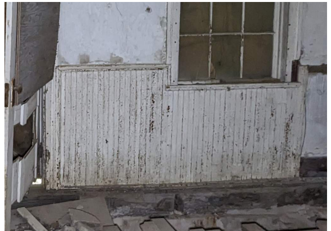
Figure 166. Remnants of beadboard wainscoting on the west wall. (Source: RRJ 2023)
