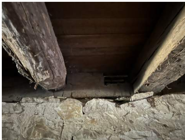
Figure 10. Opening in the sill beam cut out to accommodate the beam replacement. Round log on the left appears original to the building.
