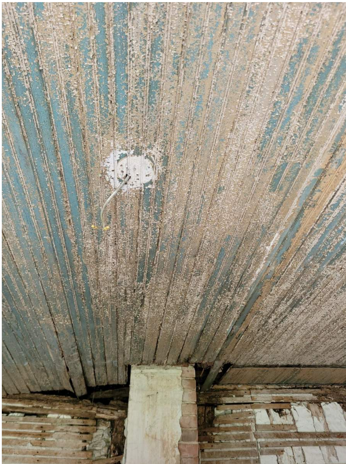
Photograph 6: LBP ceiling Room 101.
