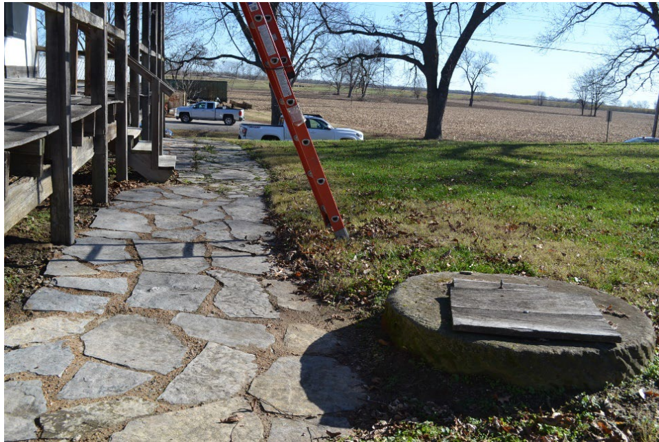
FIGURE 204. The south walkway extends along the south façade of the house. (Source: LSHLA, October 2020)
