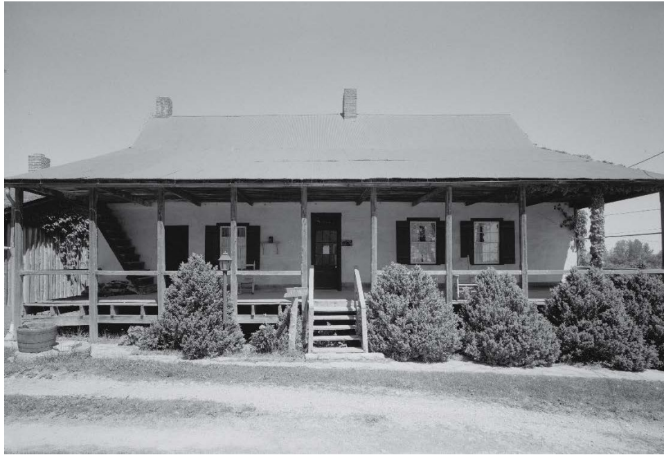
FIGURE 219. A HABS photograph from 1986 shows the south façade of the house including the driveway, wood stairs, boxwood plantings, stone walk and well/cistern with a wooden bucket. (Source: Source: HABS Survey No. MO-1113, Library of Congress)
