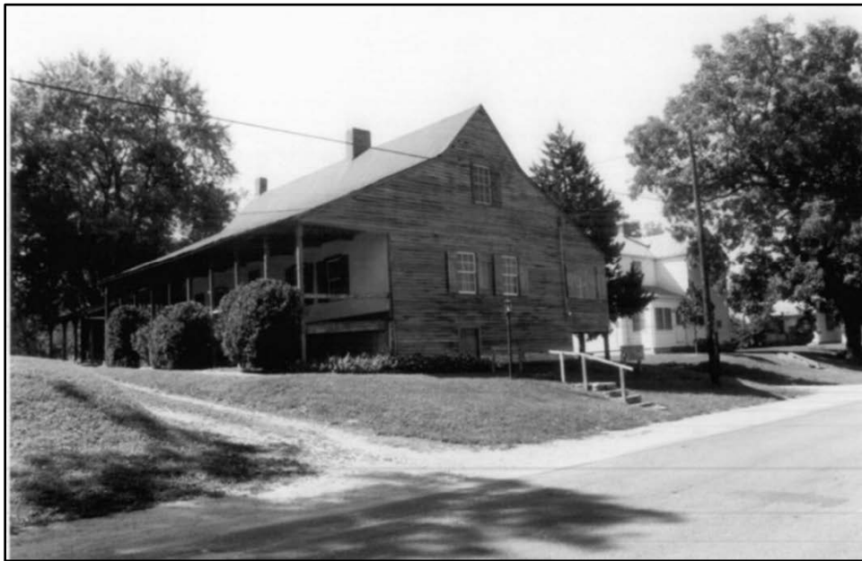
FIGURE 212. View to the House from St. Marys Road, 1986. (Source: HABS Survey No. MO-1113, Library of Congress)
