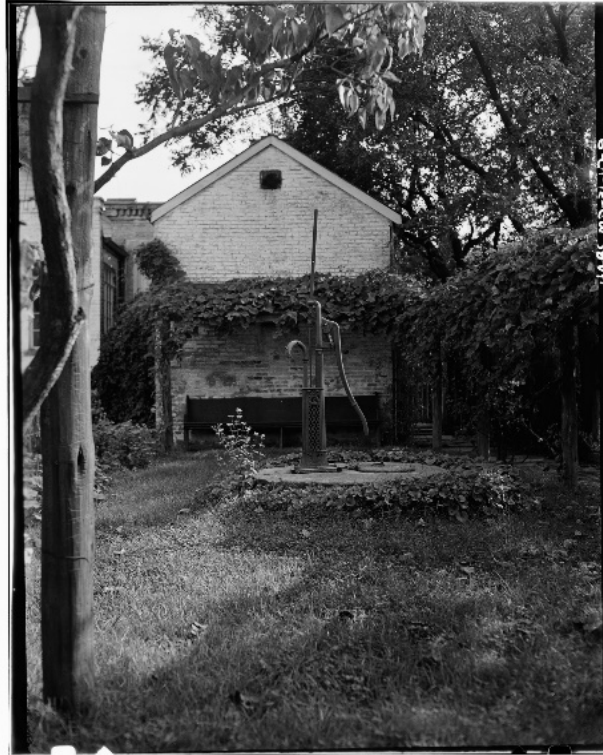
FIGURE 152. View of the grape arbor at the northwest corner of the house, with the well and pump in front, 1935. (Source: HABS MO 31-10, Library of Congress)
