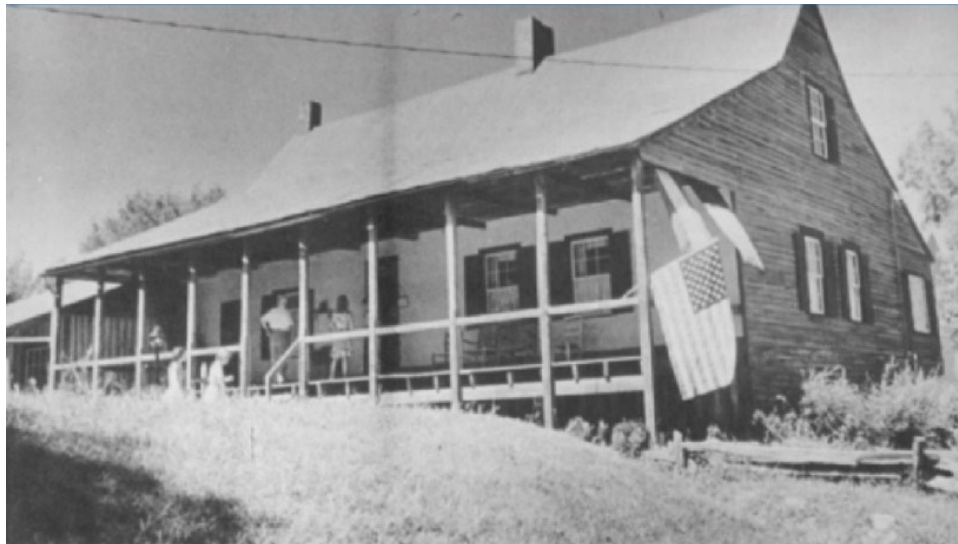
FIGURE 70. View northwest toward the Bauvais-Amoureux House circa 1970s that includes the gift shop that operated from the 1960s into the 1990s, as well as a driveway following the south façade of the house. Wood stairs lead to the porch, while a low fence and plantings appear to edge the house to the east. The house has two chimneys. (Source: HABS Survey No. MO-1113, Library of Congress)
