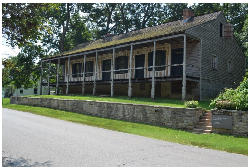
FIGURE 3. The Janis-Ziegler House (Green Tree Tavern), located along St. Marys Road.
