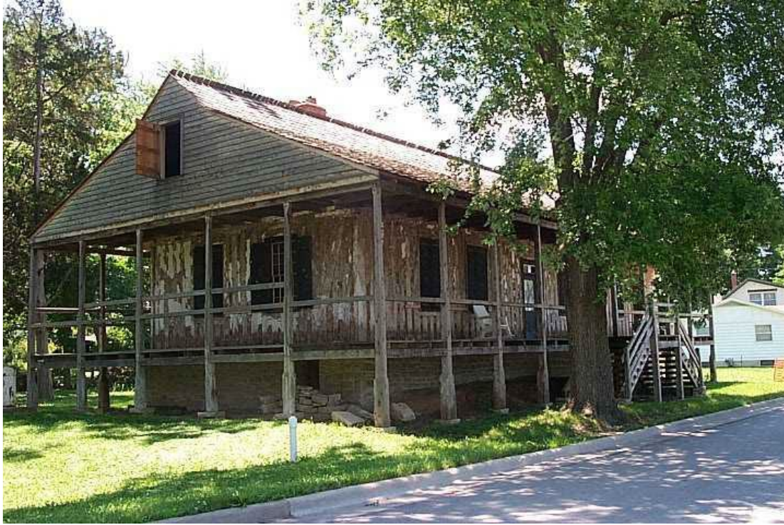
FIGURE 184. View toward the Janis-Ziegler House in 2004 across St. Marys Road after the corridor had been elevated to the top of the stone retaining wall and curb and gutter added after the 1993 flood. (Source: R. Mueller, 2004)
