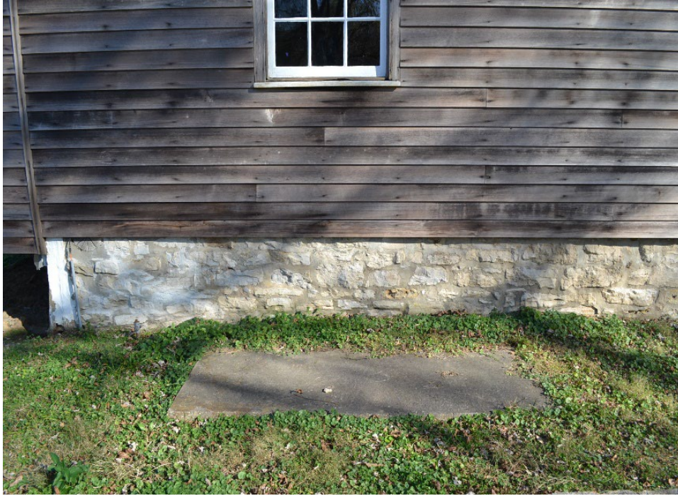
FIGURE 223. The concrete pad is likely associated with the construction of the gift shop west of the house during the period of Donze ownership. (Source: LSHLA, October 2020)
