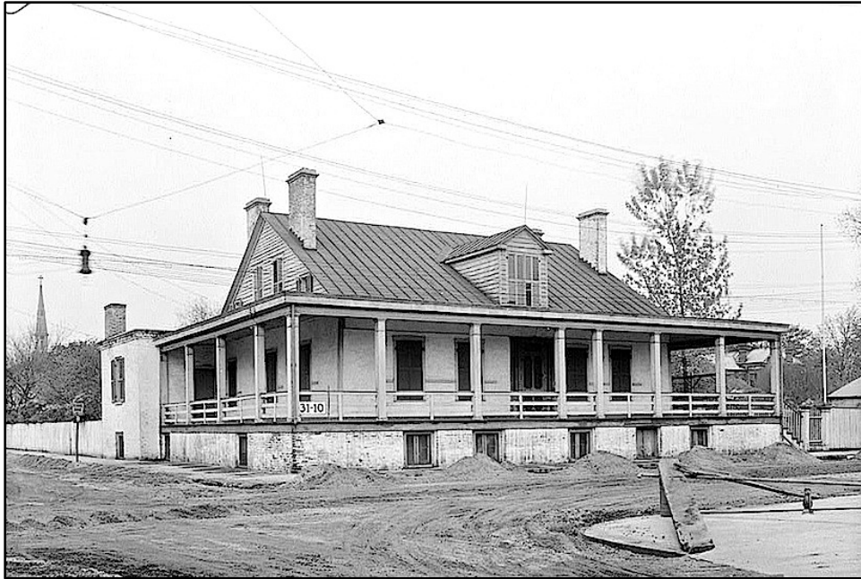
FIGURE 148. View looking west over newly constructed sidewalks to the east façade of the house, 1935. (Source: HABS MO 31-10, Library of Congress)
