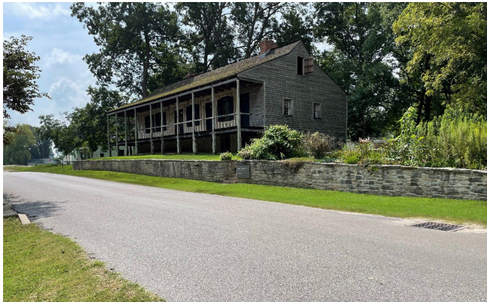
FIGURE 185. The north and east elevations of the Janis-Ziegler House. The house is sited above St. Marys Road and South Gabouri Creek.
