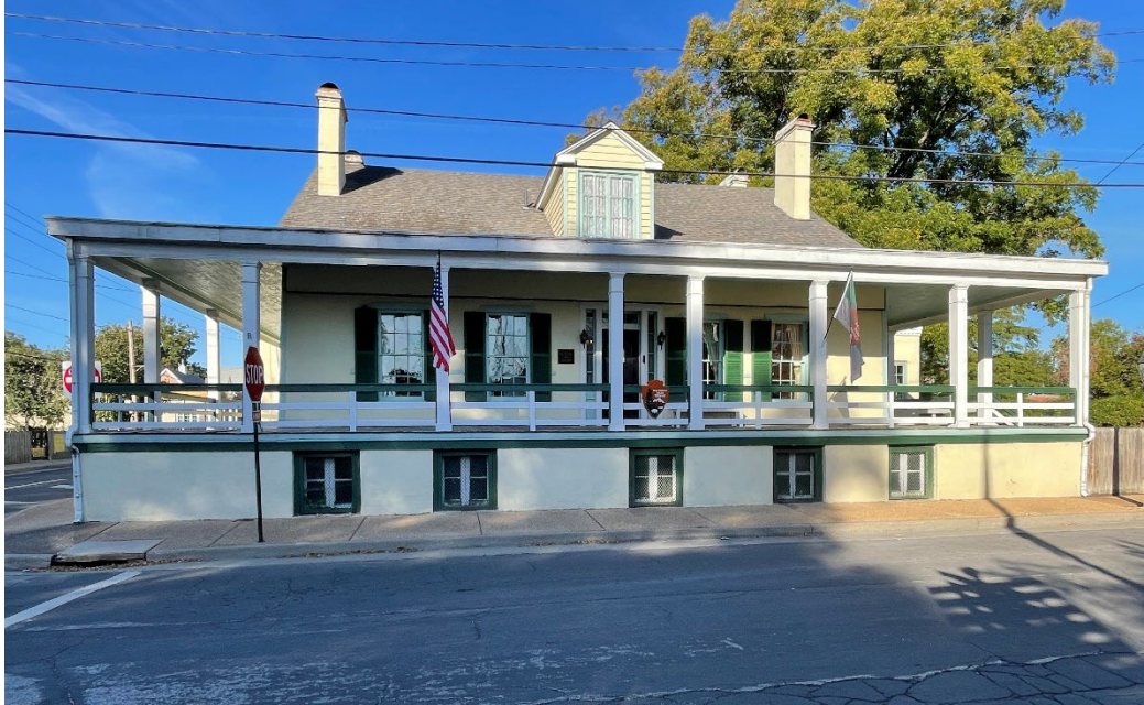
FIGURE 156. East façade of the Jean Baptiste Vallé House. (Source: LSHLA, October 2022)
