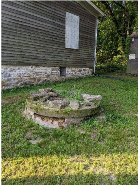
FIGURE 251. View of the cistern north of the house.
