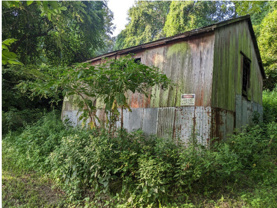
FIGURE 242. View west toward the chicken house.
