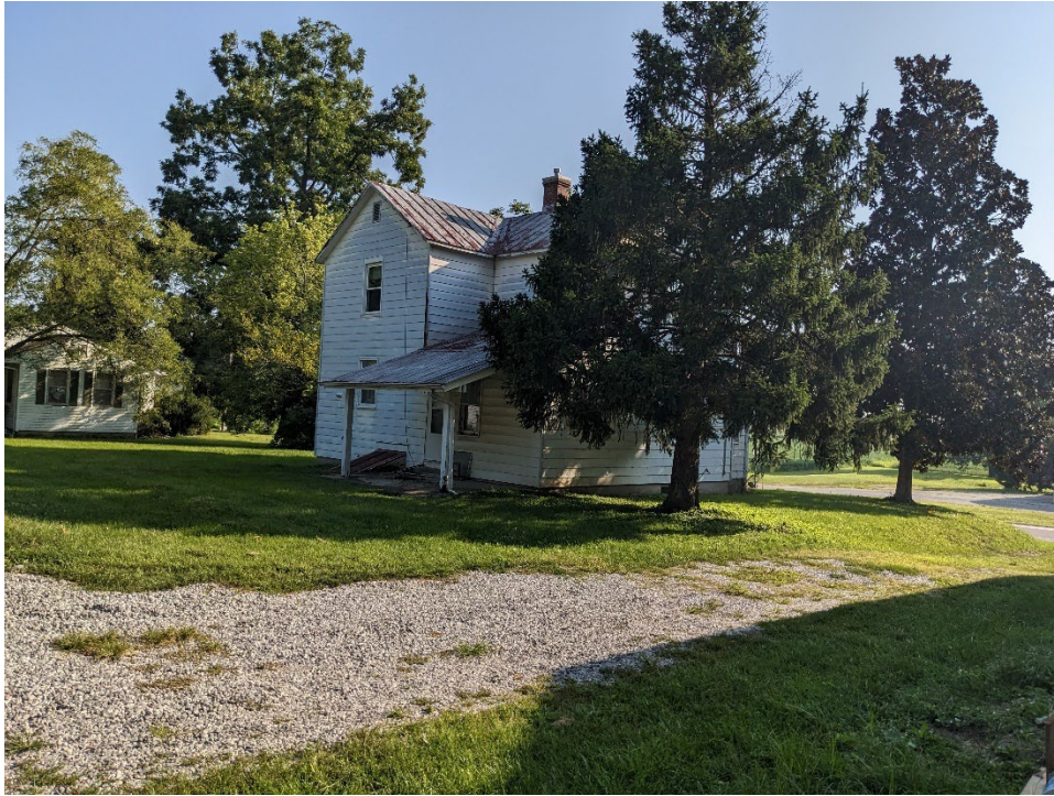
FIGURE 266. A small porch with a shed roof is attached on the west façade of the house.
