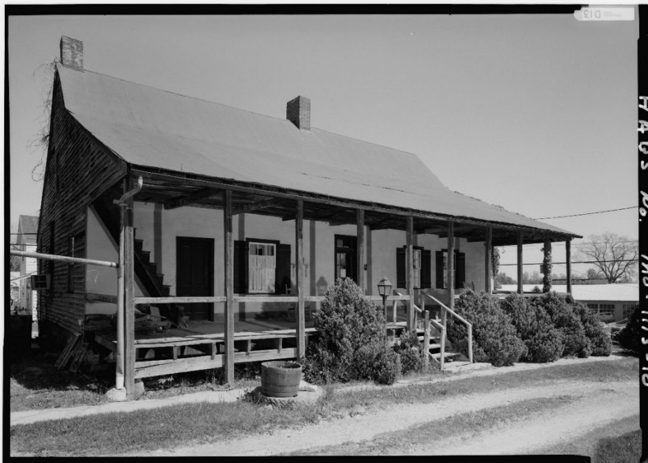
FIGURE 76. Another HABS photograph from 1986 shows the south and west façades of the house, driveway, wood stairs, boxwood plantings, stone walk, and well shown with a wooden bucket, with the boat repair shop in the background. (Source: HABS Survey No. MO-1113, Library of Congress)
