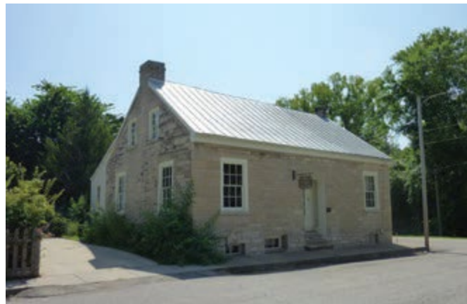
FIGURE 115. View of the Keil Stone House, an example of vernacular stone house construction. (Source: Ste. Genevieve Special Resource Study and Environmental Assessment , 2016)
