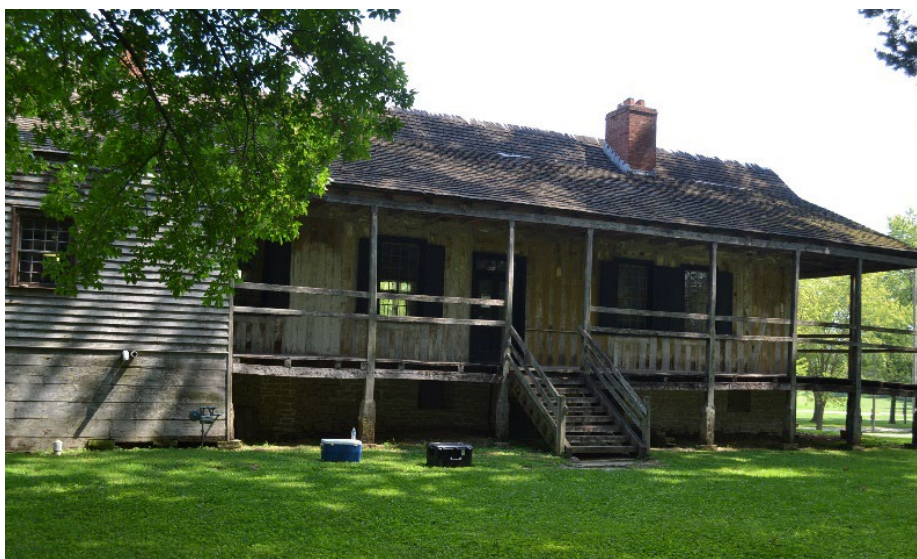
FIGURE 175. View of the wood steps leading to the gallery along the southwest façade.
