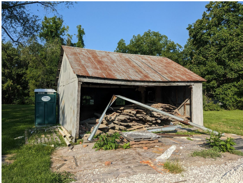
FIGURE 264. The shed behind 323 St. Marys Road used by the National Park Service for maintenance storage.
