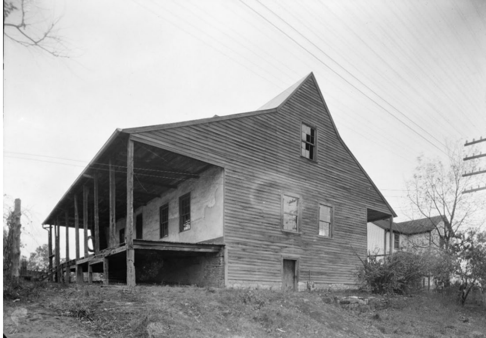
FIGURE 52. A circa 1936 photo showing the east façade and south porch of the Bauvais-Amoureux House, with an overhead electrical line along the road. A fencepost appears south of the house. A portion of the stone wall along the road remains visible, along with some shrubs and trees. A crank-handled pump and sheet metal cover are visible in association with the well or cistern inside the fence. (Source: Survey No. HABS MO-1113, Library of Congress)
