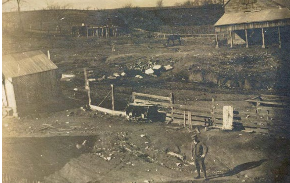
FIGURE 48. An undated photograph, circa 1910s, of the Delassus-Kern property looking northwest with the shadow of the house to the left. The outbuilding to the left is a shed, while the building to the right is a stable. Neither of these two buildings survive today. (Source: Missouri Department of Natural Resources, Felix Vallé State Historic Site archives)
