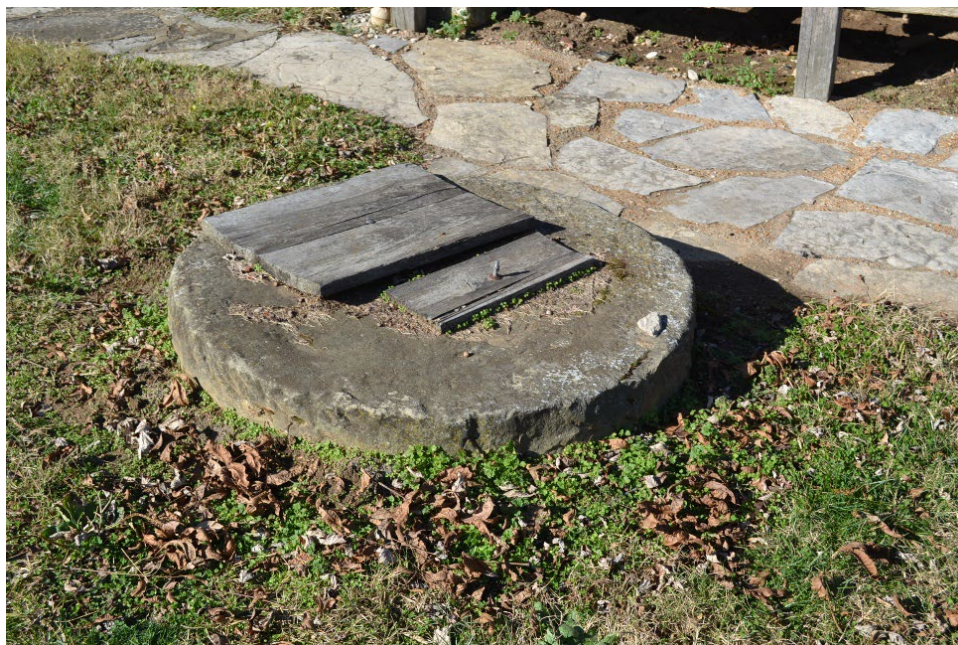
FIGURE 220. The well/cistern adjacent to the south walkway of the Bauvais-Amoureux House with a granite circular slab and wood boards attached to the top. (Source: LSHLA, October 2020)
