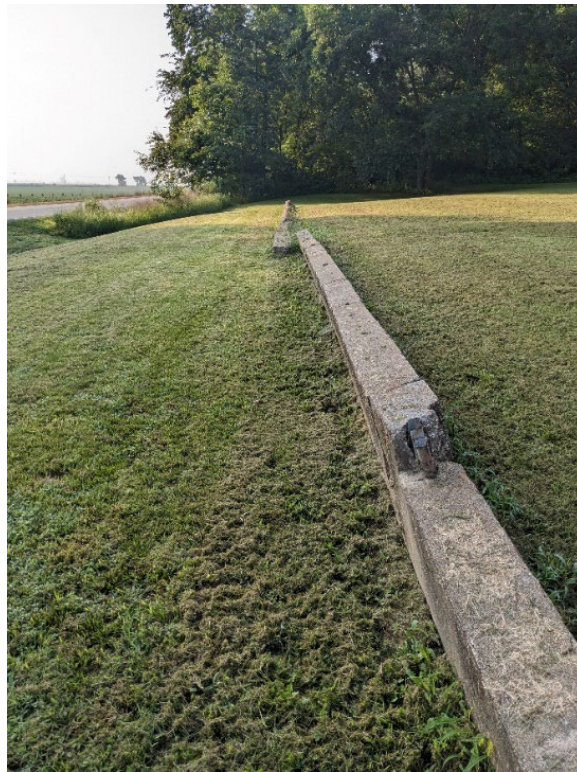
FIGURE 244. View southeast along the concrete retaining wall in the yard southeast of the house.
