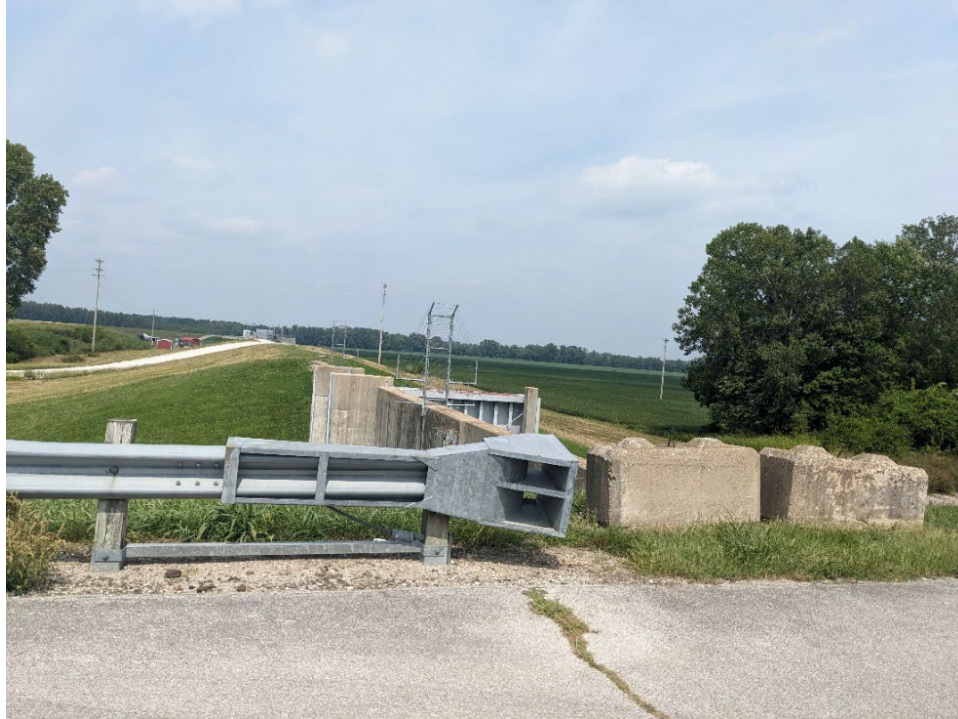
FIGURE 99. View across the levee set within le Grand Champ to protect Ste. Genevieve from Mississippi River floods.
