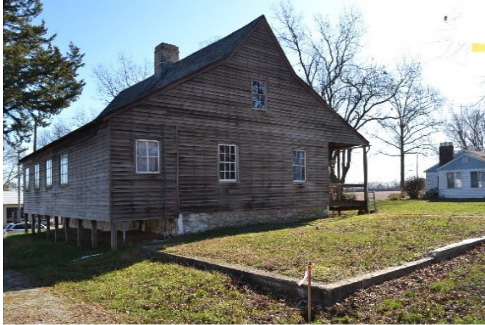
FIGURE 211. The concrete foundation is adjacent to the west façade of the dwelling. (Source: LSHLA, October 2020)
