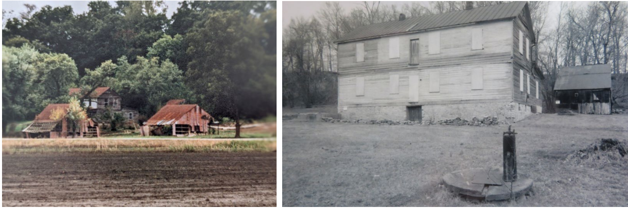
FIGURES 235 AND 236. A 1993 photograph of the property after the flood, left, and an image of the house taken in July 2000 after the porches have been removed. (Source: Ste. Genevieve NHP archives, left, Missouri Department of Natural Resources, Felix Vallé State Historic Site archives)
