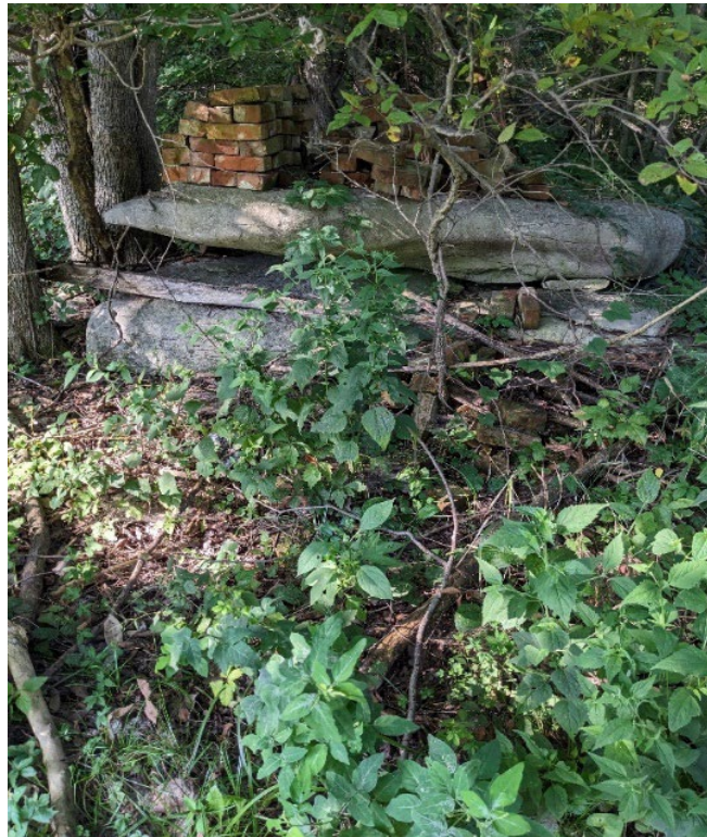
FIGURE 245. Foundation ruins and stacked building materials behind the house that may relate to a former smokehouse.
