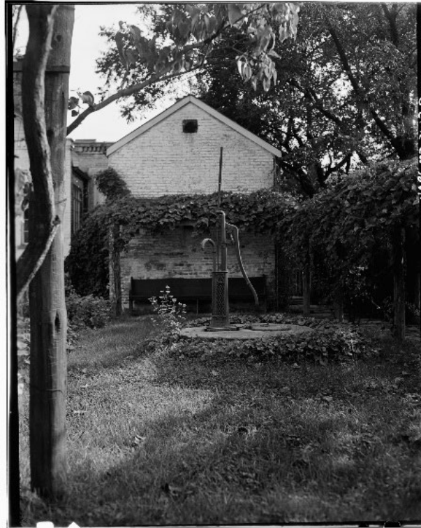
FIGURE 62. A circa 1934 view of the well looking south toward the house, showing the concrete slab at the base and a metal pump set off-center on top. (Source: HABS Survey No. MO-31-10, Library of Congress)
