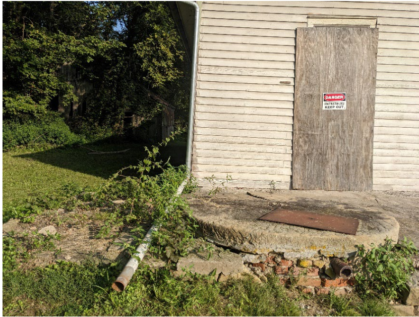
FIGURE 252. View of the cistern south of the house.
