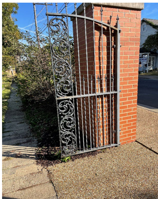
FIGURE 162. Ornamental iron gates are attached to both sets of brick entrance piers. (Source: LSHLA, October 2022)
