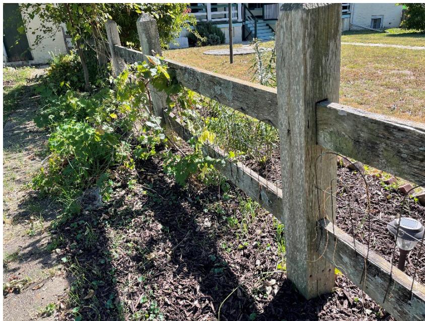
FIGURE 166. A wood post and rail garden fence separate the landscape west of the house. (Source: LSHLA, October 2022)
