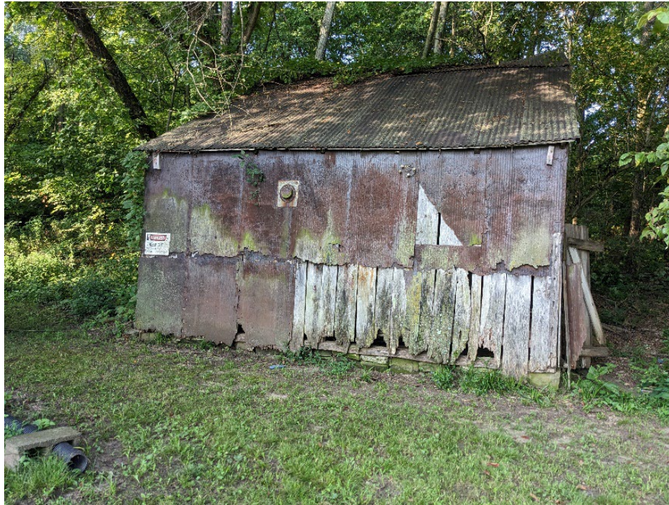
FIGURE 241. View west toward the wood shed.
