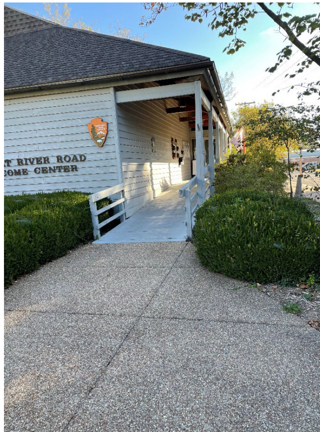
FIGURE 112. View of Welcome Center and its accessible entrance ramp.
