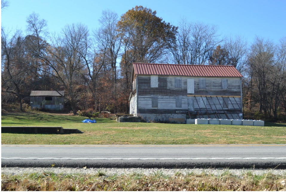
FIGURE 225. View toward the portion of the parcel located west of U.S. Highway 61 showing the open area in front of the house, with woodlands and outbuildings behind as the terrain rises toward bluffs to the west. (Source: LSHLA, November 2023)
