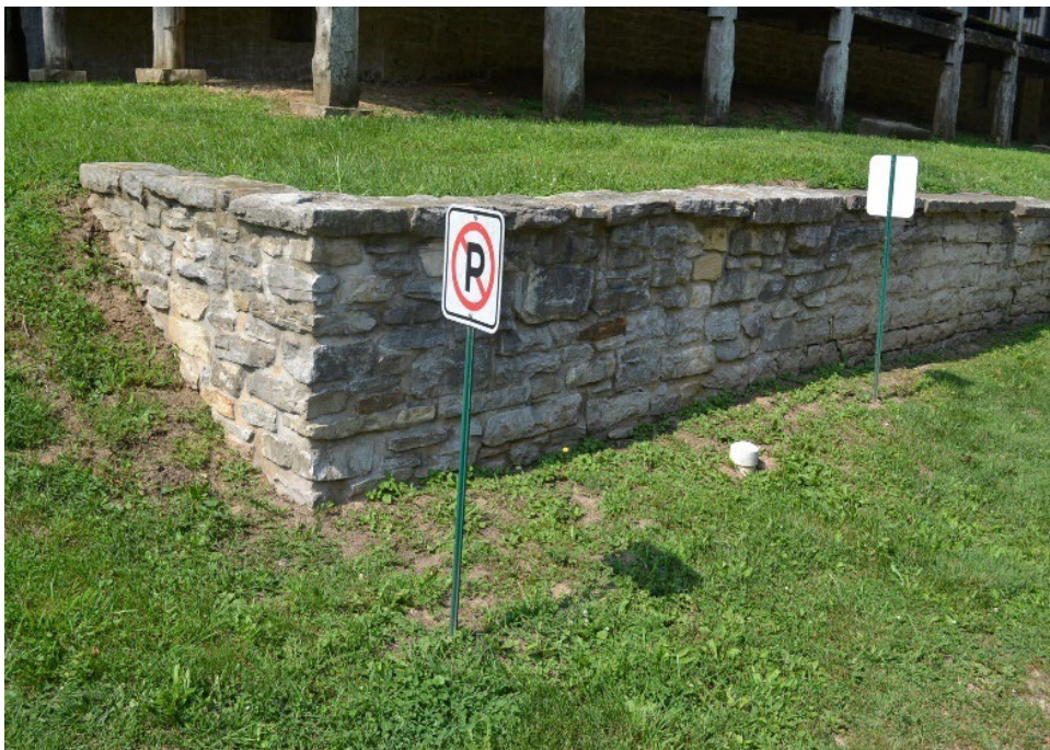
FIGURE 190. No parking signs are set in the grass in front of the stone retaining wall.
