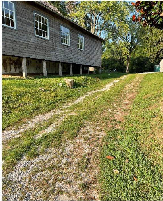
Figure 201. An access drive cuts through the embankment and is edged by steep slopes.
