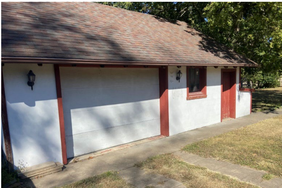
FIGURE 159. The garage is located west of the house, adjacent to the south boundary fence. (Source: LSHLA, October 2022)
