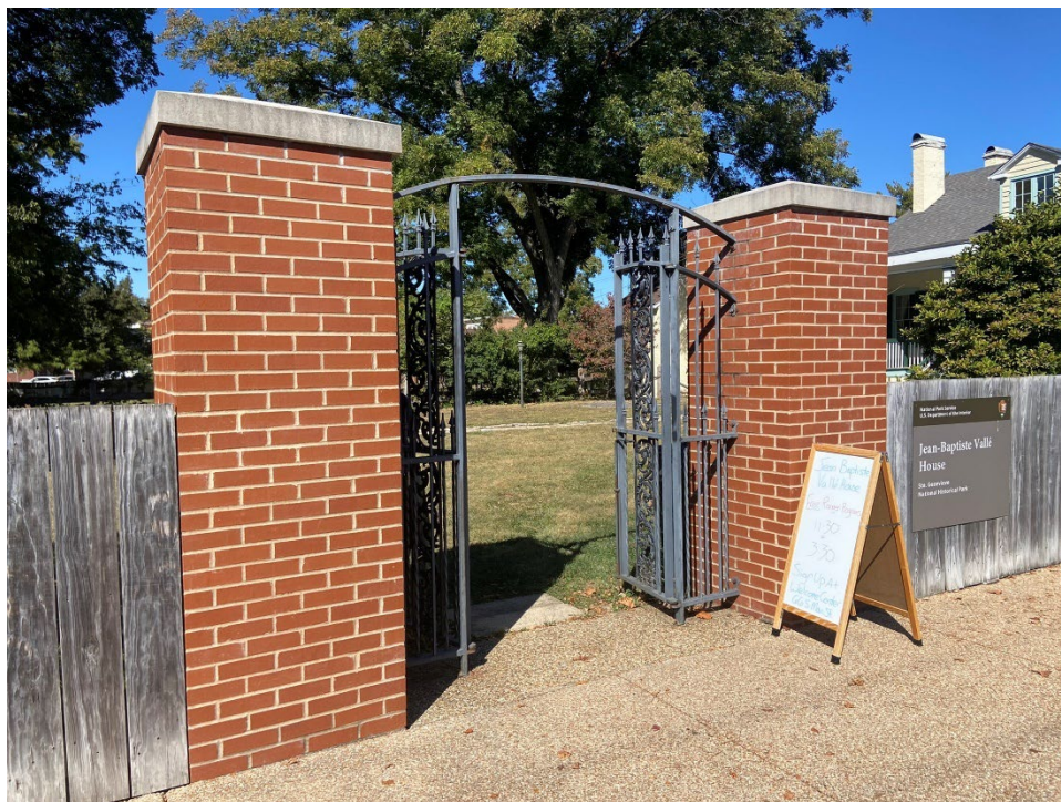
FIGURE 161. Brick entrance piers along the east boundary fence of the site. (Source: LSHLA, October 2022)
