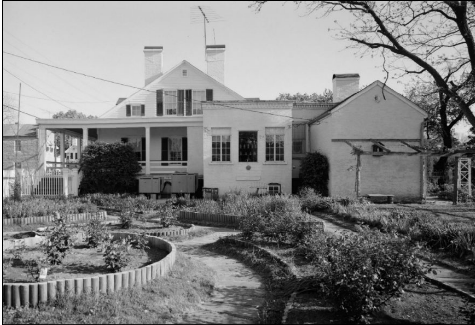
FIGURE 65. The French garden in the 1980s with new plantings, new parterre bed edging, and a general clearing of all the large shrub vegetation as seen in previous photographs. (Source: HABS Survey No. MO-31-10, Library of Congress)
