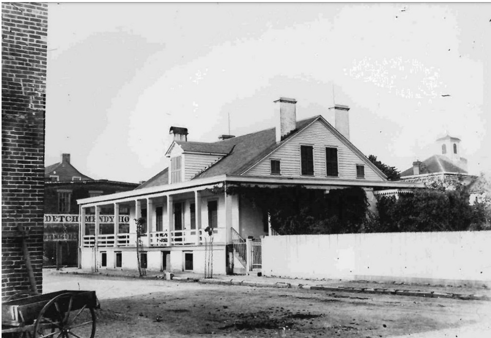
FIGURE 147. Circa 1890s photograph of the Jean Baptiste Vallé House from the northeast, possibly from the roof of the Lagrave Building (58 South Main Street). (Source: Appears in Houck, History of Missouri )
