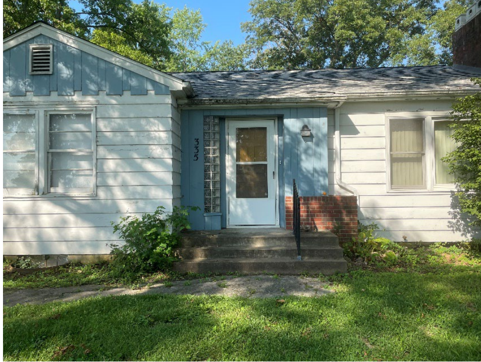
FIGURE 267. The entrance to the dwelling on the east façade is reached via a flight of concrete steps and a stone pathway that arises at the concrete driveway.
