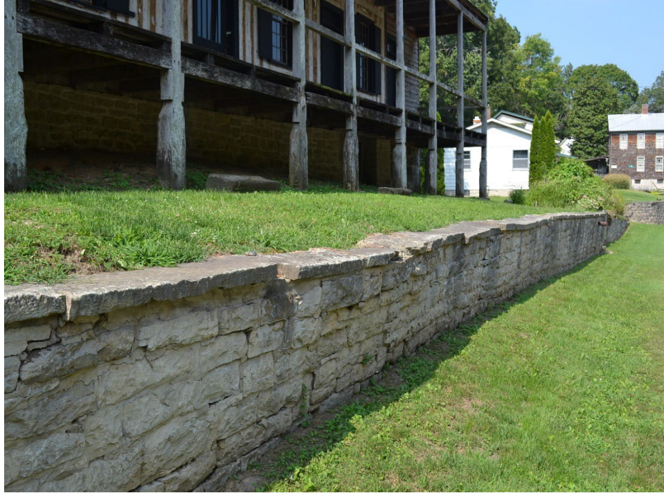
FIGURE 187. The existing stone retaining wall running parallel to the house structure has undergone changes over time due to the raising and lowering of St. Marys Road and maintenance and management of the structure.
