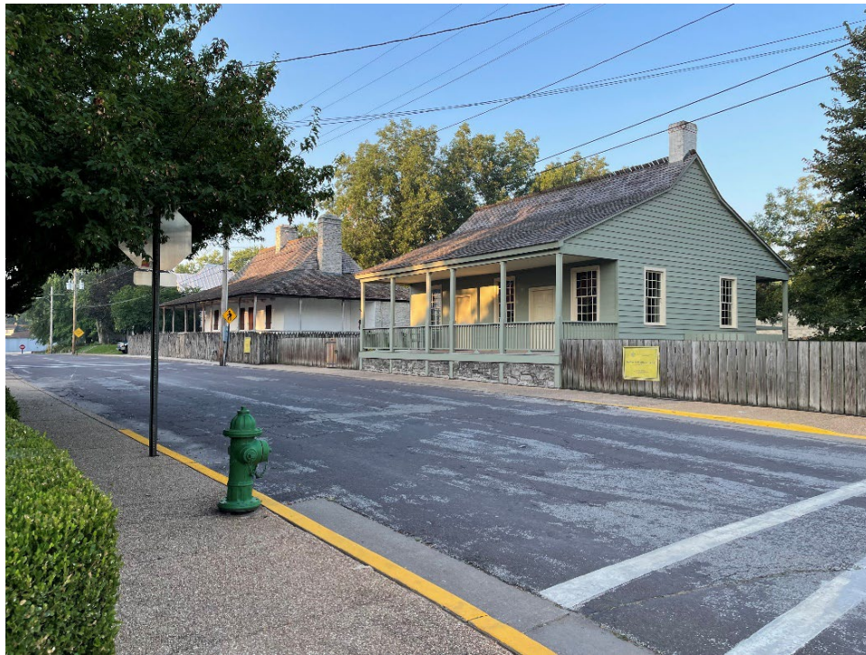
FIGURE 125. The Jean Baptiste Vallé House is part of a cluster of six historic French colonial period buildings built between 1793 and 1844 and located along South Main Street near the center of the city. These help to convey a sense of the character of Ste. Genevieve during the early nineteenth century.
