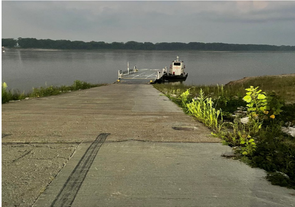
FIGURE 98. View of the Ste. Genevieve-Modoc River ferry looking east across the Mississippi River.
