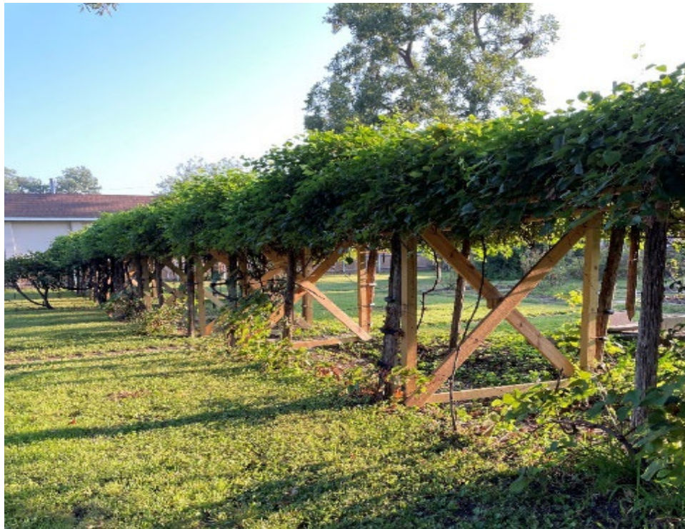
FIGURE 160. The grape arbor with new wood structural posts and cross braces.
