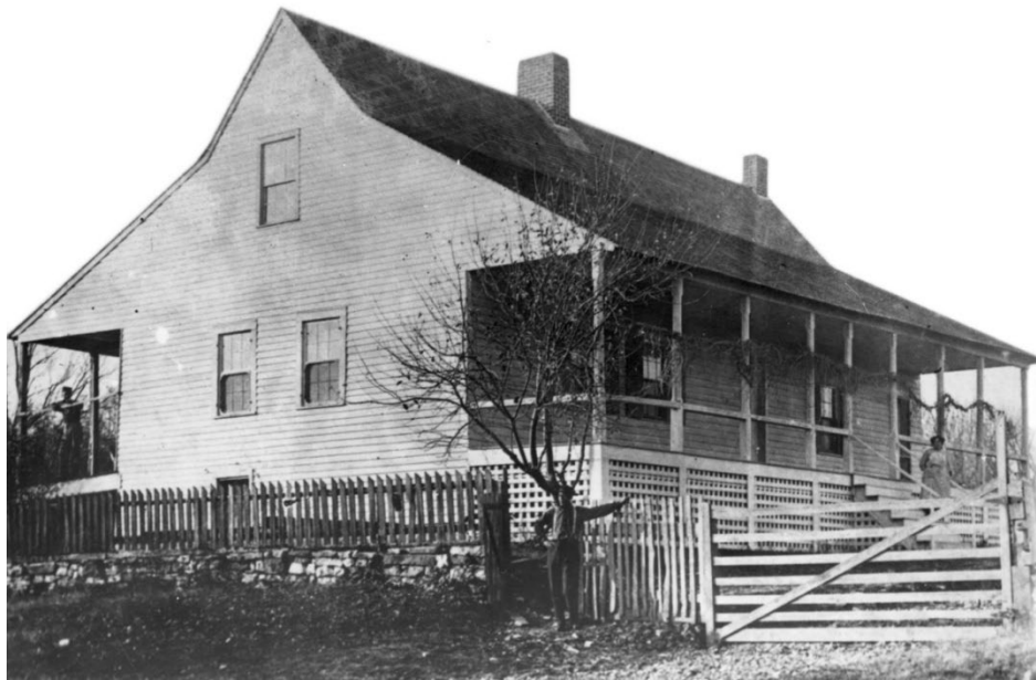
FIGURE 45. Undated circa 1920s photograph of the house from a similar angle showing the stone wall and wooden picket fence, gate at the north drive, adjacent tree, and the addition of lattice underneath the north porch. (Source: Missouri State Historical Society, https://mohistory.org/collections/item/N38681 )
