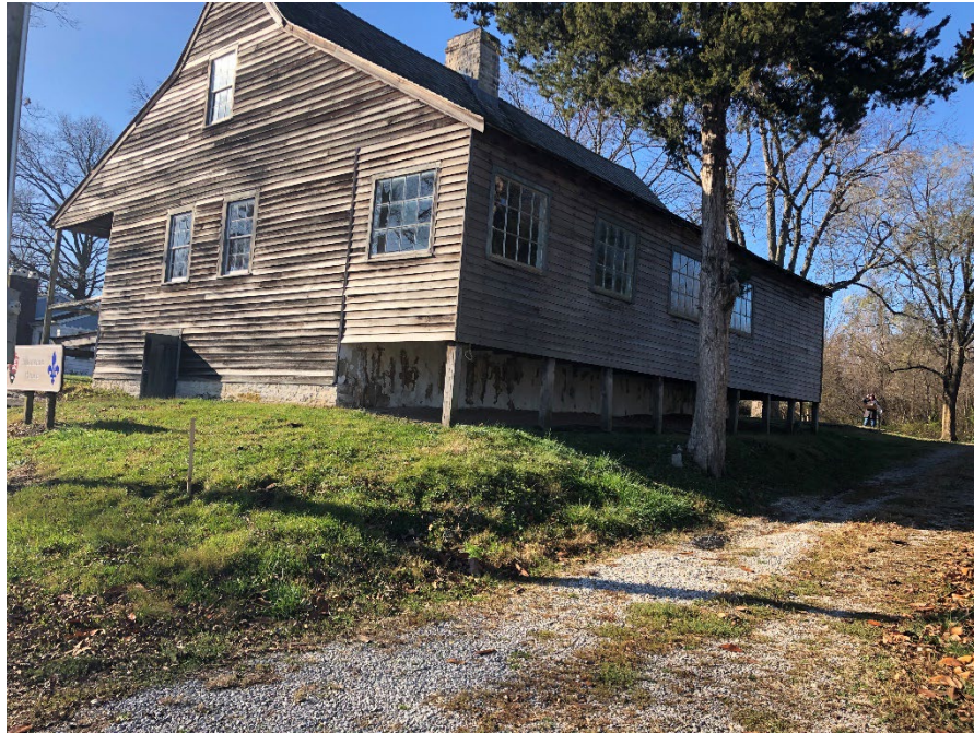
FIGURE 210. View of the east and north façades of the Bauvais-Amoureux House sited atop the embankment west of St. Marys Road. (Source: LSHLA, October 2020)
