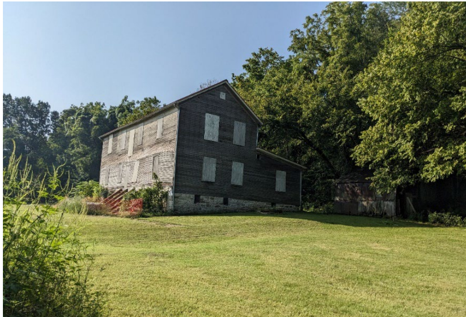
FIGURE 227. View south toward the house with the graded landform of the driveway visible.
