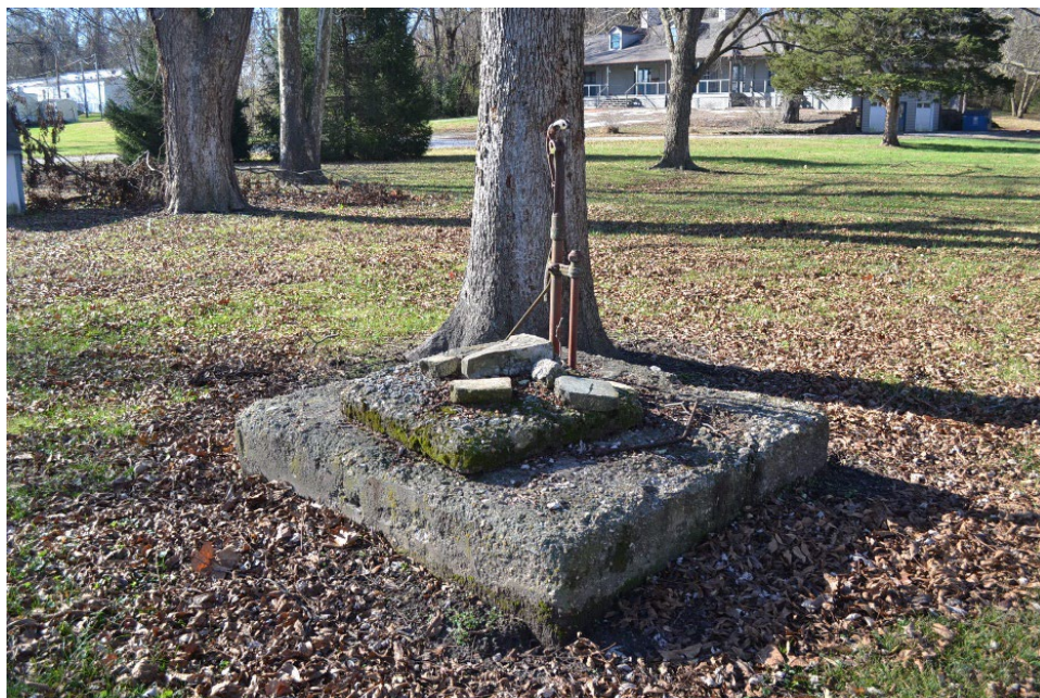
FIGURE 221. The well/cistern on adjacent property is located next to a large pecan tree and consists of a large stone base with a metal pump. (Source: LSHLA, October 2020)
