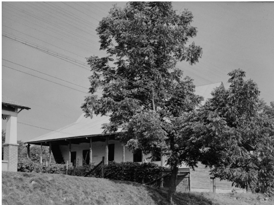
FIGURE 53. A circa 1937 photo of the south façade of the Bauvais-Amoureux House showing the adjacent house, and a fence between the two. A walnut or ash tree is along the road. (Source: Survey No. HABS MO-1113, Library of Congress)
