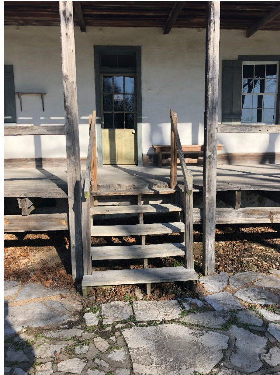
FIGURE 205. The wood steps connect the south walkway with the south gallery of the house. (Source: LSHLA, October 2020)
