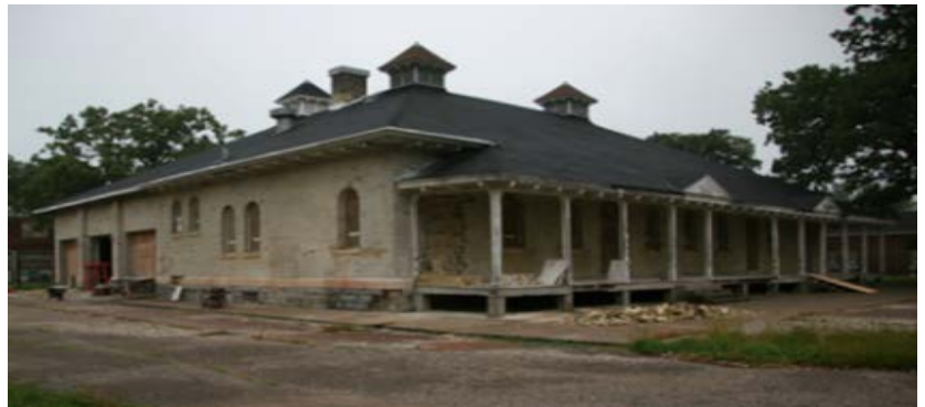
Renovation of Building 165, the Territorial Jail, Fort Snelling National Historic Landmark. A large portions of the roof that had collapsed has been repaired and the brick and stone have been cleaned, replaced and repaired, with much of the work being done by Hennepin County Sentencing to Service crews.
