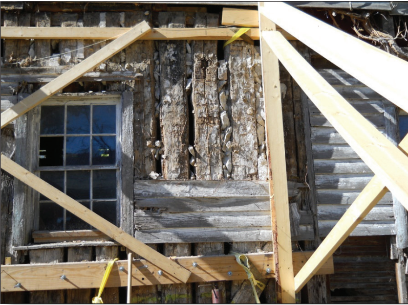
Figure 6. View of an exterior wall of the Lalumandiere House, constructed ca. 1829, showing vertical log construction with pierreotage. (Bonnie Stepenoff)
