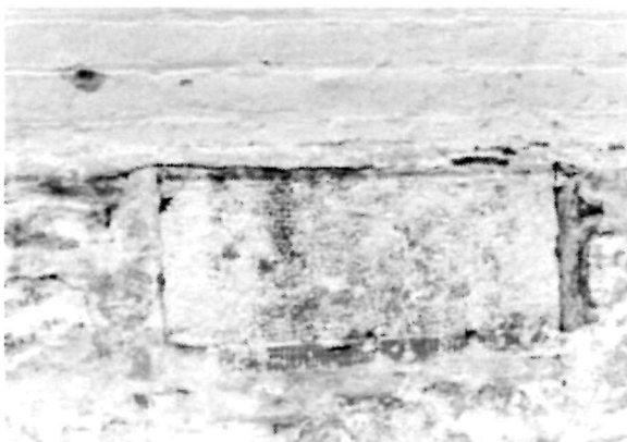
Figure 32 Detail view of the flush stone lintel (its purpose unknown) located near the east end of the north elevation of the Keeper's Dwelling, 1994.
