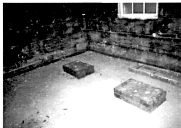
Figure 73 View looking toward the northeast corner of the Machinery Room in the Fog Signal Building, 1995. The concrete pads formerly supported two diesel generators.
