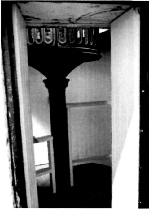
Figure 46 View looking into the Lantern Room of the Tower toward the cast iron pedestal, which formerly supported the third order Fresnel lens, 1994.
