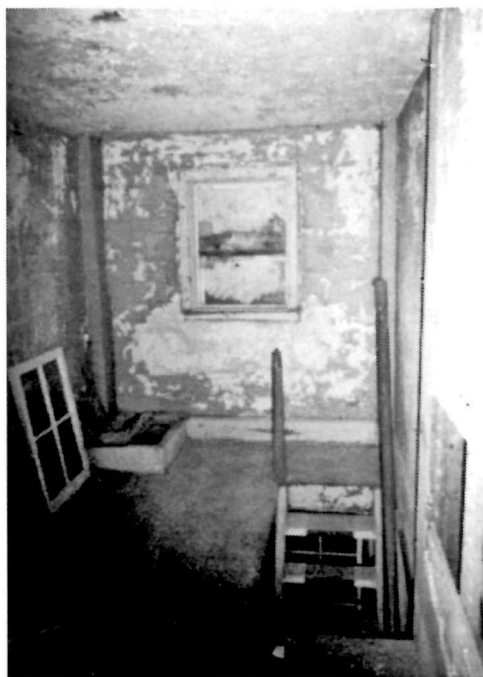
Figure 2 View looking east in the finished portion of the Dwelling's attic, 1994. The raised wood platform at the northeast corner once supported a ship's ladder, which led up to the roof lantern.
