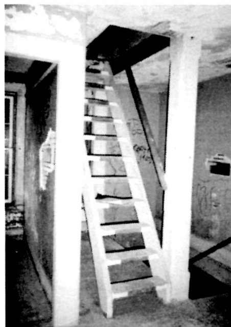
Figure 1 View of the wood ship's ladder at the second floor central hall of the Dwelling, which leads up to the attic, 1994. Note the "scoop" at the corners of the wood treads and the painted runner.
