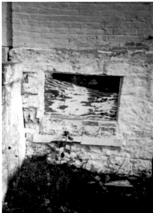
Figure 29 View of the basement window (D-1) at the east end of the south elevation of the Keeper's Dwelling, 1994. Note the deteriorated foundation wall between the window and the concrete steps.
