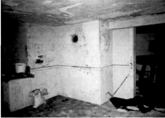
Figure 57 View looking northwest in the Assistant Keeper's Kitchen (Room B-06). Note the deterioration of the plaster at both the ceiling and walls.
