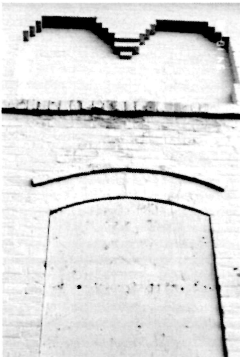
Figure 15 View of the south wall of the Keeper's Dwelling, showing the cracked keystone, 1995.
