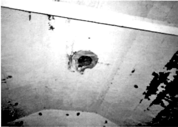
Figure 69 Detail view of an opening in the ceiling of the Fog Signal Building, 1995. A metal chimney stack once extended through this opening.
