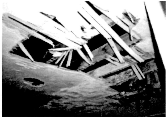
Figure 68 View of the ceiling in the southwest bedroom (Room 205), 1994. Note the large amount of missing plaster and broken lath, both the result of vandalism.
