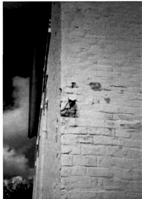
Figure 34 View looking west at the southeast corner of the Keeper's Dwelling, 1994. Note the deteriorated condition of both the cementitious parging and the underlying brick.
