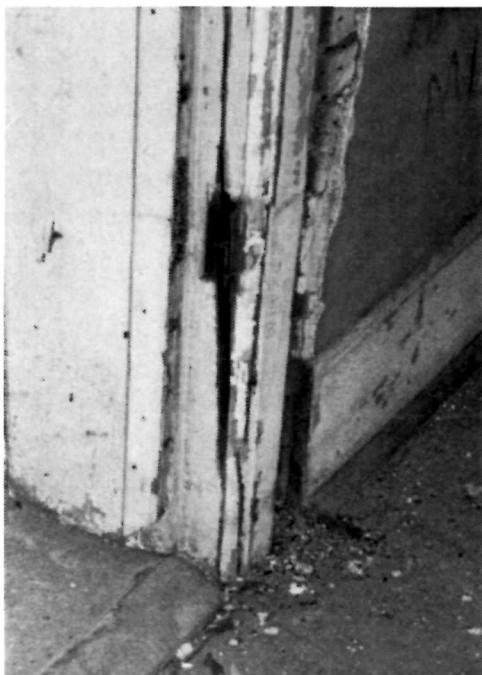
Figure 59 Detail view of the deteriorated and damaged wood door jamb at Door E-4 in Room 101 of the Keeper's Dwelling, 1994.
