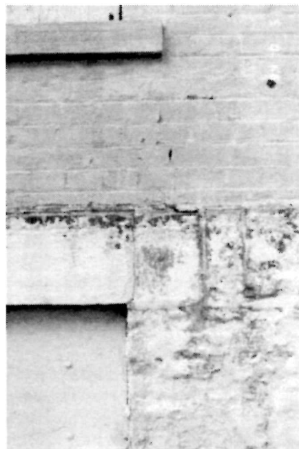
Figure 11 View of the east wall of the Keeper's Dwelling, south side, showing the window head stone cracking, 1995.
