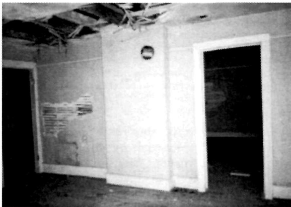
Figure 17 View of the south wall in the northwest bedroom (Room 204) in the Keeper's Dwelling, 1994. Note the rust at the plaster surface from the metal duct within the wall framing (at the bottom left corner of the photograph).
