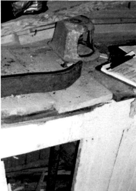
Figure 58 Detail view of the wood beaded board cabinet and the remaining piece of the metal hand pump at the sink in the northwest corner of the Assistant Keeper's Kitchen (Room B-06), 1995.
