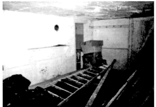
Figure 15 View looking toward the southwest corner of the kitchen (Room B-05) in the Dwelling. Note the overall deteriorated condition of the surfaces and finishes, and that the fireplace remains infilled with brick and plaster.
