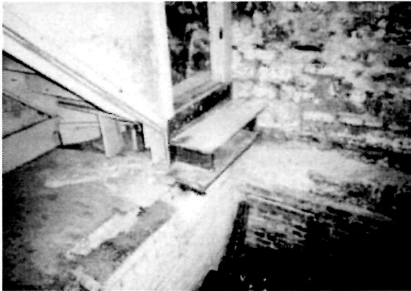
Figure 54 View of the stair that hangs precariously over the subcellar (Room B-03) in the Keeper's Dwelling, 1994
