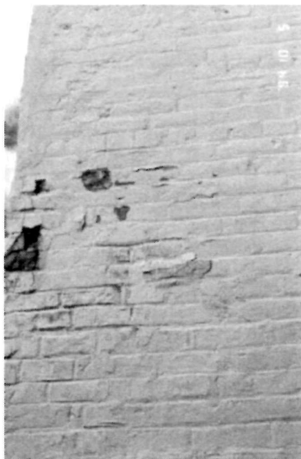
Figure 12 View of the east wall of the Keeper's Dwelling, south side, showing surface spalls near corner, 1995.
