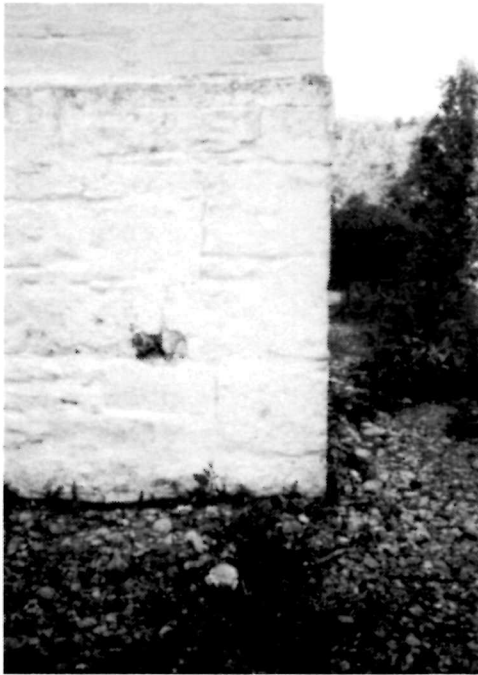
Figure 31 View of the northeast corner of the stone foundation wall at the Keeper's Dwelling, 1994. Note the cracking of the cementitious parge coat along the profile of the cut stone quoining.
