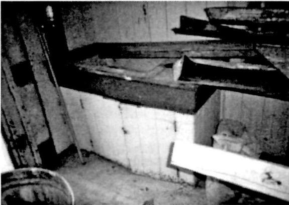
Figure 12 View looking at the northwest corner of the kitchen (Room B-05) in the Dwelling, 1994. Note the area of missing wood wainscot at the left edge of the photo, revealing an earlier wall treatment.
