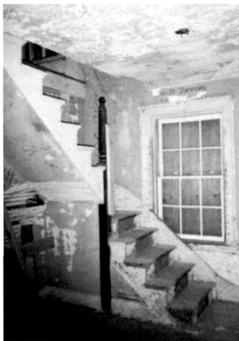
Figure 62 View looking northeast in the Entrance Hall (Room 101) toward the stair, 1994. Note that the balustrade and some of the tread nosing are missing at the stair, and the deteriorated condition of the adjacent plaster surfaces
