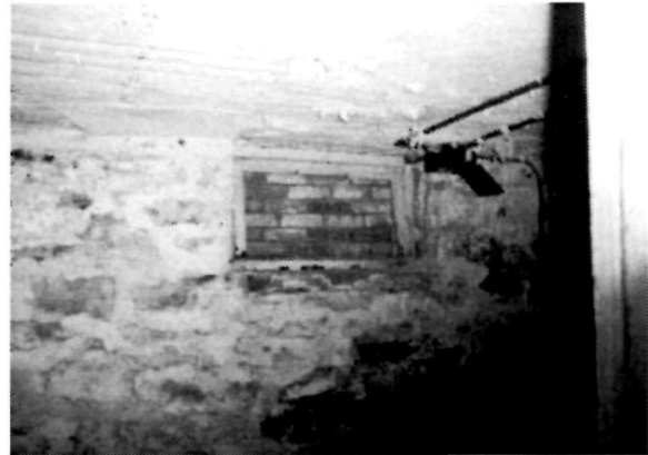
Figure 53 View of the east wall in the northeast basement storage room (Room B-03) of the Keeper's Dwelling, 1994. Note that most of the parging has worn or broken off of the stone wall surface.
