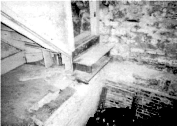
Figure 11 View looking northwest in the storage room (Room B-03) in the Dwelling, 1994. Note the door opening at the left leading from the stair, which has one step leading into this room that is precariously hanging over the subcellar.
