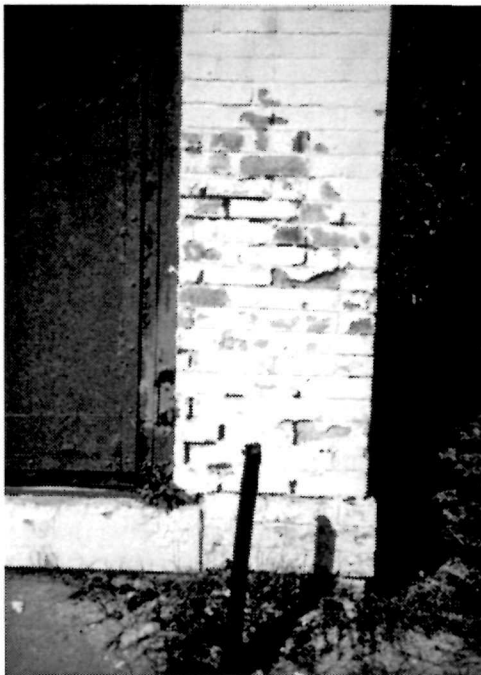
Figure 77 Detail view of the north end of the east elevation of the Brick Oil House, 1994. Note the spalling brick and deteriorated mortar joints.
