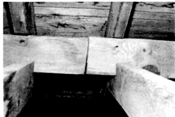
Figure 19 View of the beam butt joint at the south side of the roof, 1995.
