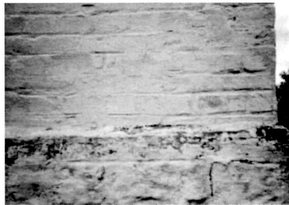
Figure 28 View of the west end of the north elevation of the Keeper's Dwelling, 1994. Note that the parging is crudely tooled to resemble mortar joints, a typical condition of the exterior brick wall surfaces.
