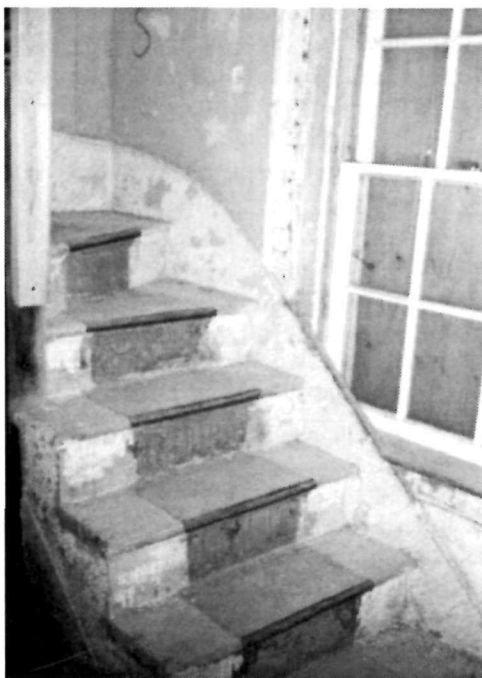
Figure 60 Detail view of the face of the stair risers that are painted a darker gray to give the appearance of a continuous stair runner, 1994.
