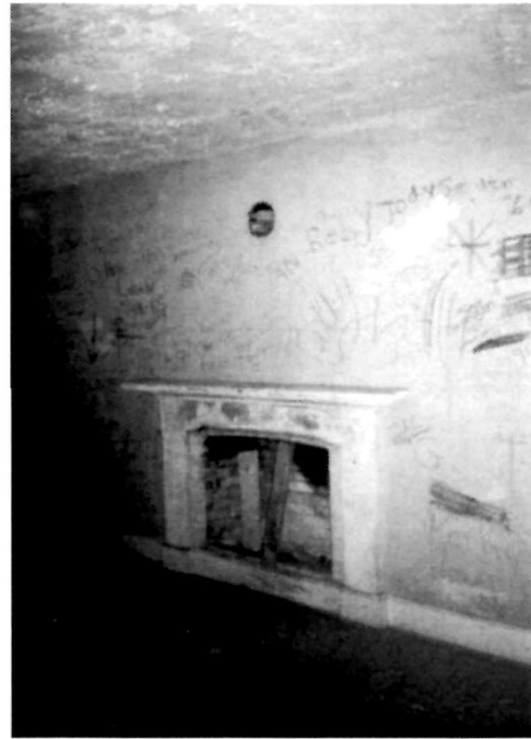
Figure 64 View of the fireplace along the north wall of the South Parlor (Room 104), 1994. Note that although the brick and plaster infill has been removed at this fireplace, the baseboard remains across the opening.
