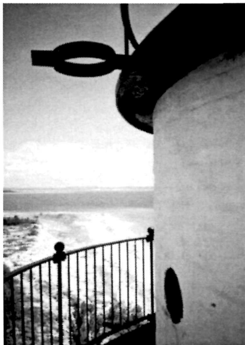
Figure 42 Detail view of the exterior of the Tower, including a remaining metal bracket, which formerly supported the chimney stack from the stove in the work room, 1994.
