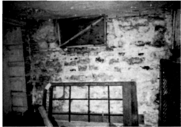
Figure 50 View of the east wall in the southeast basement storage room (Room B-01) of the Keeper's Dwelling, 1994. Note the remnants of the parging that was tooled to resemble masonry.
