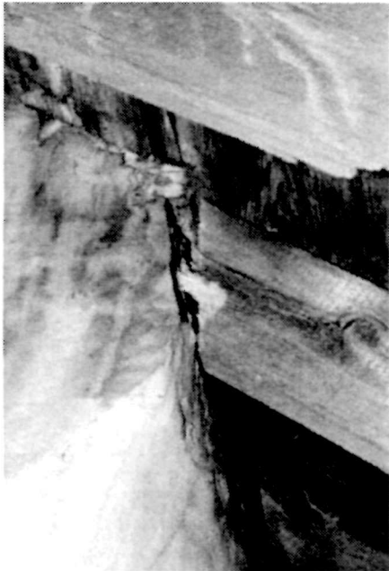
Figure 20 View of a rafter cut at the spiraling chimney of the Keeper's Dwelling, 1995.
