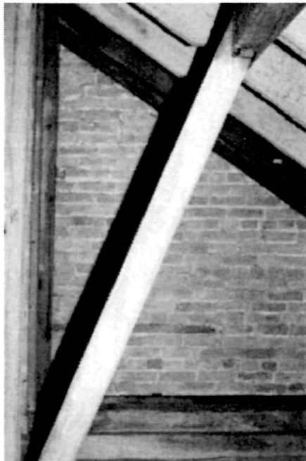
Figure 17 View of the diagonal strut and birds mouth jointing in the attic of the Keeper's Dwelling, 1995.
