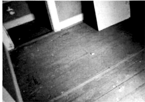
Figure 66 View looking southwest at the floor of the Stair Hall (Room 202), 1995. The heavy paint buildup has caused the paint to fail and loosen in large chunks.
