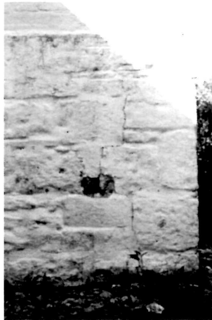
Figure 10 View of the foundation wall distress of the east wall of the Keeper's Dwelling, 1995.
