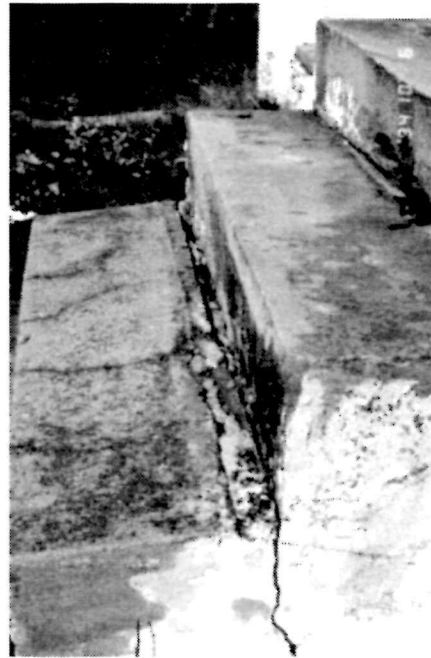
Figure 16 View of the stair distress at the south exterior stair of the Keeper's Dwelling, 1995.
