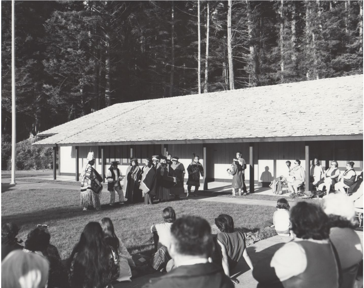
Circa 1971 photo of the triangular lawn area with the flagpole in its original location and a portion of the concrete entry sidewalk that was removed in the late 1970s. A deciduous tree that was planted near the entry sidewalk and flagpole is no longer present. A pedestrian pathway was installed in 2000 that matches a section of this historic alignment (SITK 15656 D).
