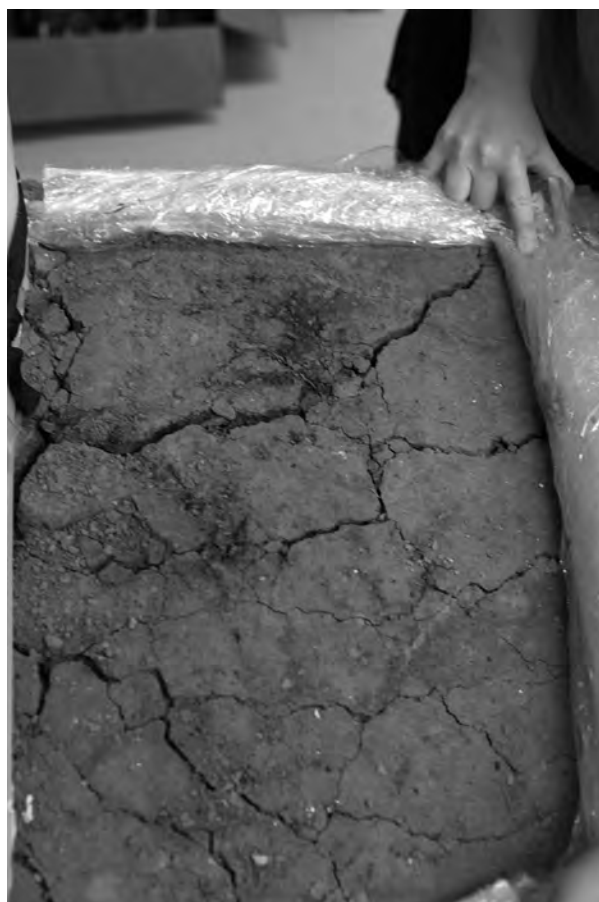
Figure 19-05. Lower step of Block A, Feature 147. Note extensive desiccation and seismic cracking.
