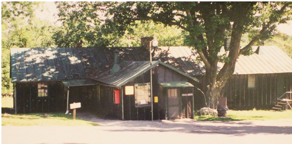
Figure 3.19. Technical Building, west façade, ca. 1995. (Image courtesy of Steve Bair)
