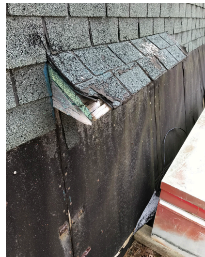
Figure 4.1. Crawl space access door and pent roof, August 24, 2020. (Image by author)
