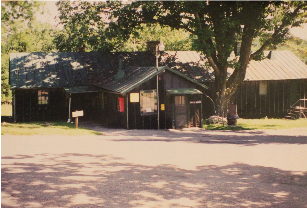
Figure 2.7. West elevation of Technical Building in early 1990s. (Courtesy of Steve Bair)
