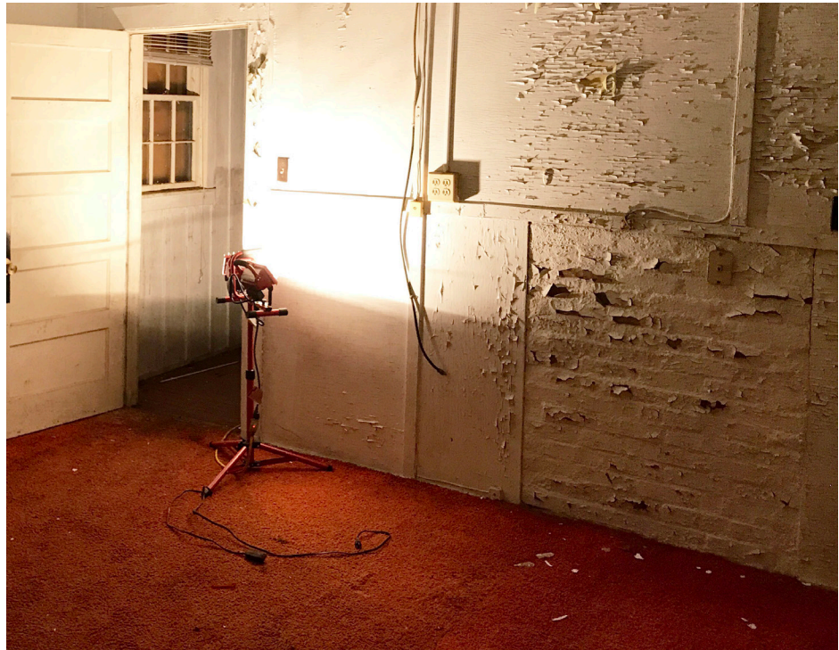
Figure 4.43. R106 looking towards north wall (Image taken by the author) February 25, 2020.
