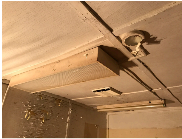
Figure 4.40. (left) R106 ceiling (Image taken by the author) February 25, 2020.
