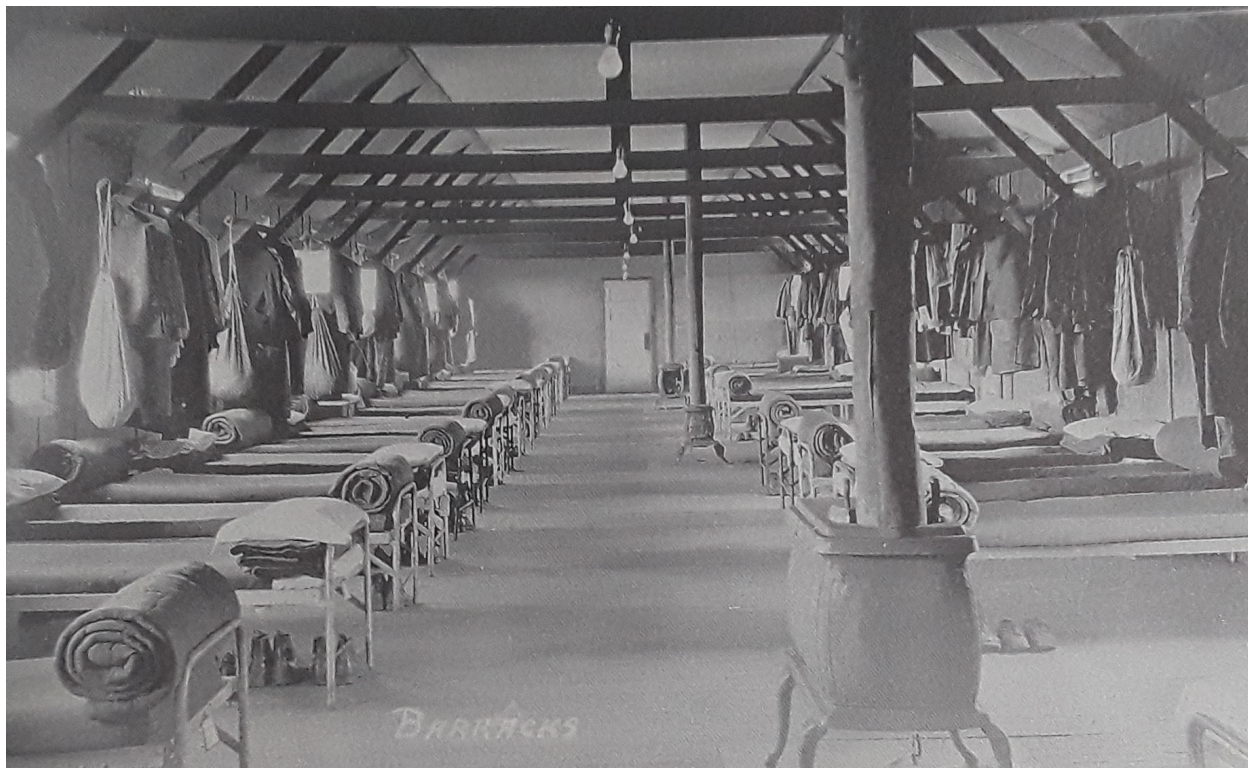
Figure 3.3. Big Meadows (NP-2), Shenandoah National Park. Barrack heated with wood stove. (Reed L. Engle, Everything was Wonderful )
