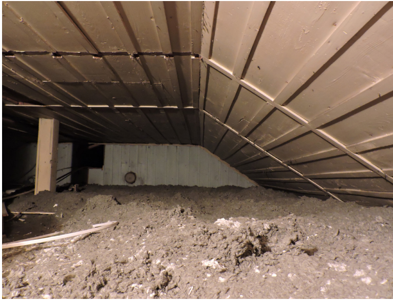
Figure 3.6. (above) Original vaulted ceiling in R102, now encapsulated in the attic, 2015. (Image by Eric Breitzkreutz)
