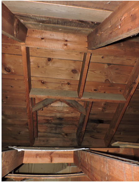
Figure 3.10. Attic above R108, 1935 roof jack framing, 2015. (Image taken by Eric Breitzkreutz)
