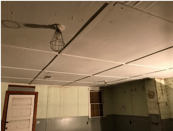
Figure 4.53. (above) R108, looking northwest, February 25, 2020. (Image by author)
