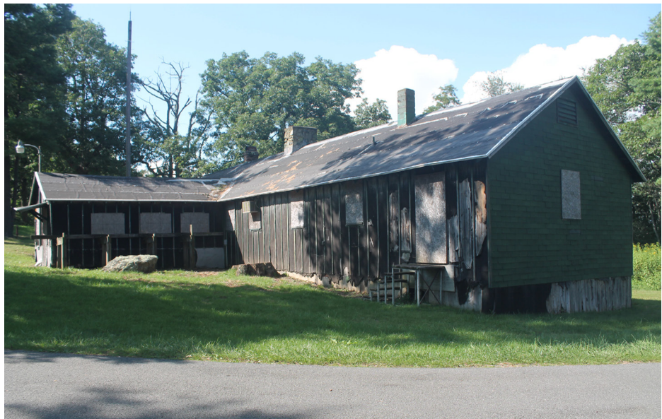
Figure 4.5. (top) West elevation shimmed rafter tails, August 25, 2020. (Image by author)
