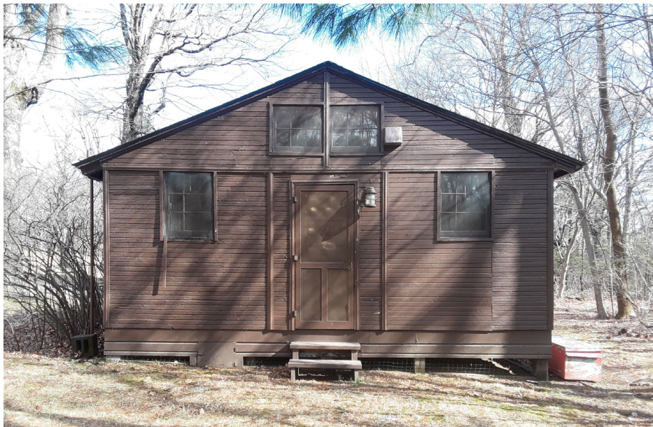
Figure 3.2. The Pinnacles CCC Structure, south elevation, Shenandoah National Park, February 26, 2020. (Image by author)
