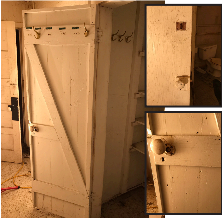
Figure 4.52. R107 CL107 door. Inset A: Exterior hardware. Inset B: Interior hardware, February 25, 2020. (Image by author)
