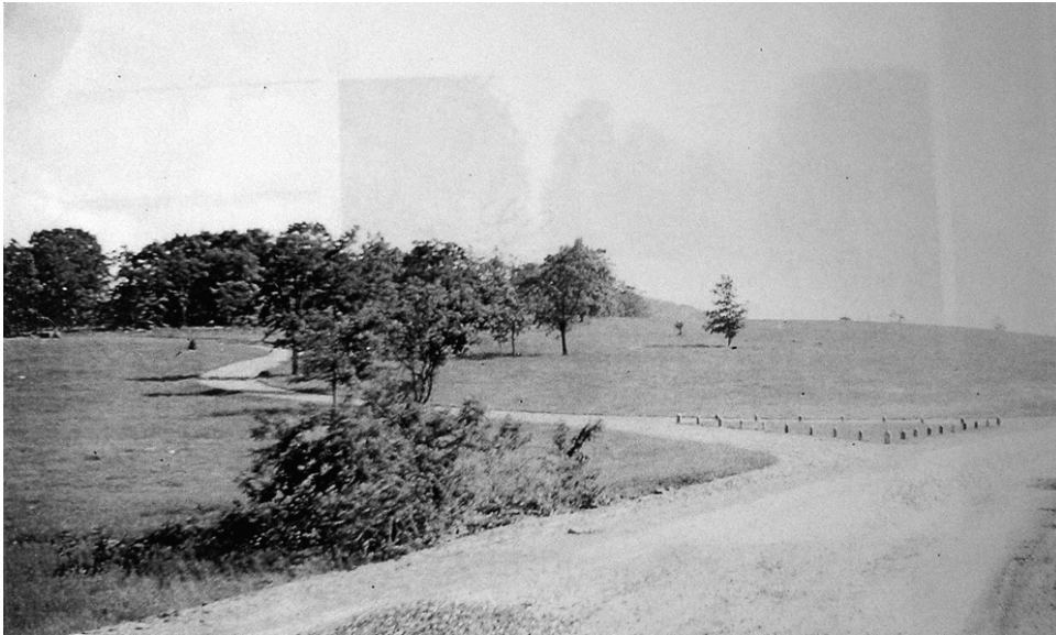
Figure 2. Same view looking south at the South River Picnic Grounds entrance from Skyline Drive, with the entrance completed, June 1935 (Shenandoah NP Archives, SHEN 29640, ACC 1568, Box 13).
