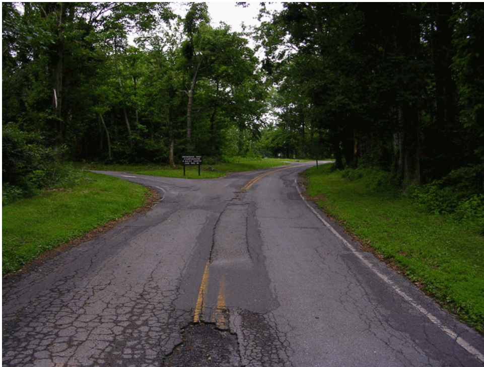
Figure 19. The site's loop road begins as a two-way approach from Skyline Drive. This view looks south at the large wye intersection (OCLP, 2008).
