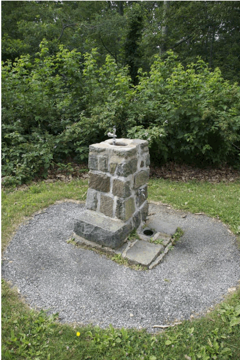
Figure 24. The historic mortared stone water fountains also feature a spigot on the side and a stone step (OCLP, 2008).
