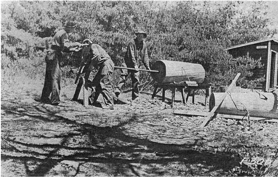
Figure 10. CCC crews building log water fountains like those originally used at South River Picnic Grounds (From "The Greatest Single Feature...A Sky-Line Drive," by Reed L. Engle).
