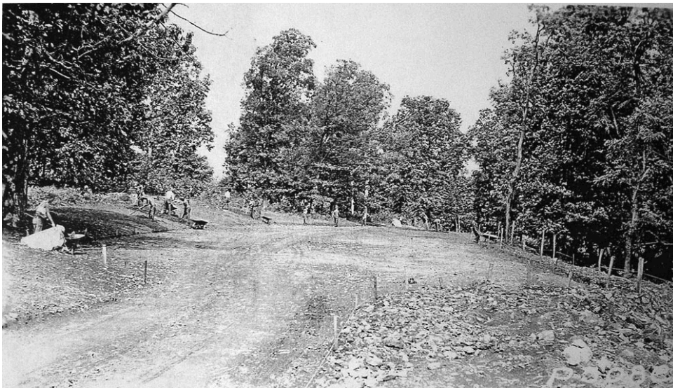
Figure 3. CCC crews building the south parking lot at the South River Picnic Grounds, view looking east, September 1935 (Shenandoah NP Archives, SHEN 52092-16B, Box 13, Folder 1-21, File No. 348c).
