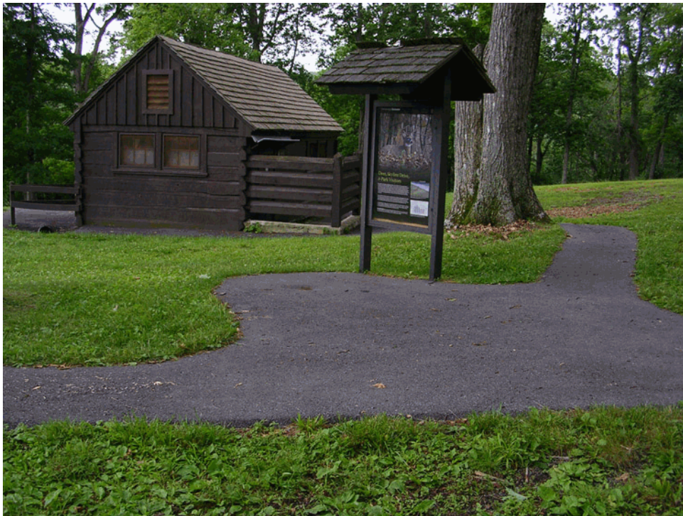
Figure 22. View looking south at the historic comfort station at South River Picnic Grounds. See also Figure 4 (OCLP, 2008).
