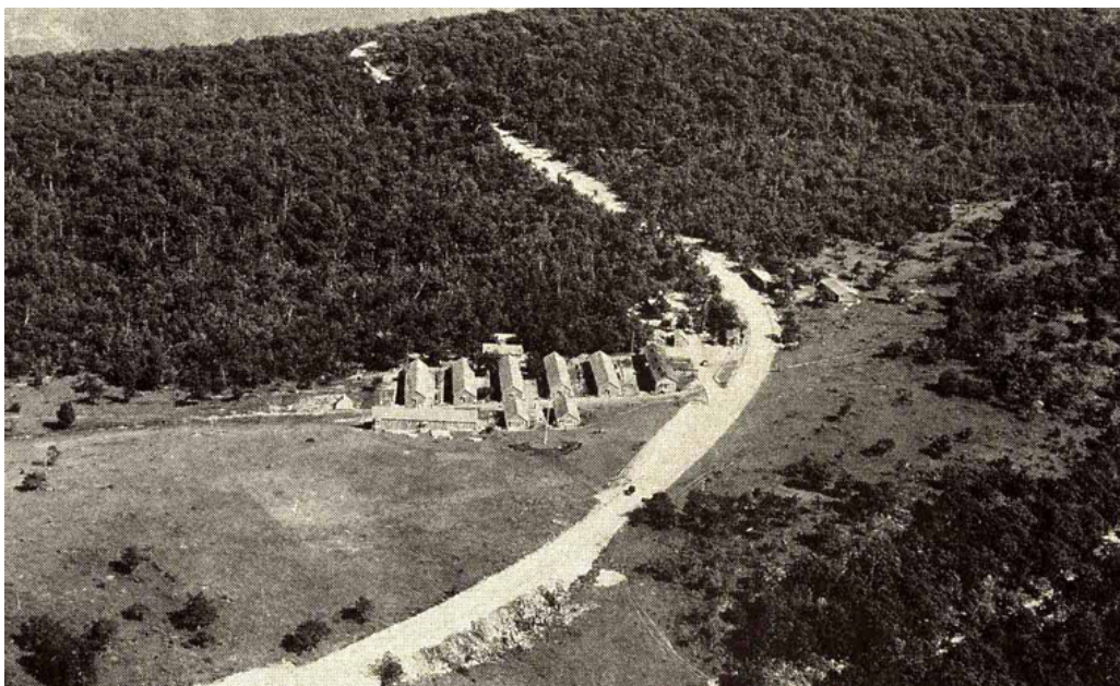
Figure 17: View of CCC Camp NP-1 at Skyland, from 1934 (Engle, 2003).
