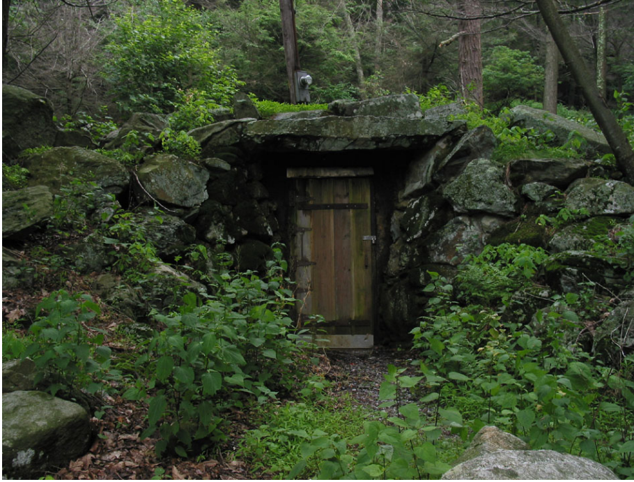
Figure 27: CCC pump house (OCLP, 2006).
