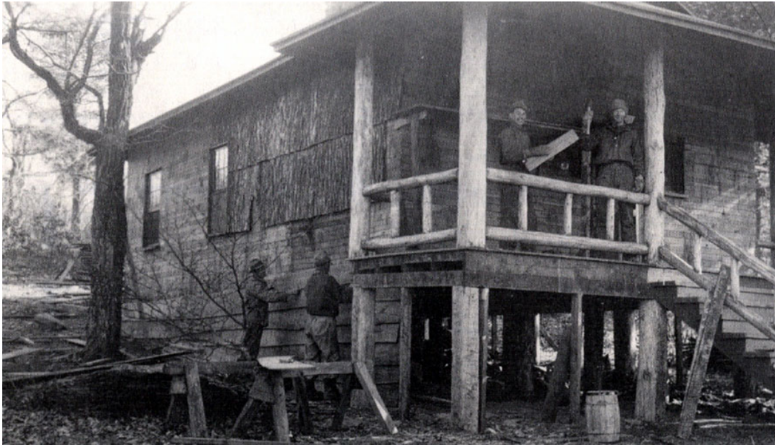
Figure 18: Renovations of many of the cabins at Skyland were undertaken by the Civilian Conservation Corps. This view is from 1937 (Engle, 2003).
