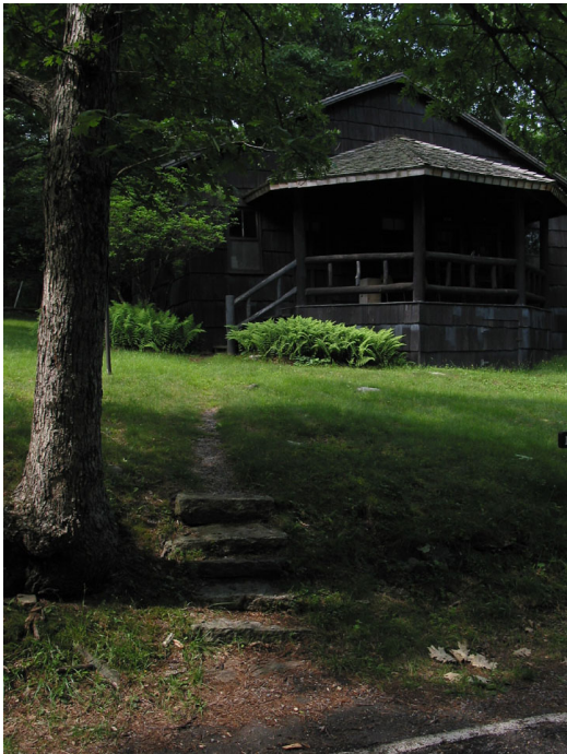
Figure 24: Historic gravel path and steps in front of the Boulder Cabin (OCLP, 2006).
