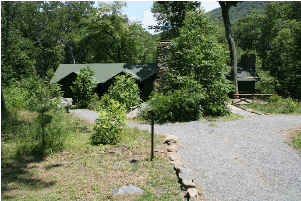
Figure 14. View of the restored roads and paths leading to the President's Cabin at Rapidan Camp (OCLP 2008).
