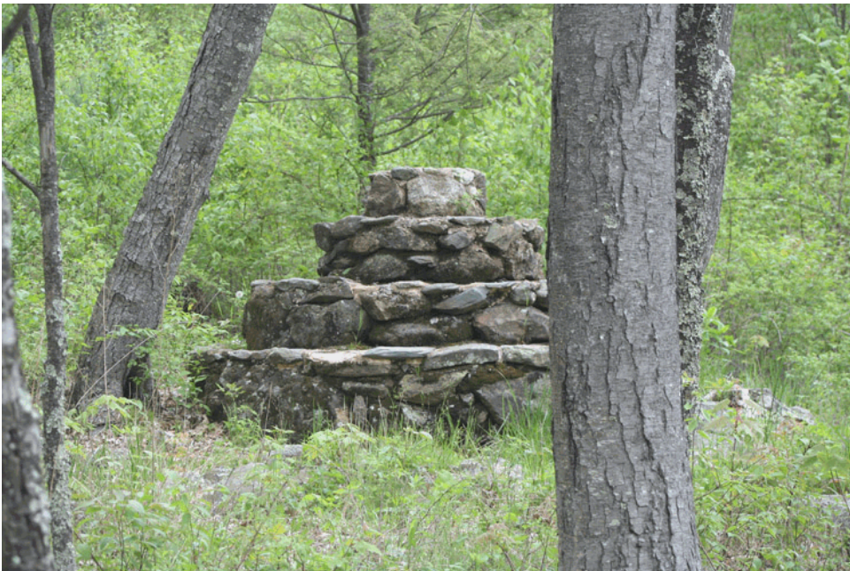
Figure 20. View looking west at the stone fountain and overgrown adjacent pools (OCLP 2008).
