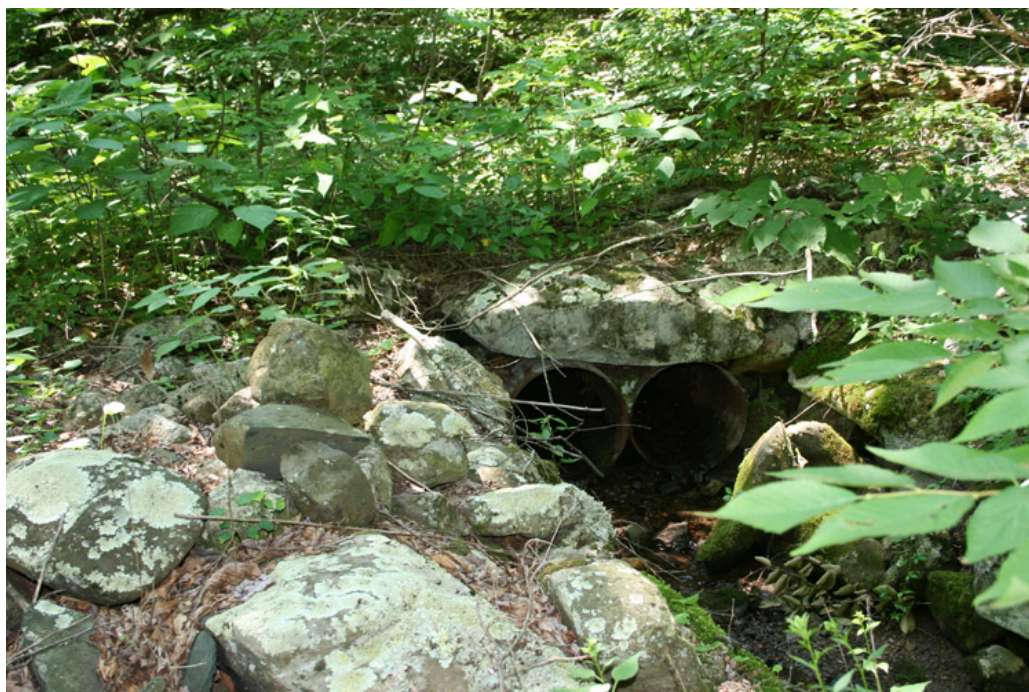
Figure 28. View of the third crossing from the sluice gate along Hemlock Run (OCLP 2008).
