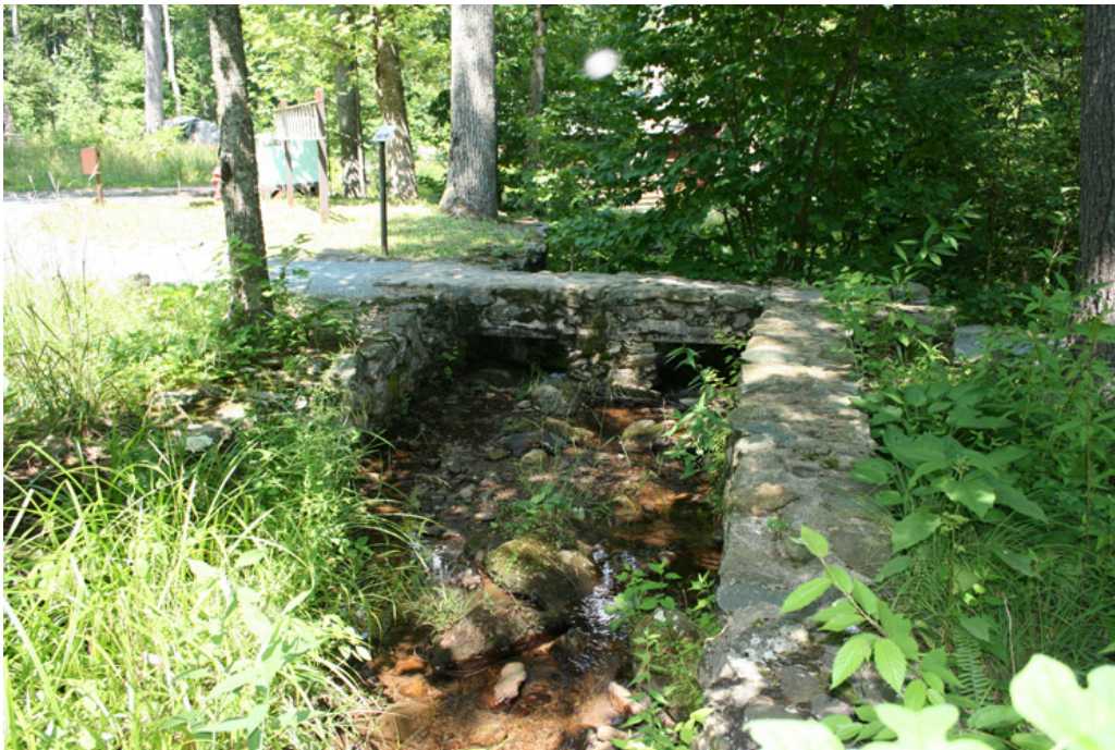
Figure 17. The mortared stone retaining walls along the man-made water channel, Hemlock Run, have recently been restored. View looking north (OCLP 2008).
