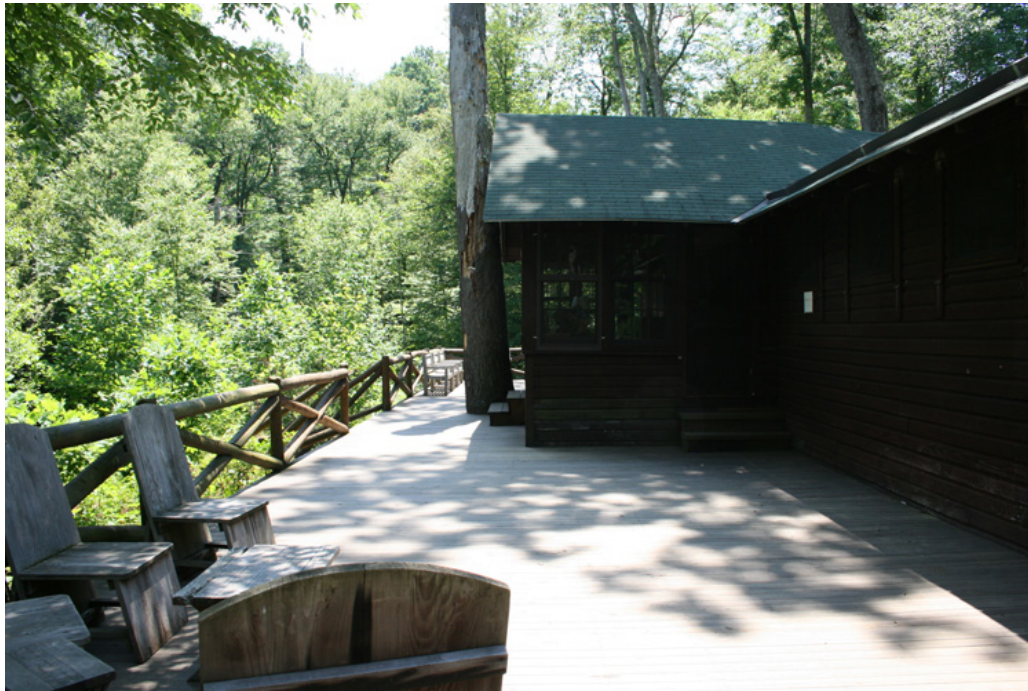
Figure 21. View looking south from the President's Cabin porch. The tree in the porch has since died and the hole has been patched with contrasting planking to indicate its former location (OCLP 2008).
