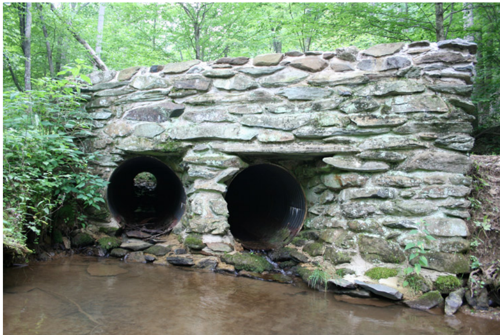
Figure 25. View from downstream of the recently repaired mortared stone bridge on the Entrance Road (OCLP 2008).
