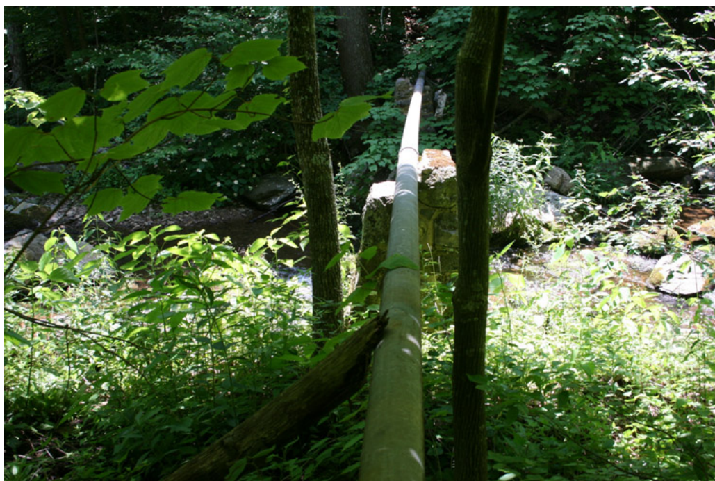
Figure 30. Although the septic system is no longer used, the sewer pipe and stone supporting piers over Laurel Prong have been retained (OCLP 2008).
