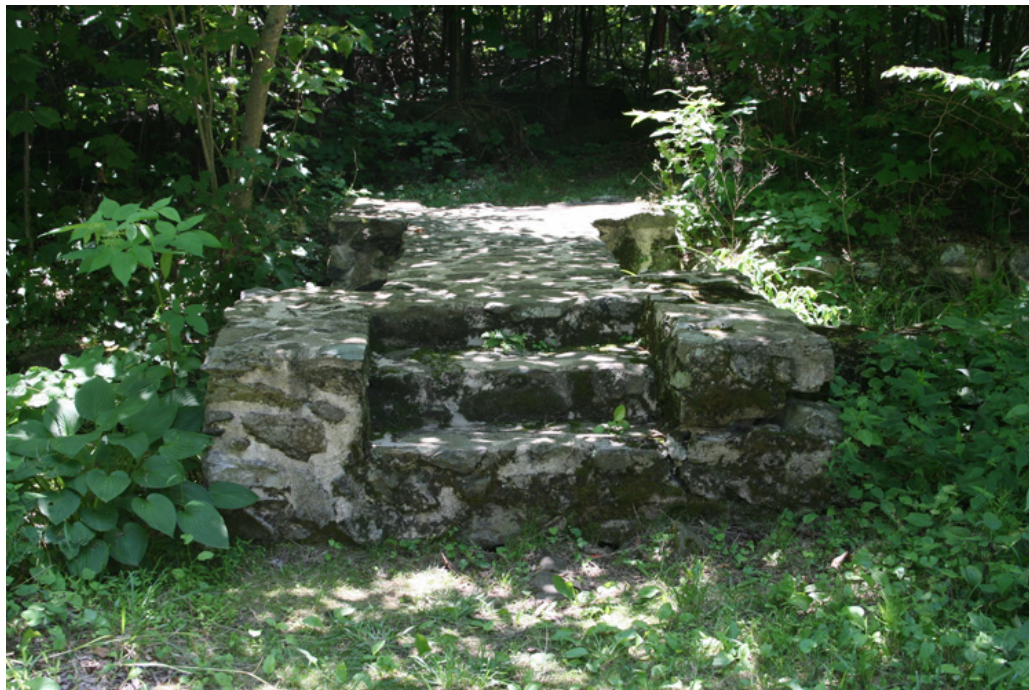
Figure 29. View of the fourth crossing from the sluice gate along Hemlock Run (OCLP 2008).
