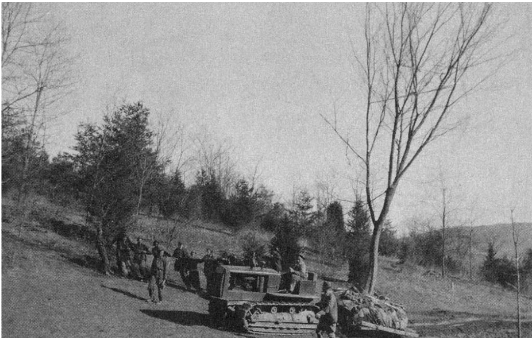
This tree, balled-and-burlapped by a crew from NP-10 and being moved by a bulldozer, gives an indication of the extent to which the CCC went to create a natural looking landscape (Engle 1999, 85).
