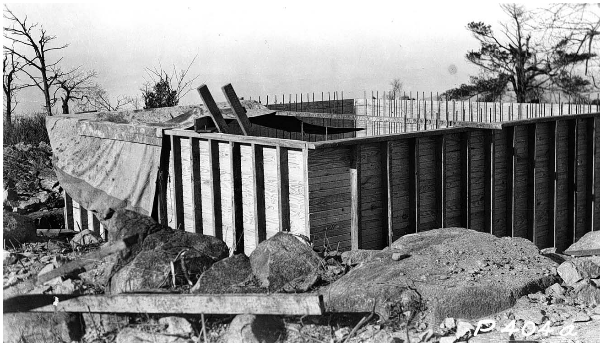
This 1936 photograph shows the Pinnacles Reservoir under construction (SHEN Archives 1936, ANCS 10415).
