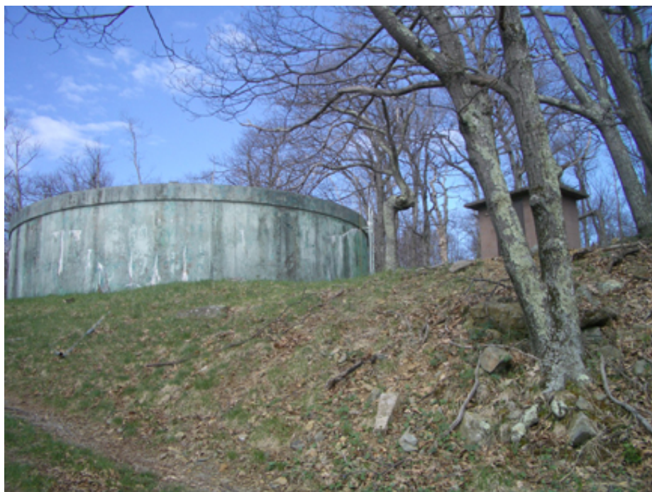
Fig. 26: Looking west at the water tank and shed on the Piney Ridge. (OCLP 2005)
