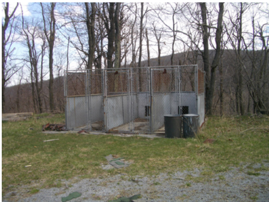
Fig. 32: Abandoned dog kennels are located behind the Maintenance/Equipment Shed-CCC. (OCLP 2005)
