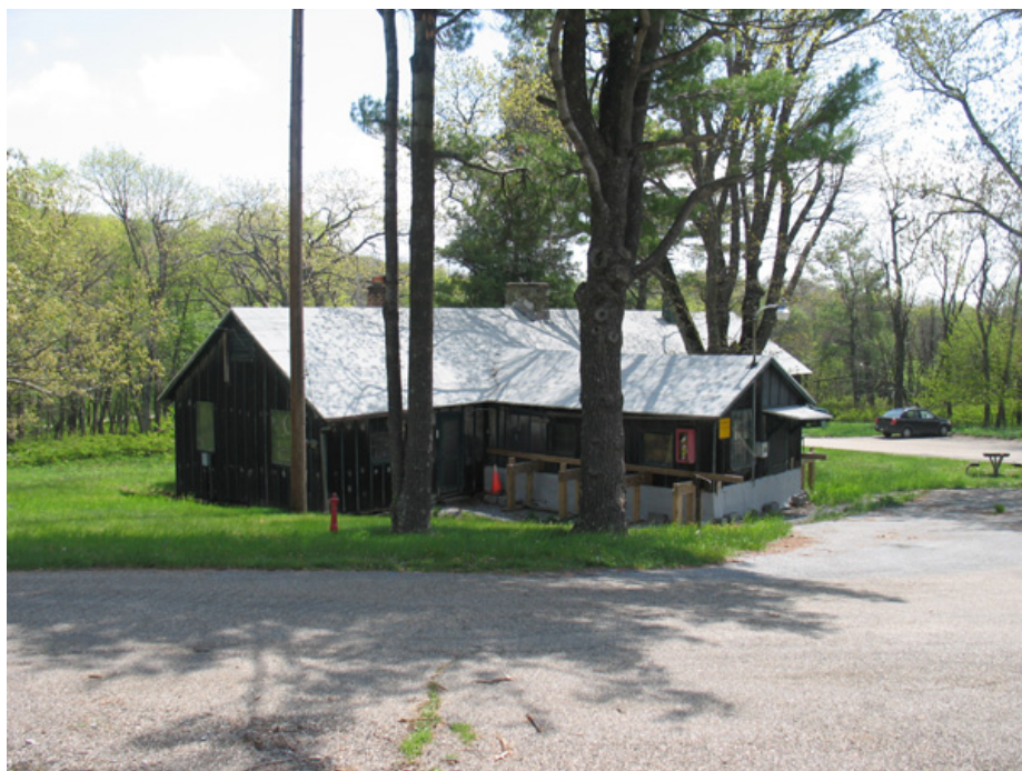
Fig. 23: Looking southeast at the Maintenance Office-CCC Technical Office. (OCLP 2006)
