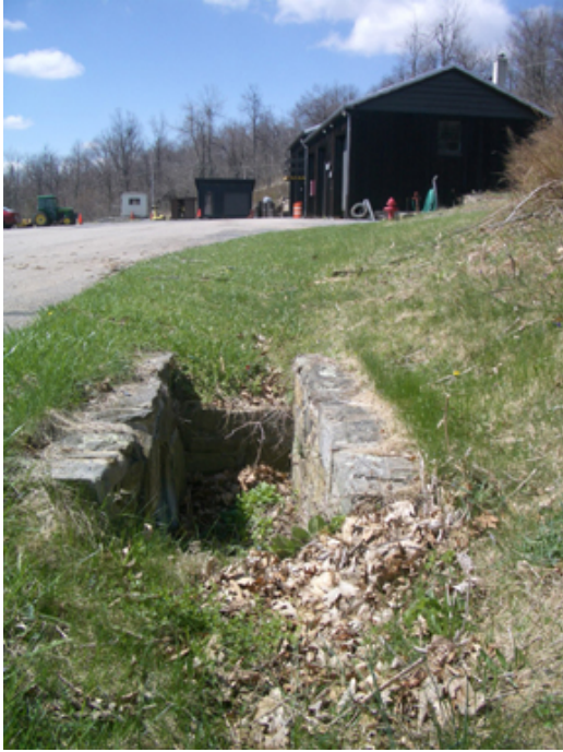
Fig. 27: Looking southwest at the stone culvert inlet along the road to the Maintenance Building. (OCLP 2005)
