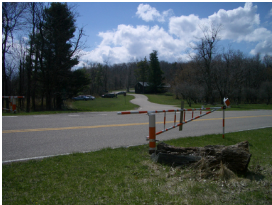
Fig. 18: View looking west at the access road from Skyline Drive. (OCLP 2005)
