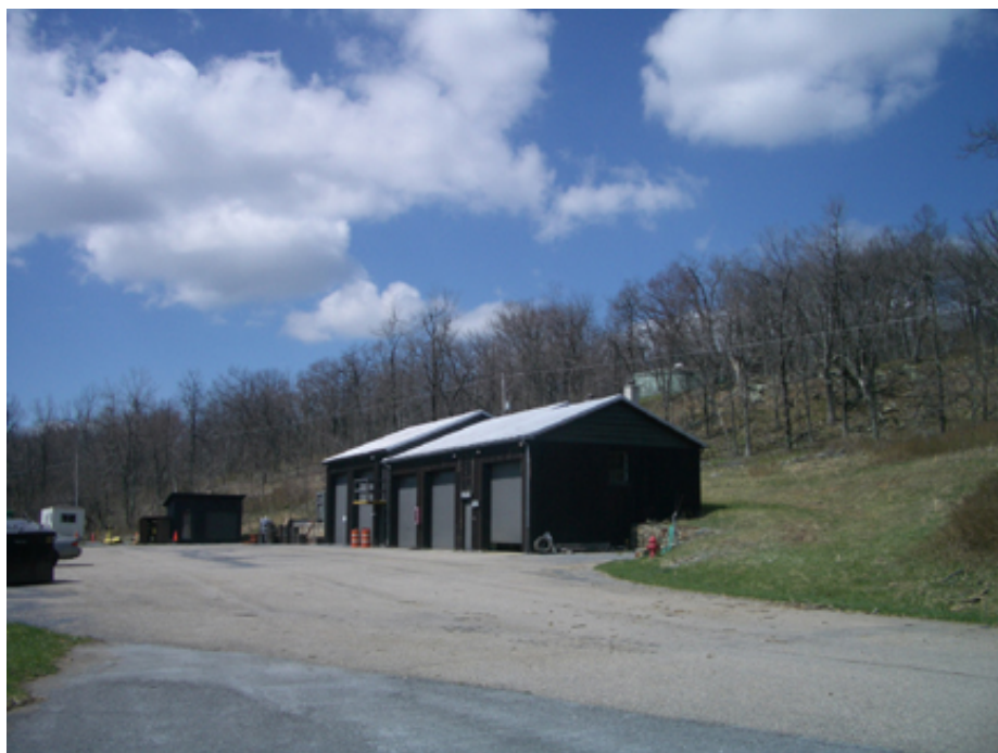
Fig. 12: View looking southwest at the Maintenance Building area. (OCLP 2005)
