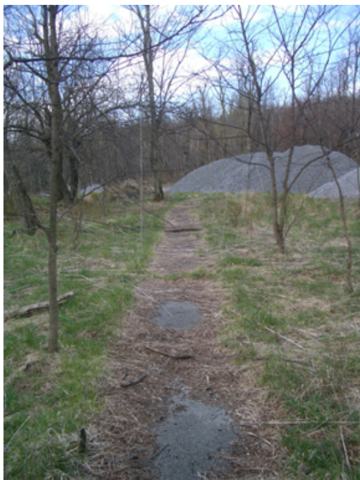
Fig. 22: Looking northeast at a remnant asphalt path built for trailer housing. (OCLP 2005)
