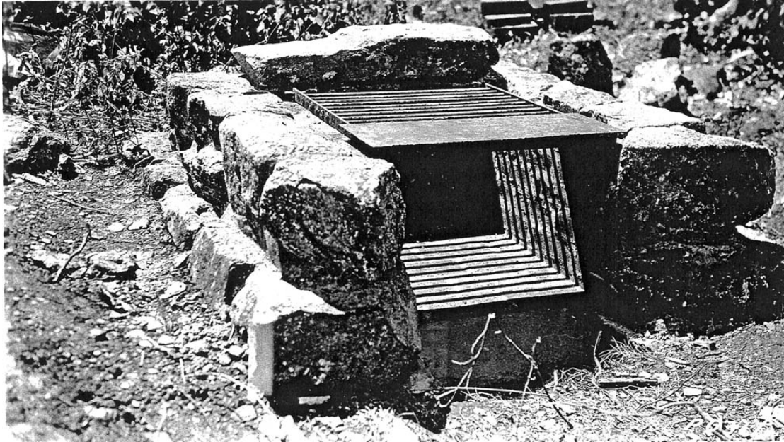
Figure 9. Typical stacked stone grill constructed by CCC at the campground at Big Meadows in 1937 (Shenandoah NP Archives, Negative No. 665-5).
