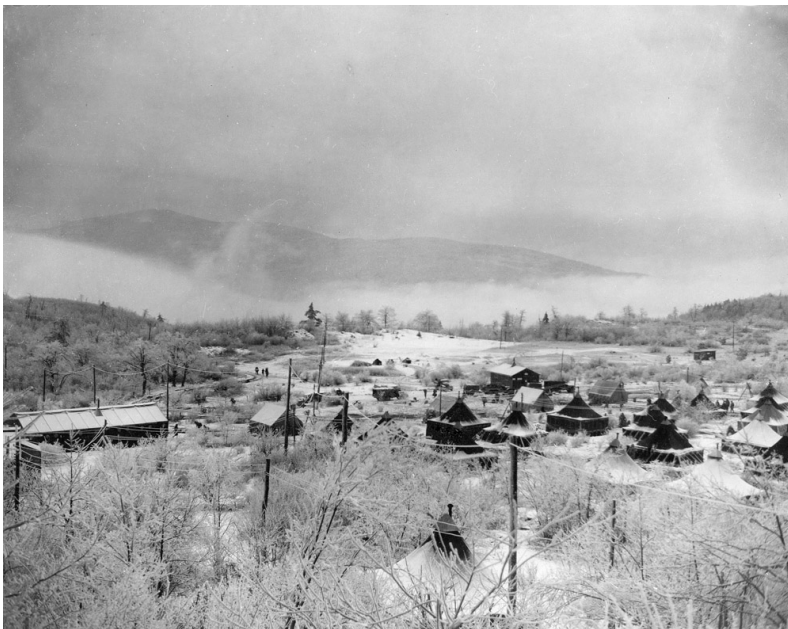
Figure 18. View of camp set up by U.S. Army Corps of Engineers in 1942 for training activities during World War II (Shenandoah NP website).
