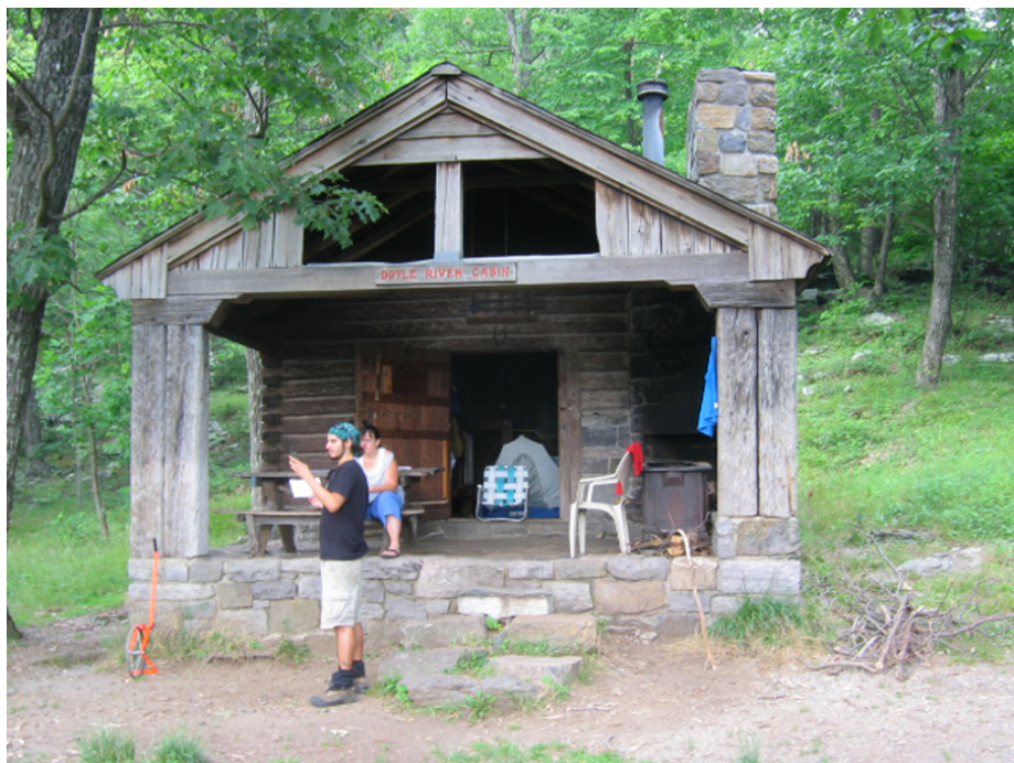
Figure 22: Doyle River Cabin was constructed by the CCC in 1936. It illustrates the NPS Rustic style of using local material and building techniques. (SUNY, 2006)
