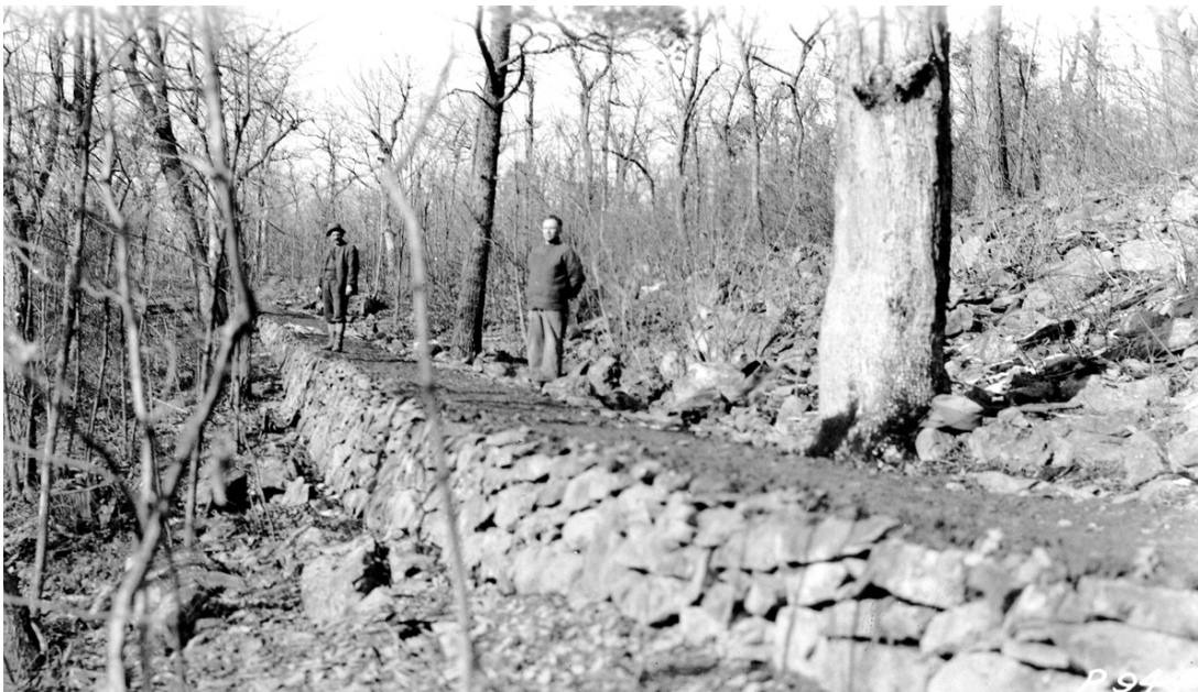
Figure 9: CCC photo of AT near Blackrock, circa 1936, showing incorporation of native vegetation and existing trees. The 42-48 inch wide gravel trail is supported by a stone retaining wall. (Shenandoah NP Archives)
