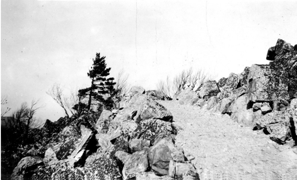
Figure 6: CCC photo showing the completed section of trail along Blackrock, circa 1936. The treadway is evenly graded and surfaced with gravel. The trail width is 42-48 inches with a 3 percent cross pitch. (Shenandoah NP Archives)
