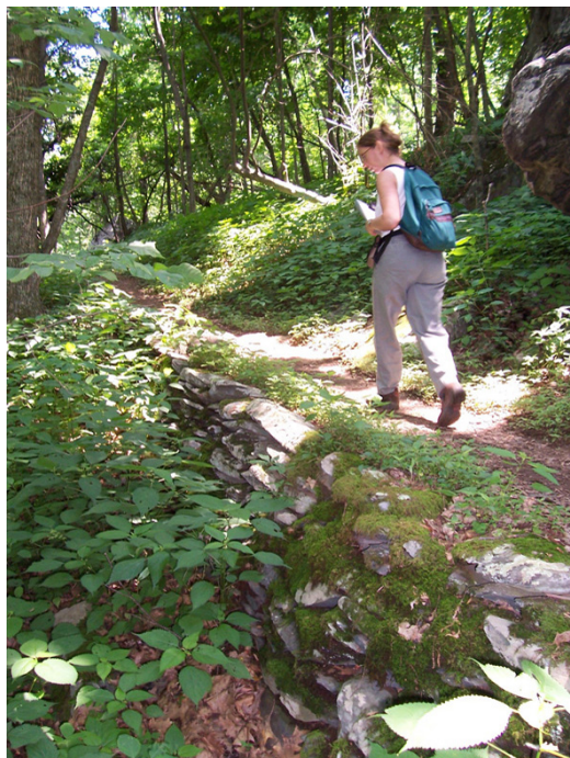
Figure 23: A CCC-built stone retaining wall supports the AT treadway on the way to Hightop. (SUNY, 2006)
