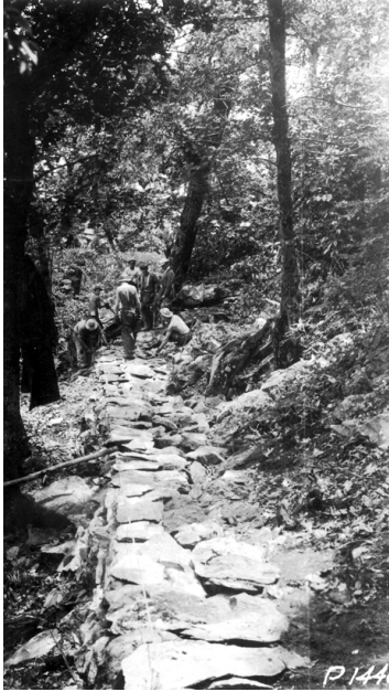
Figure 12: A CCC crew constructing a retaining wall for the AT, which will be surfaced with a gravel walking tread, circa 1935. A string line is used to guide stone placement (location of photograph unknown). (Shenandoah NP Archives)
