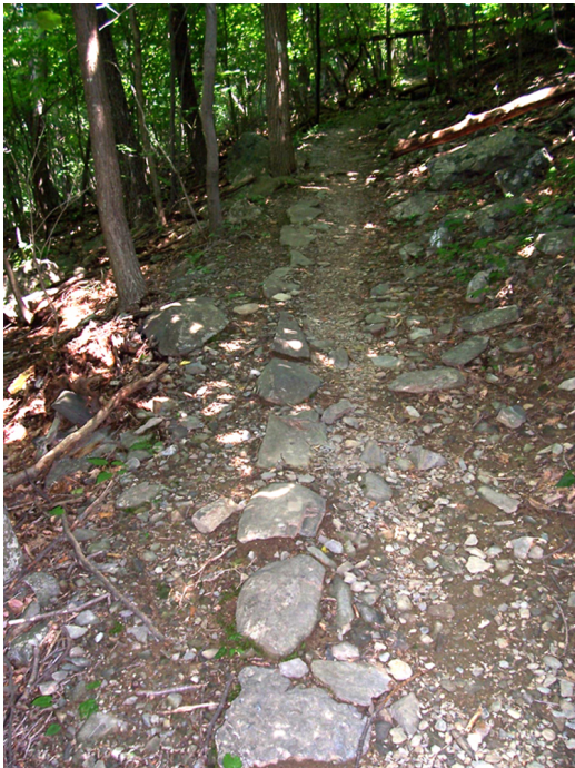
Figure 21: Stone edging still supports the treadway along the AT to Hightop Mountain. The tread surface has lost its top-layered gravel courses. (SUNY, 2006)
