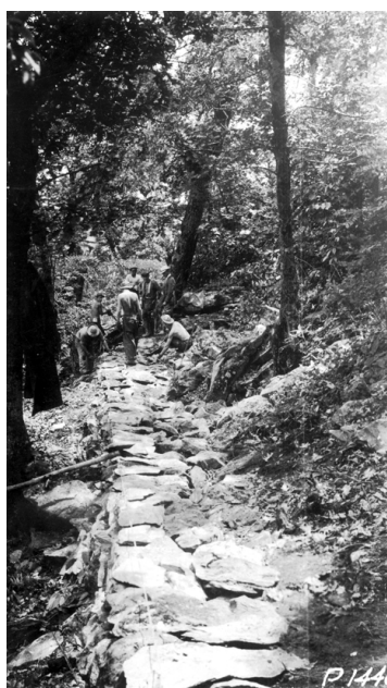
Figure 5: A CCC crew constructing a retaining wall for the AT, which will be surfaced with a gravel walking tread, circa 1935. A string line is used to guide stone placement (location of photo unknown). (Shenandoah NP Archives)
