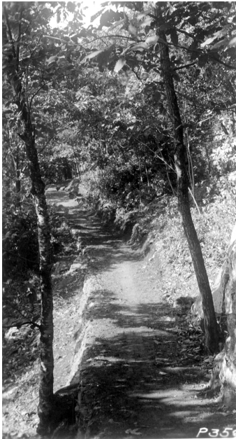
Figure 6: CCC photo showing a completed section of the AT with a bench cut into the natural slope, a lower retaining wall, and graded gravel tread at an even grade and width, circa 1935 (location unknown). (Shenandoah NP Archives)
