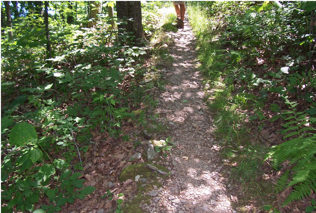
Figure 21: Some sections of stone edging placed along the AT by the CCC to define the trail is disappearing because of erosion and heavy use near Neighbor Mountain Trail. (SUNY, 2006)
