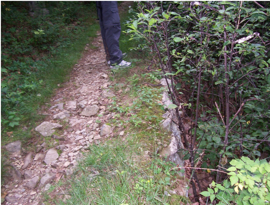
Figure 18: A CCC-built stone retaining wall supports the AT treadway near Compton Peak. (SUNY, 2006)
