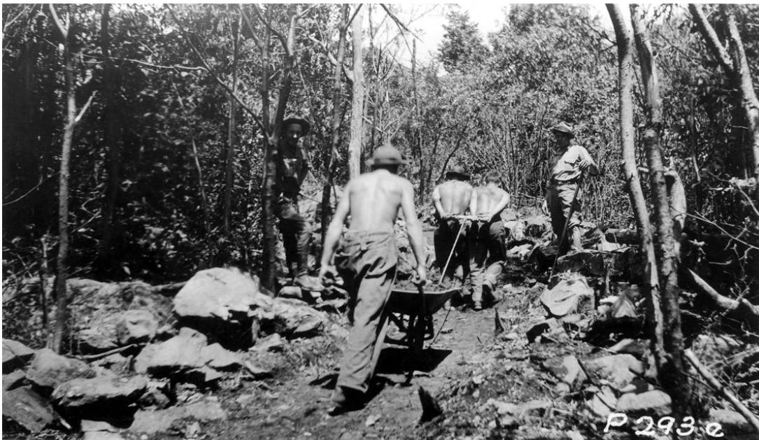
Figure 11: CCC photo showing heavy hauling during the construction of the AT south of Mt. Marshall Trail, circa 1935. The CCC used wheelbarrows to bring in material from borrow pits for surfacing the trail tread. (Shenandoah NP Archives)
