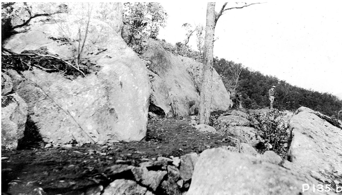
Figure 7: CCC photo showing completed AT to Mary's Rock circa 1935. The trail engages the topography and winds among the rock outcrops. The trail bed is supported by stone edging and low retaining walls. (Shenandoah NP Archives)
