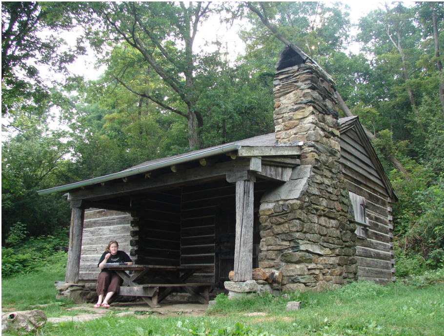
Figure 20: Pocosin Cabin was constructed by the CCC in 1937. It shows the NPS Rustic style of using local material and building techniques. The cabin can accommodate twelve hikers. (SUNY, 2006)
