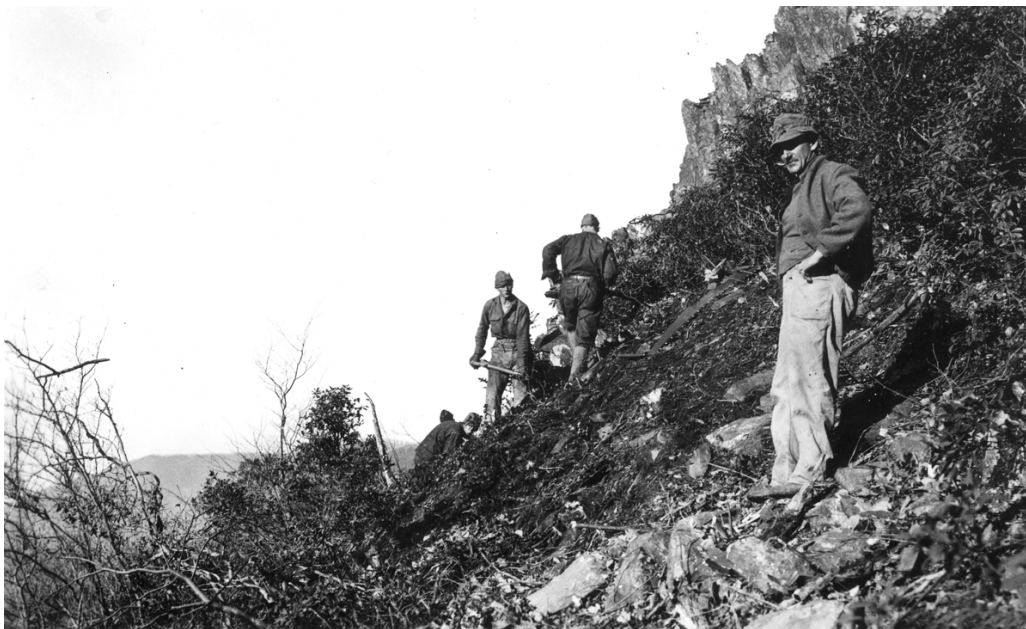
Figure 4: Civilian Conservation Corps (CCC) photo shows men conducting preliminary work on the AT south of Crescent Rock. The trail bed was built out from the steep slope to support the trail circa 1935. (Shenandoah NP Archives)
