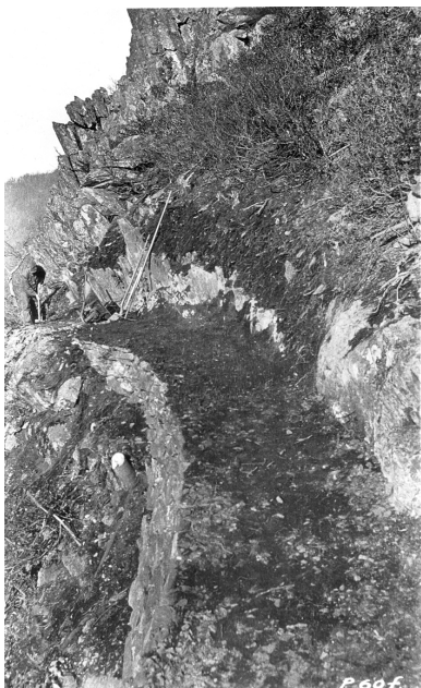
Figure 5: Mid-construction of the AT south of Crescent Rock. The trail bed was cut out of the slope and built up from below with retaining walls. (Shenandoah NP Archives)
