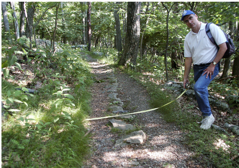
Figure 17: The CCC-graded trail has eroded and not retained the three-percent cross pitch. The trail has migrated and the stone edging that once supported the treadway now appears to bisect the trail. (SUNY, 2006)
