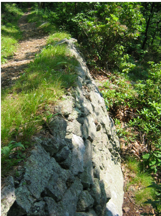
Figure 21: A CCC-built stone retaining wall supports the AT treadway near Spitler Knoll. (SUNY, 2006)
