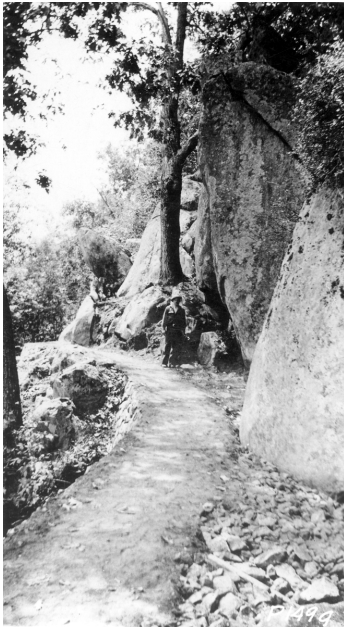
Figure 8: CCC photo showing completed AT to Mary's Rock, circa 1935. The trail has a width of 42-48 inches, is surfaced with gravel, and is supported by a stone retaining wall. (Shenandoah NP Archives)
