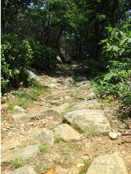
Figure 19: Stone edging still supports the treadway along the AT to Mary's Rock. The tread surface has lost its top-layered gravel courses. (SUNY, 2006)
