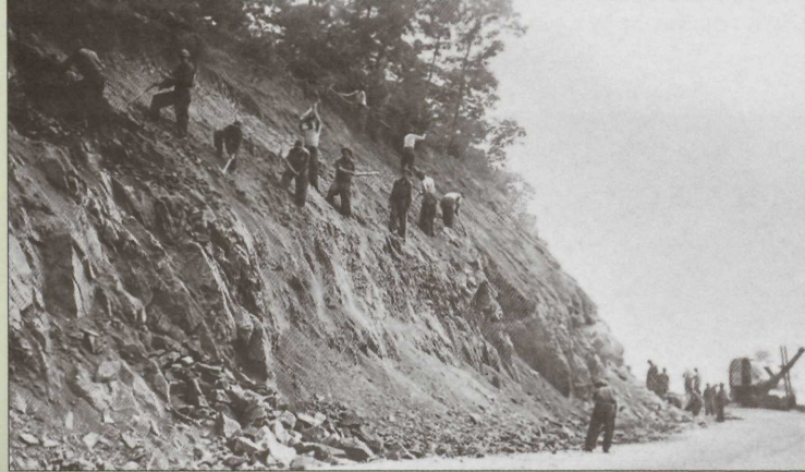
CCC workers build erosion controls along Skyline Drive.
