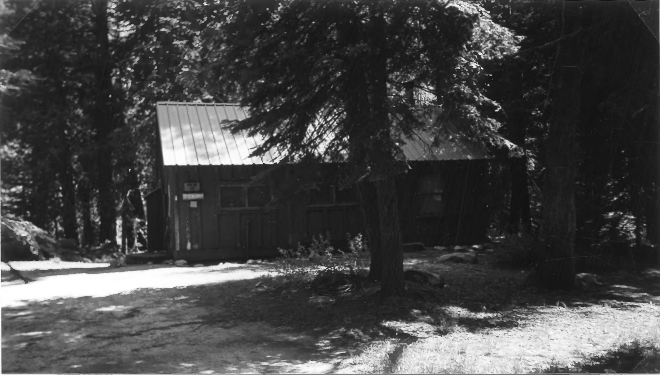
Figure 9 Cabin with Vertical Board-And-Batten Siding, West Mineral King
