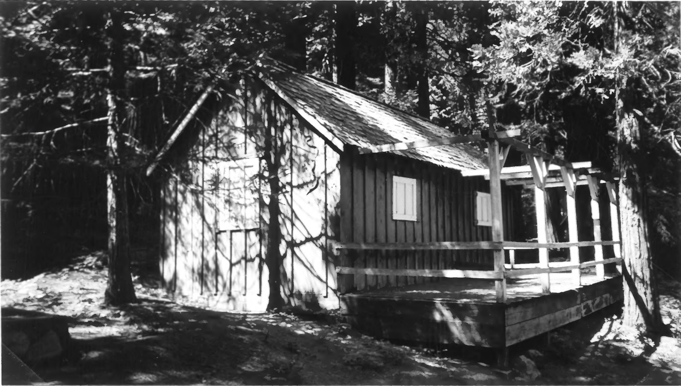
Figure 6 Rustic Cabin with Vertical Board-And-Batten Siding, Cabin Cove
