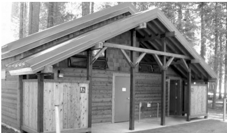
Picnic area restroom built with fee dollars.
