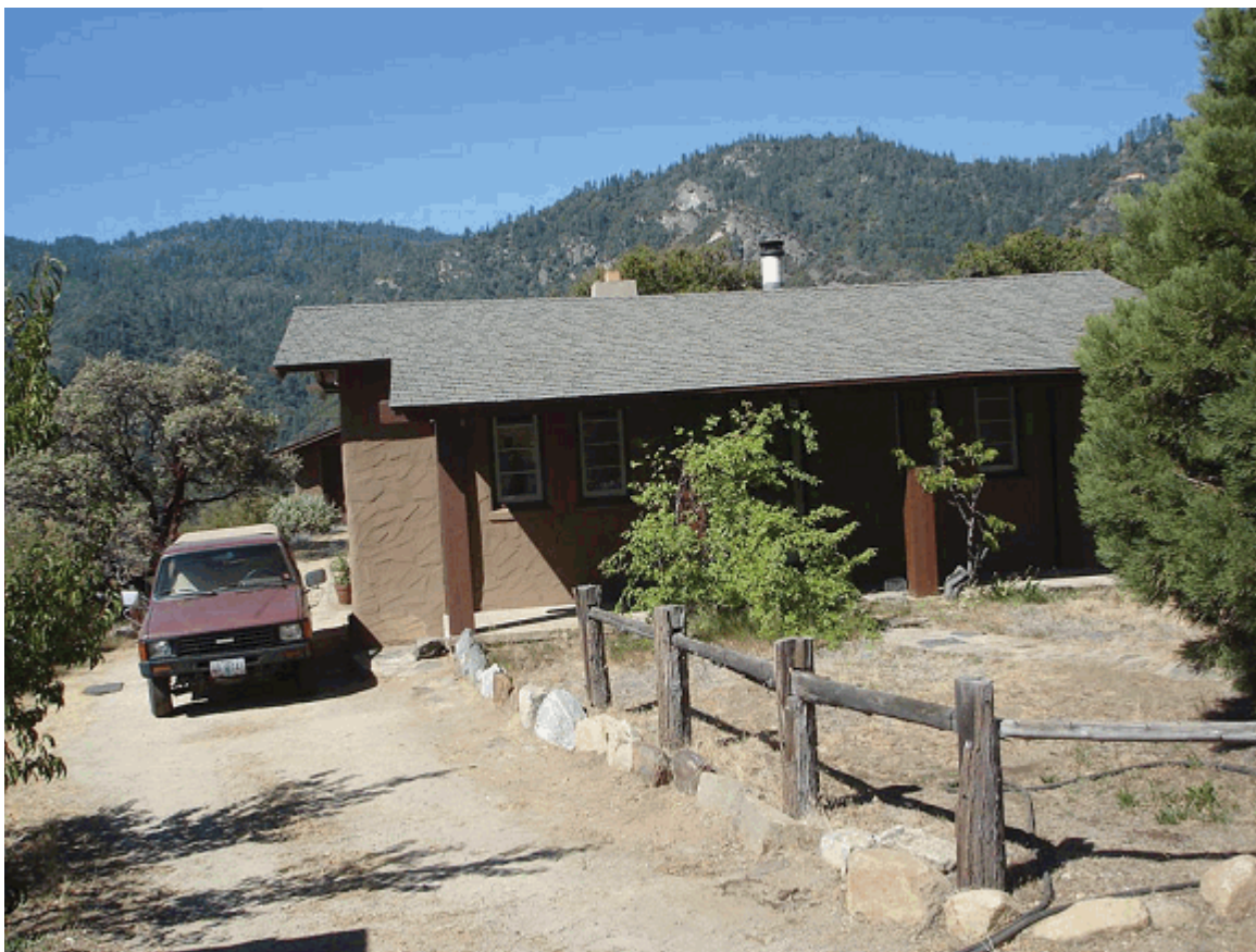
Buildings and Structures #1: CCC-constructed Lookout Point Ranger Station (1936), facing southwest. Both the ranger station (foreground) and the garage (background) were built out of adobe. (SEKI, 2008)
